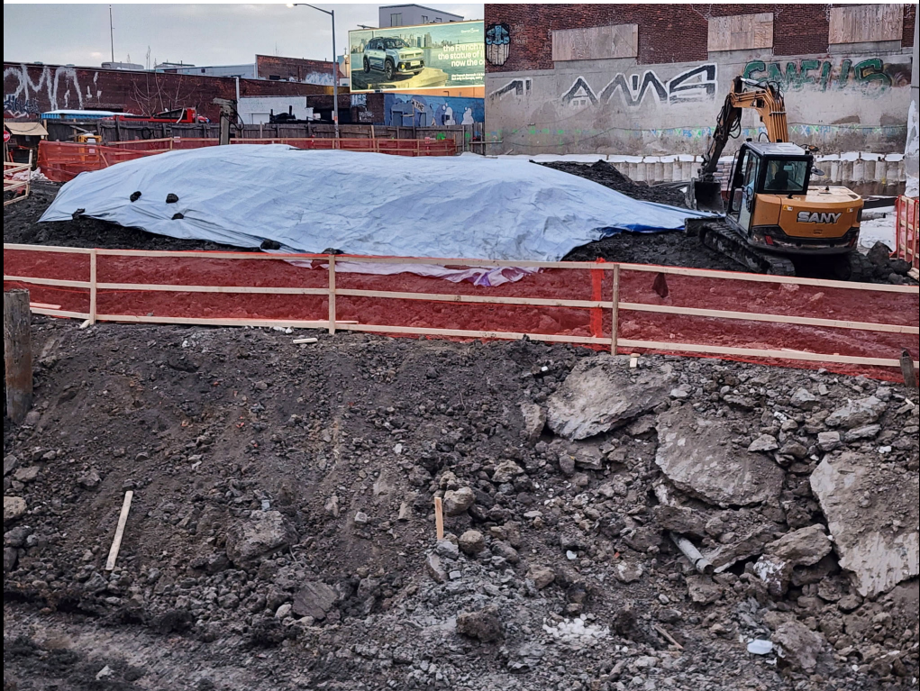
Photo 2: View of stockpiled soil being covered at the end of the work day.
