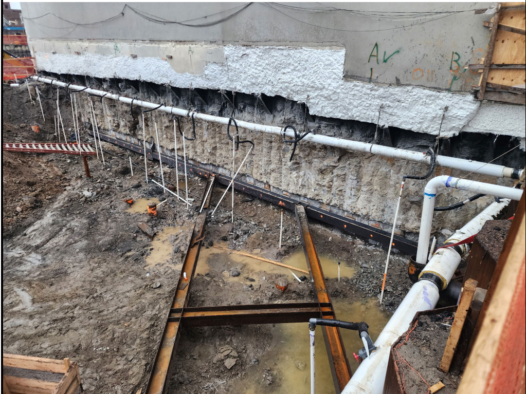
Photo 2: View of dewatering header pipe following installation.
