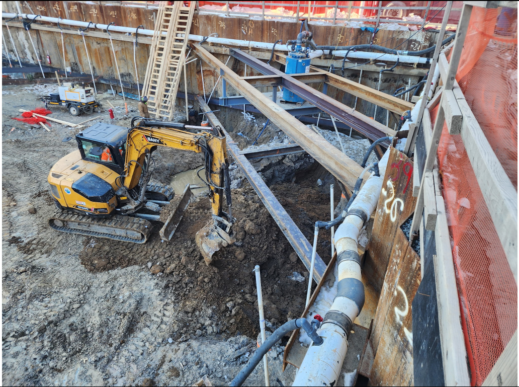
Photo 2: View of excavation for SOE.
