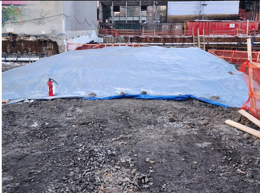
Photo 1: View of a covered soil stockpile awaiting offsite disposal.
