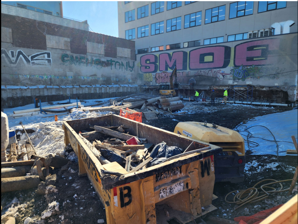
Photo 2: View of concrete removal along adjacent building's foundation.
