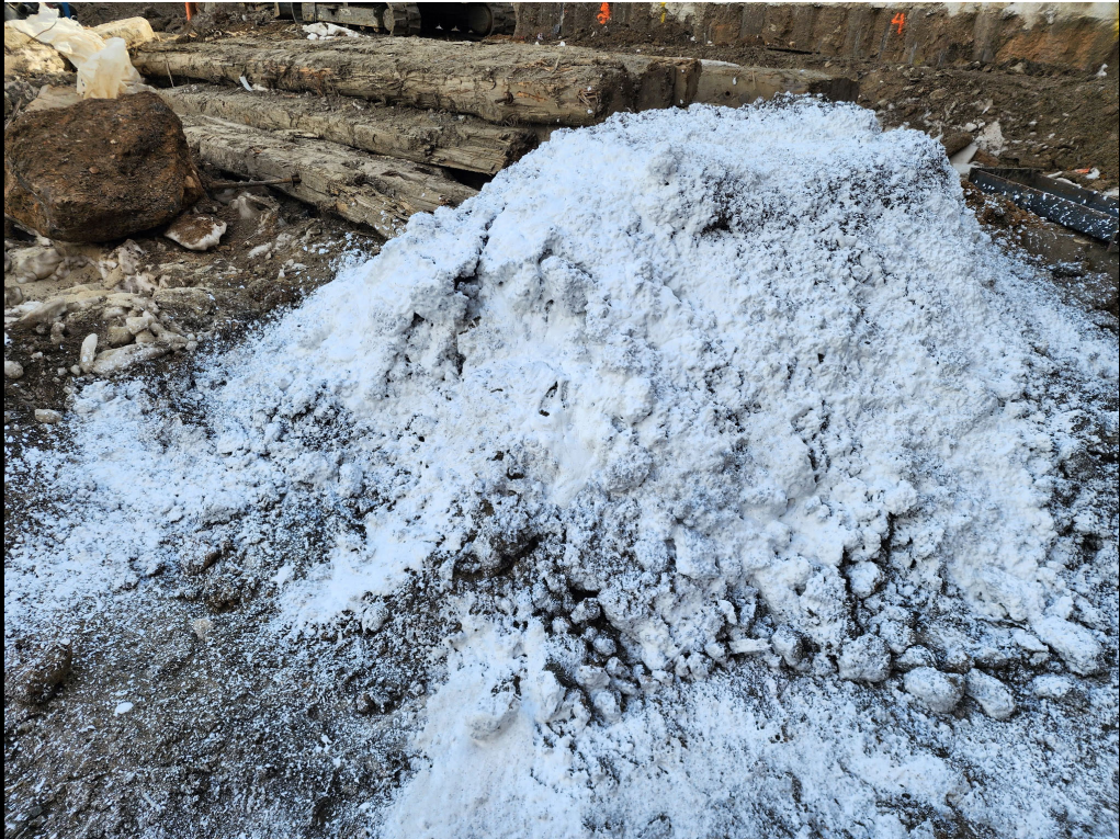
Photo 2: View of a soil stockpile covered with foam.
