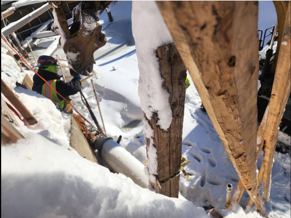
Photo 2: View of dewatering header pipe adjustments.
