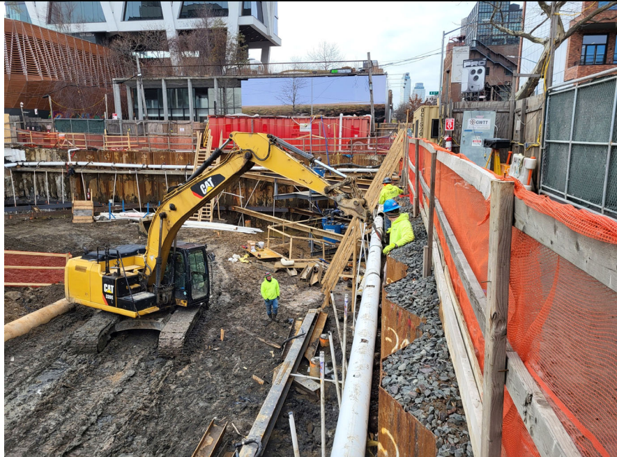
Photo 1: View of dewatering system header pipe installation.
