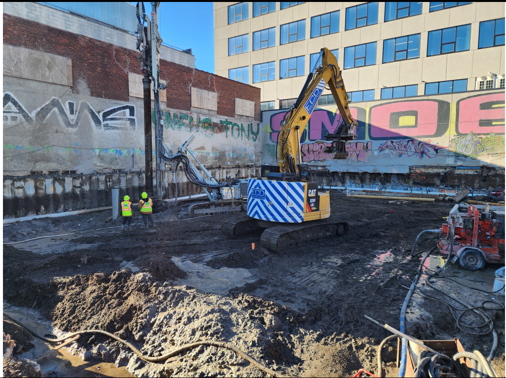
Photo 2: View of pile installation.
