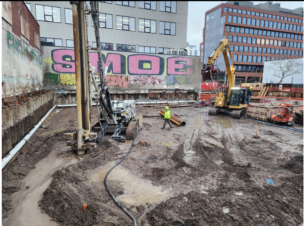
Photo 2: View of pile installation.
