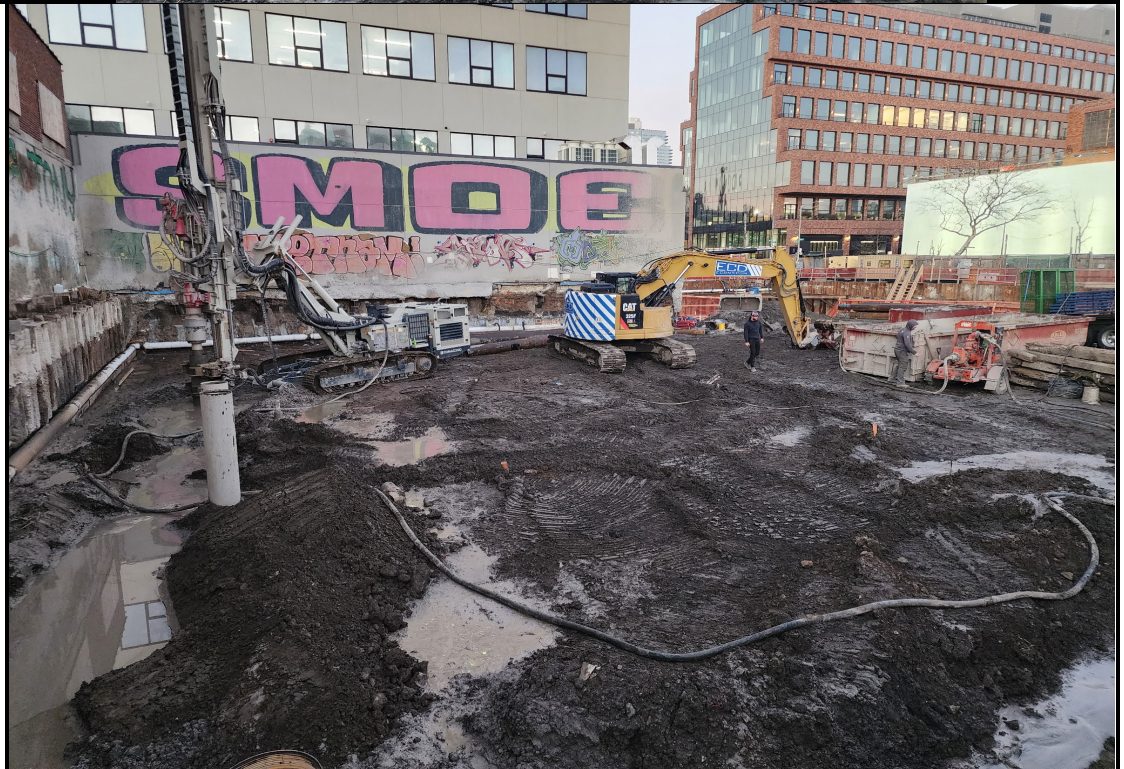
Photo 2: View of pile installation.
