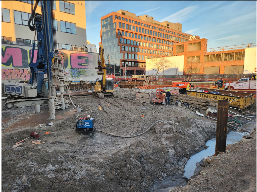
Photo 2: View of pile installation.
