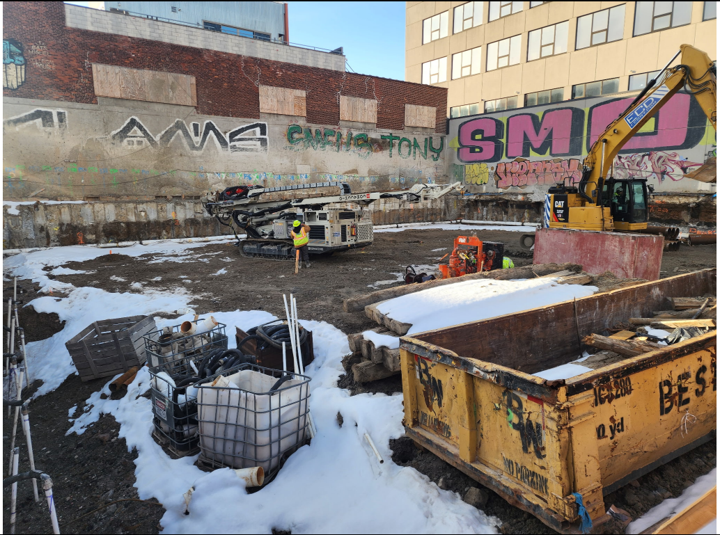
Photo 2: View of drill mobilized on-site.
