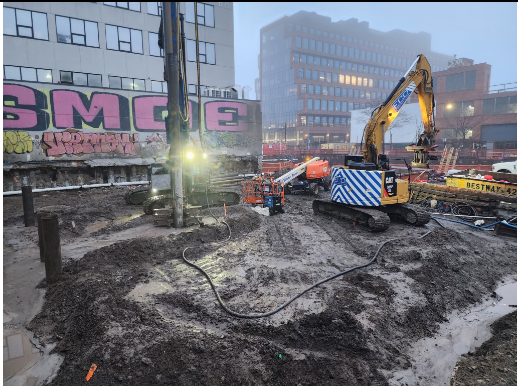
Photo 2: View of pile installation.
