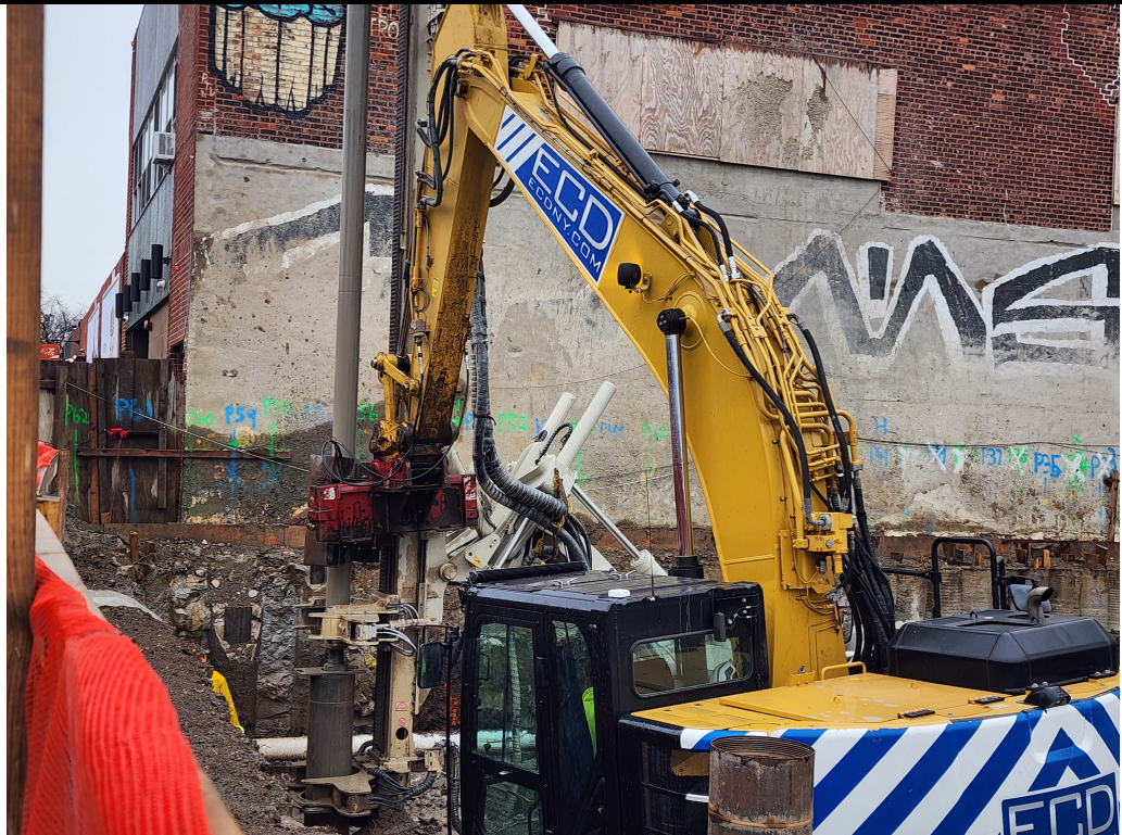
Photo 2: View of pile installation.
