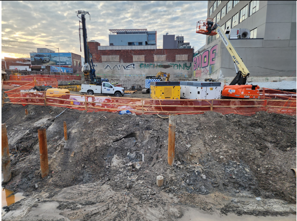
Photo 2: View of pile installation activities.
