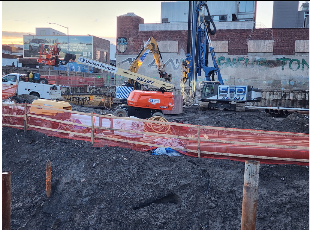
Photo 2: View of pile installation.
