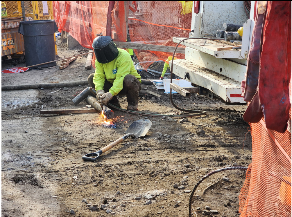
Photo 2: View of welding work.
