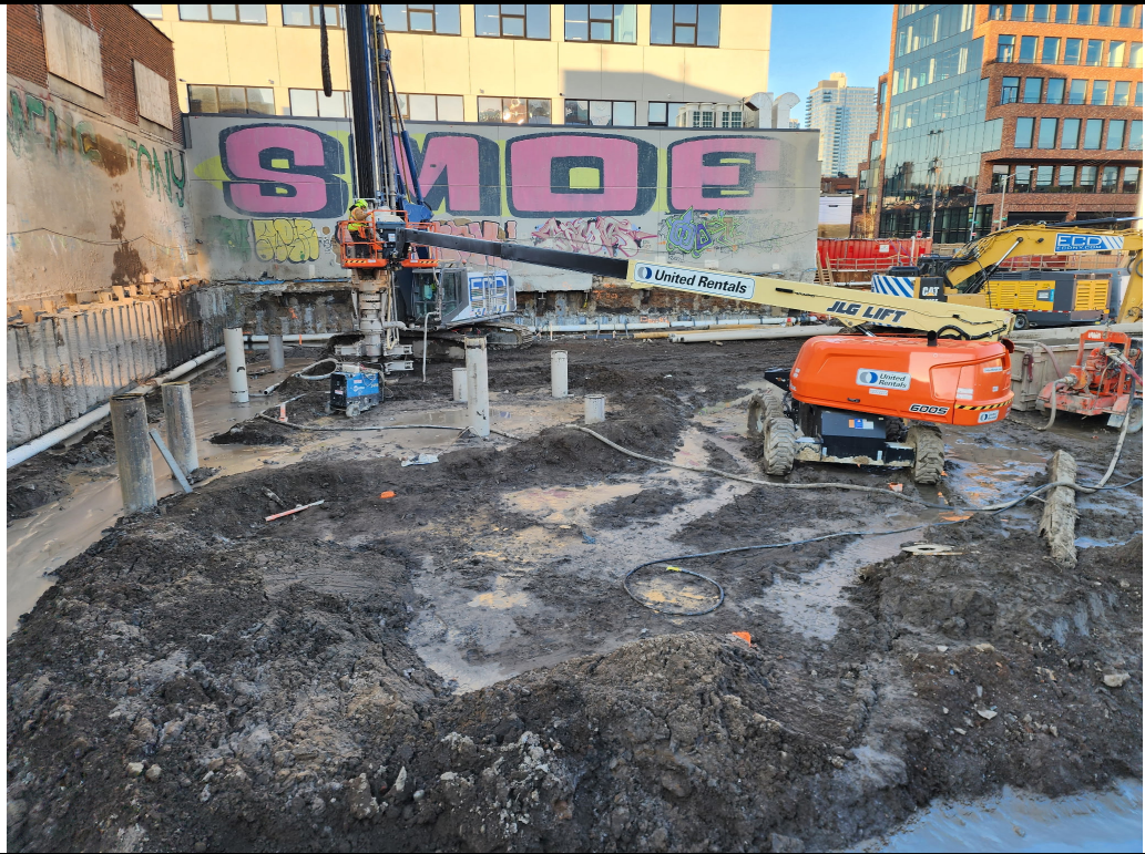
Photo 2: View of pile installation.
