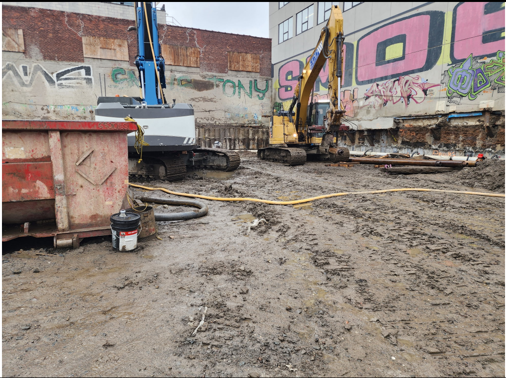
Photo 2: View of pile installation.
