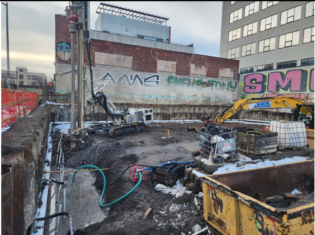
Photo 2: View of pile installation.
