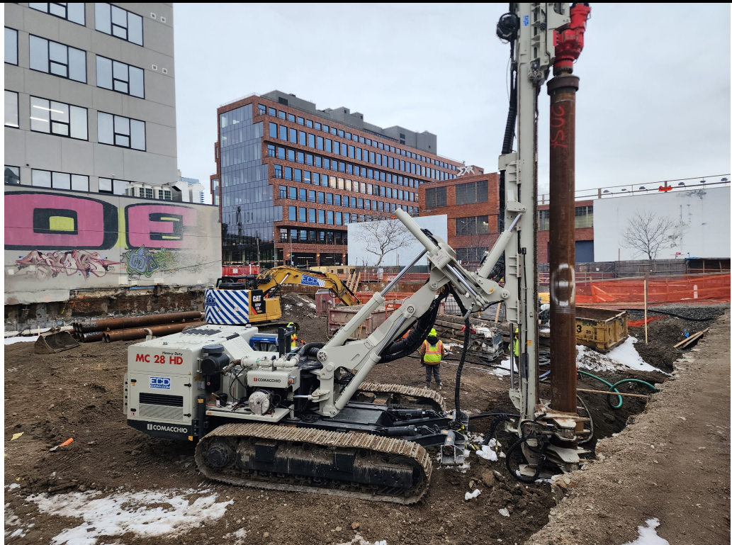
Photo 2: View of pile installation.
