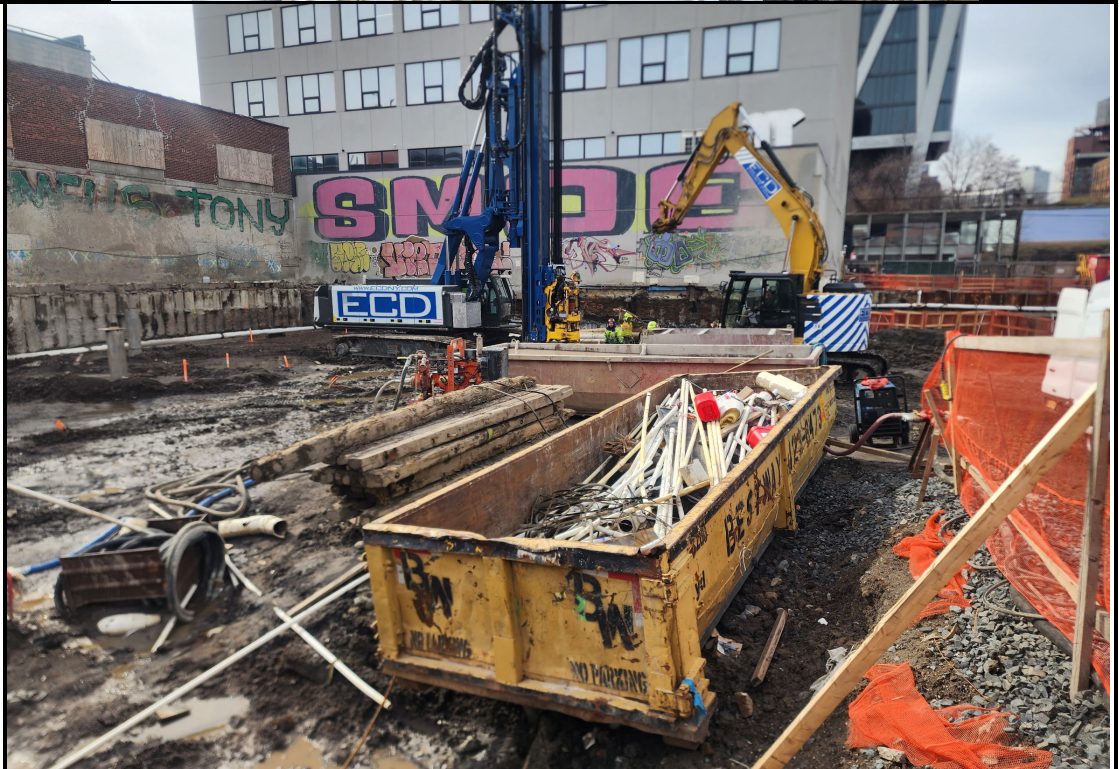
Photo 2: View of equipment mobilization.
