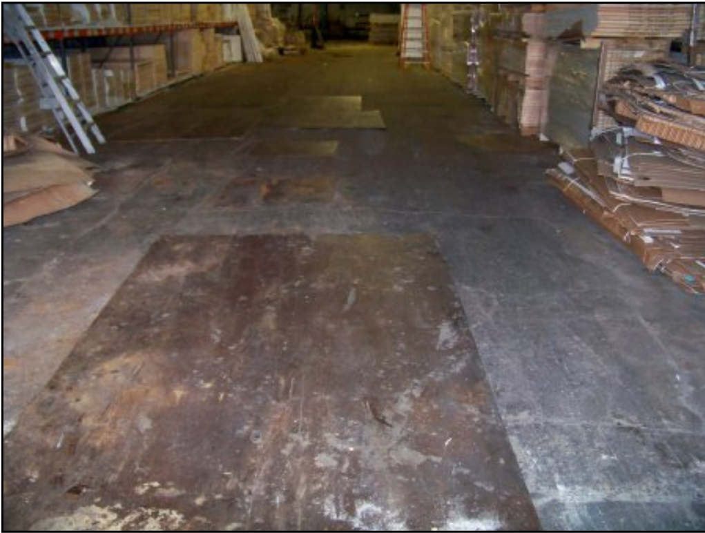
Facing south, looking at steel plates on floor within Lot 48 warehouse for 'Exclusive Doors and Moldings' to cover up broken up concrete floors for the forklifts.
