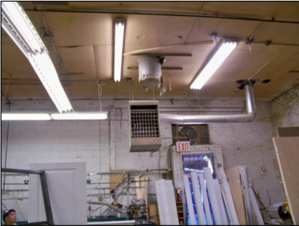
Facing south, looking at overhead natural gas heaters within 'Exclusive Doors and Moldings' warehouse.
