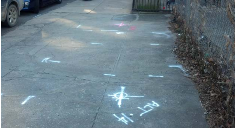
Photograph 9. View of soil boring locations TRC-SB-14 and TRC-SB-15 marked out on the 8 th Street sidewalk.
