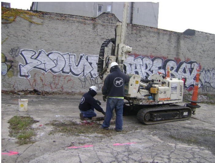
Photograph 3. View of soil boring installation at TRC-SB-10.
