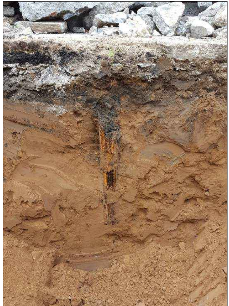
Looking northwest at clean soils at a shallow depth (2 to 3 feet) 5 beneath the two concrete slabs in Trench 4.
