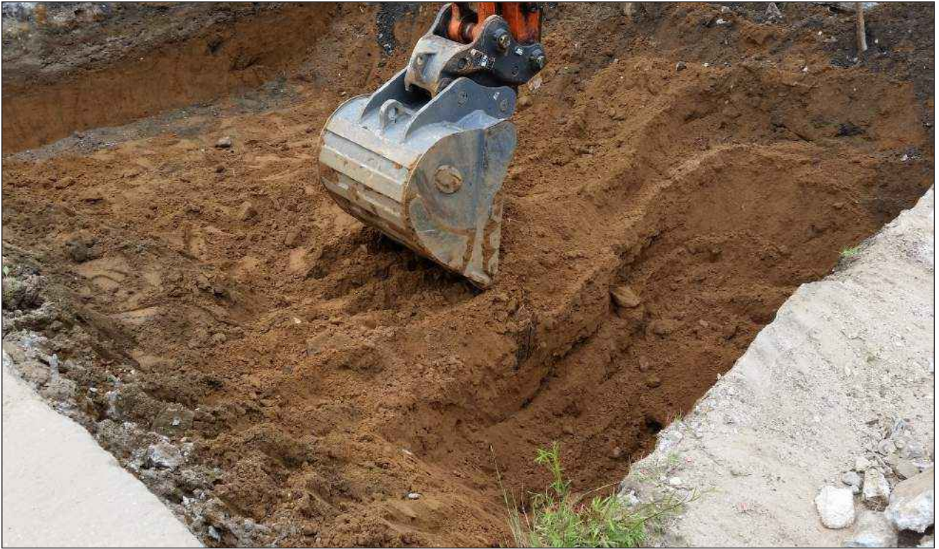
Looking northwest at clean soils at a shallow depth (2 to 3 feet) 5 beneath the two concrete slabs in Trench 4.
