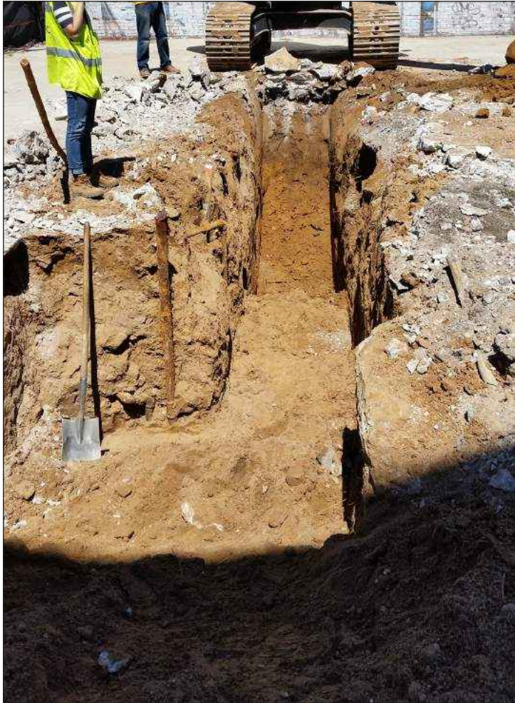
Looking west at Trench 8; the pipes at left lead to at least two buried gasoline tanks and the lighter soil in the background appears to be clean subsoil. 11
