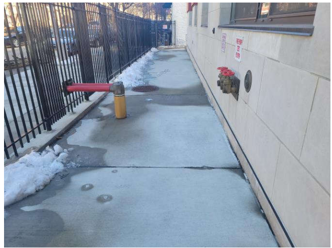
Photo 8. View of concrete walkway cover system along 8 th Street.
