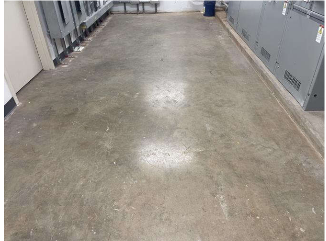
Photo 8. View of a typical bare concrete floor in Room C002.
