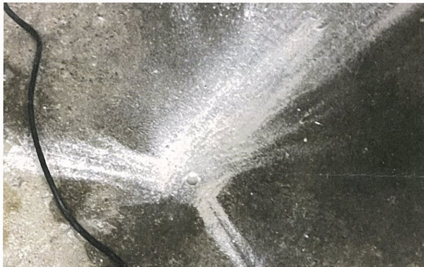
Image 1: View of an example of sub-slab soil for sampling drill hole.
