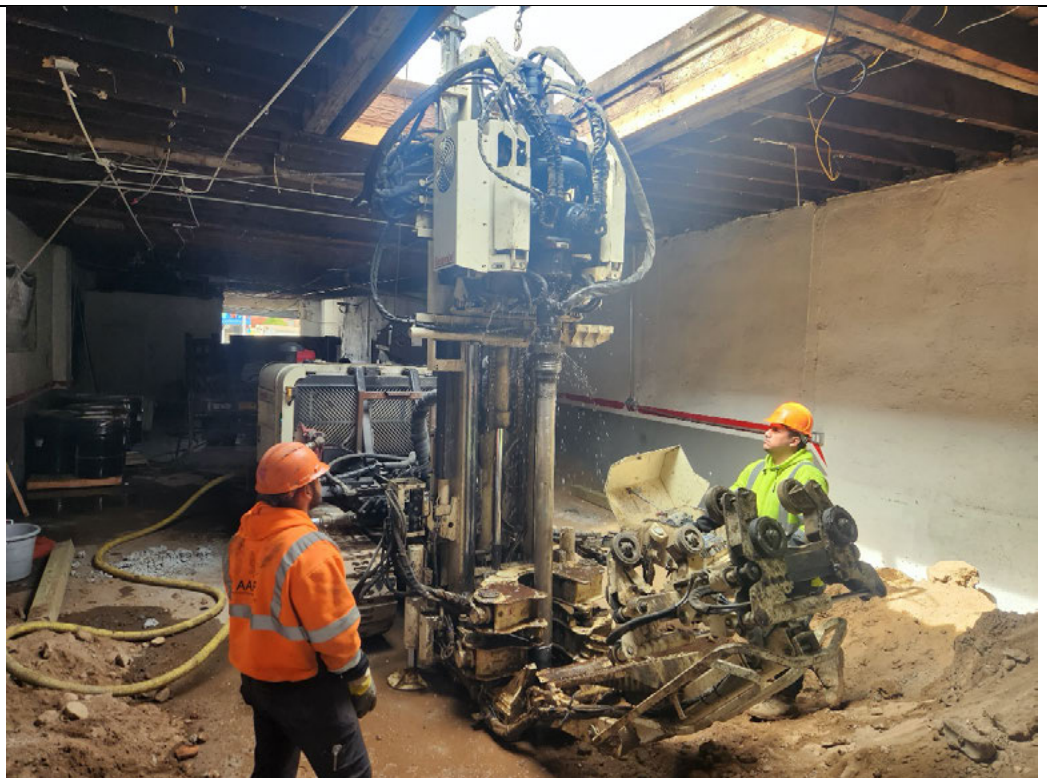
Photo 3 – View of work area.
