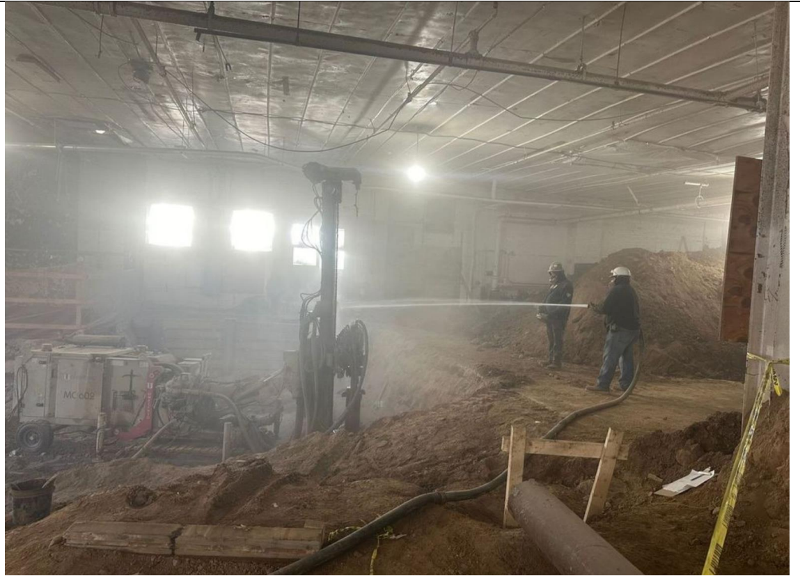
Photo 1 – View of pile installation and use of water as dust suppressant.
