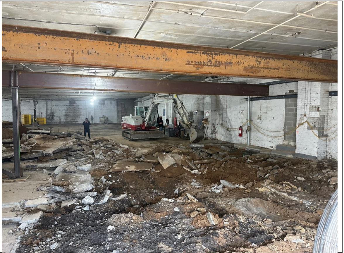
Photo 3 – View of demolition of concrete building slab.
