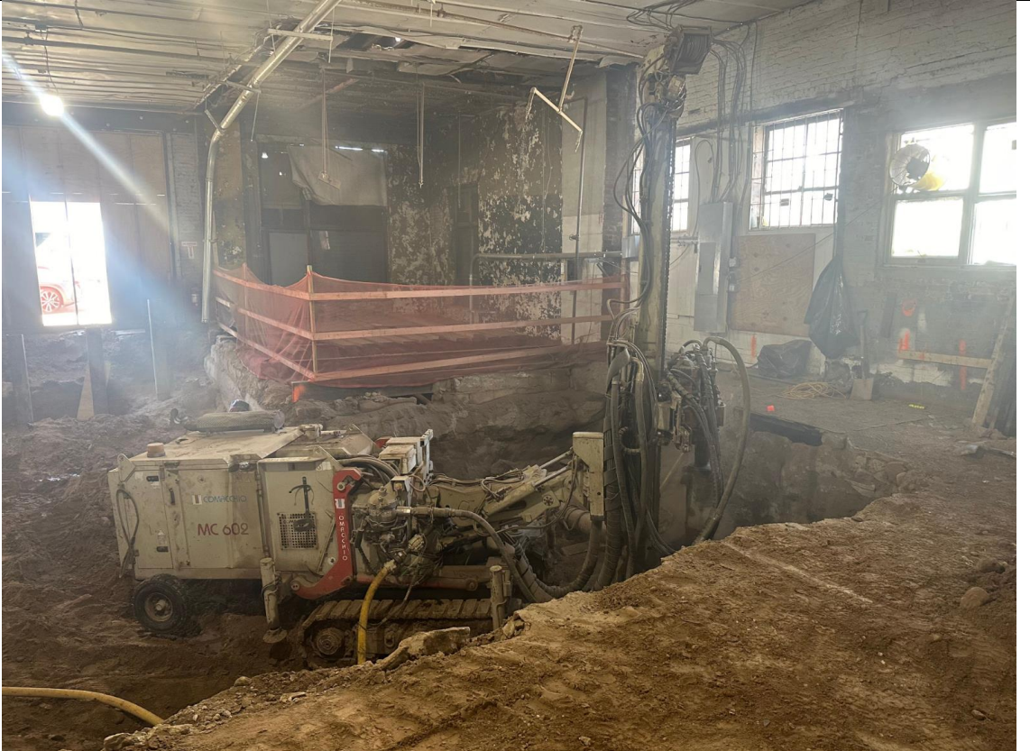
Photo 2 – View of pile installation.
