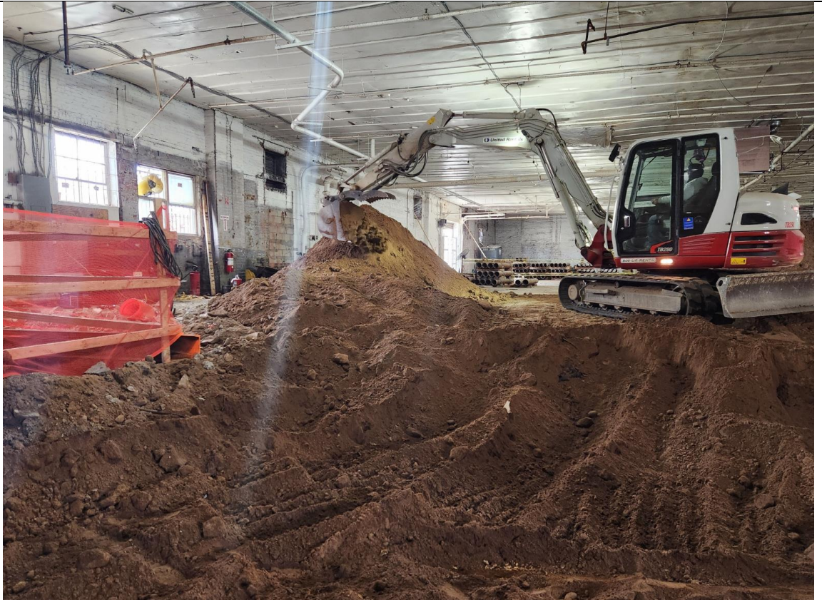
Photo 1 – View of soil excavation.
