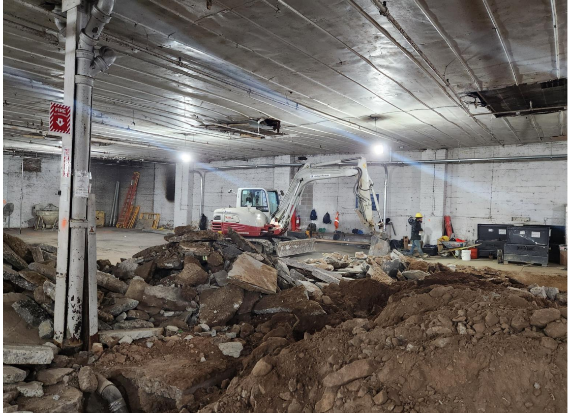
Photo 2 – View of concrete slab demolition for off-site disposal.
