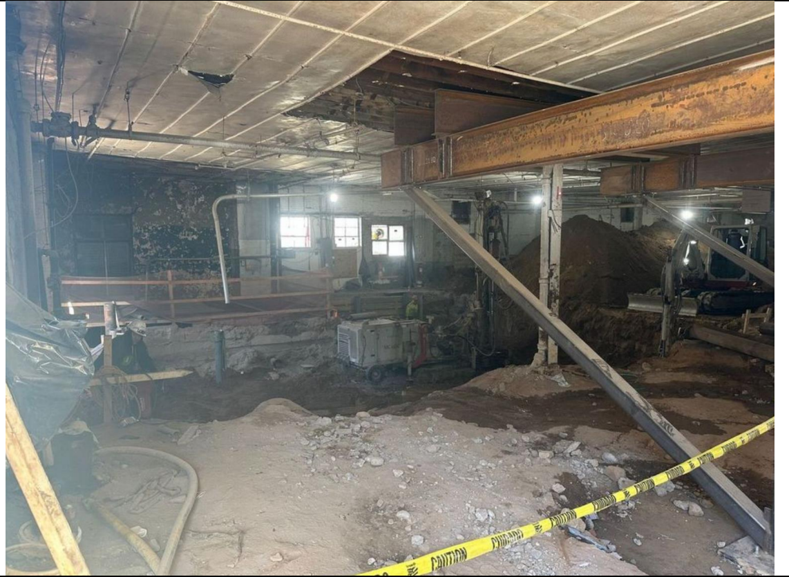
Photo 3 – View of soil stockpiling and pile installation.
