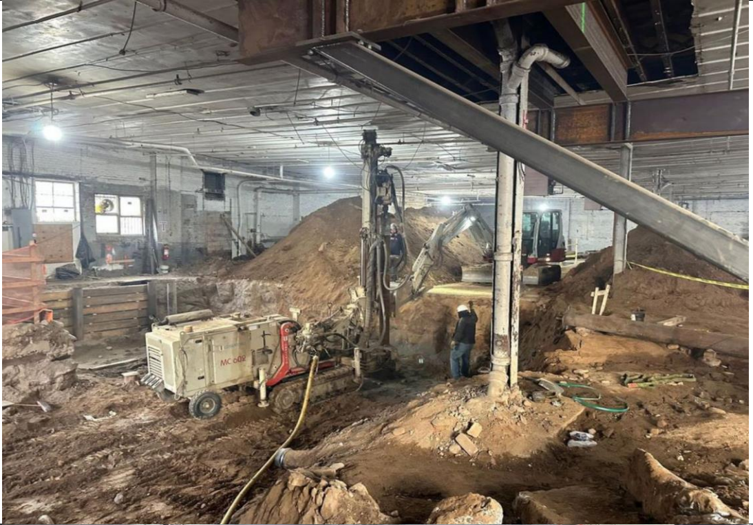
Photo 1 – View of pile installation and soil excavation.
