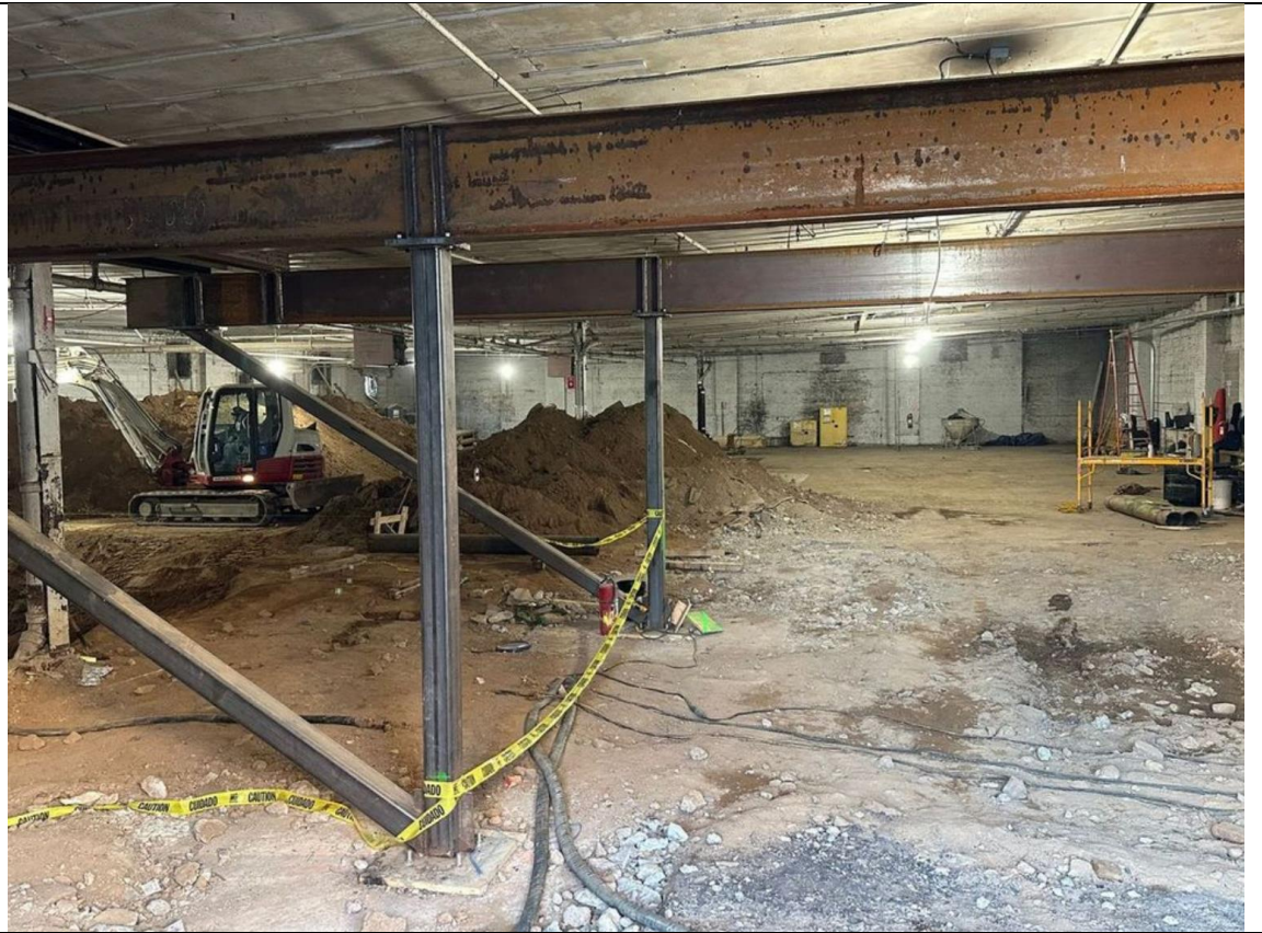
Photo 3 – View of soil stockpiling.
