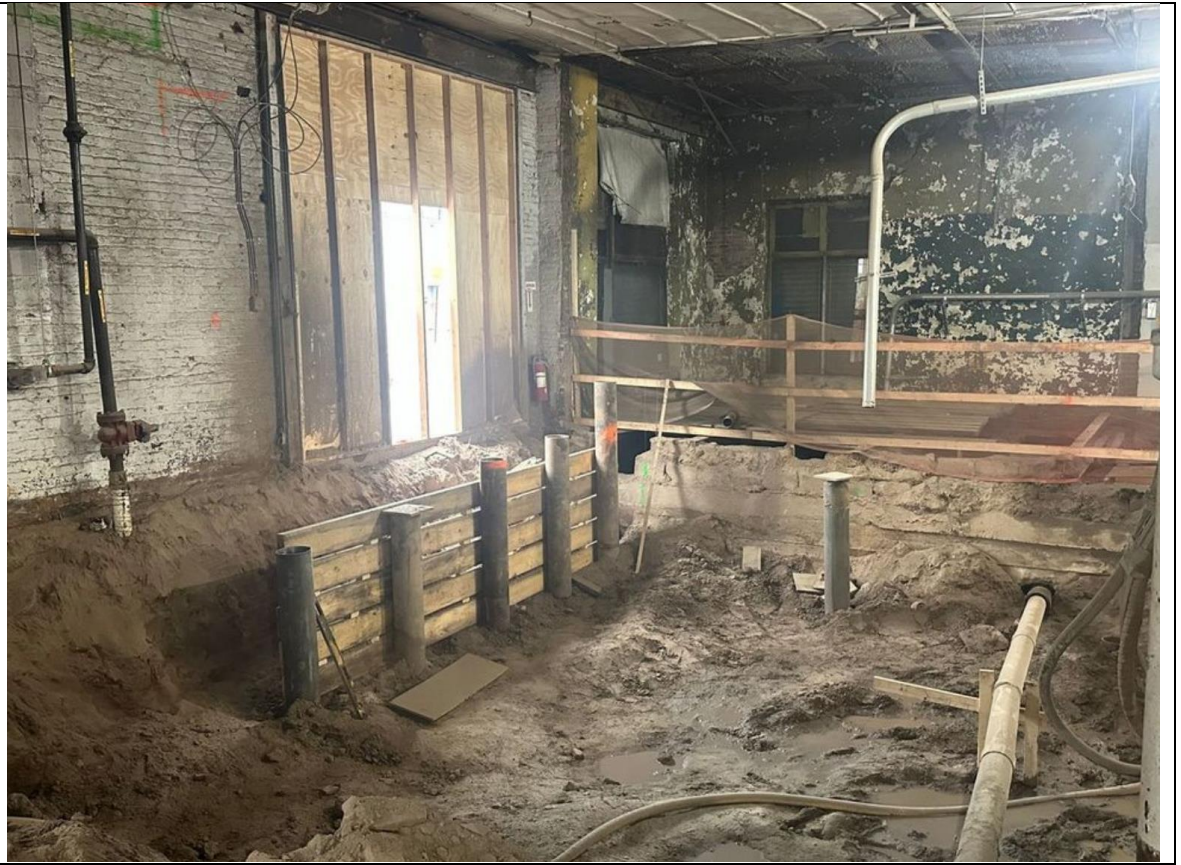
Photo 3 – View of support of excavation.
