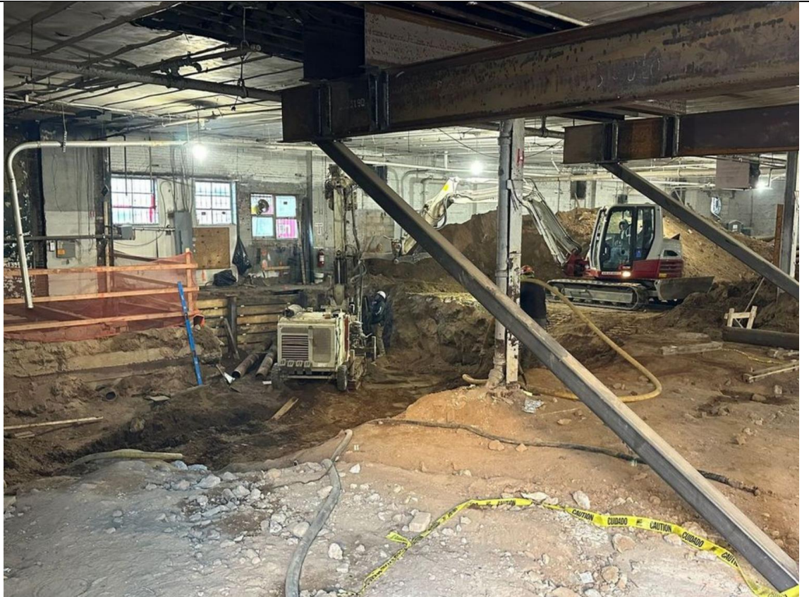
Photo 1 – View of Site conditions and pile installation.
