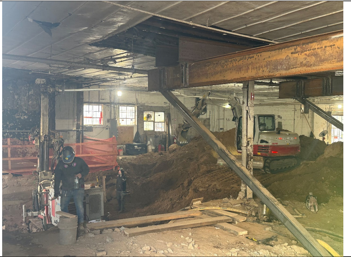
Photo 3 – View of the Site at the end of the work day.
