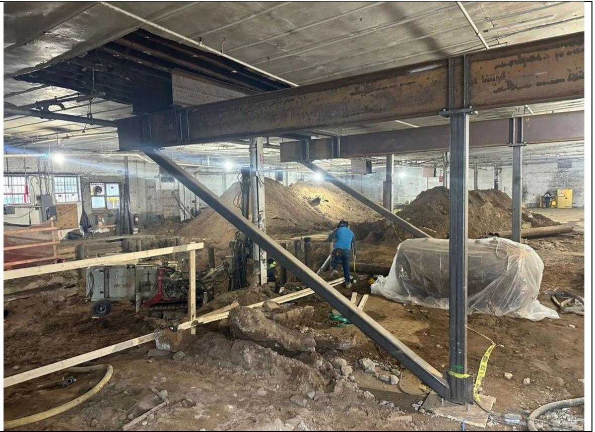
Photo 3 – View of soil stockpiles and Site conditions.
