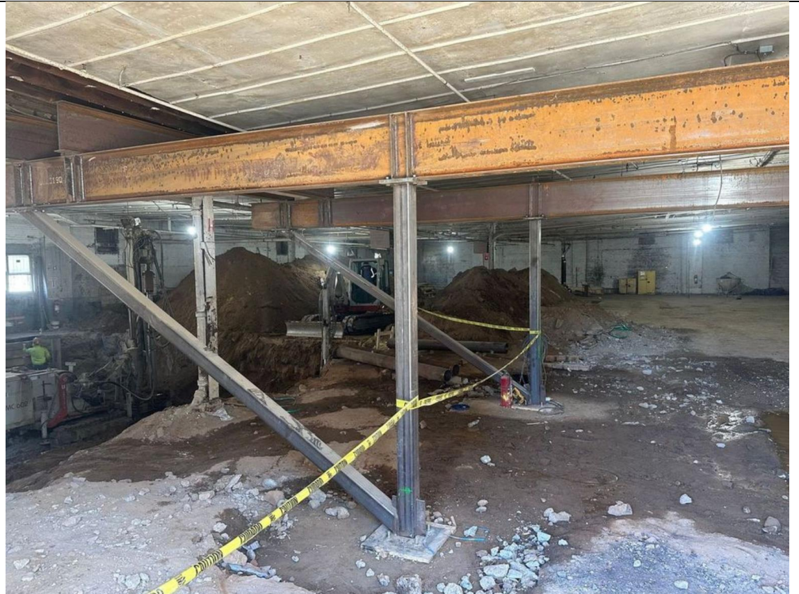
Photo 2 – View of site conditions and soil stockpiles.
