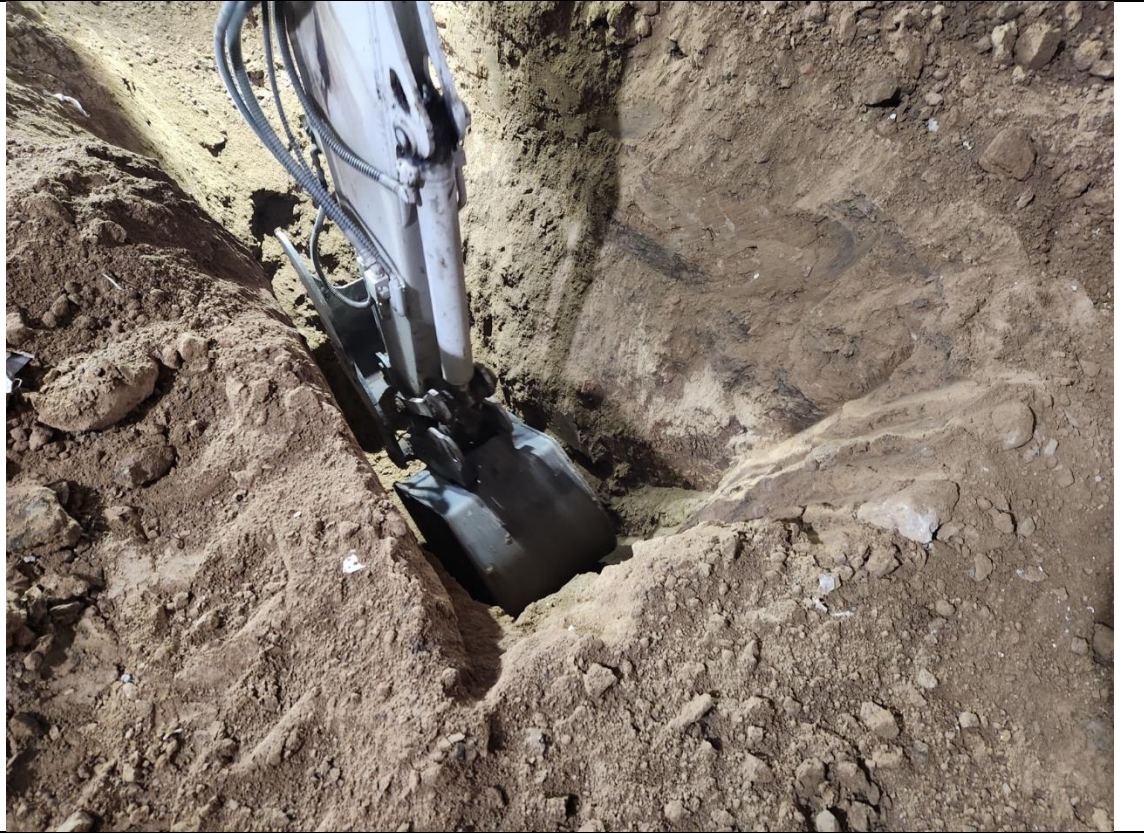
Photo 3 – View of excavation for waste characterization sampling.
