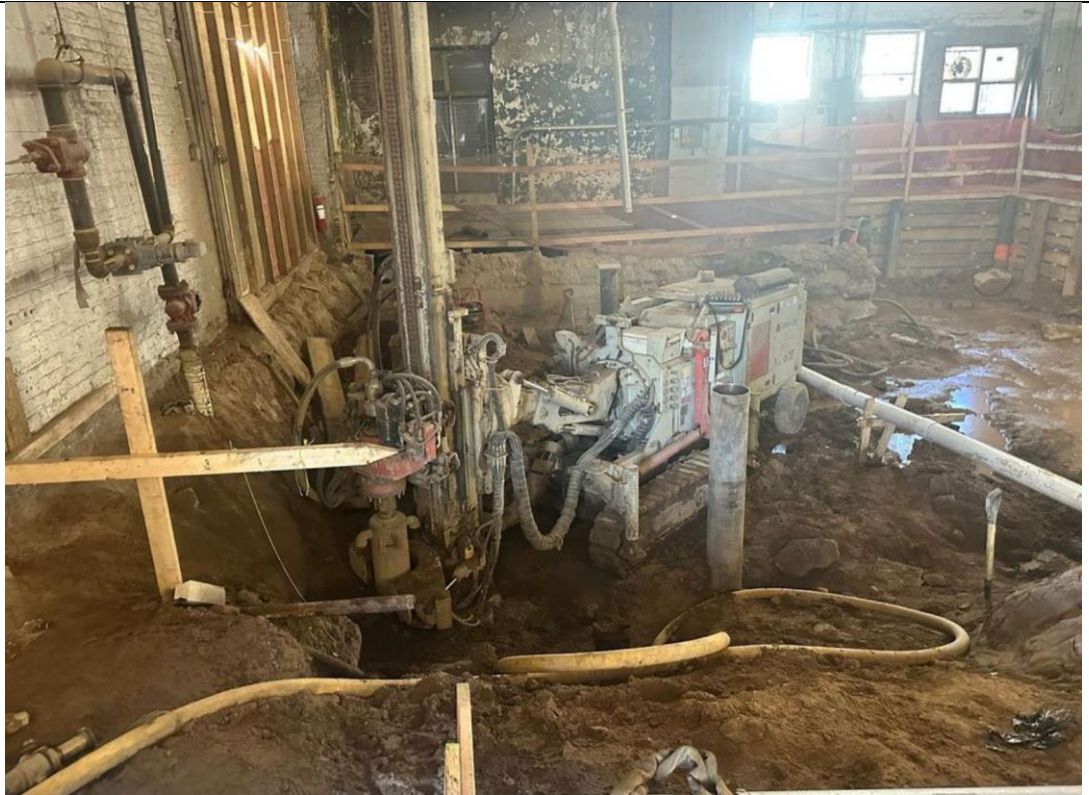
Photo 1 – View of pile installation for support of excavation.
