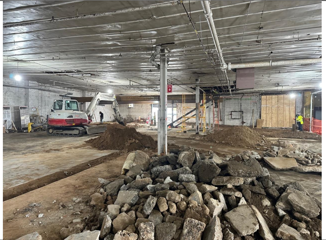
Photo 2 – View of soil and concrete stockpiles.
