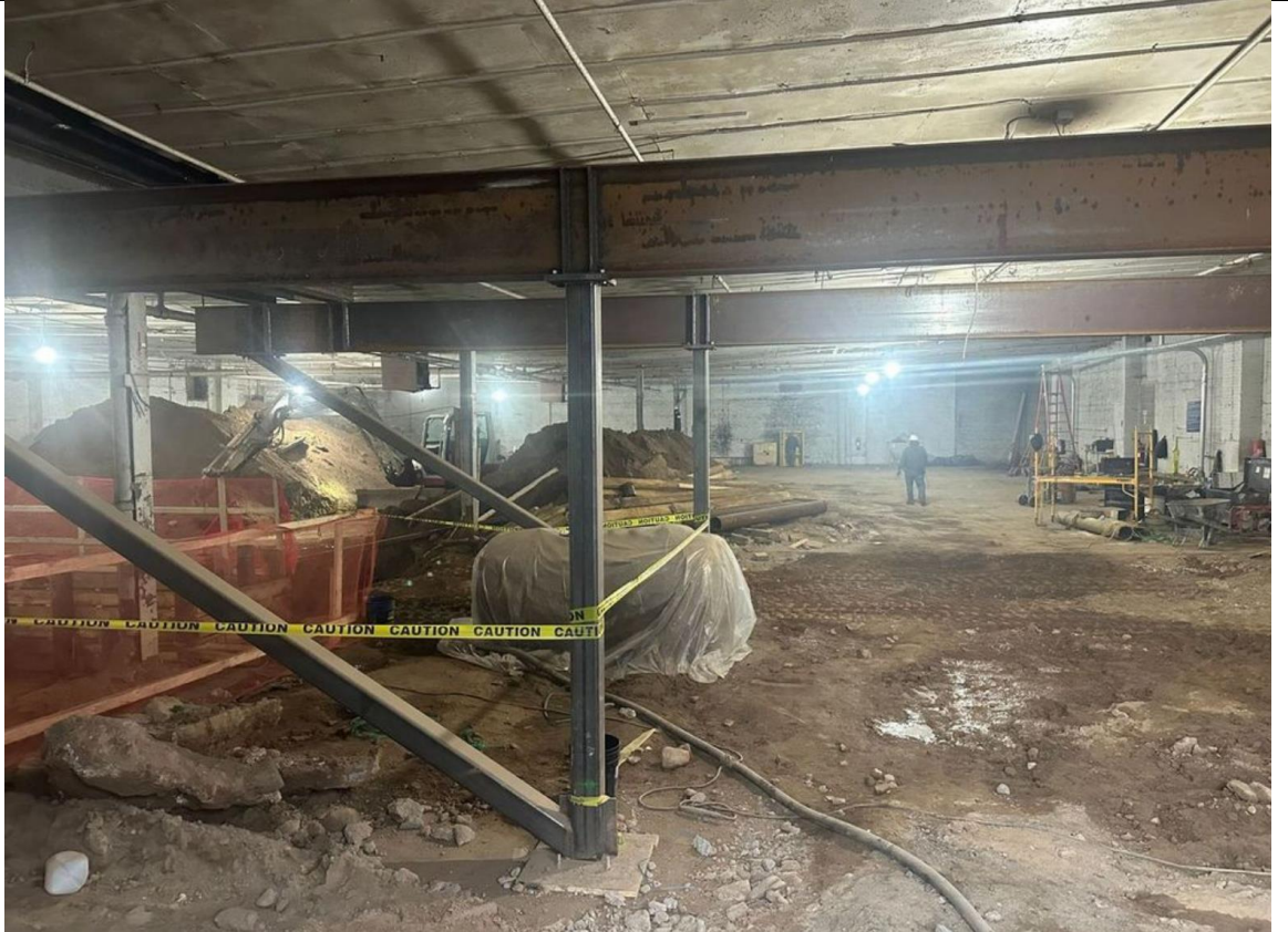
Photo 2 – View of Site conditions and soil stockpiles.
