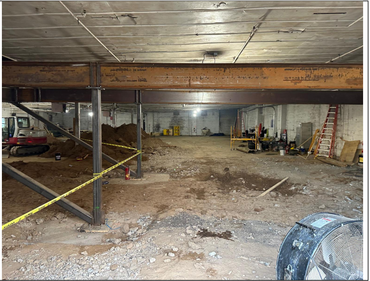
Photo 3 – View of soil stockpiling.
