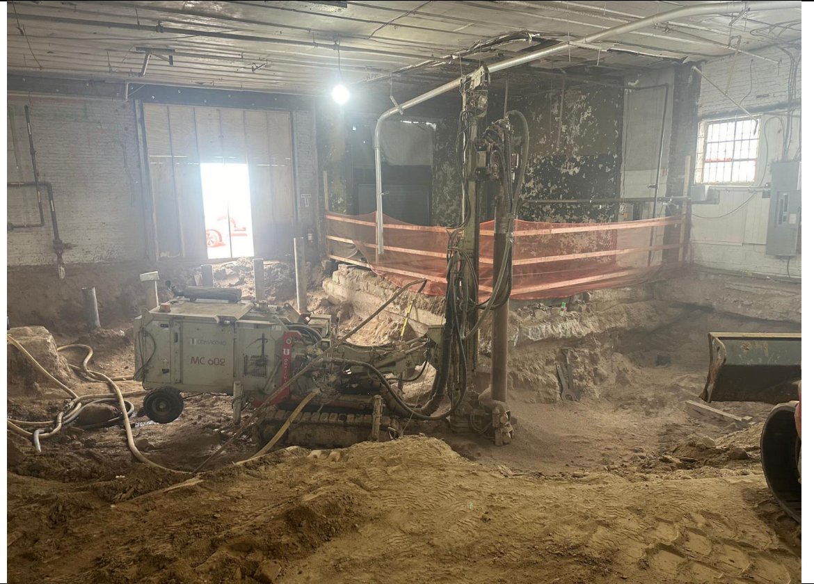
Photo 2 – View of pile installation.
