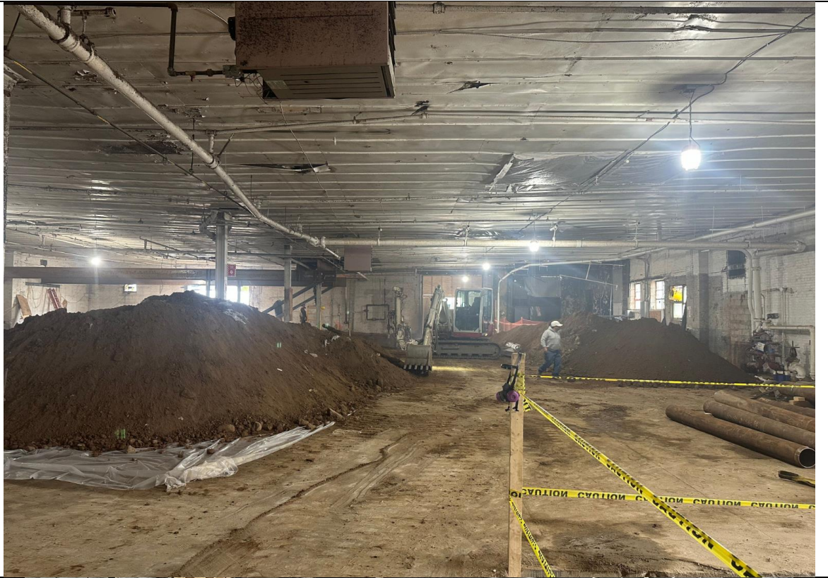
Photo 1 – View of soil excavation and stockpiling.
