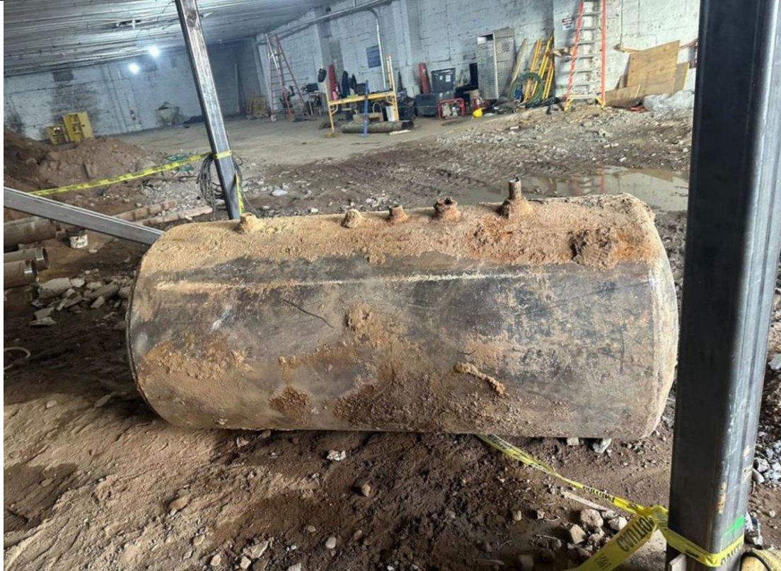
Photo 2 – View of a tank removed from the ground.
