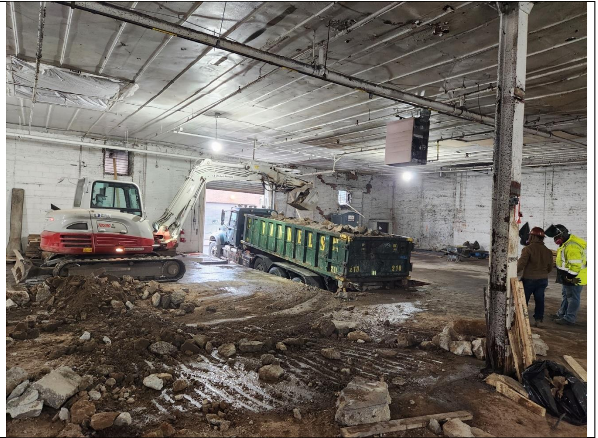
Photo 3 – View of truck loading for off-site concrete disposal.
