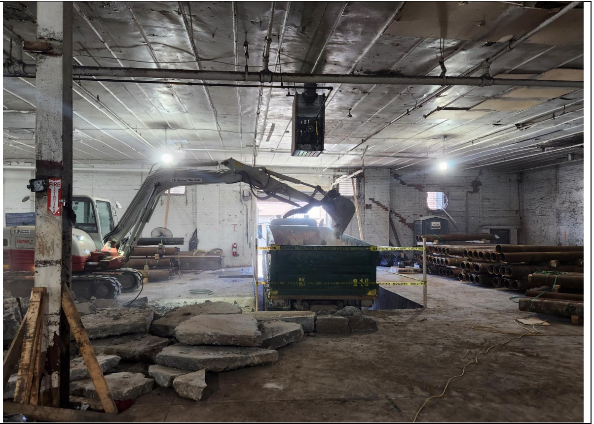
Photo 3 – View of container loading for off-site concrete disposal.
