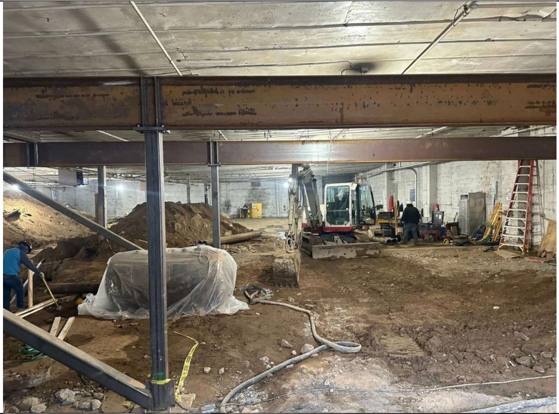
Photo 1 – View of Site conditions.
