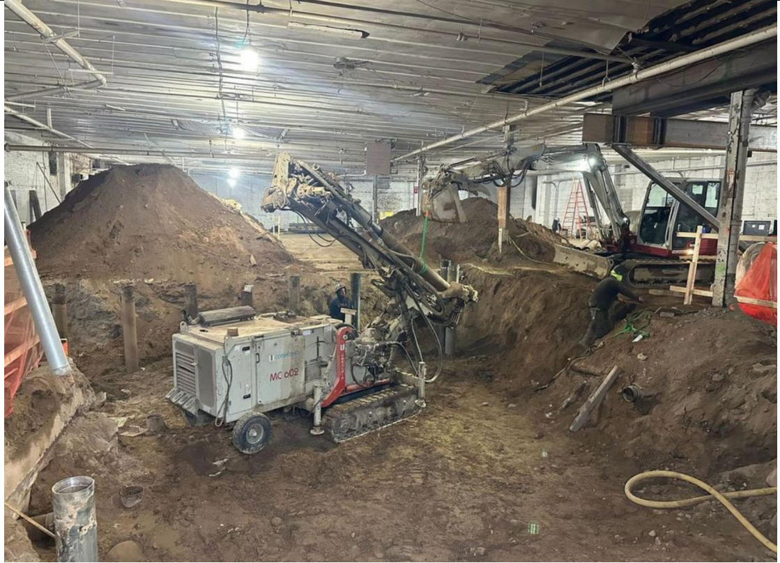
Photo 2 – View of soil excavation and pile installation.
