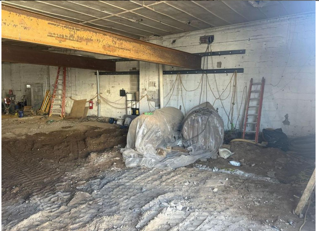
Photo 2 – View of staged tanks.
