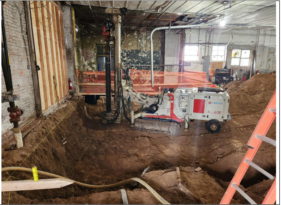
Photo 3 – View of pile installation.
