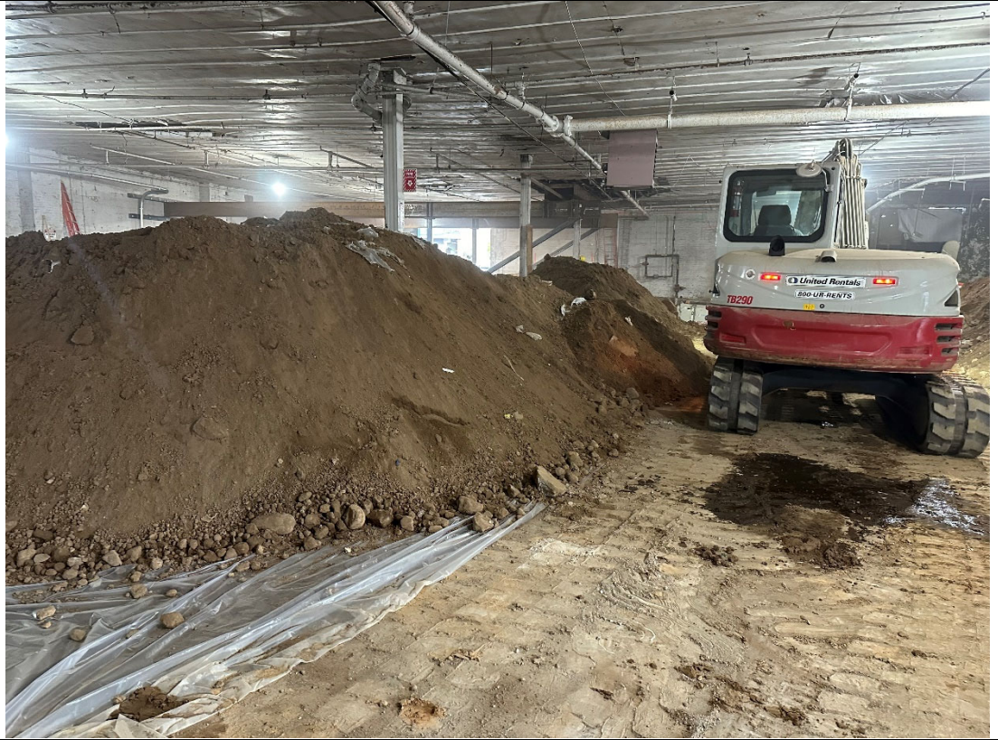
Photo 1 – View of stockpiled soil.
