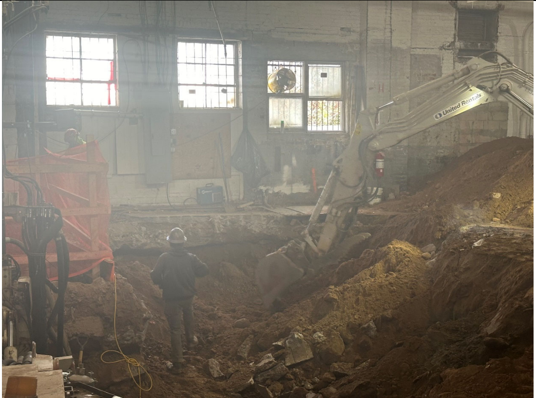
Photo 2 – View of soil excavation.
