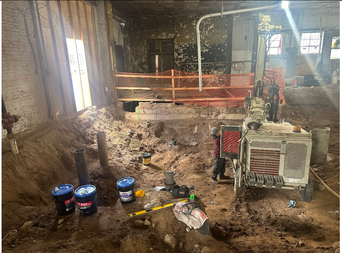
Photo 2 – View of pile installation.
