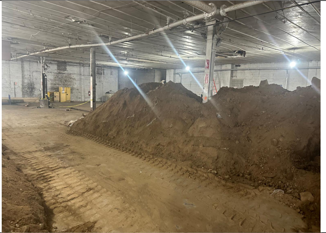
Photo 1 – View of Site conditions and soil stockpiles.
