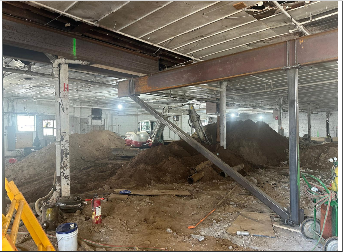
Photo 3 – View of soil excavation.
