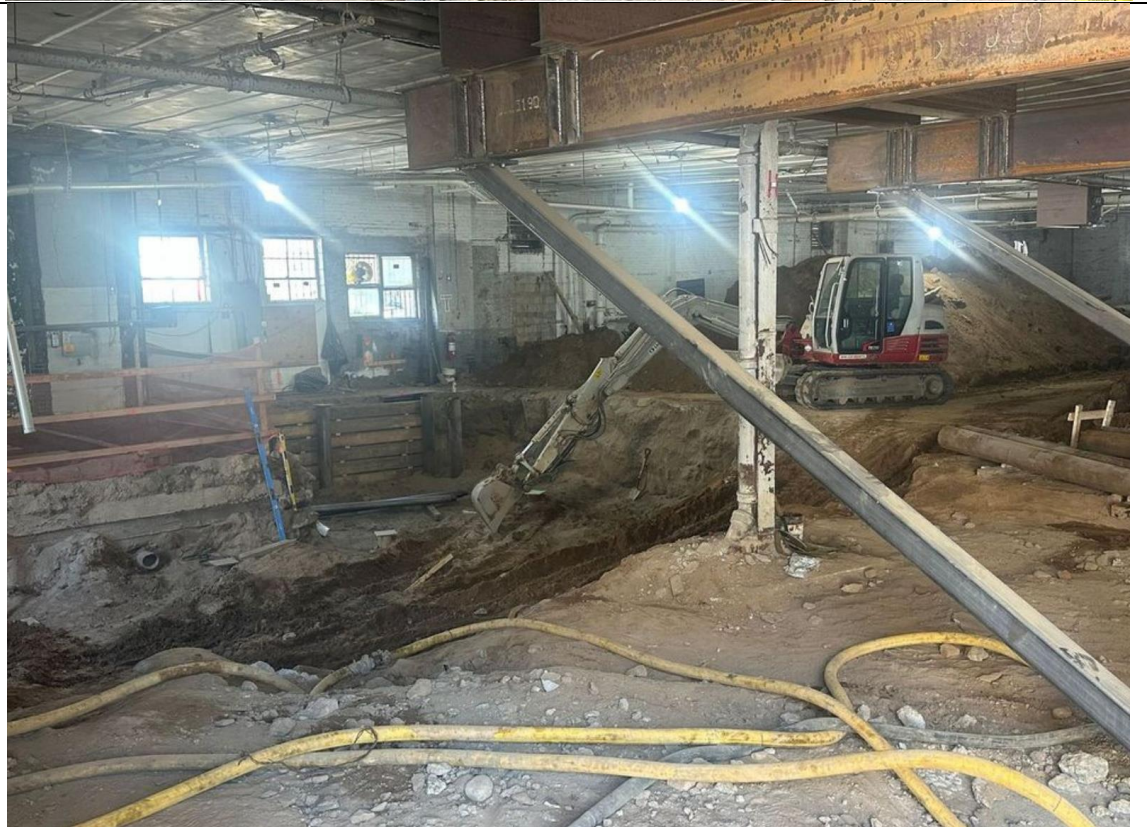
Photo 2 – View of soil excavation.
