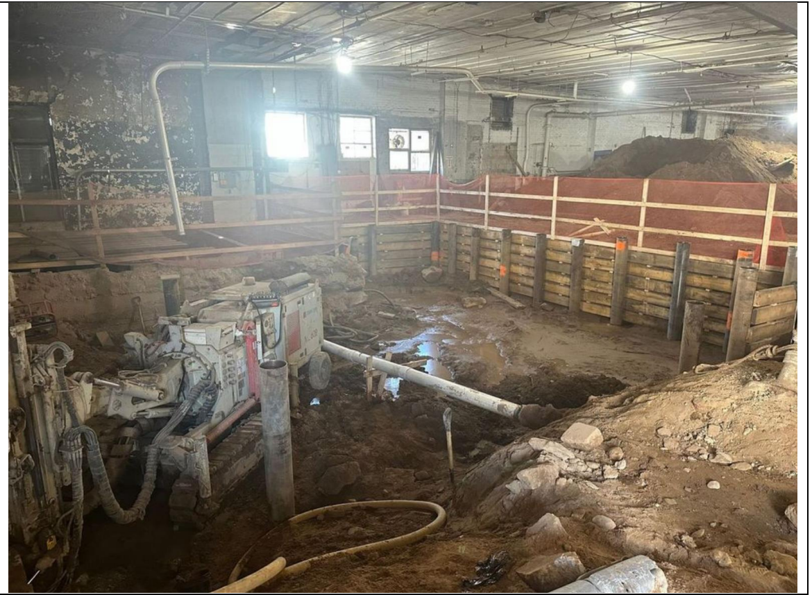
Photo 3 – View of Site conditions and SOE.
