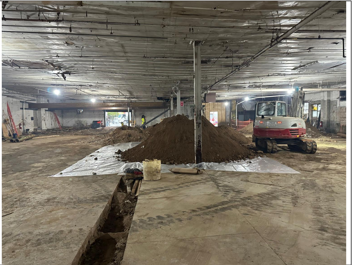
Photo 3 – View of stockpiled soil.
