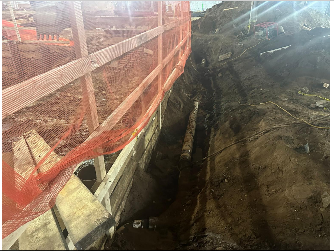
Photo 3 – View of drainage piping installation.
