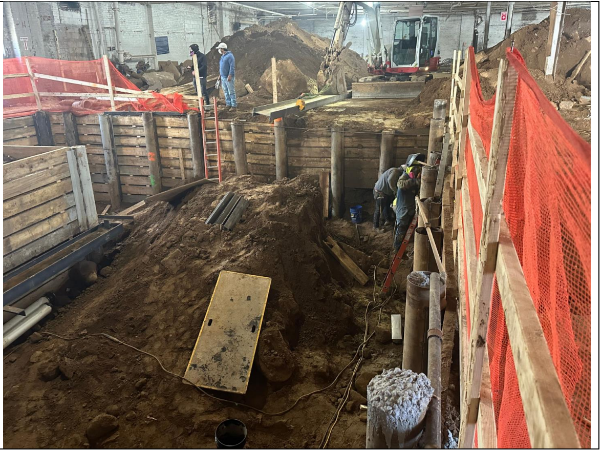
Photo 3 – View of lagging installation and welding.
