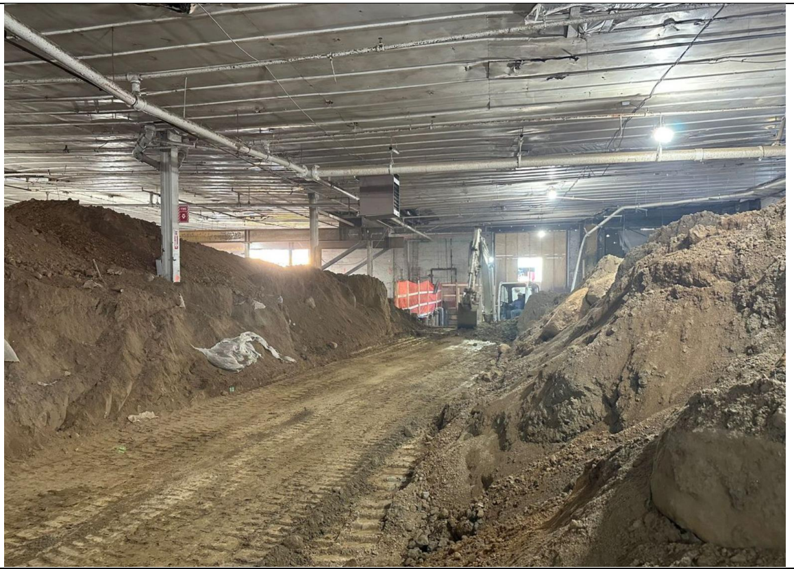
Photo 3 – View of soil stockpiled for off-site disposal.
