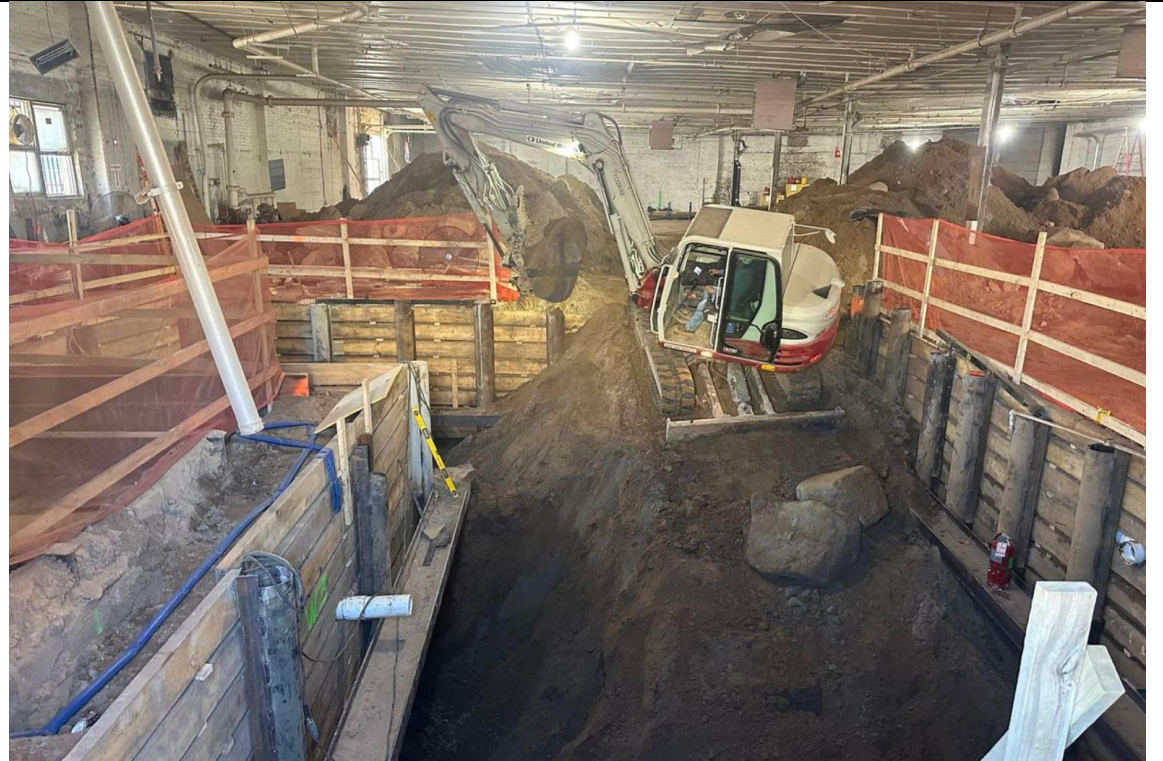
Photo 2 – View of soil excavation.
