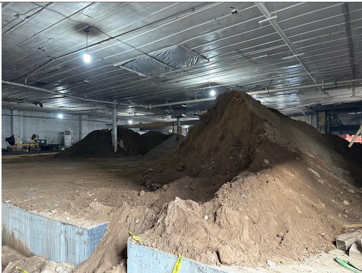
Photo 3 – View of Remaining soil stockpiles.
