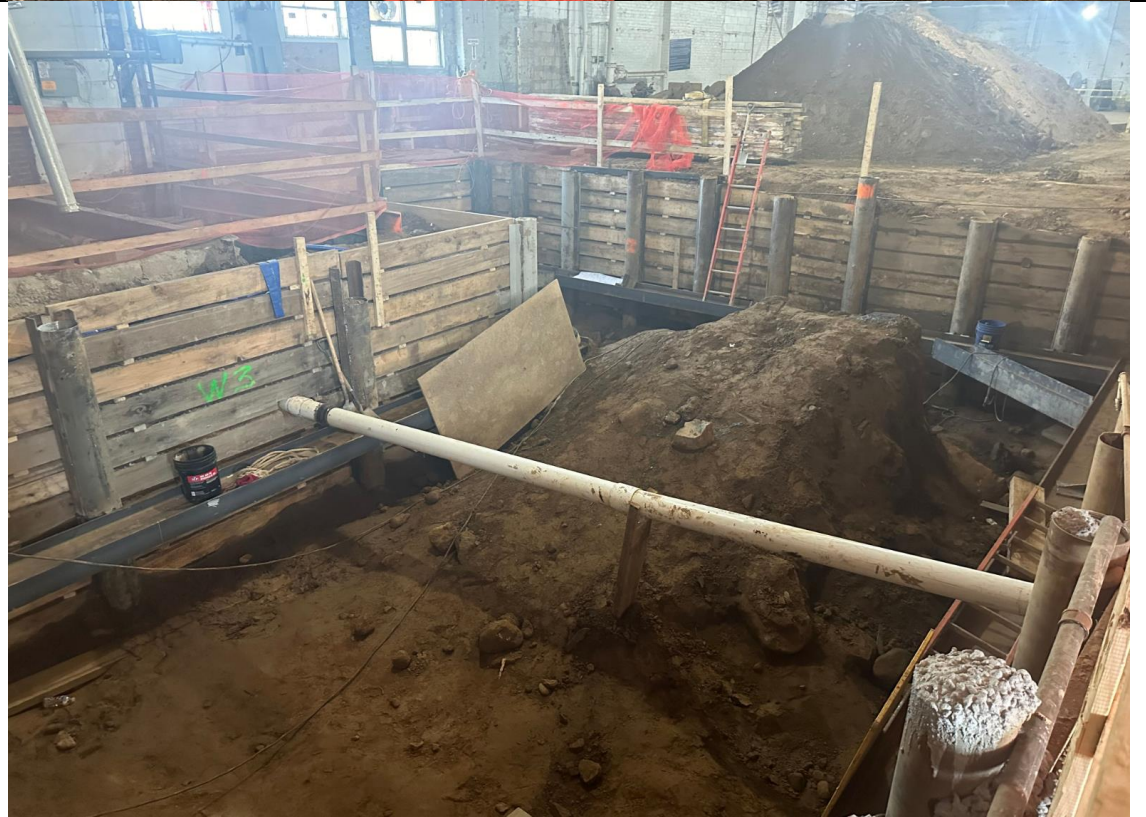
Photo 2 – View of the excavation and installed drainage pipe.
