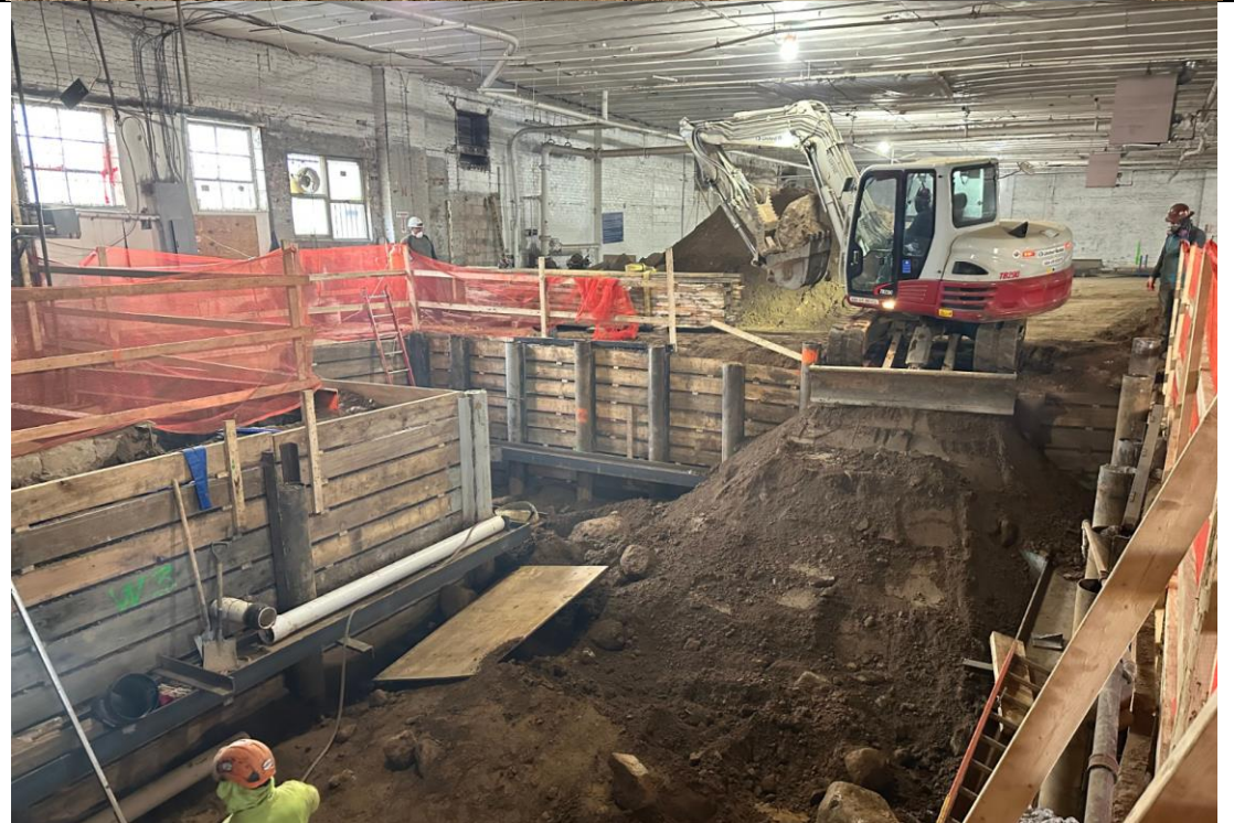
Photo 2 – View of soil excavation.
