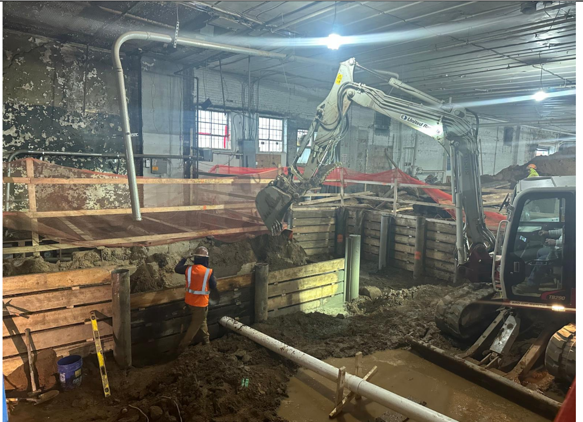
Photo 1 – View of excavation and lagging installation.
