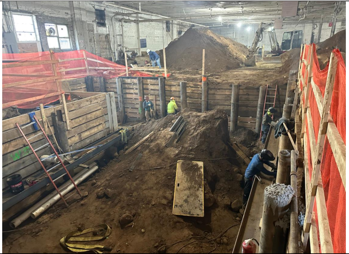
Photo 3 – View of lagging installation and welding.
