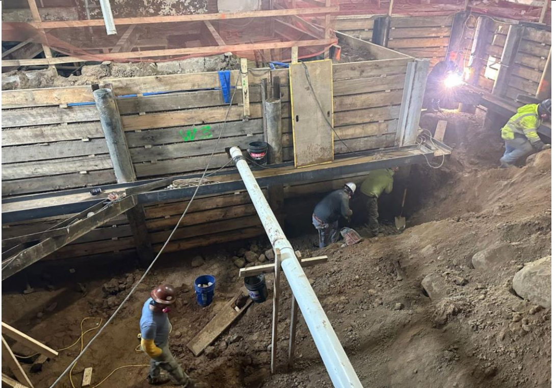
Photo 1 – View of Site conditions and welding activities.
