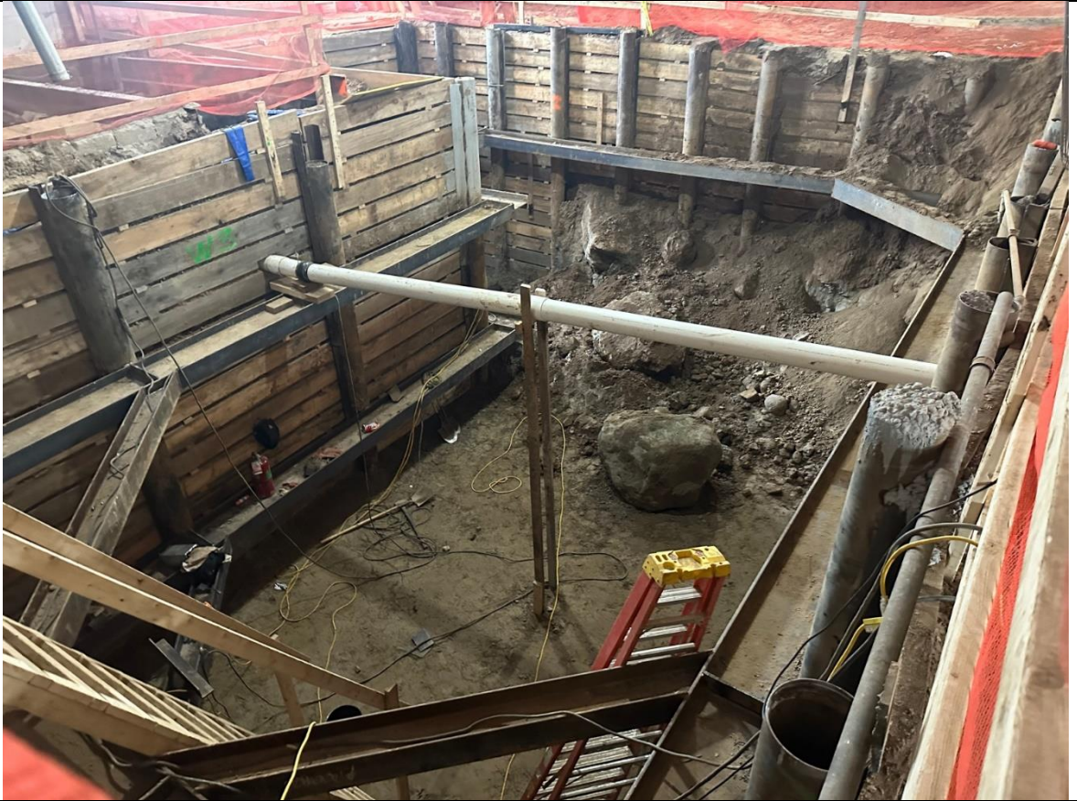
Photo 1 – View of the excavation.
