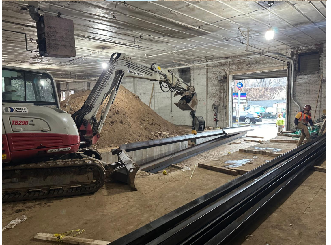
Photo 2 – View steel delivery.
