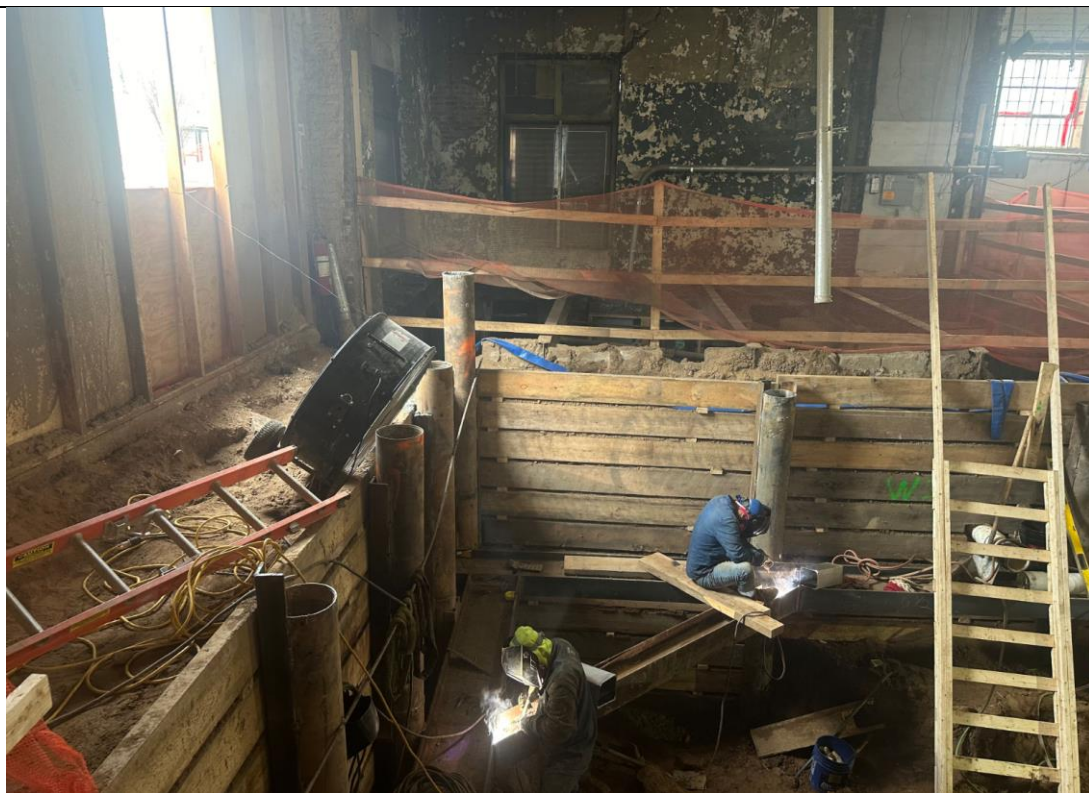
Photo 3 – View of welding activities.
