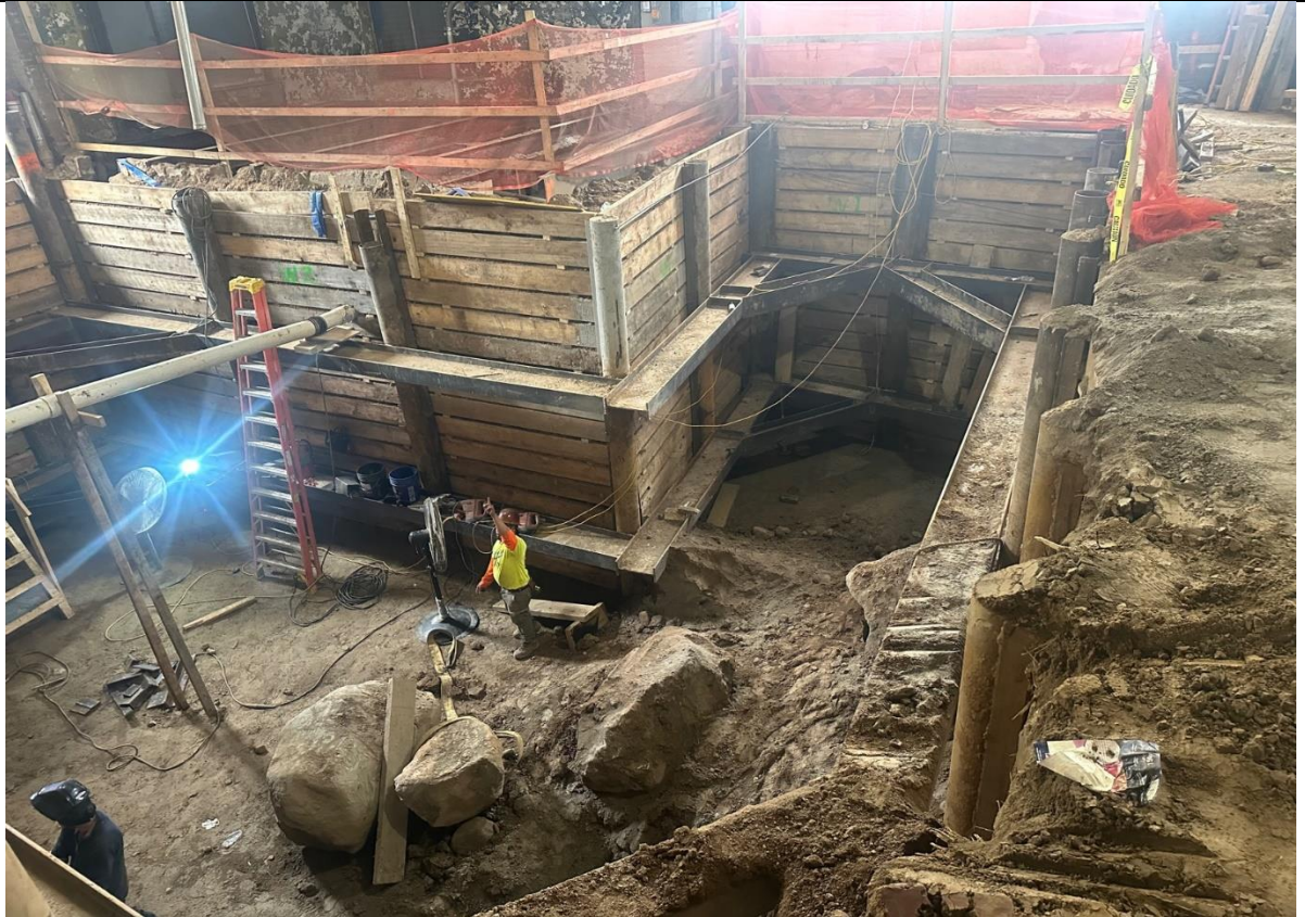
Photo 1 – View of the excavation.
