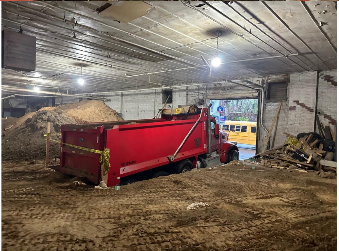
Photo 2 – View of truck loading for off-site soil disposal.
