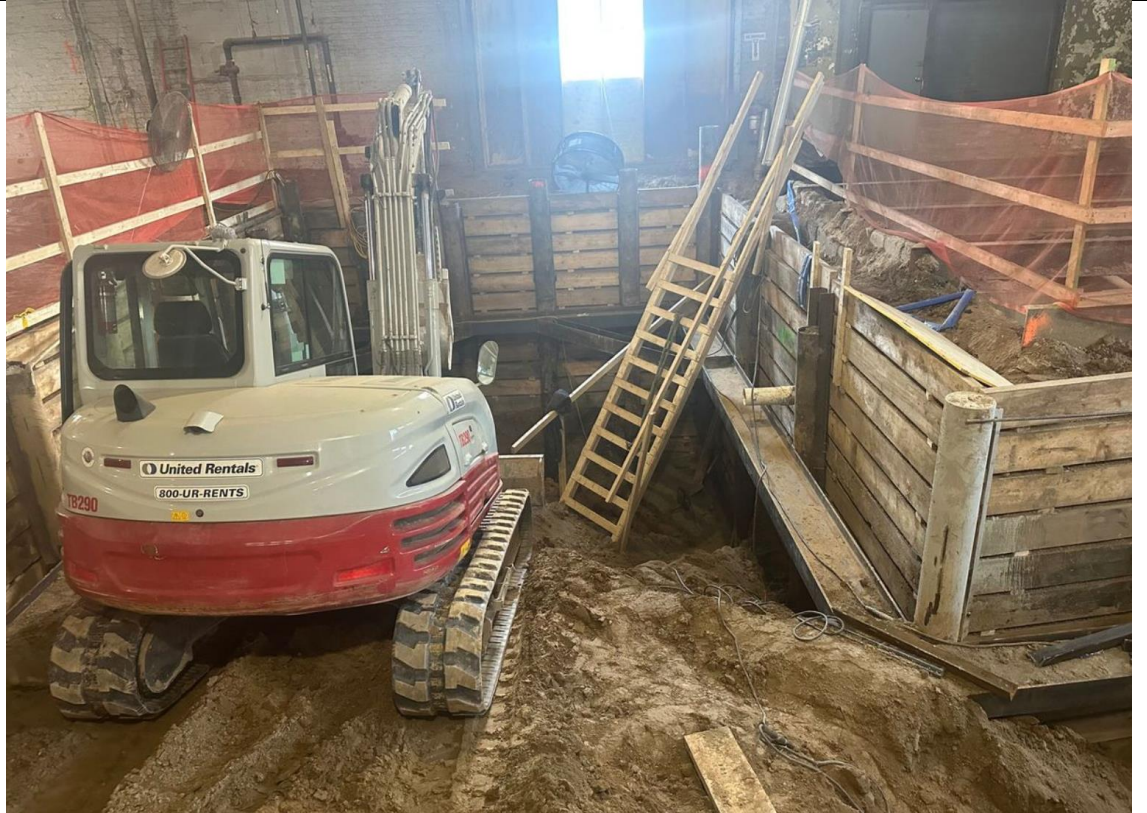
Photo 2 – View of soil excavation.
