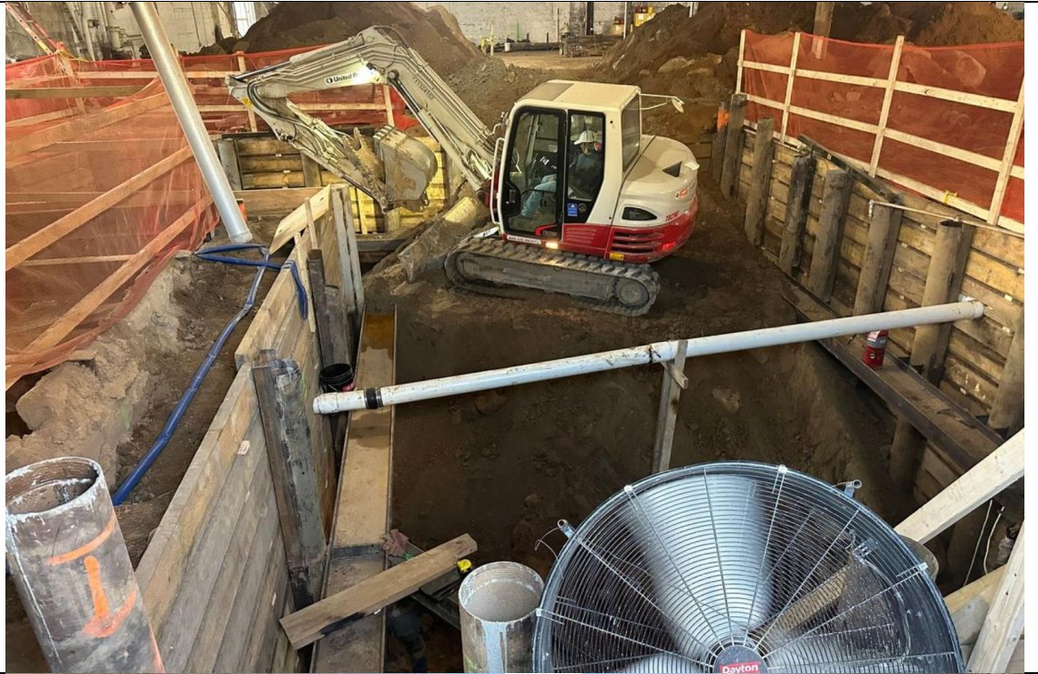
Photo 1 – View of soil excavation.
