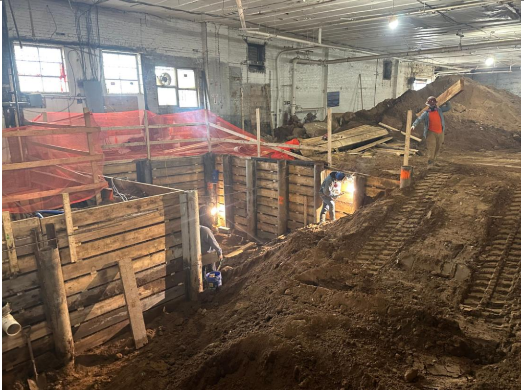
Photo 1 – View of Site conditions and welding.
