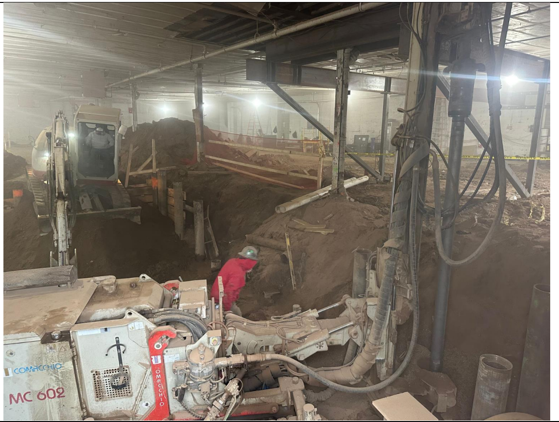
Photo 3 – View of pile installation.
