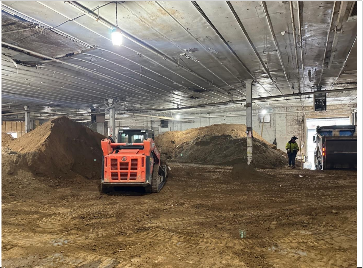
Photo 3 – View of remaining soil stockpiles.
