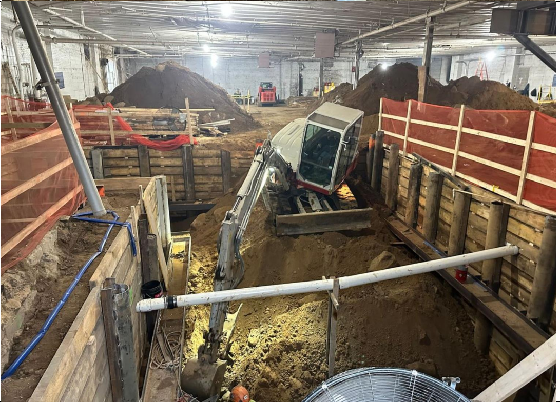
Photo 2 – View of soil excavation.
