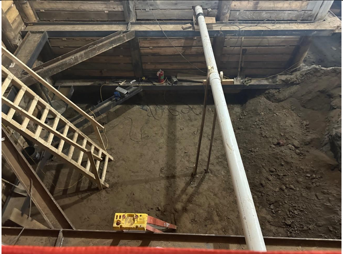
Photo 1 – View of the excavation.
