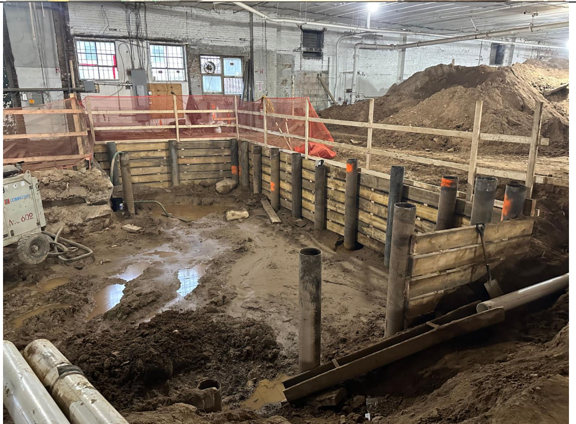
Photo 2 – View piles and lagging.
