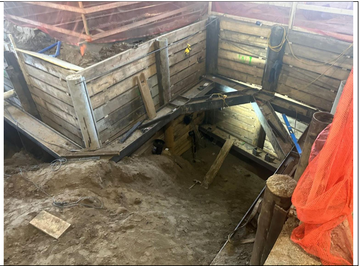
Photo 3 – View of soil excavation.
