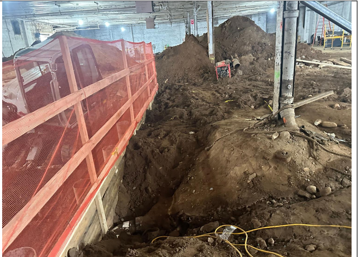
Photo 3 – View of backfilling after drainage piping installation.
