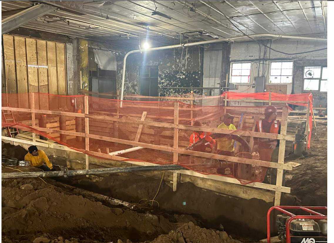
Photo 2 – View of pile grouting.
