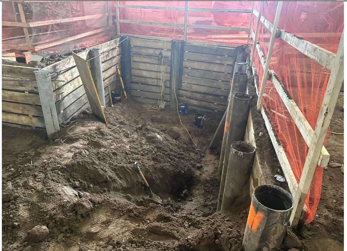
Photo 2 – View of soil excavation and SOE installation.
