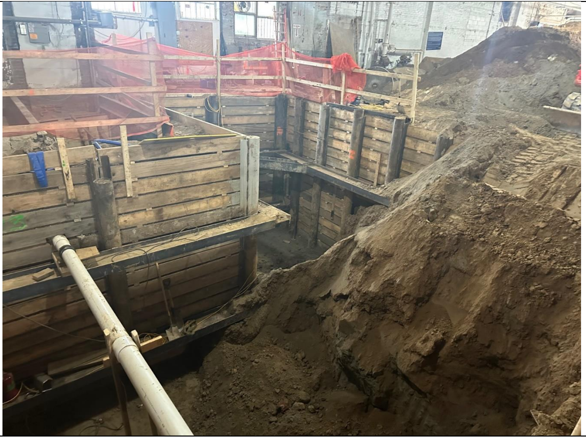
Photo 3 – View of the excavation.
