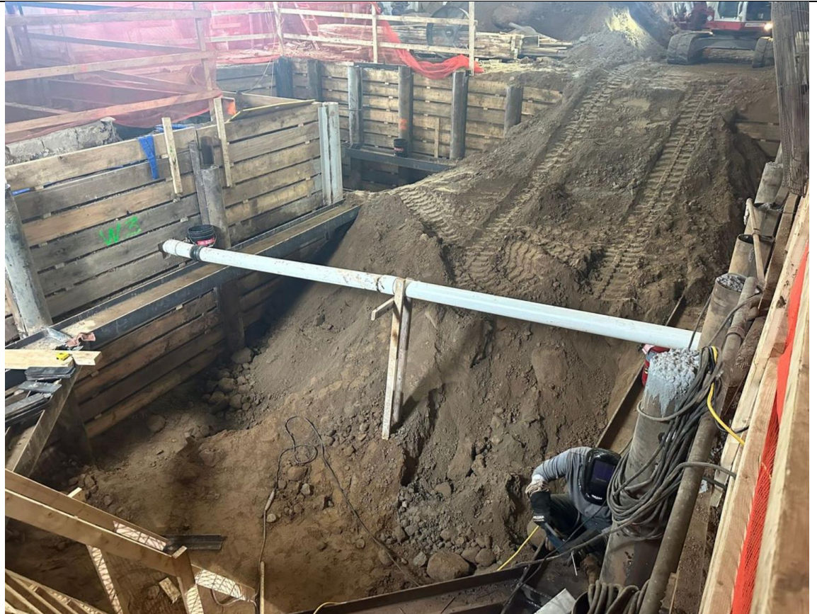
Photo 2 – View of soil excavation and welding activities.
