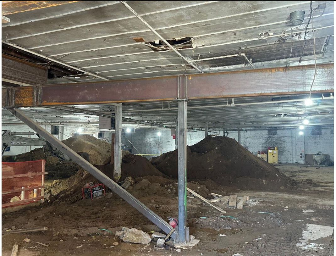
Photo 1 – View of Site conditions and soil stockpiles.
