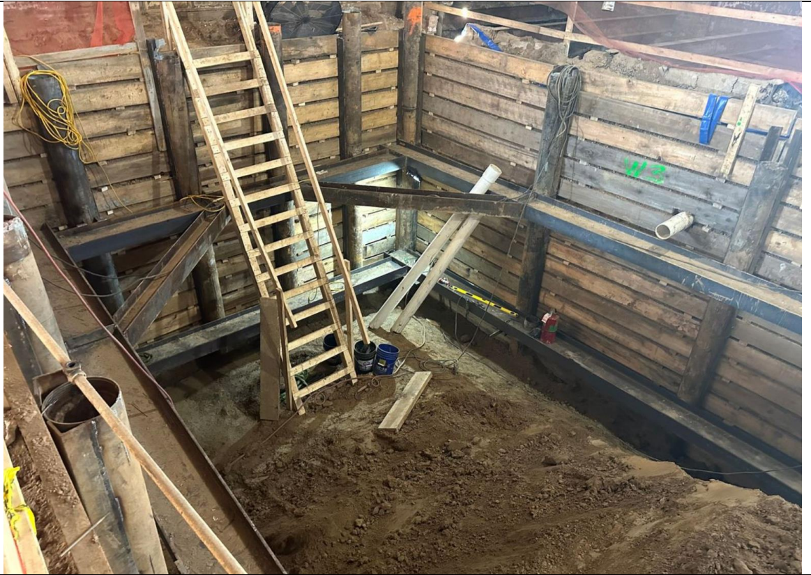
Photo 1 – View of the excavation.
