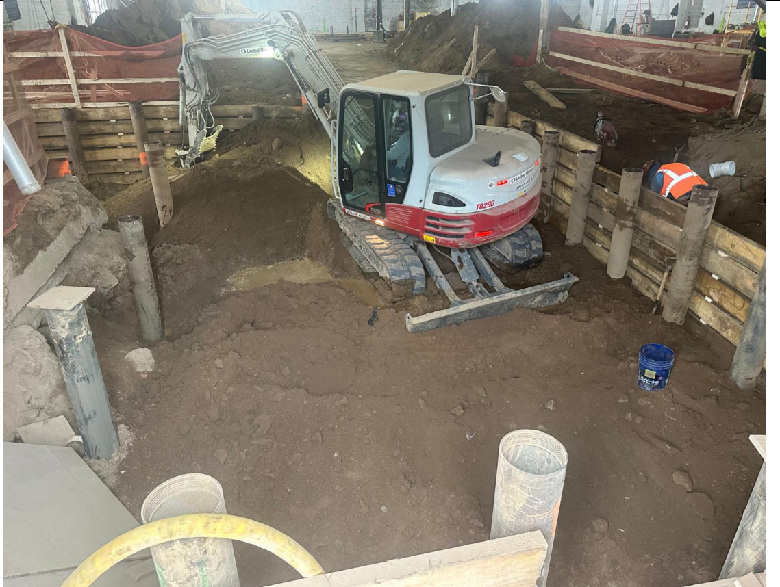
Photo 1 – View of soil excavation and SOE installation.
