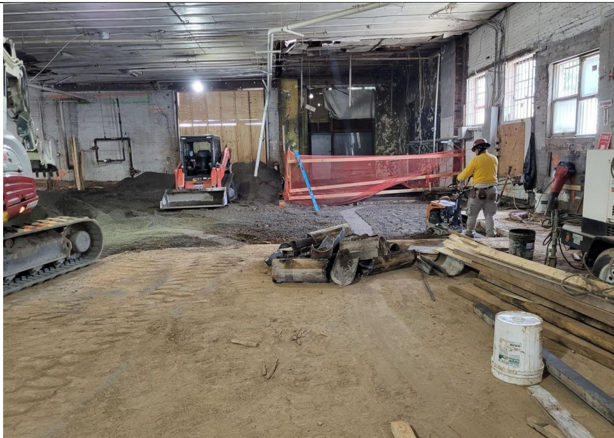
Photo 3 – View of RCA backfilling in the remedial excavation.
