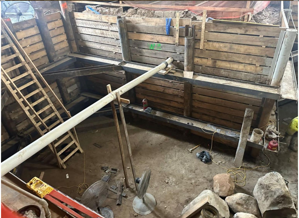
Photo 2 – View of the excavation.
