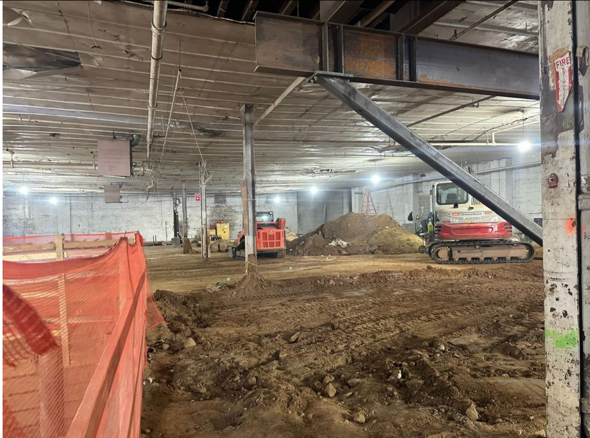
Photo 2 – View of remaining soil for off- site disposal.
