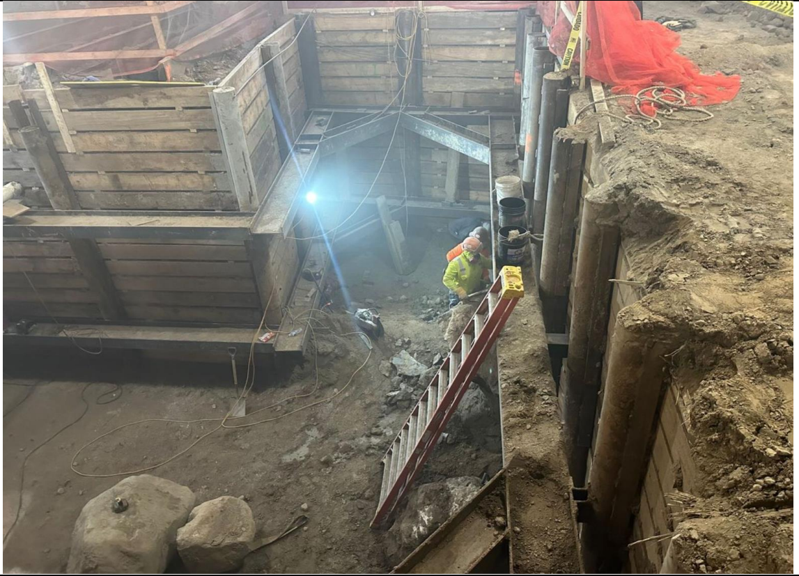
Photo 3 – View of SOE component welding.
