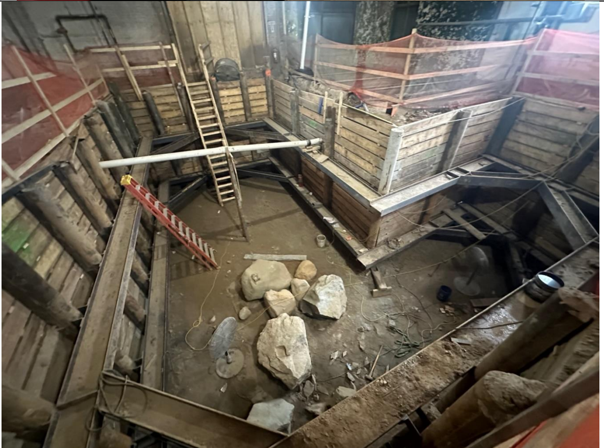
Photo 2 – View of the excavation.
