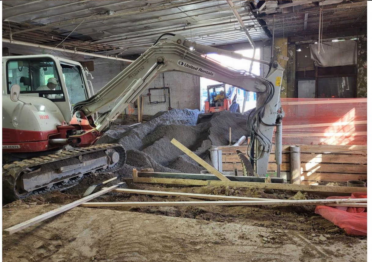
Photo 2 – View of RCA imported for backfilling.
