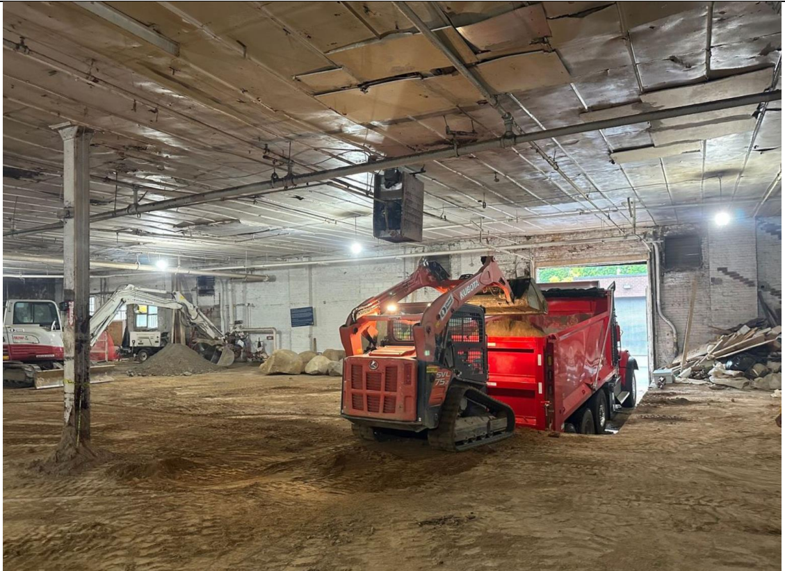
Photo 1 – View of truck loading for off-site soil disposal.
