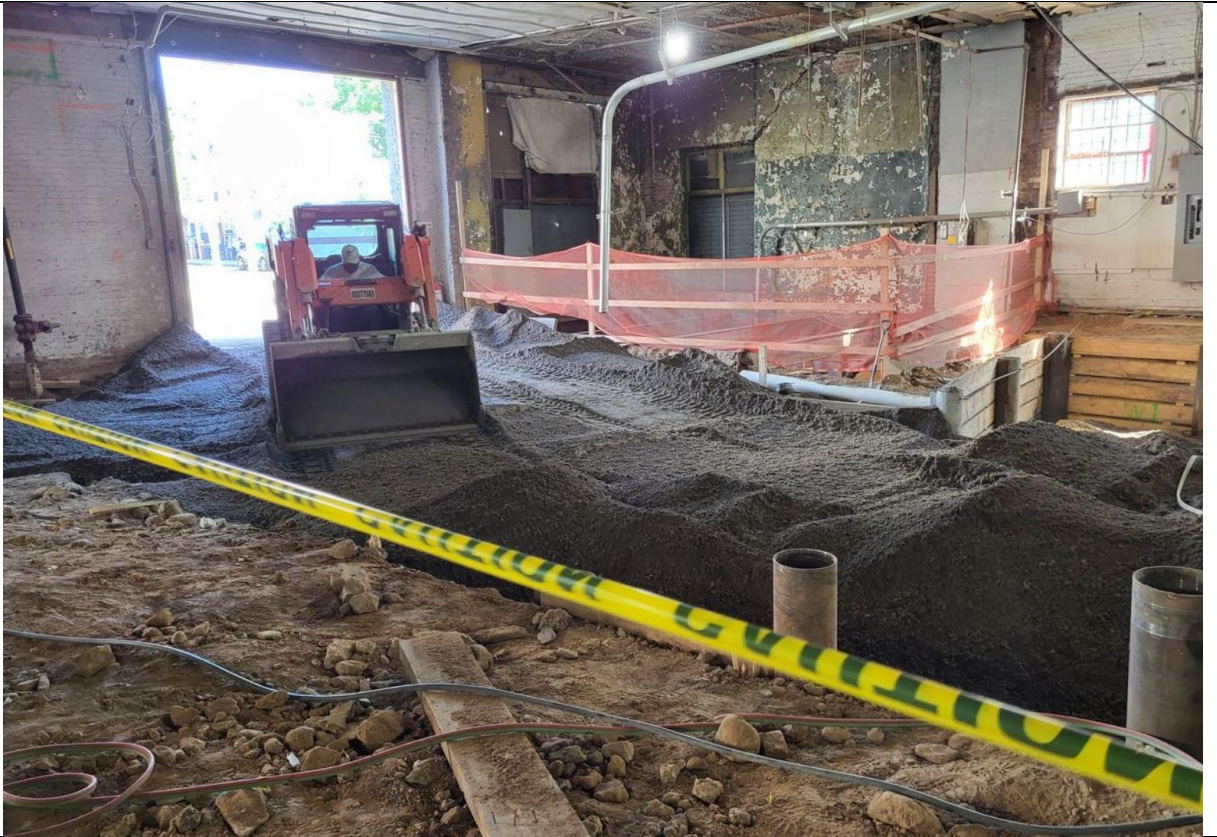
Photo 1 – View of backfilling the remedial excavation.
