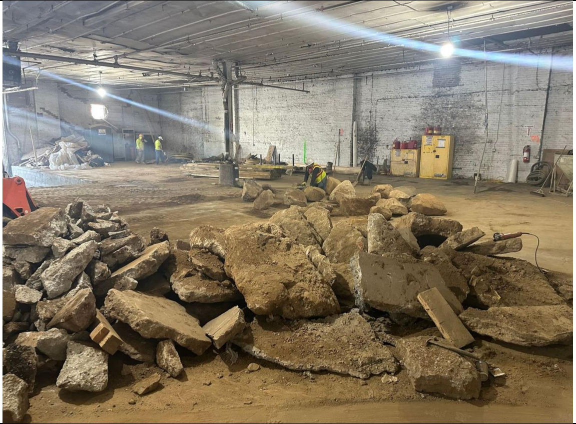
Photo 3 – View of Site conditions and boulder cleaning.
