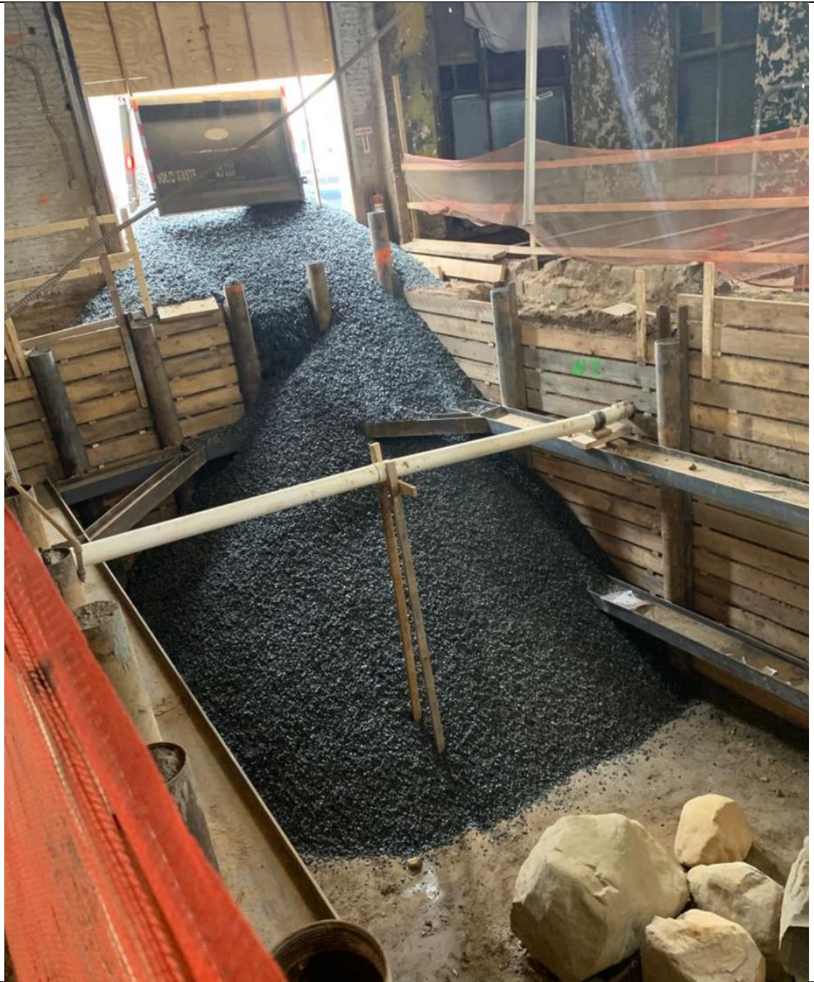
Photo 3 – View of stone backfilling in the remedial excavation.
