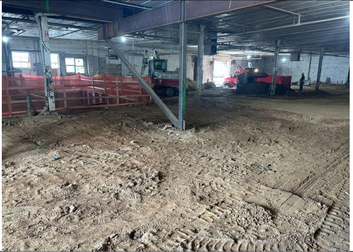
Photo 3 – View of site conditions and truck loading for off-site soil disposal.
