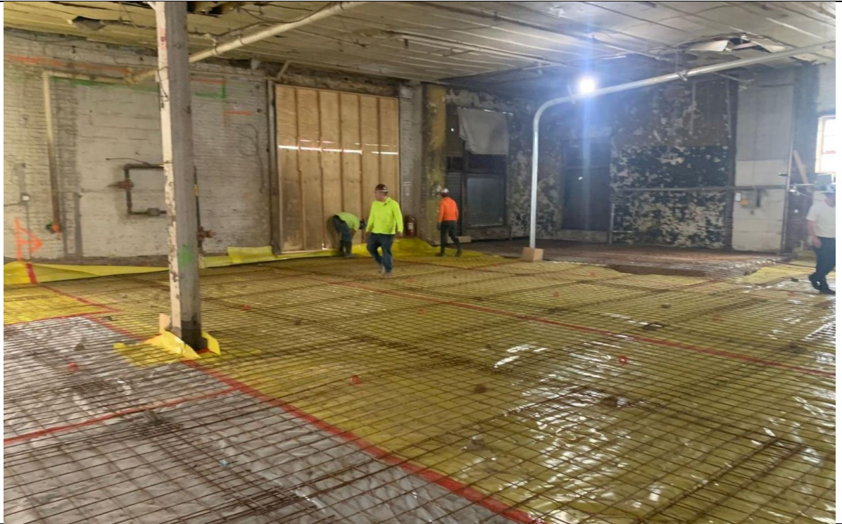
Photo 1 – View of vapor barrier installation.
