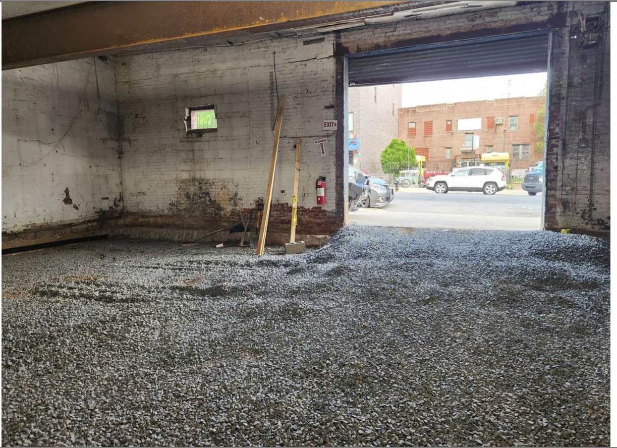
Photo 1 – View of RCA backfill.
