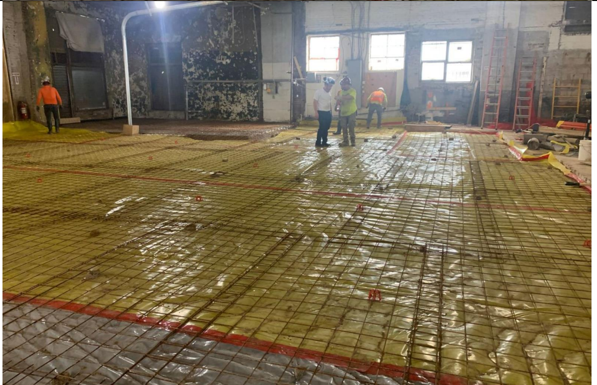
Photo 2 – View of vapor barrier installation.
