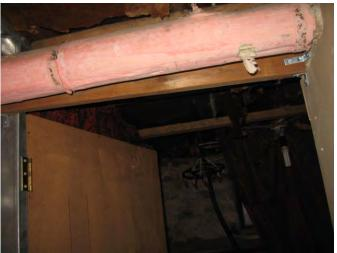
7. View of damaged suspect ACM aircell pipe insulation in the building basement
