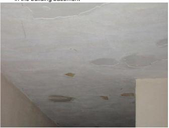
View of damaged/chipping paint at the second floor hallway
