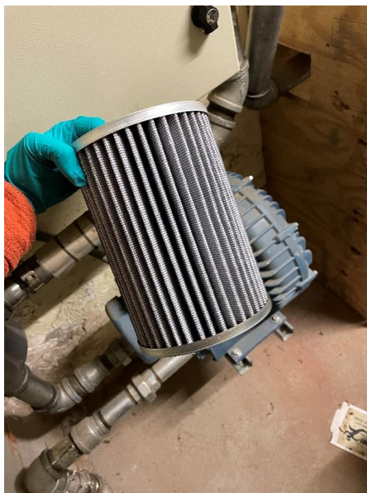
Photo 12, 11/29/2023: SVE blower filter inspection.
