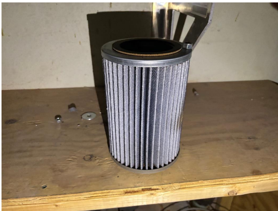
Photo 4, 12/12/2024: View of soil vapor extraction (SVE) system blower filter (facing north).
