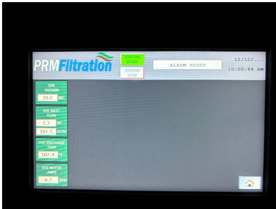
Photo 10, 12/12/2024: View of the SVE system control panel (facing north).
