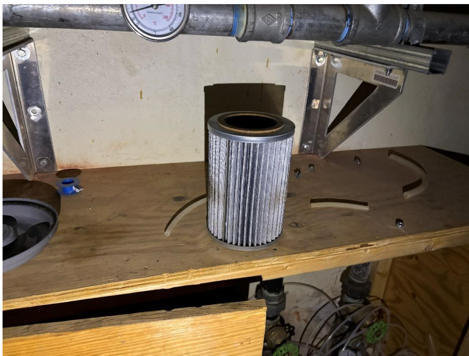
Photo 4, 12/12/2025: View of soil vapor extraction (SVE) system blower filter (facing north).
