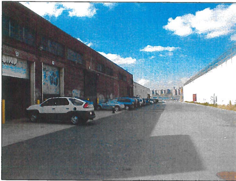
View of the north side of the warehouse along India Street
