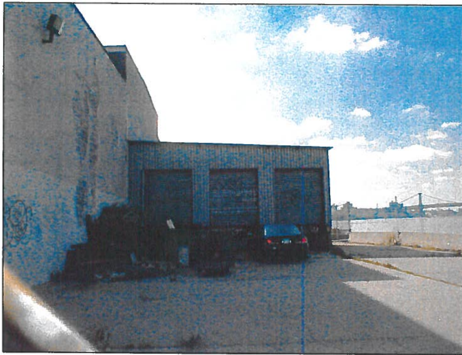
View of the dumpster and west end loading bays
