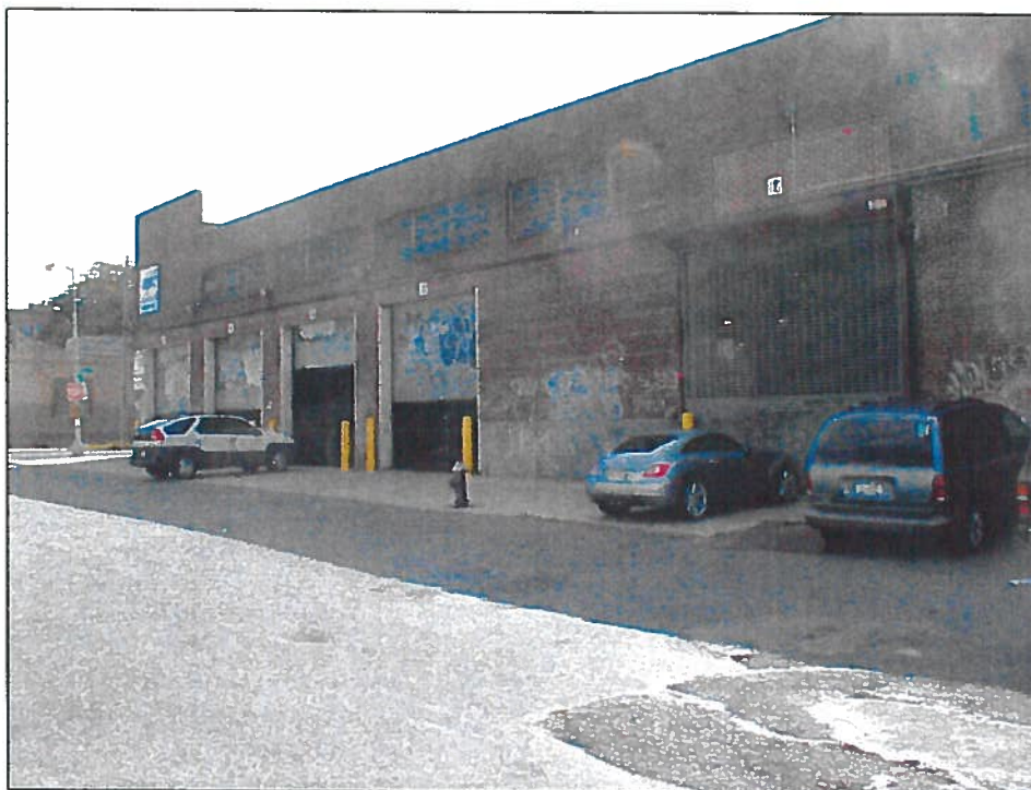
View of 5 of the 10 loading docks
