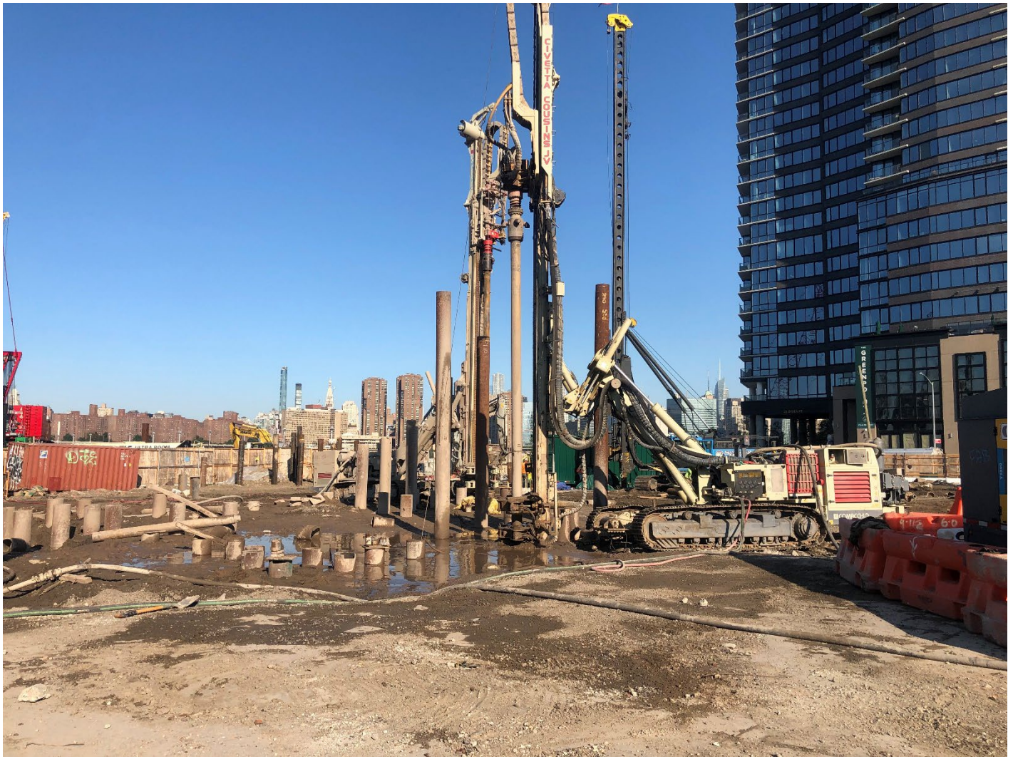
Photo 5: Looking northwest: CCJV continues with caisson drilling in the center area of grid cell SC-4.
