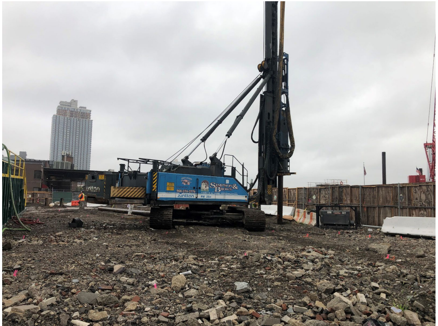
Photo 5: Looking south: Simpson & Brown starts pile driving activities in in grid cells SC-1 and SC-2.
