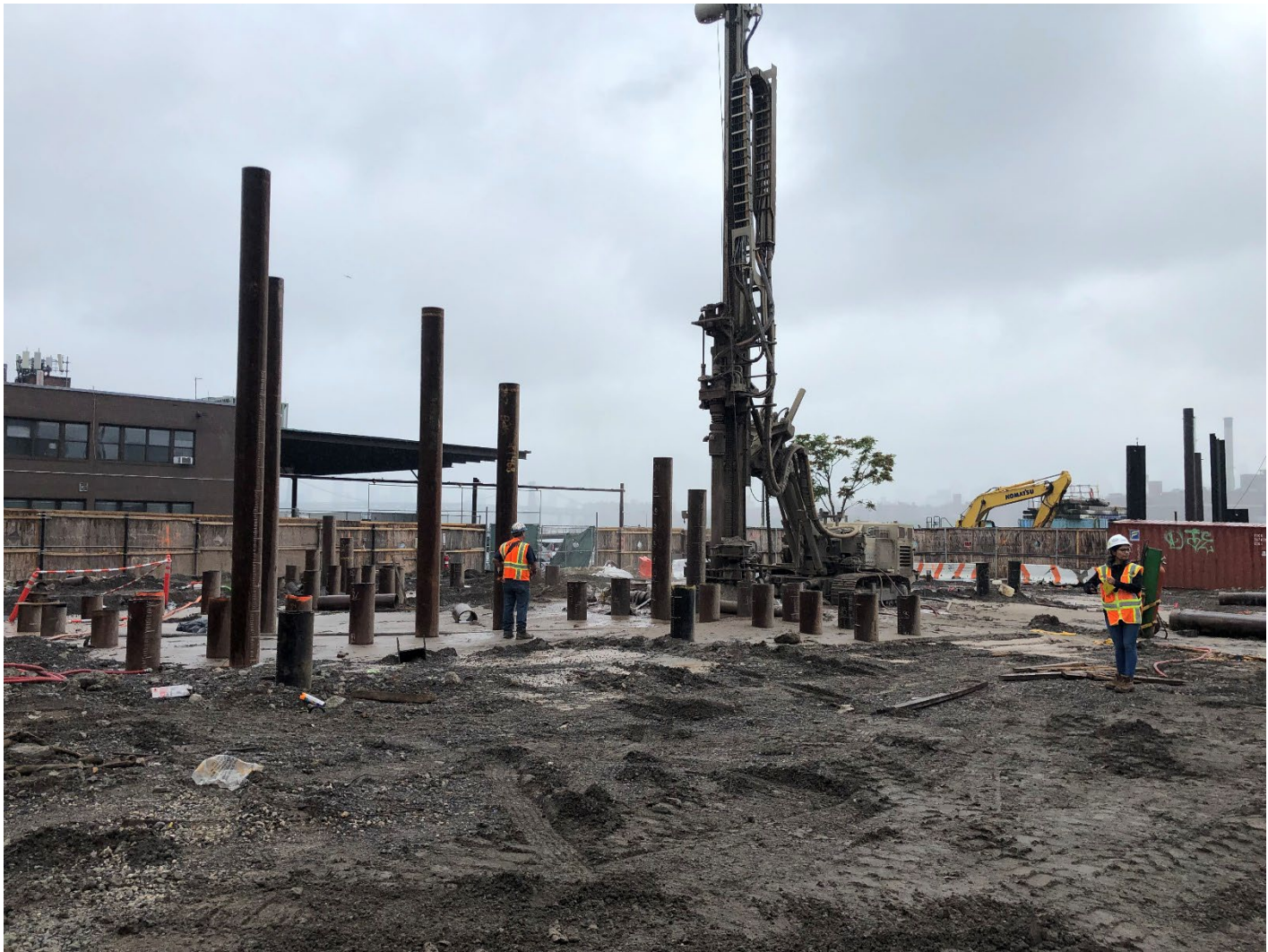
Photo 4: looking east: CCJV continues caisson drilling within the center area of grid cell SC-4.
