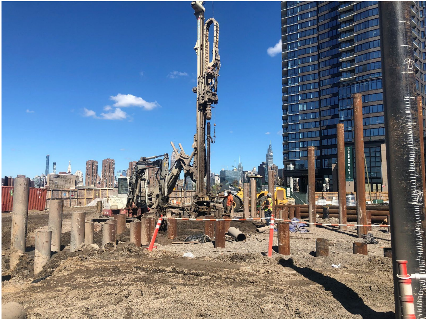
Photo 4: looking east: CCJV starts caisson drilling within the south center area of grid cell SC-4.
