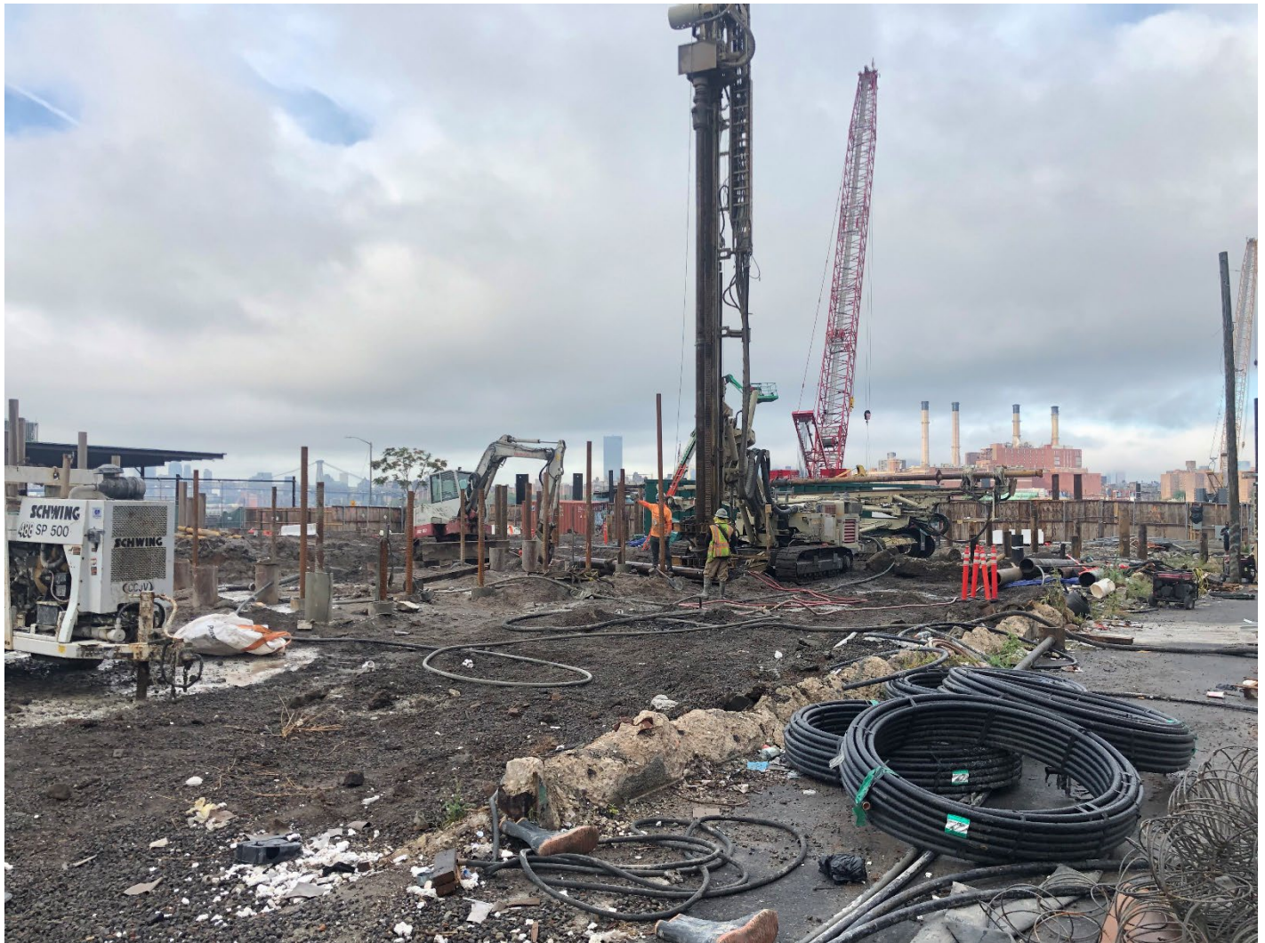
Photo 4: Looking south: CCJV removing sediments from installed caissons in the north area of grid cell SC-4.
