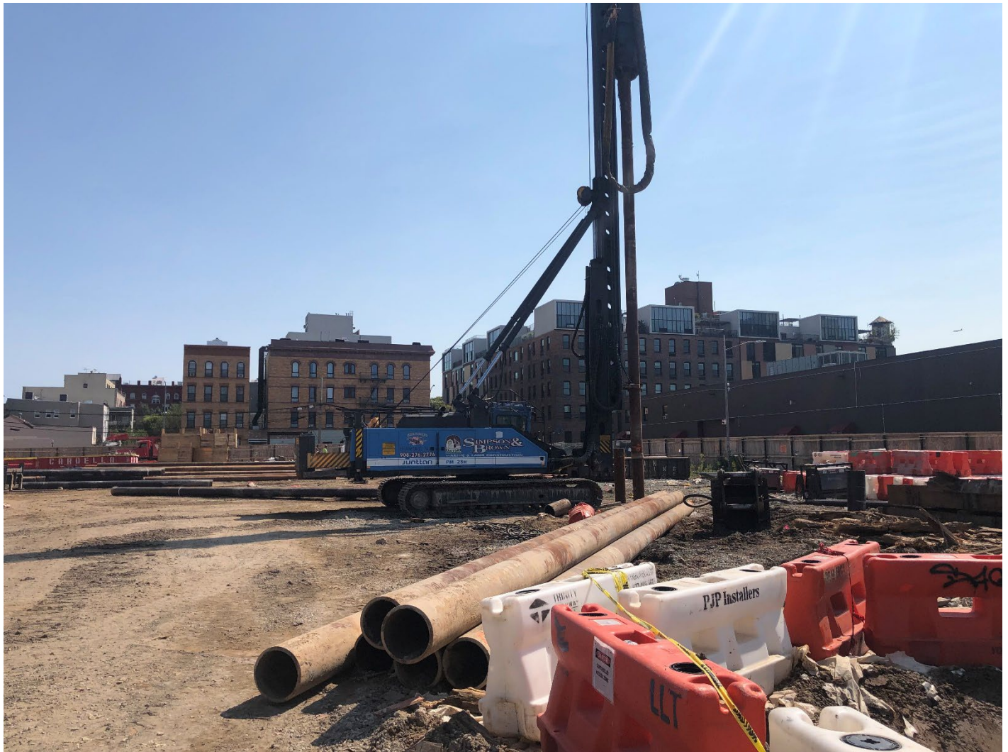
Photo 3: Looking east: Simpson & Brown performing pile driving in grid cell SC-11.
