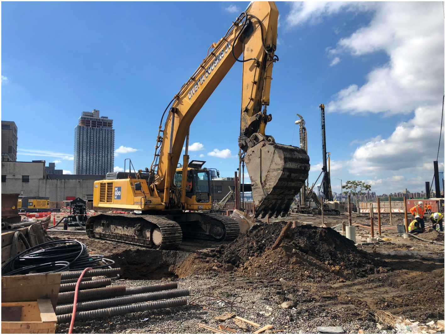
Photo 4: looking south: CCJV starts excavating test pit for soil sampling in the north area of grid cell SC-4.
