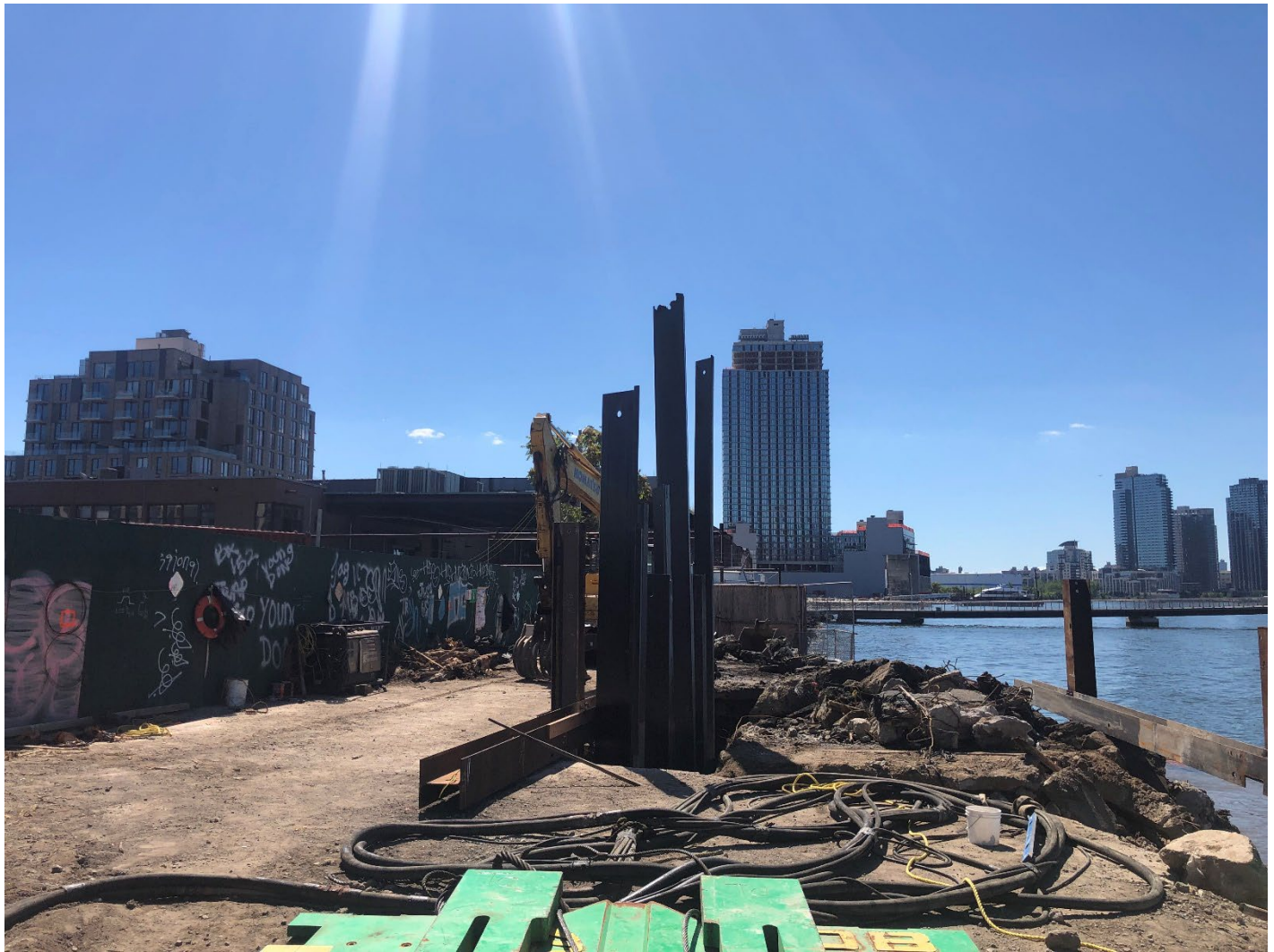
Photo 3: Looking south-southeast: Trevcon continuing with sheet pile driving in grid cell SC-2.
