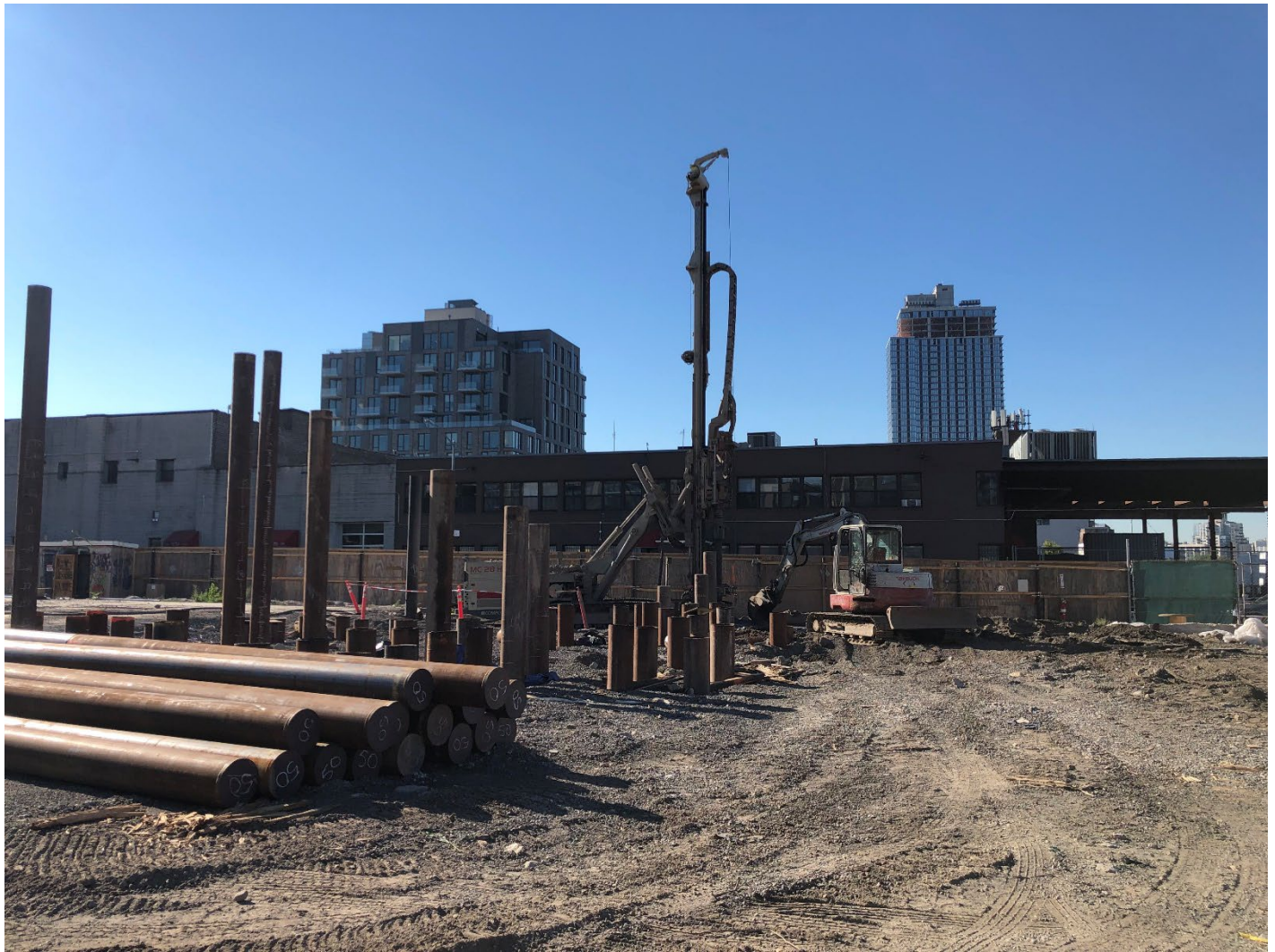
Photo 4: looking west: CCJV continues with caisson drilling within the south area of grid cell SC-4.
