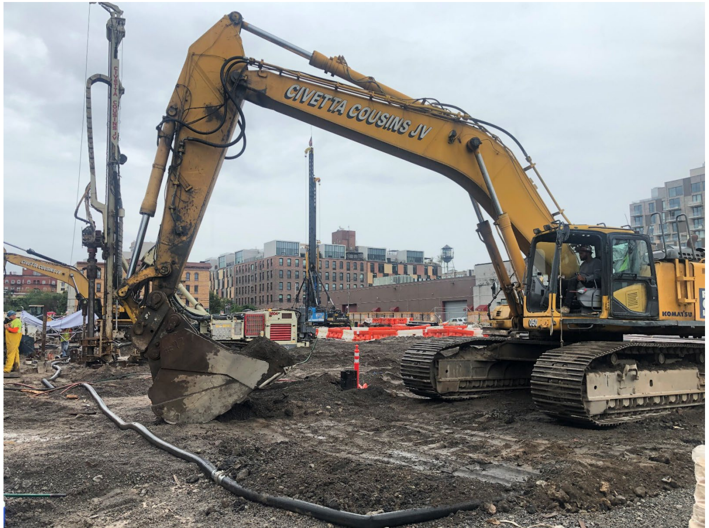
Photo 4: looking east: CCJV starts excavating test pit for soil sampling in the north area of grid cell SC-4.
