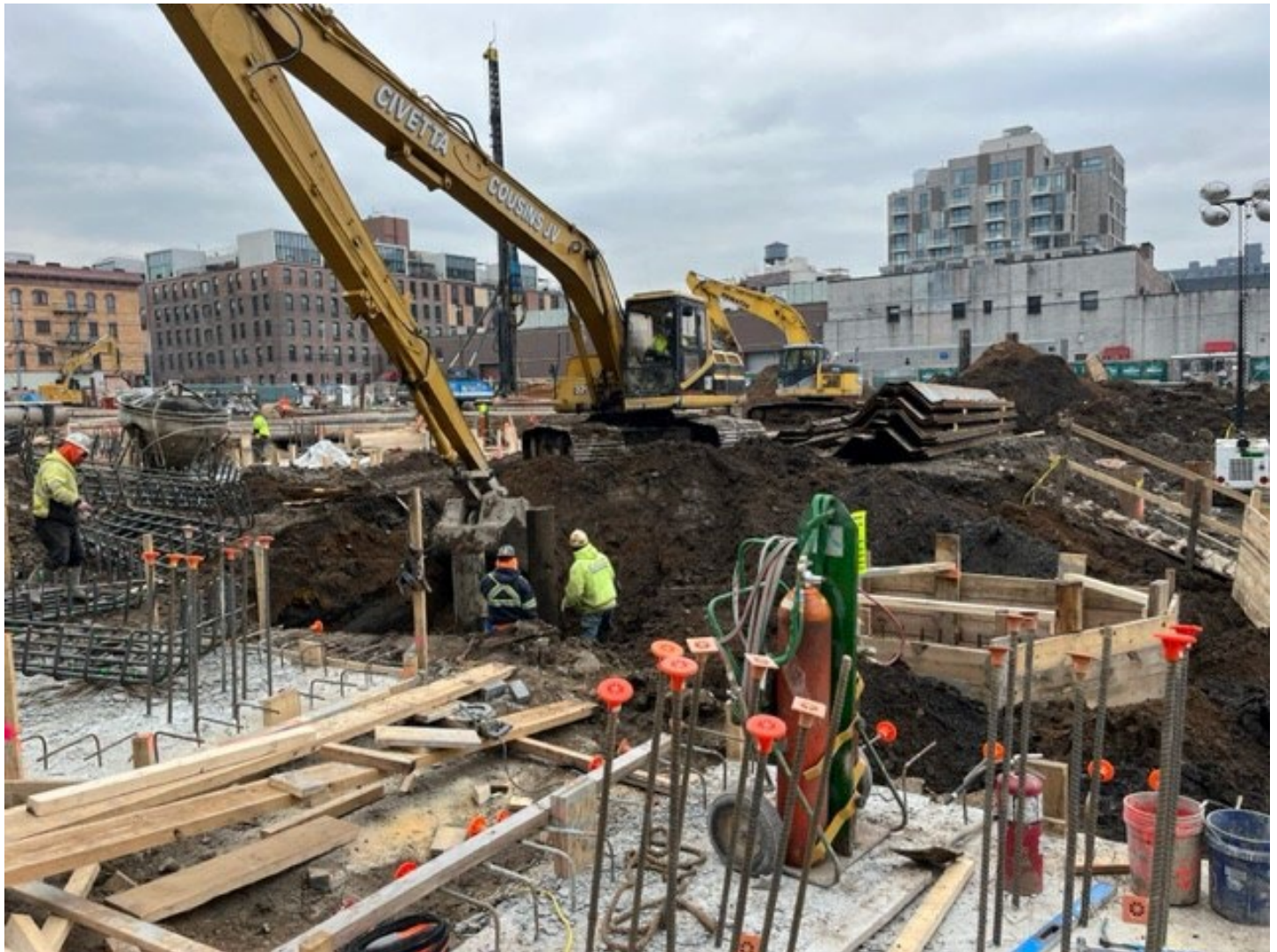
Photo 2: View facing southeast, CCJV excavating in grid cell SC-8 in order to install foundation footings.
