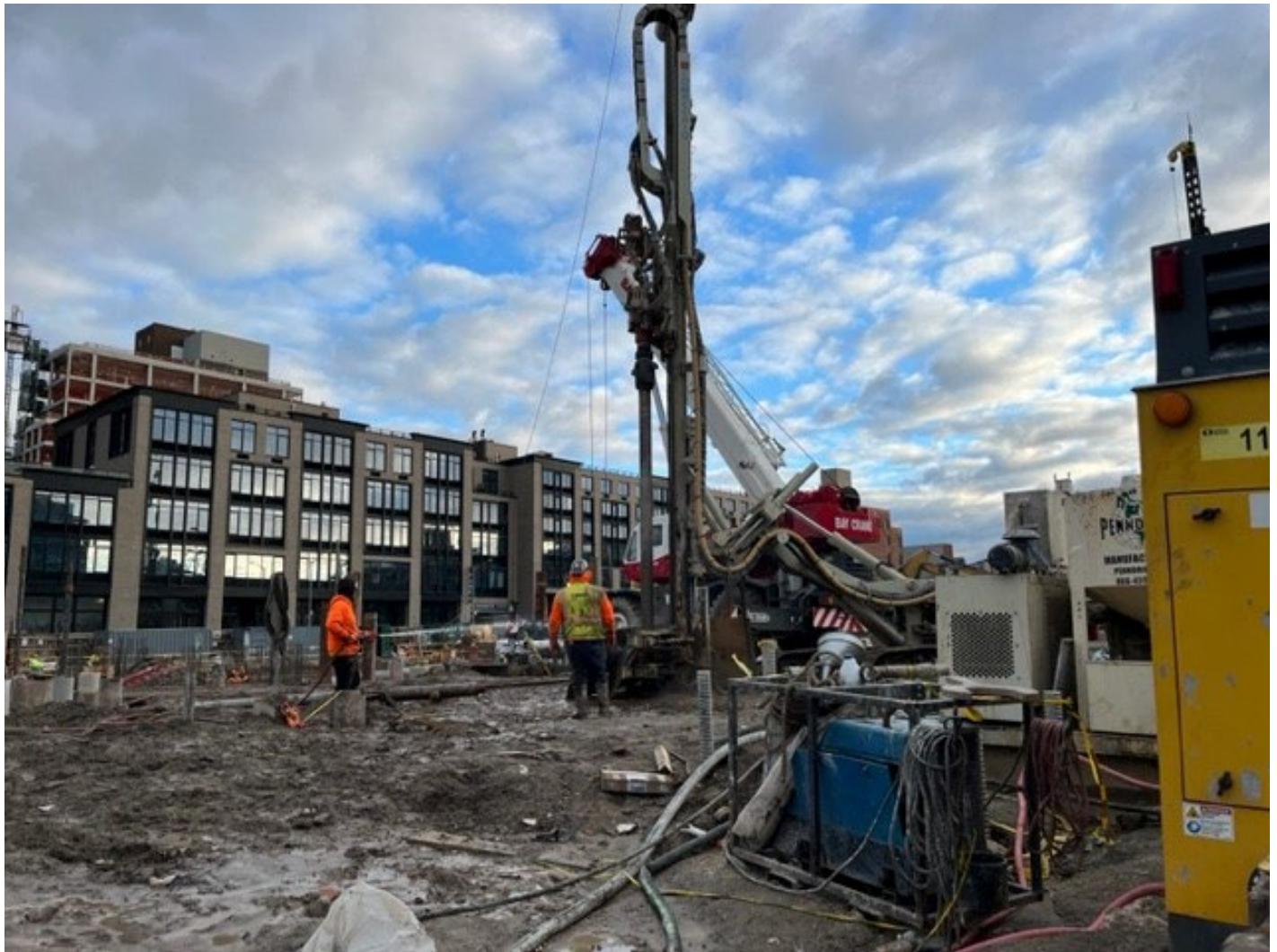
Photo 3: View facing northeast, CCIJ performing caisson drilling in grid cell SC-4.
