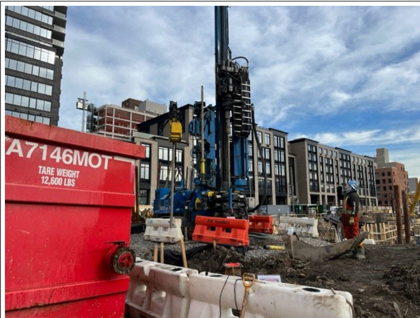
Photo 1: View facing northeast, Brightcore drilling a geothermal well in grid cell SC-4.
