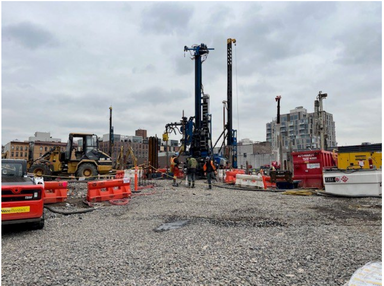
Photo 1: View facing southeast, Brightcore performing geothermal well installation in grid cell SC-4.
