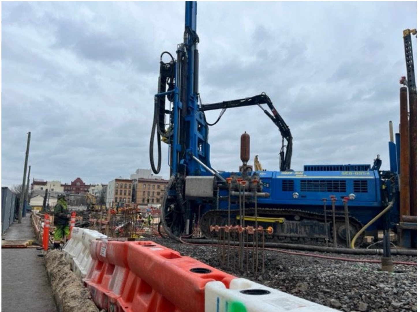
Photo 1: View facing south, Brightcore drilling a geothermal well in grid cell SC-4.
