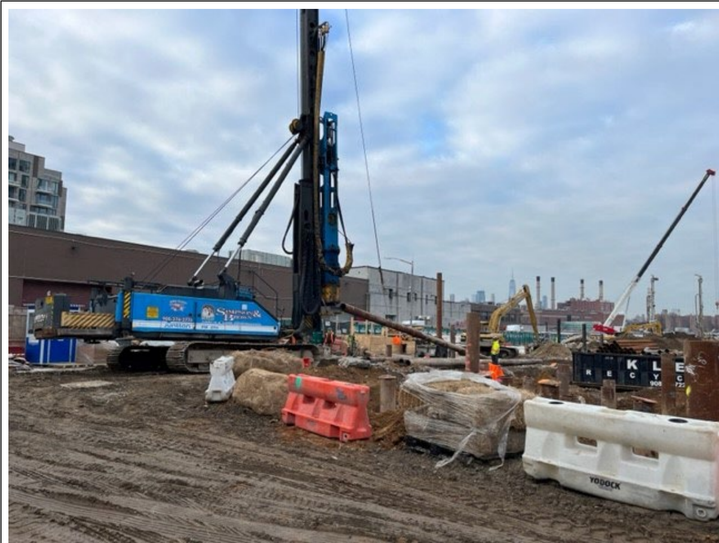
Photo 4: View facing southwest, Simpson & Brown performing pile driving in grid cell SC-16.
