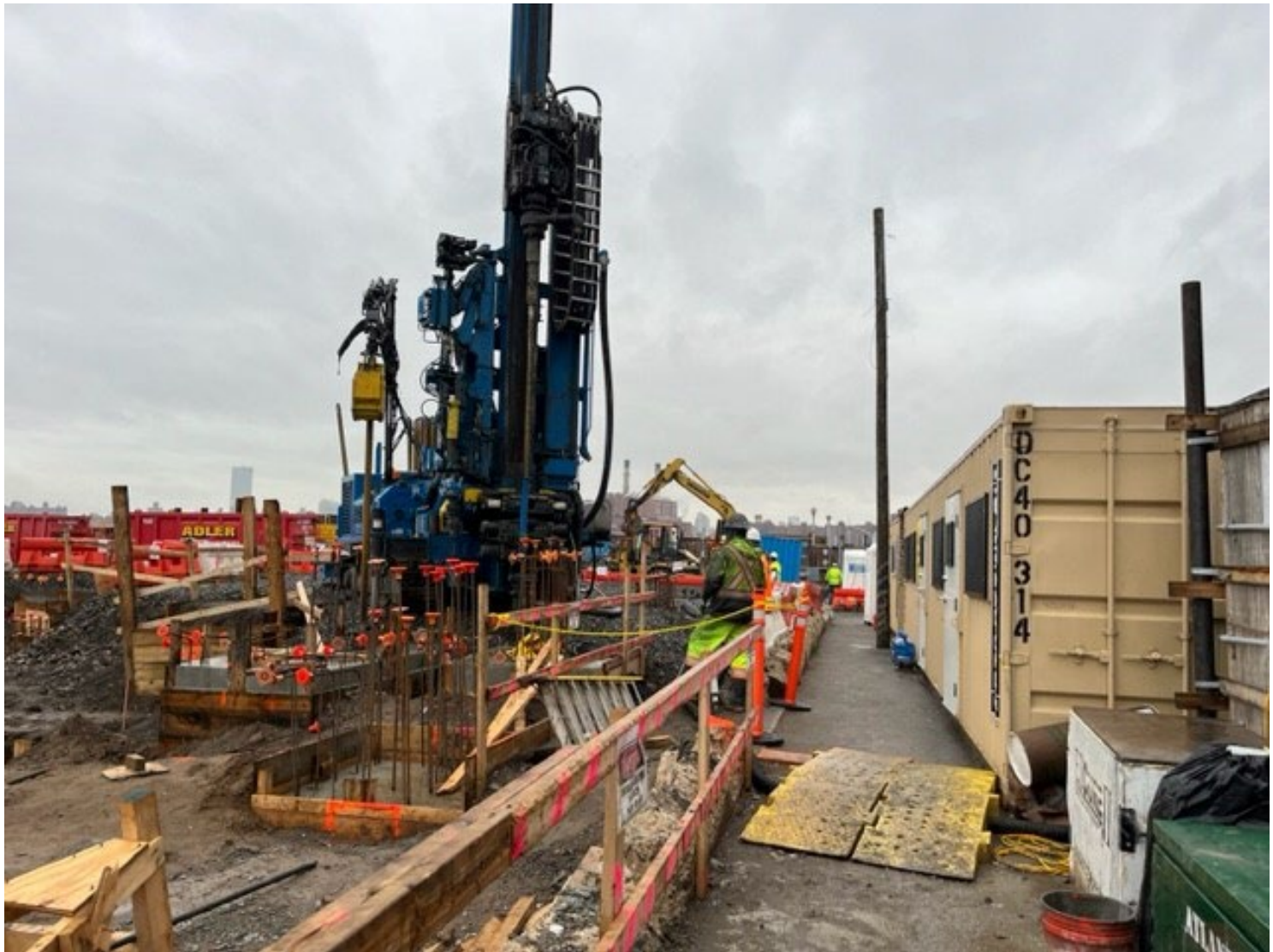
Photo 1: View facing west, Brightcore drilling a geothermal well in grid cell SC-4.
