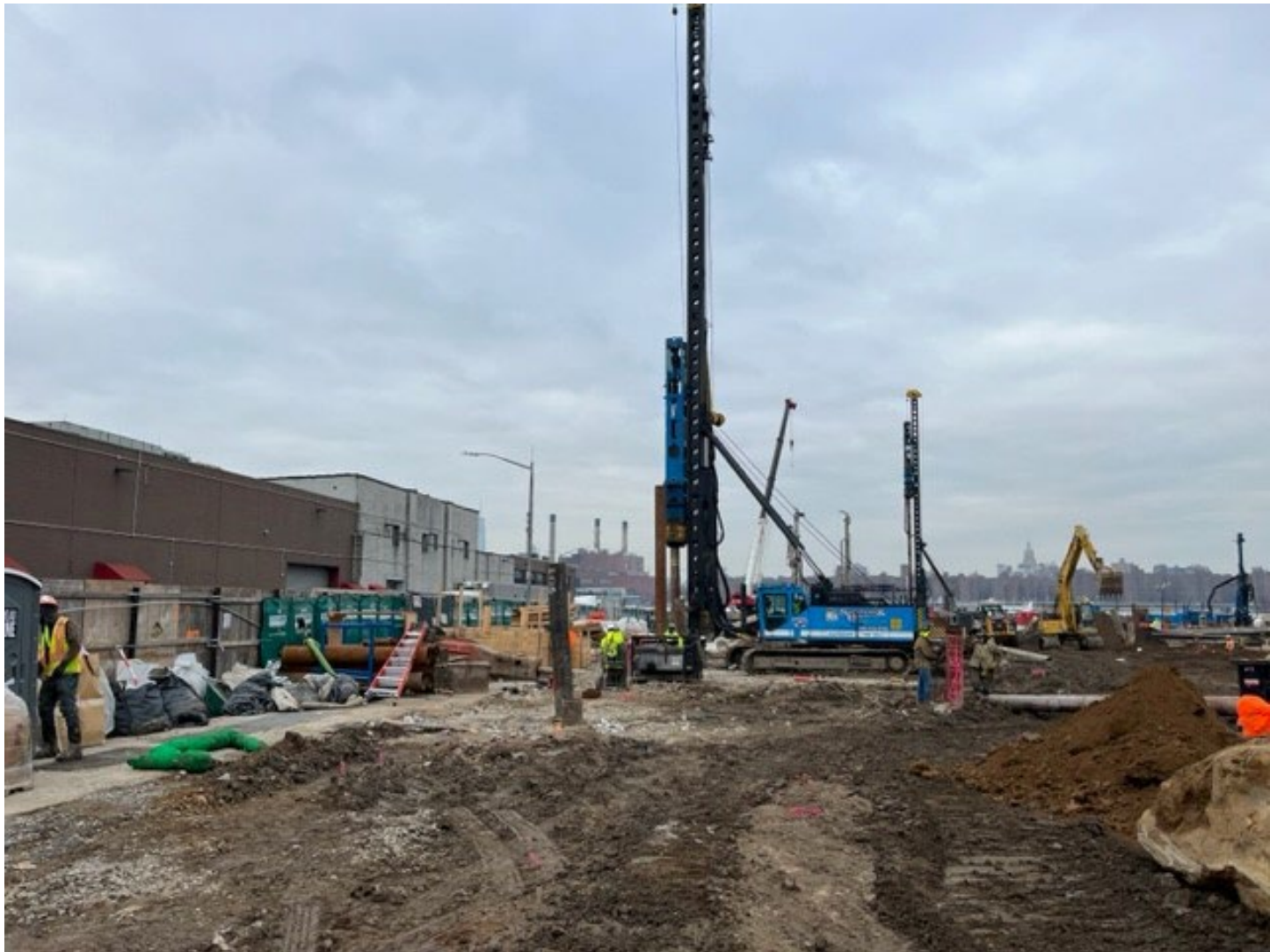
Photo 4: View facing west, Simpson & Brown performing pile driving in grid cell SC-11.
