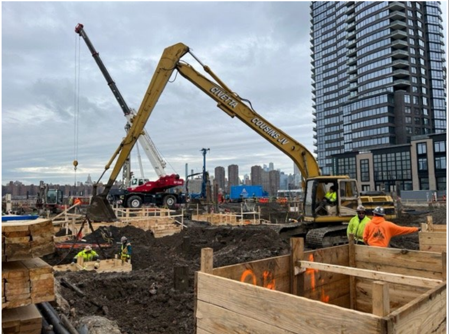
Photo 1: View facing west, CCJV installing foundation footing in grid cell SC-6.
