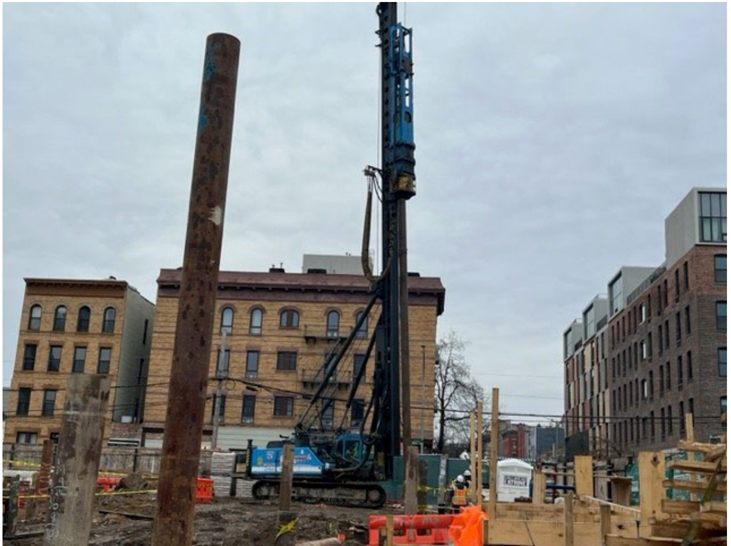
Photo 4: View facing east, Simpson & Brown performing pile driving in grid cell SC-16.
