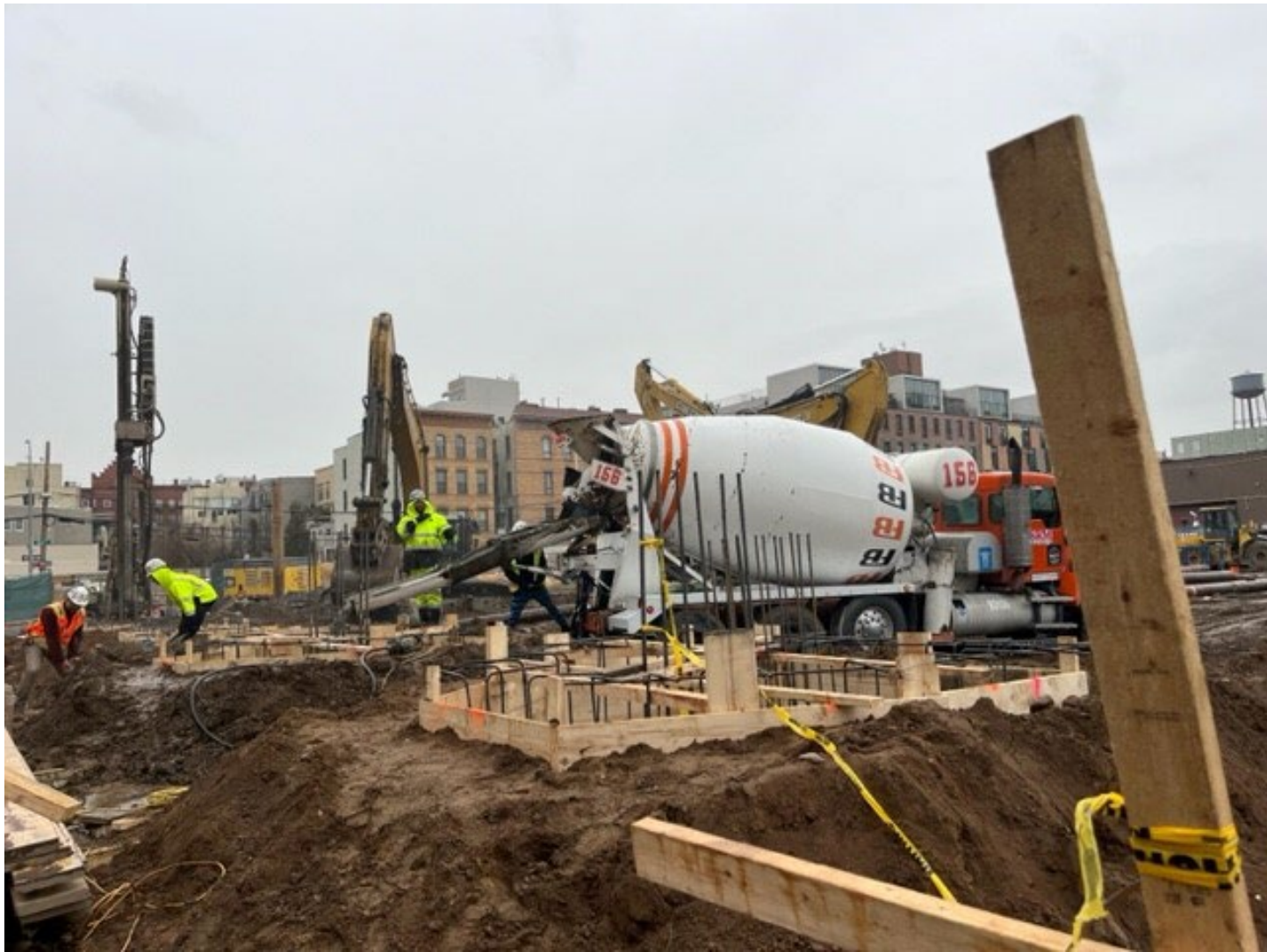
Photo 2: View facing southeast, CCJV pouring concrete into foundation footings in grid cell SC-7.
