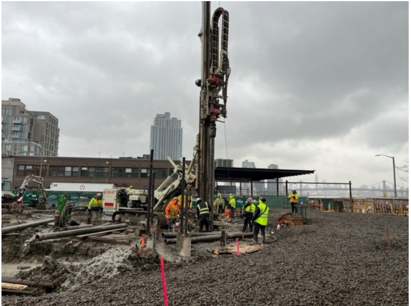
Photo 2: View facing south, CCJV caisson drilling/flushing in grid cell SC-4.
