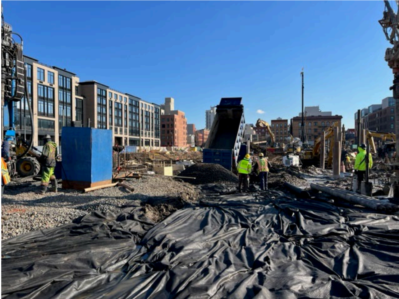
Photo 3: View facing northeast, CCJV imported 1.5" bluestone being delivered on site to be graded in grid cell SC-4 to support geothermal well installation.
