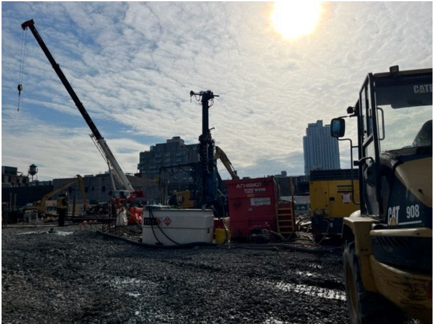
Photo 4: View facing southeast, Brightcore/Geosource drilling geothermal well in grid cell SC-4.
