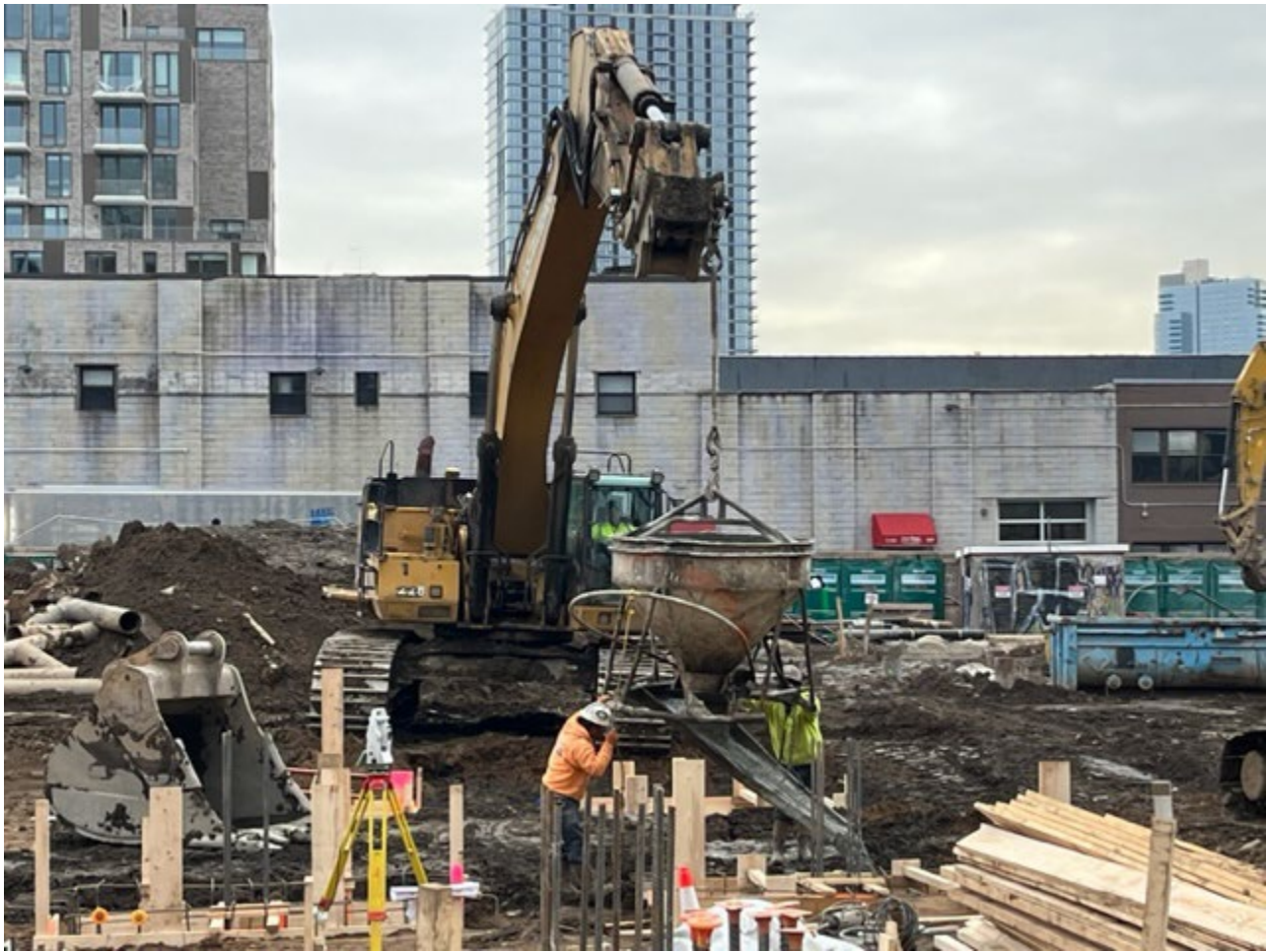
Photo 2: View facing south, CCJV pouring concrete into foundation footing located in grid cell SC-9.
