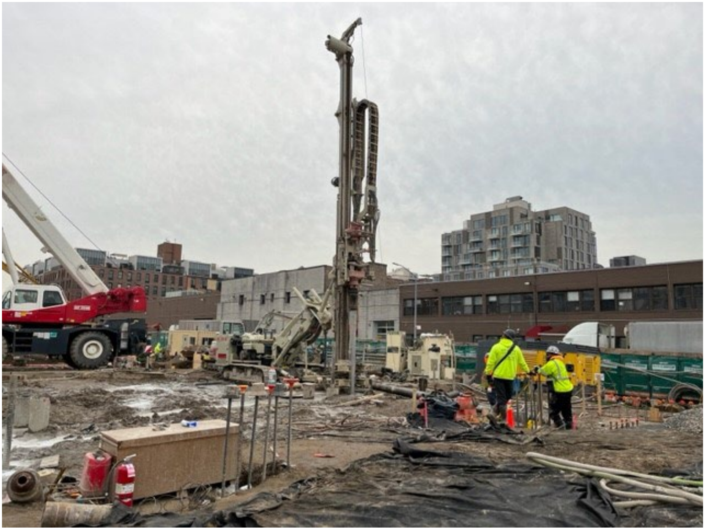
Photo 2: View facing southeast, CCJV caisson drilling/flushing in grid cell SC-4.
