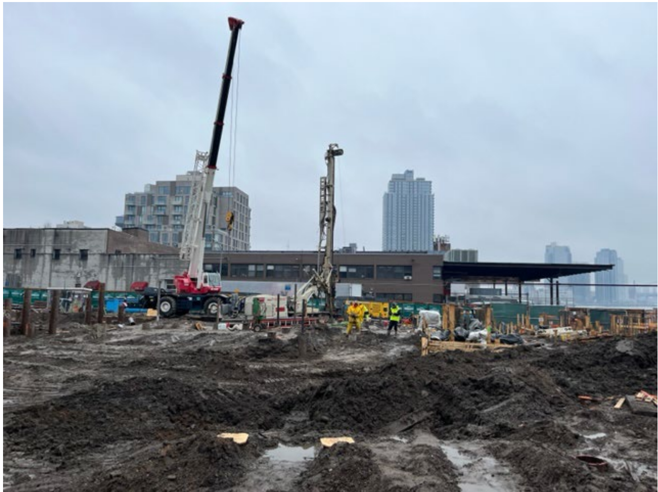
Photo 4: Looking South; CCJV caisson drilling in grid cell SC-4.
