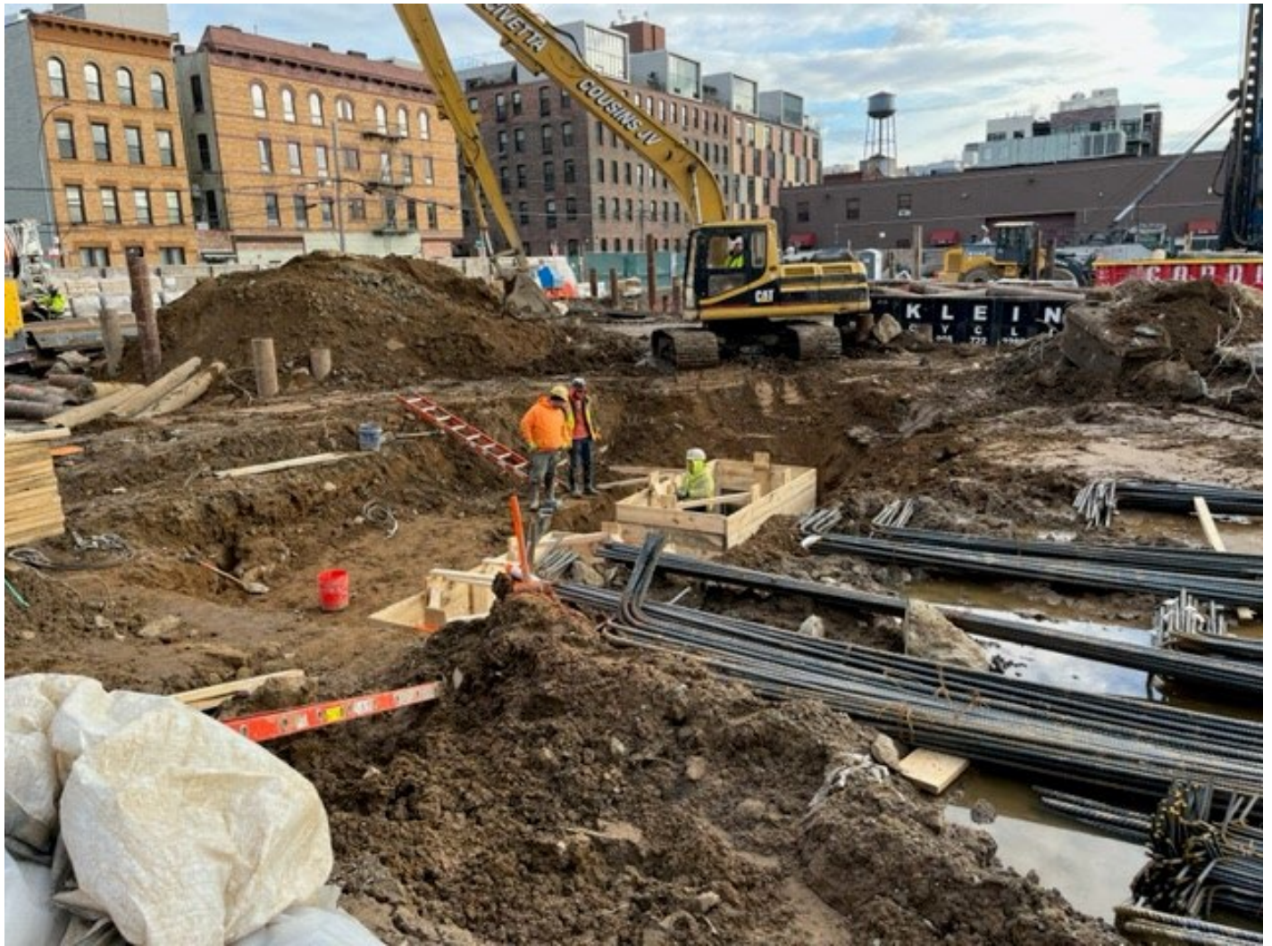
Photo 4: View facing southeast, Atlantic Reinforcing and CCJV installing foundation footing elements, while excavating/backfilling in grid cell SC-12.
