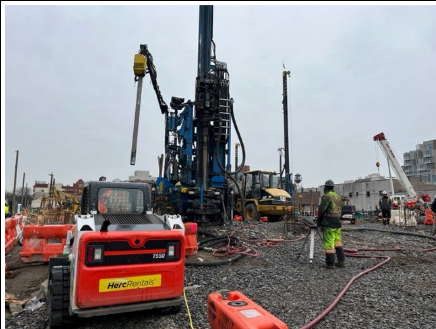
Photo 1: View facing east, Brightcore drilling a geothermal well in grid cell SC-4.
