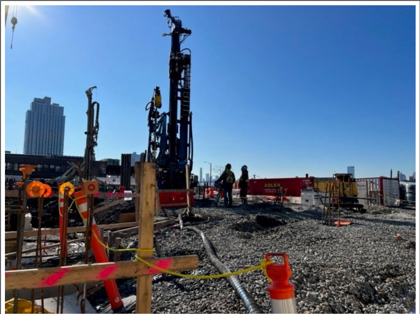
Photo 1: View facing southwest, Brightcore drilling a geothermal well in grid cell SC-4.
