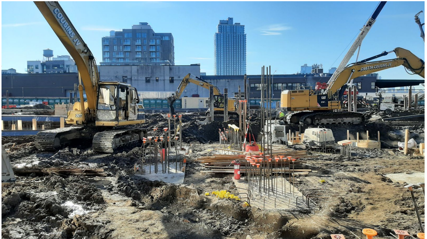
Photo 1: View facing south, CCJV performing excavation in grid cell SC-6 for foundation element installations at the start of the day.
