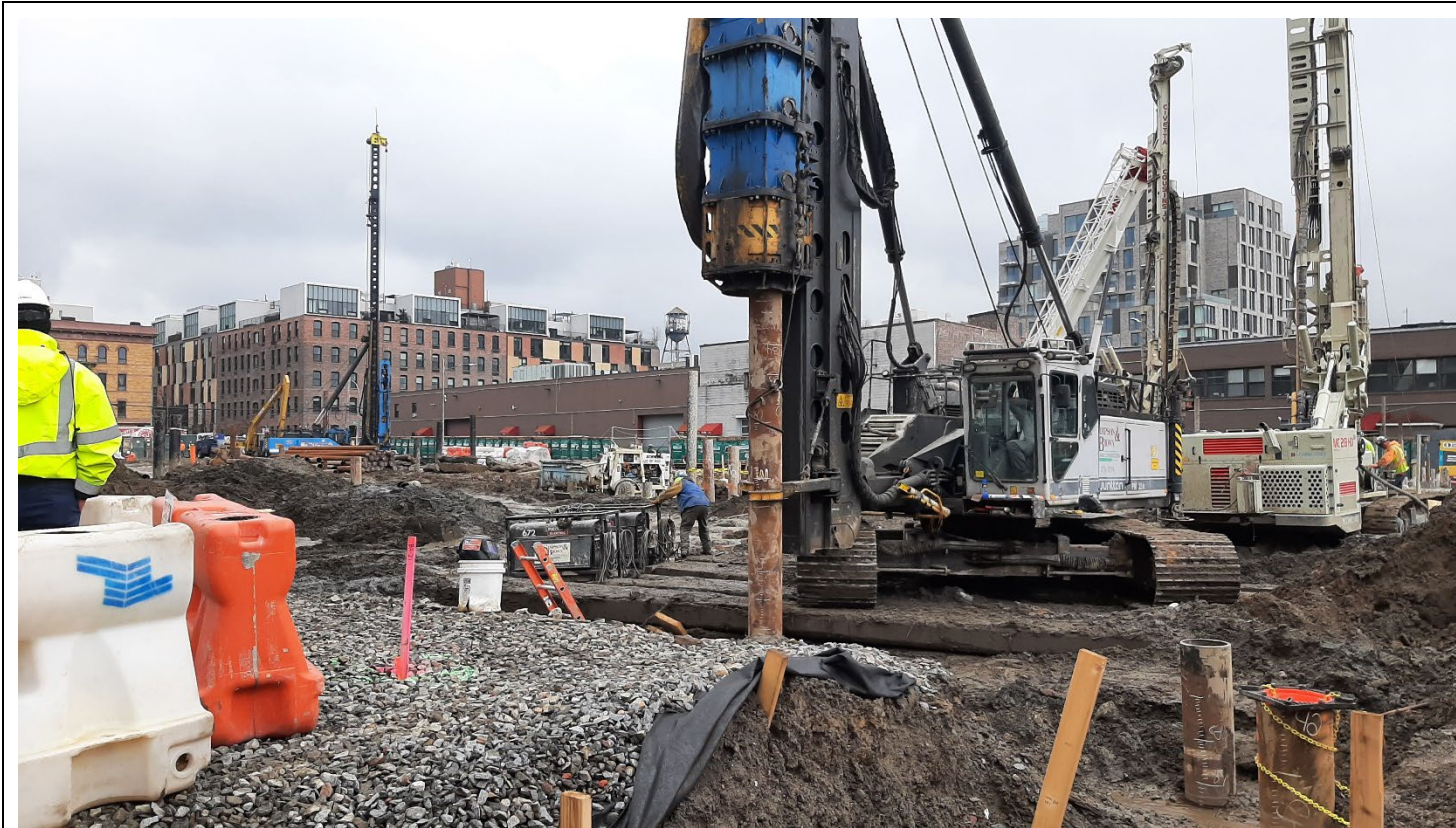
Photo 4: View facing southeast, Simpson & Brown performing pile driving in grid cell SC-4.
