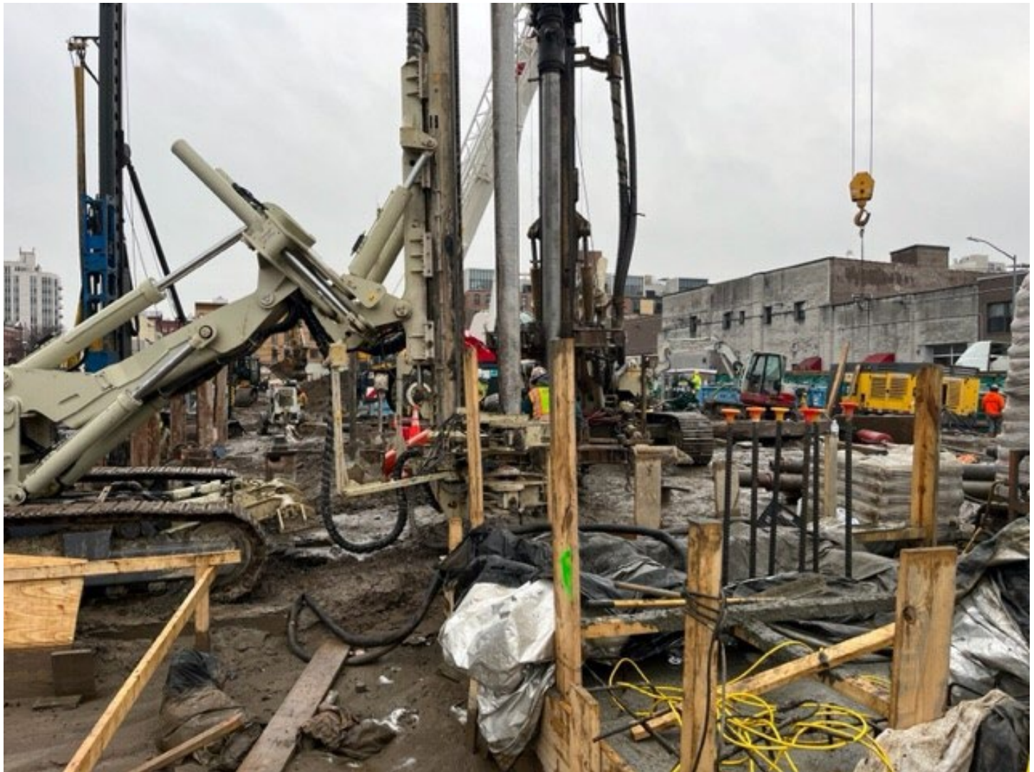
Photo 3: View facing east, CCJV caisson drilling in grid cell SC-4.
