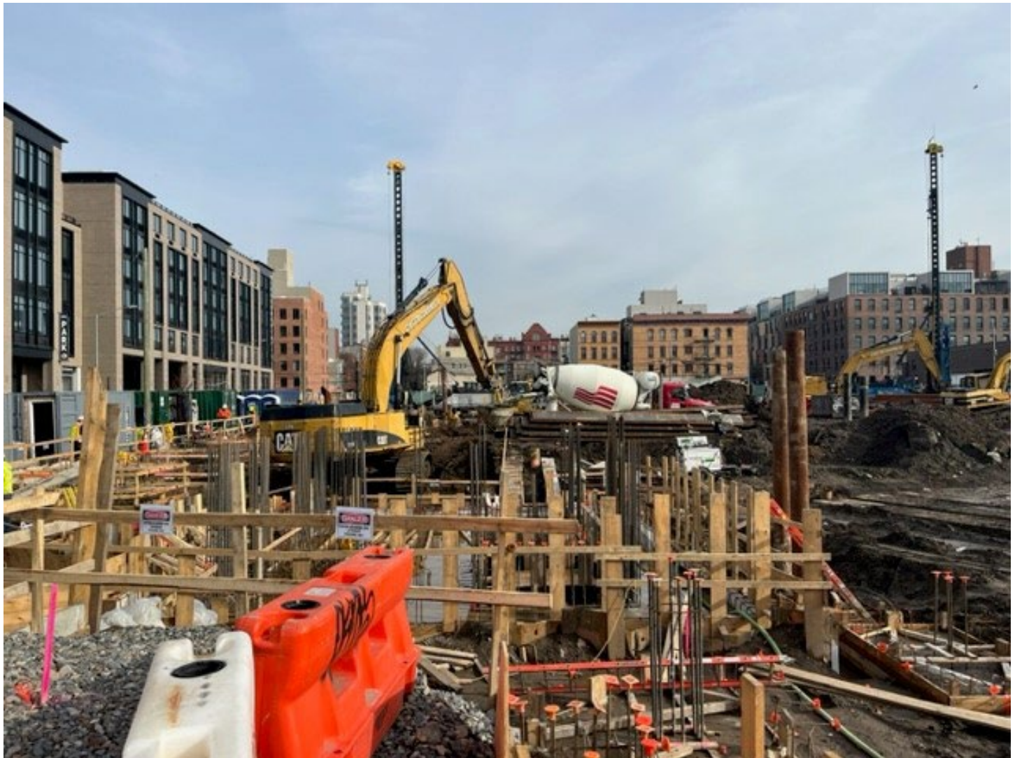
Photo 3: Looking East; CCJV filling foundation elements with concrete in grid cell SC-4.
