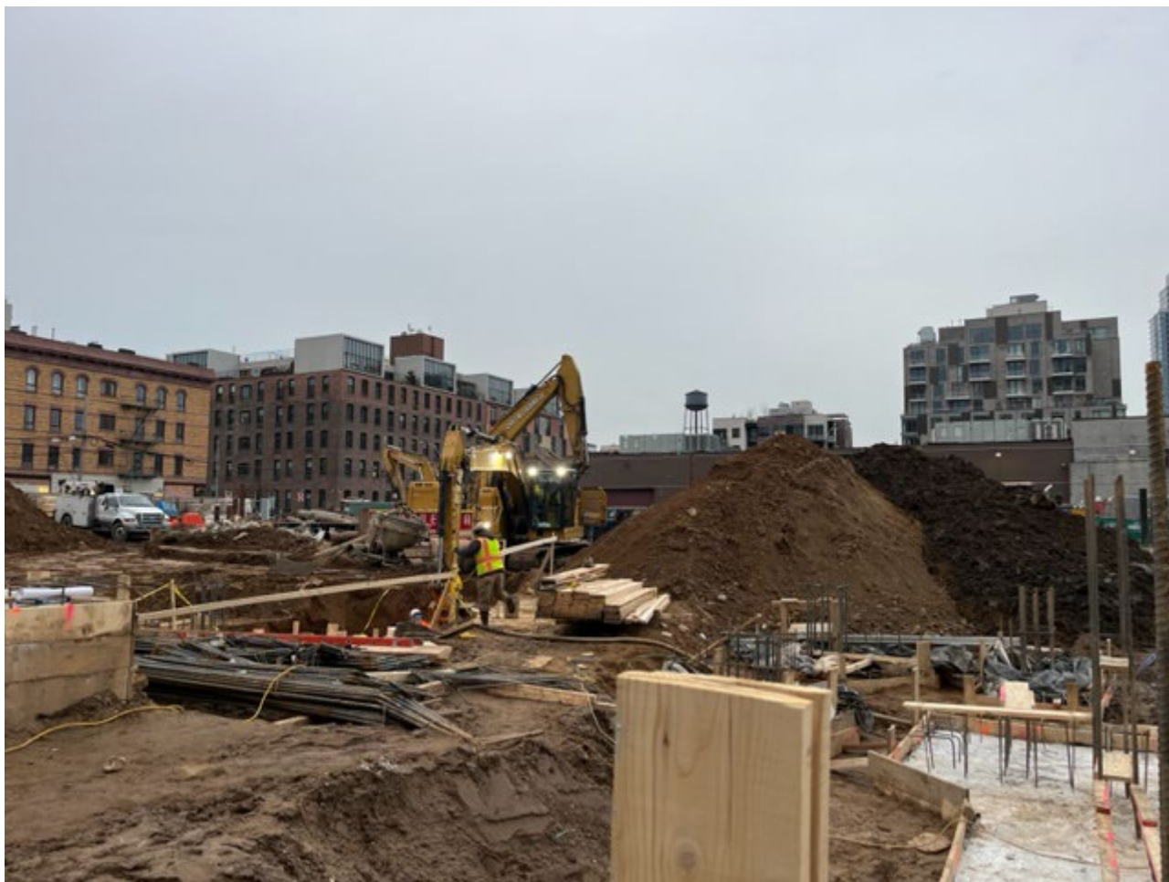
Photo 1: View facing south, CCJV excavating to aid the installation of foundation elements by CCJV and Atlantic Reinforcing in grid cell SC-8.
