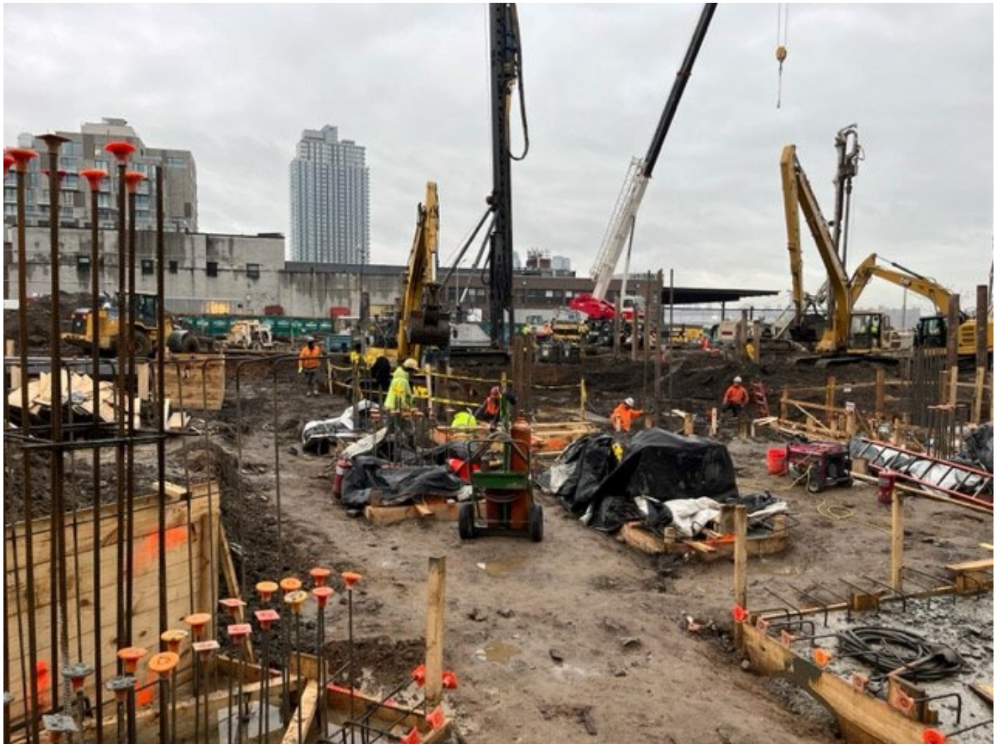
Photo 2: View facing south, CCJV & Atlantic Reinforcing installing foundation elements in grid cells SC-8 and SC-9.
