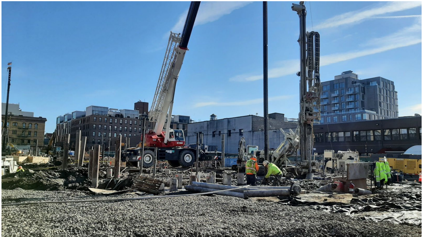
Photo 2: View facing southeast, CCJV inserting steel rods into installed caisson in grid cell SC-4.
