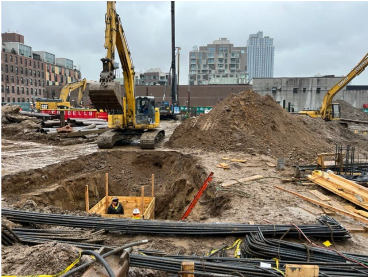
Photo 4: View facing south, Atlantic Reinforcing and CCJV installing foundation footing elements, while excavating/backfilling in grid cells SC-7 and SC-8.
