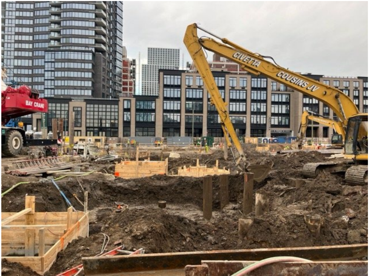
Photo 3: View facing north, CCJV excavating to support foundation footing installation in grid cells SC-5 and SC-6.
