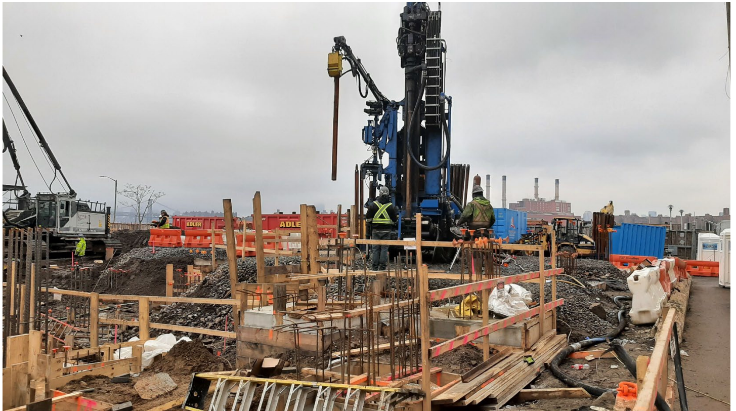
Photo 1: View facing southwest, Brightcore performing geothermal well installation in grid cell SC-4.
