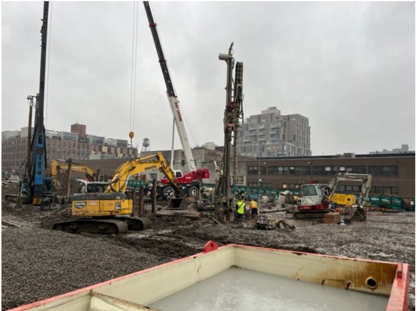
Photo 3: View facing southeast, CCJV performing caisson drilling in grid cell SC-4.
