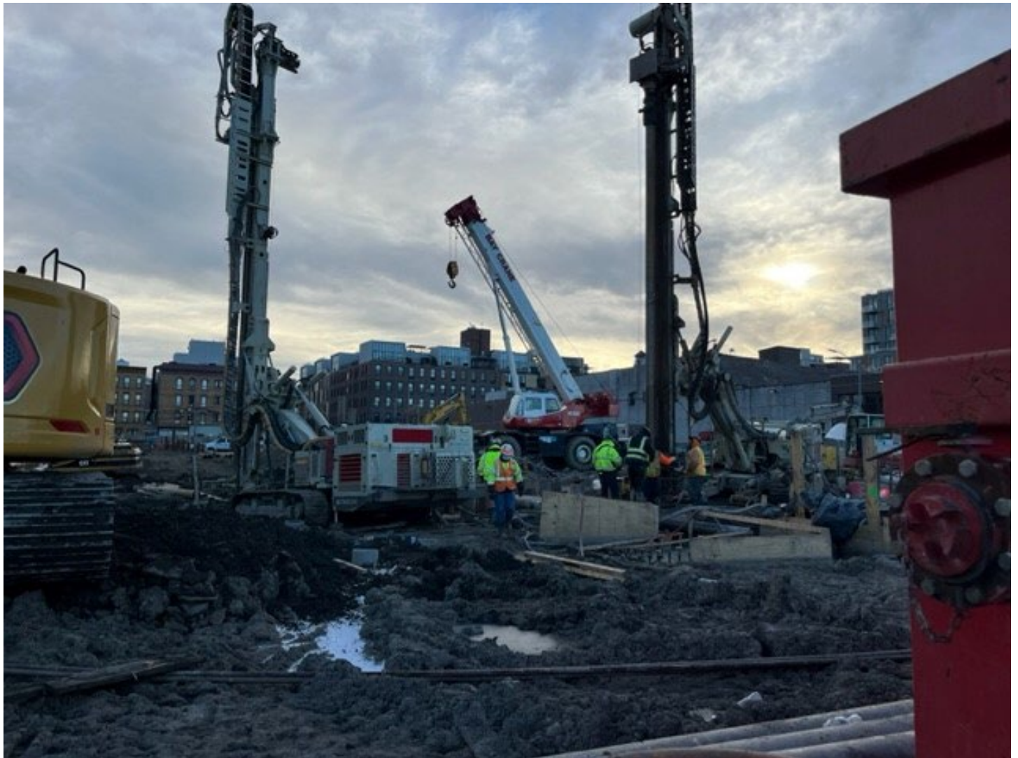
Photo 3: View facing east, CCJV performing caisson drilling in grid cell SC-4.
