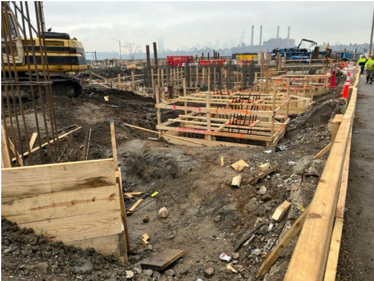
Photo 1: Looking West; CCJV installing foundation footings in grid cell SC-4.
