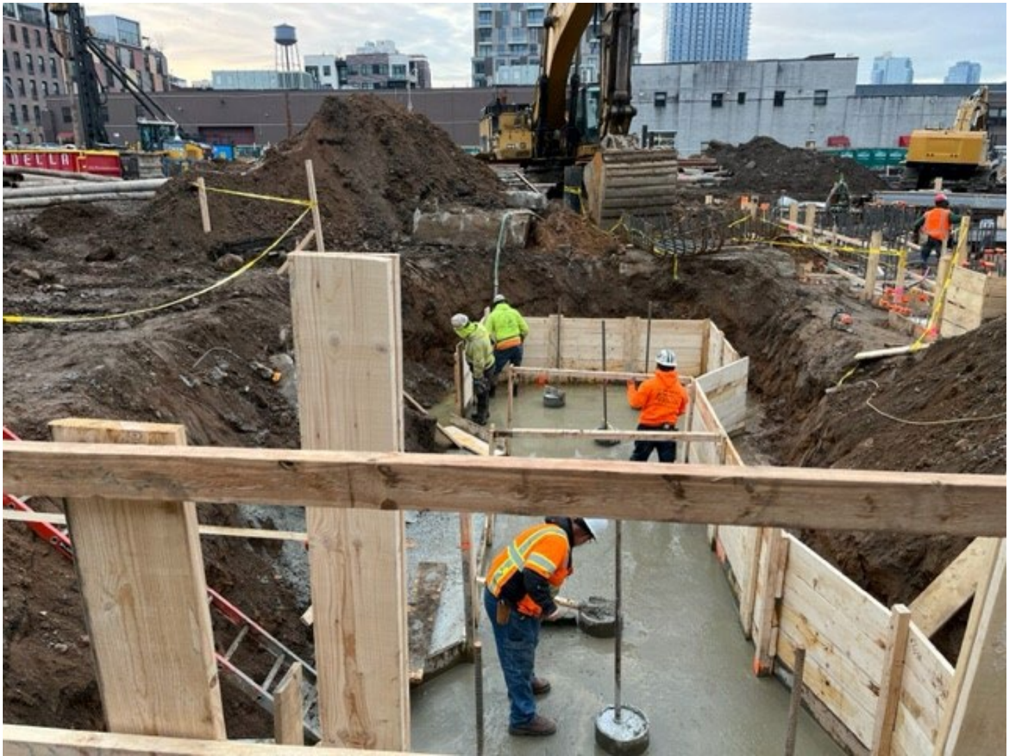
Photo 4: View facing south, CCJV installing foundation footing in grid cells SC-7 and SC-8
