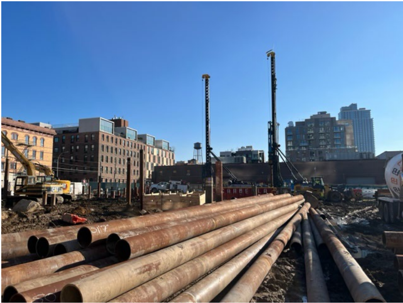
Photo 4: View facing south, Simpson & Brown performing pile driving in grid cell SC-11.
