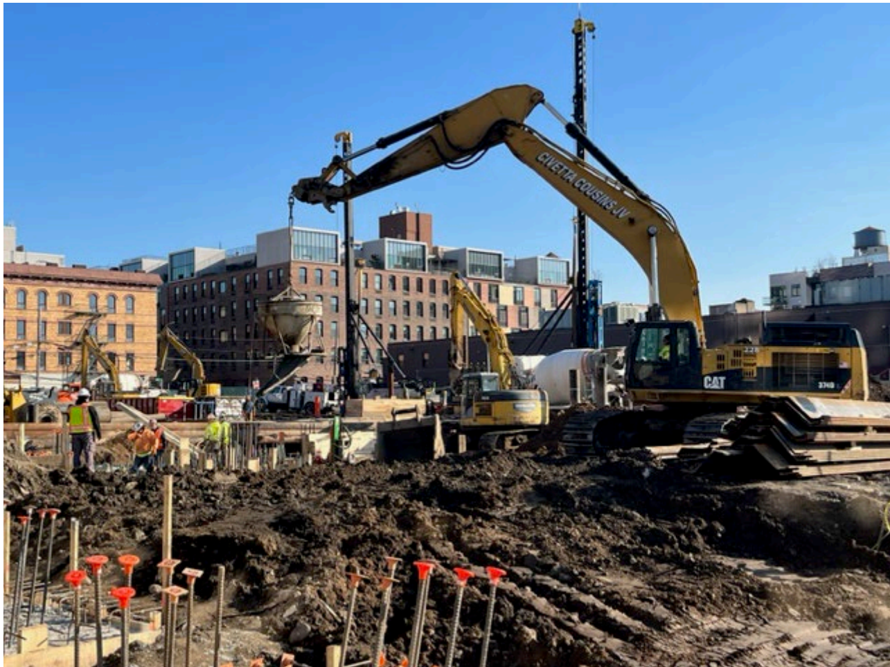
Photo 2: View facing southeast, CCJV filling foundation footings with cement in grid cell SC-8.
