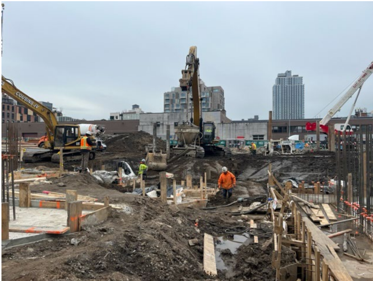
Photo 4: View facing south, CCJV preparing to pour concrete into foundation footings in grid cell SC-8.
