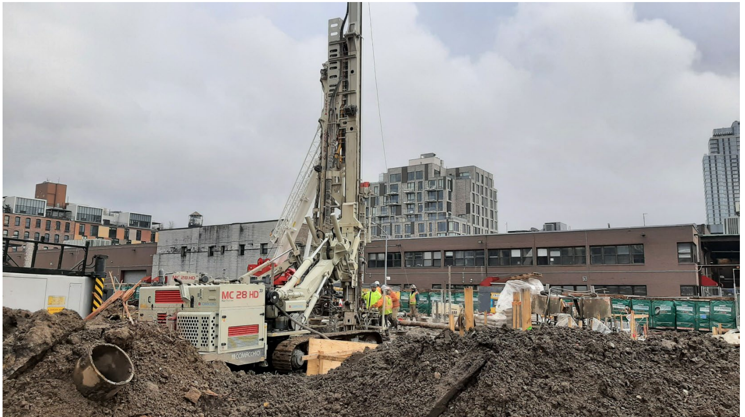
Photo 3: View facing southeast, CCJV performing caisson drilling in grid cell SC-4.
