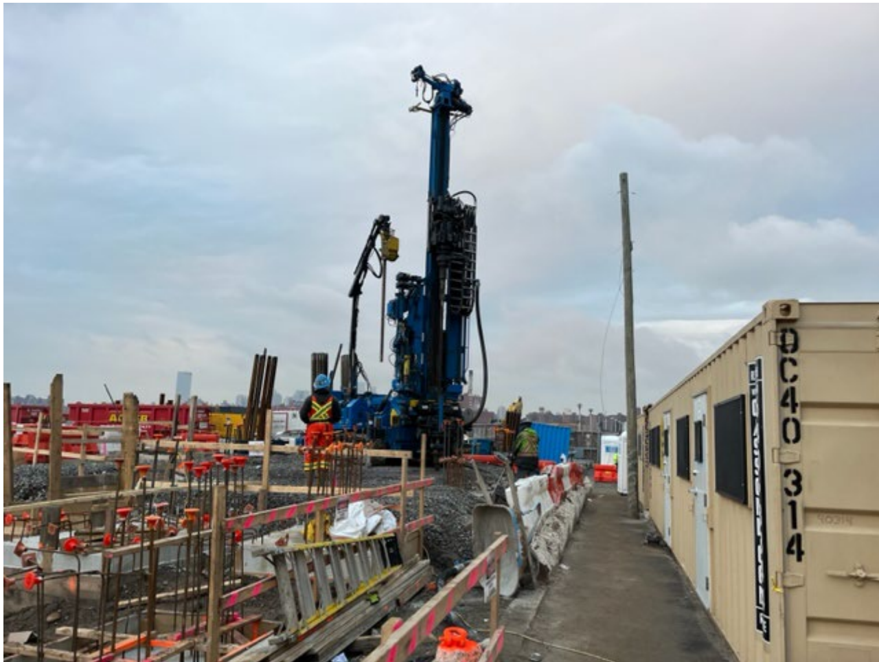
Photo 1: View facing west, Brightcore performing geothermal well installation in grid cell SC-4.
