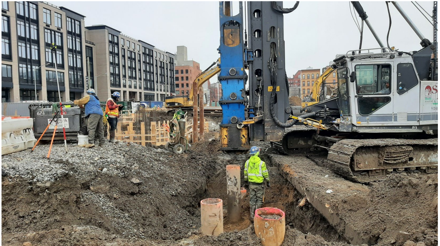
Photo 4: View facing east-northeast, Simpson & Brown performing pile driving in grid cell SC-4.
