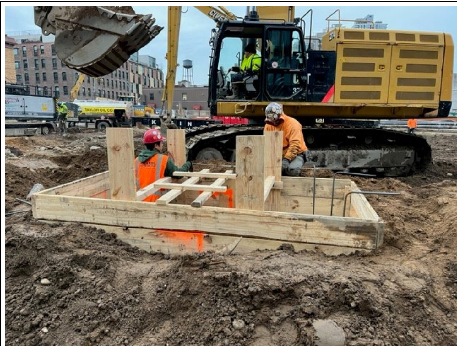
Photo 4: View facing south, Atlantic Reinforcing and CCJV installing foundation footing elements, while excavating/backfilling in grid cell SC-12.
