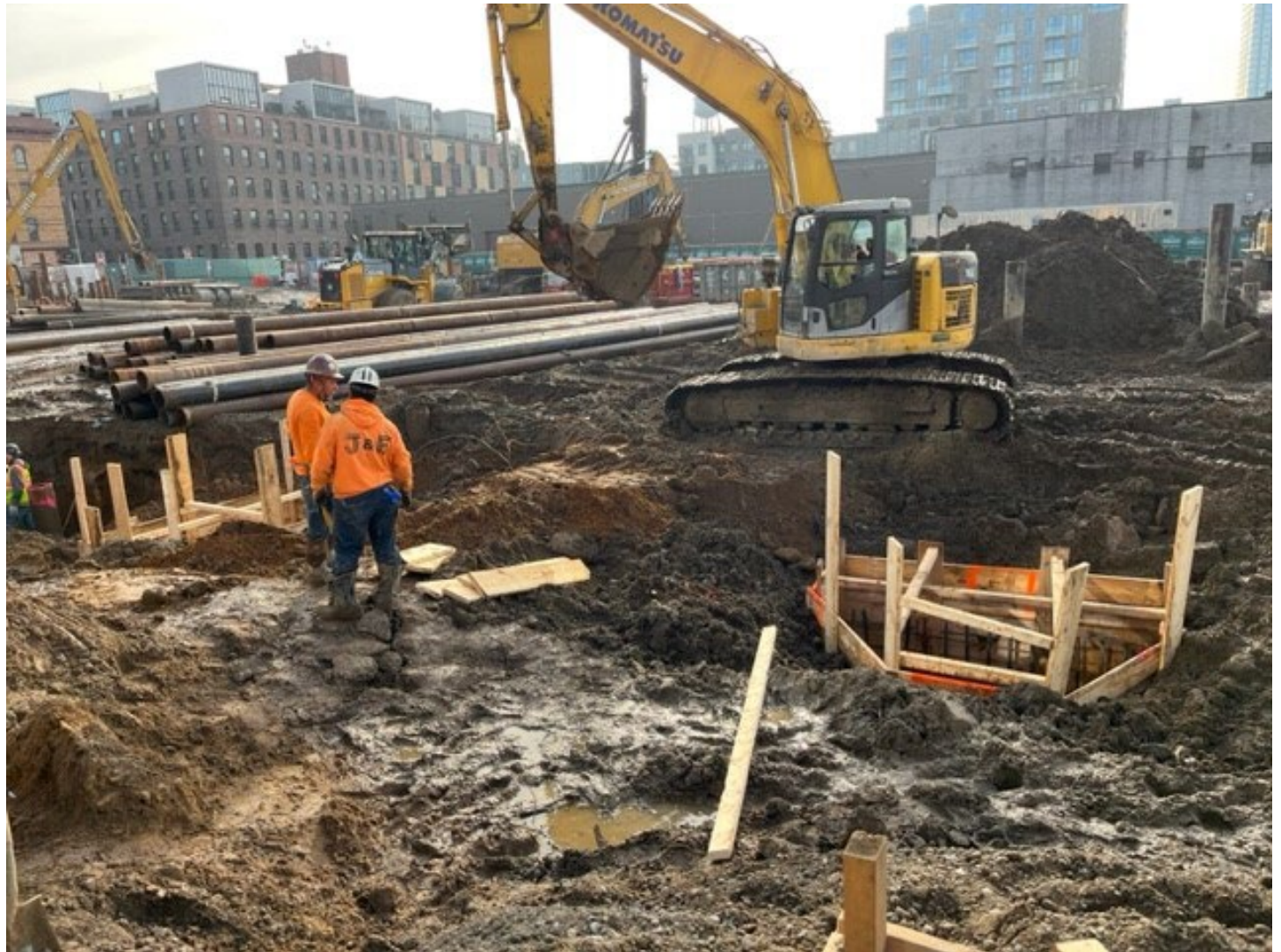
Photo 1: Looking Southeast; CCJV backfilling in grid cell SC-7 while installing foundation footings.
