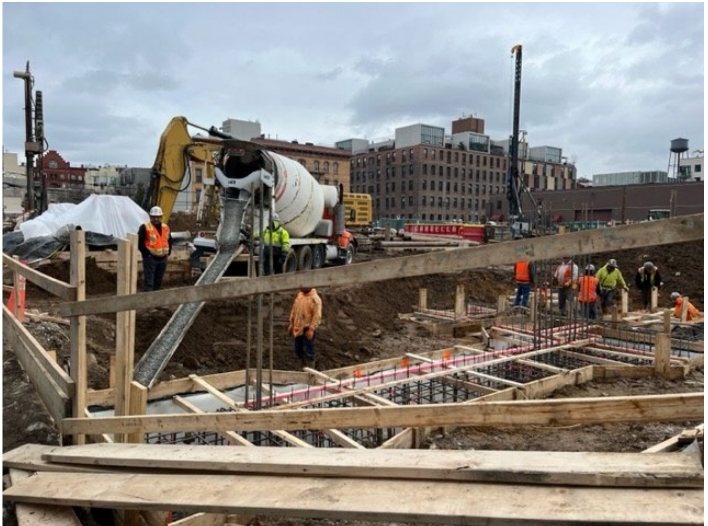
Photo 2: View facing southeast, CCJV pouring concrete into foundation footings in grid cells SC-7 and SC-8.
