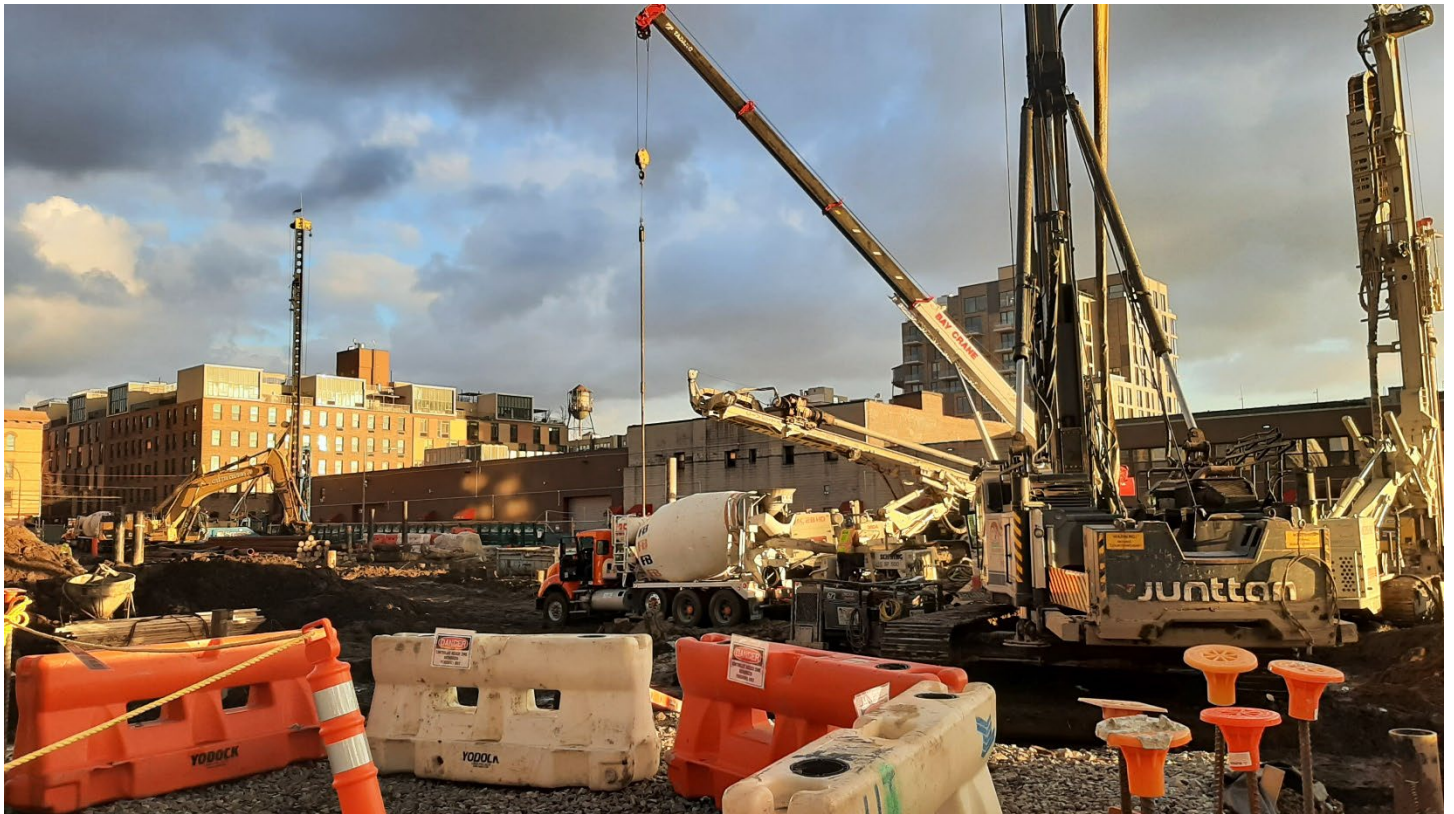
Photo 2: View facing southeast, CCJV filling caissons with cement and installing rebar.
