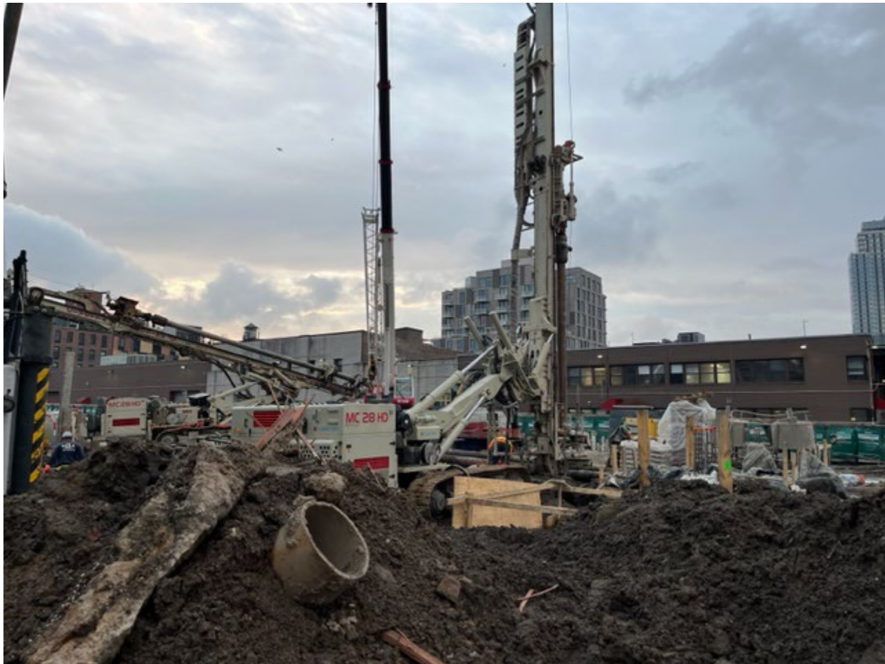
Photo 3: View facing southeast, CCJV preparing to begin caisson drilling in grid cell SC-4.
