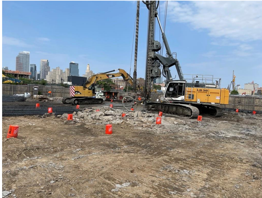
Photo 1: JEL installing a building foundation displacement pile in the southeast part of the site (facing north)
