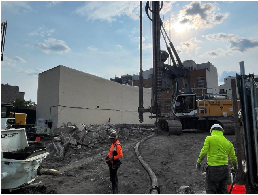
Photo 1: JEL installing a building foundation displacement pile in the northwest part of the site (facing west)
