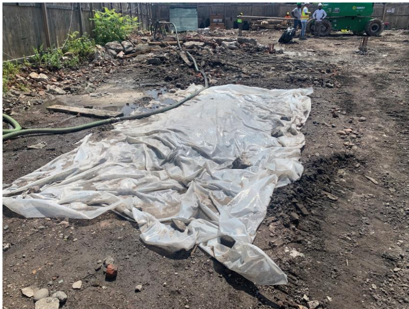
Photo 2: Stockpiled drilling spoils on and covered with polyethylene sheeting in the northern part of the site (facing east)
