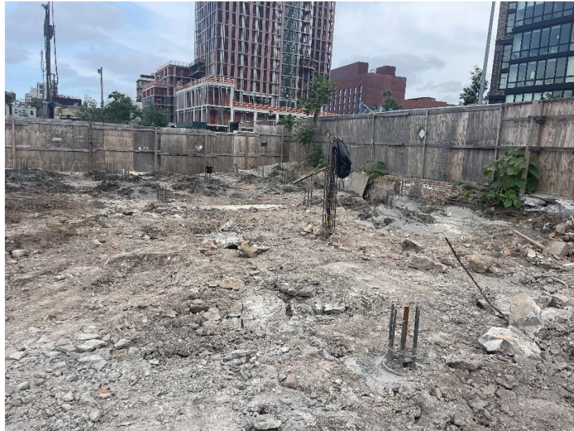
Photo 1: View of building foundation displacement piles in the southeast part of the site (facing southeast)
