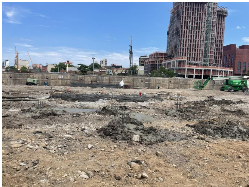
Photo 2: Building foundation displacement piles in the central part of the site (facing east)
