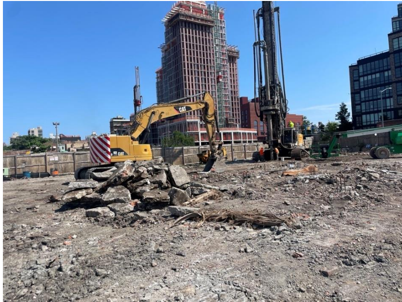
Photo 1: JEL advancing a building foundation displacement pile in the southeast part of the site (facing southeast)
