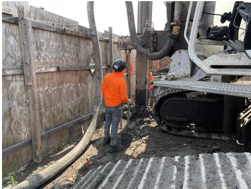
Photo 2: JEL installing a building foundation displacement pile in the northeastern part of the site (facing east)
