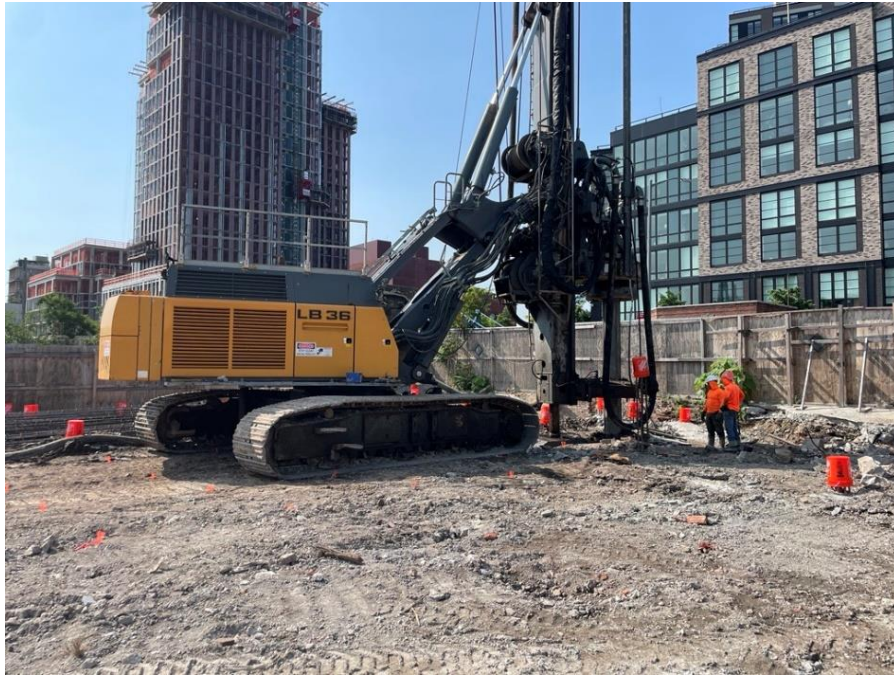
Photo 1: JEL installing a foundation displacement pile in the southeast part of the site (facing southeast)
