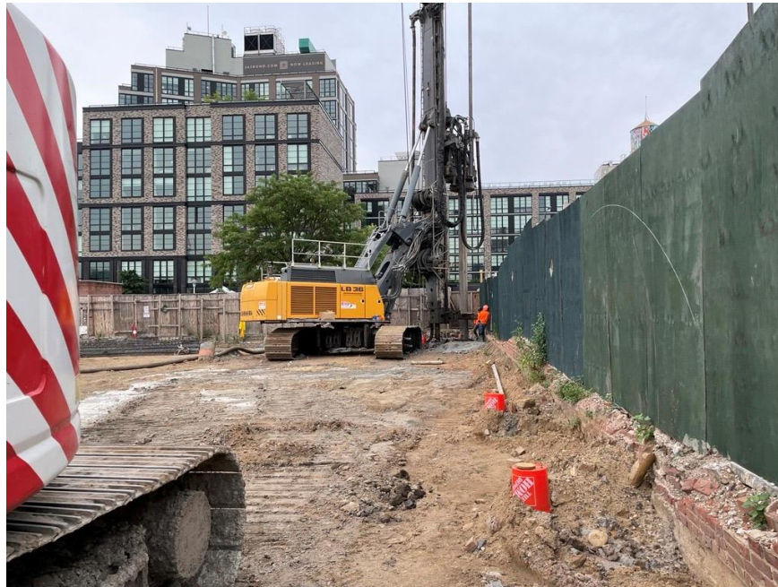
Photo 1: JEL installing a building foundation displacement pile in the southwestern part of the site (facing south)
