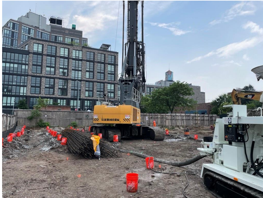
Photo 1: JEL installing a building foundation displacement pile in the southwest part of the site (facing south)
