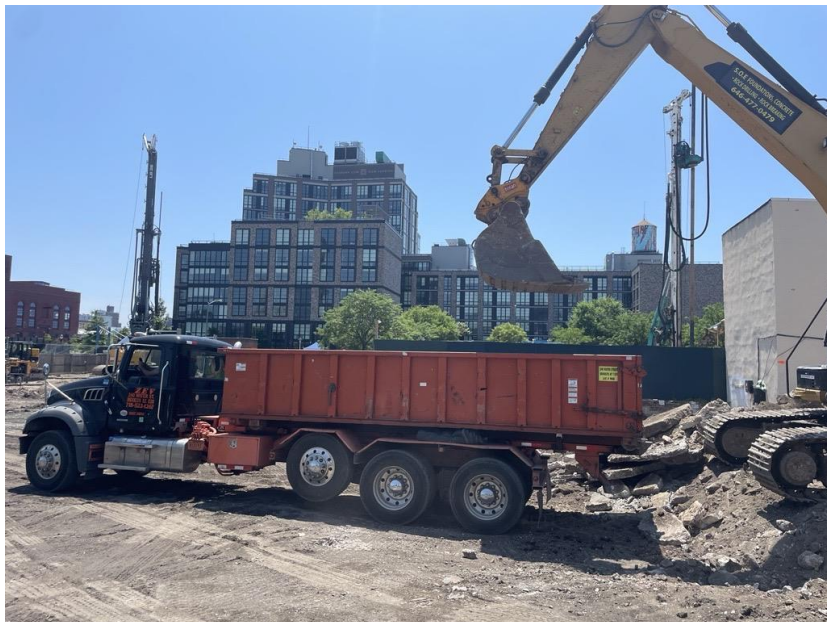
Photo 2: JEL loading a truck with C&D for off-site disposal (facing south)
