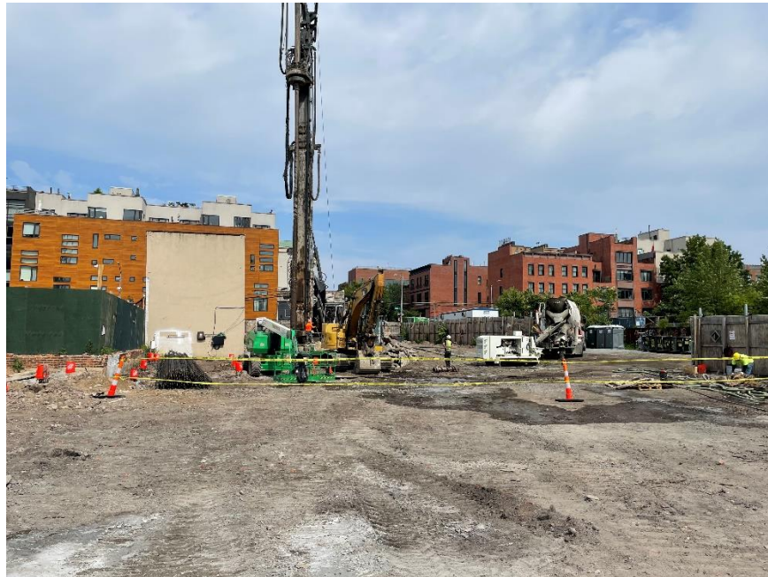
Photo 1: JEL installing a building foundation displacement pile in the northwest part of the site (facing northwest)
