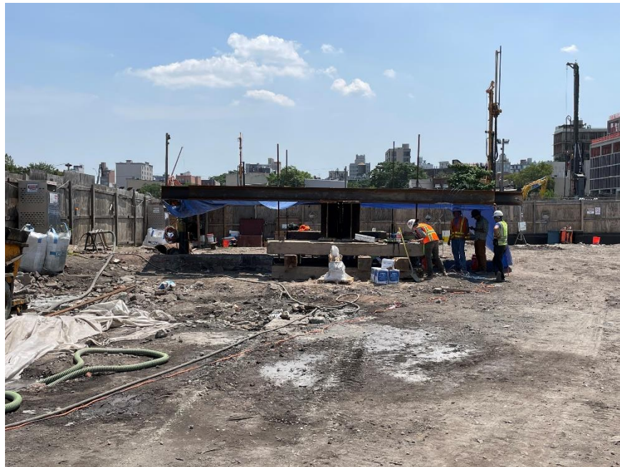
Photo 2: View of the foundation pile load test in the central part of the site (facing southeast)
