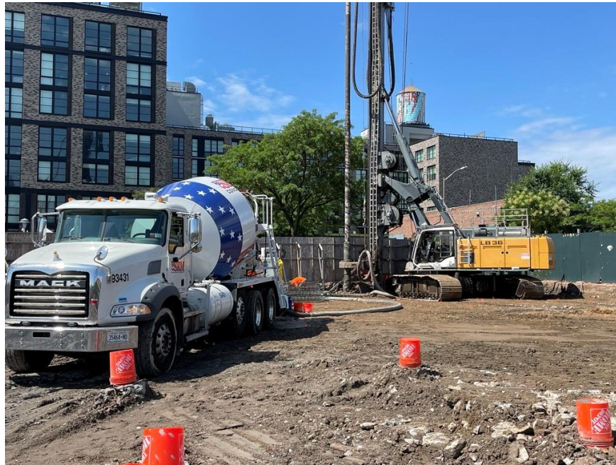
Photo 1: JEL installing a building foundation displacement pile in the southwestern part of the site (facing southwest)
