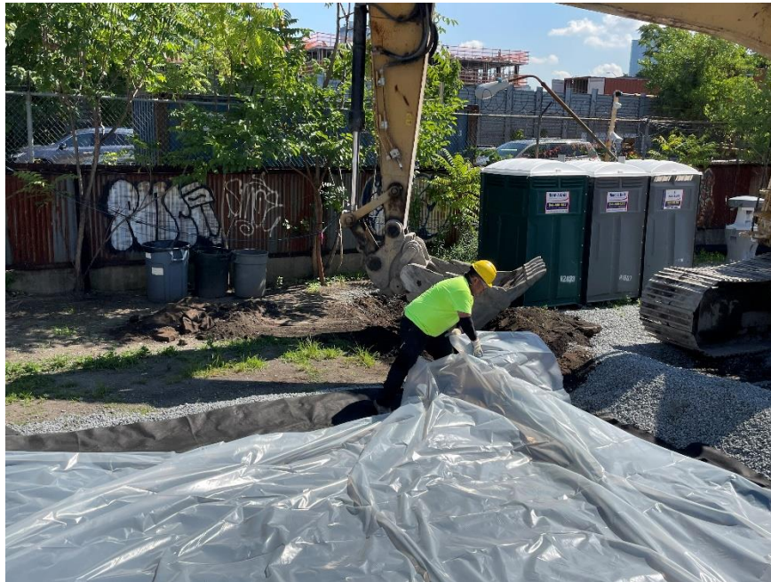
Photo 1: JEL installing a truck wash in the northwest part of site (facing east)
