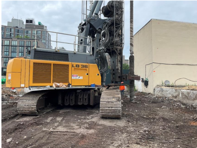
Photo 1: JEL installing a foundation displacement pile in the southeast part of the site (facing east)
