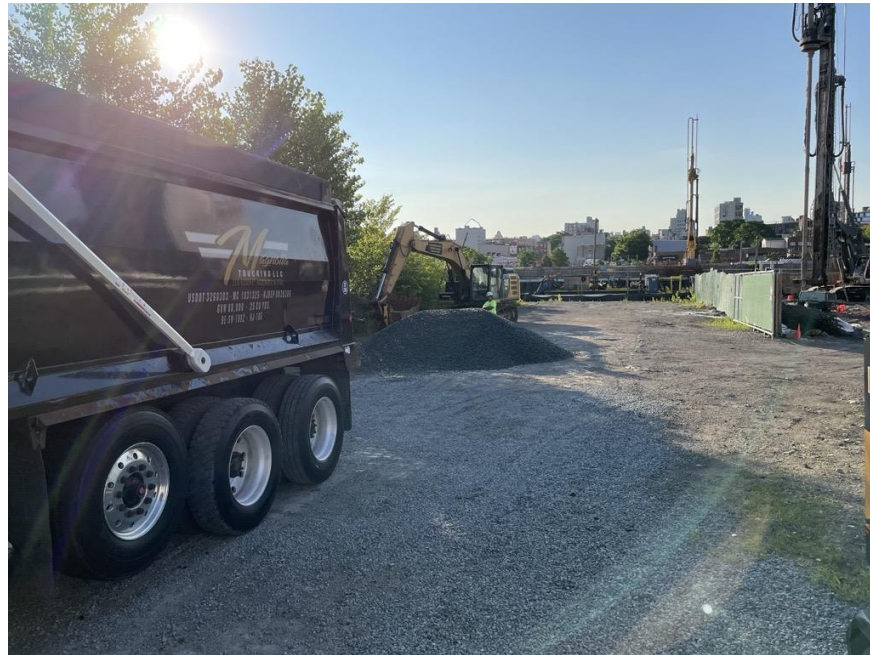
Photo 1: View of imported 3/4-inch virgin stone placed in the western part of the site for maintenance of the stabilized construction entrance (facing east)
