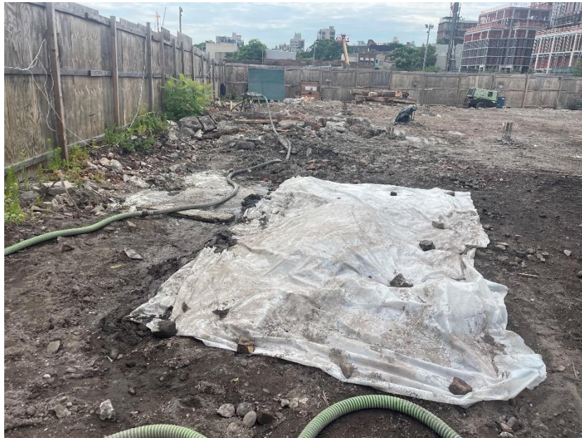
Photo 1: Stockpiled drilling spoils on and covered with polyethylene sheeting in the northern part of the site (facing east)
