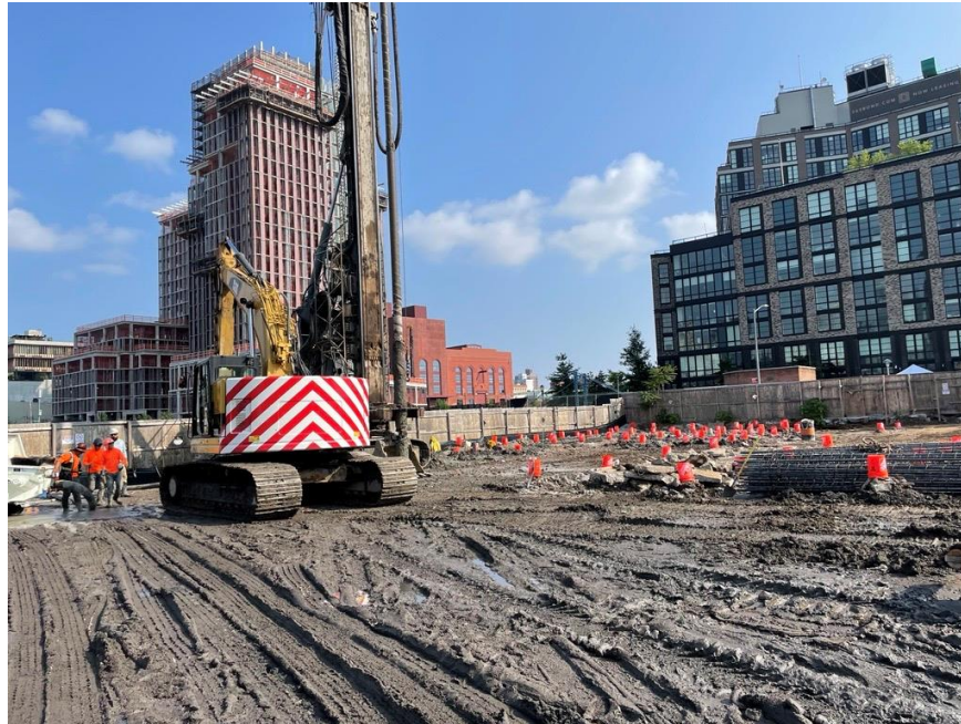
Photo 1: JEL installing a building foundation displacement pile in the southeast part of the site (facing east)
