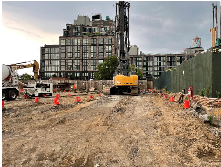
Photo 2: JEL installing a building foundation displacement pile in the southwestern part of the site (facing south)
