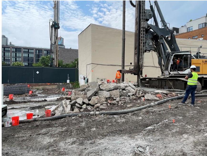
Photo 1: JEL installing a building foundation displacement pile in the northwest part of the site (facing south)
