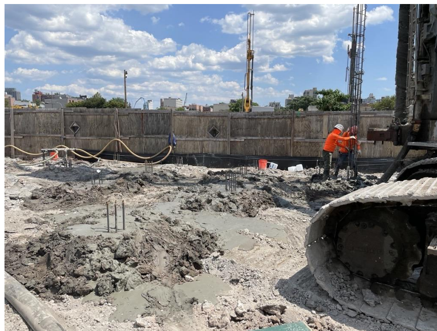
Photo 2: JEL installing a building foundation displacement pile in the northeastern part of the site (facing north)
