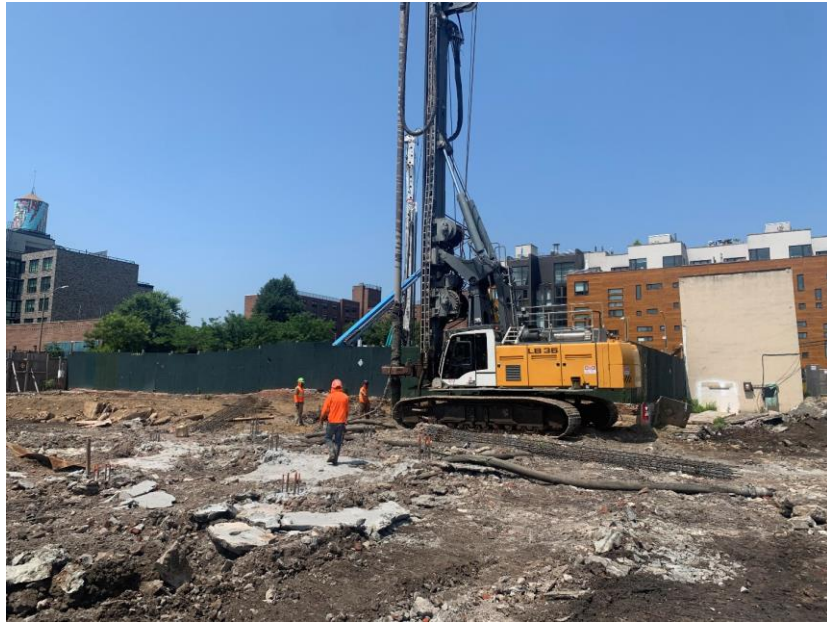
Photo 1: JEL advancing a building foundation displacement pile in the central part of the site (facing west)
