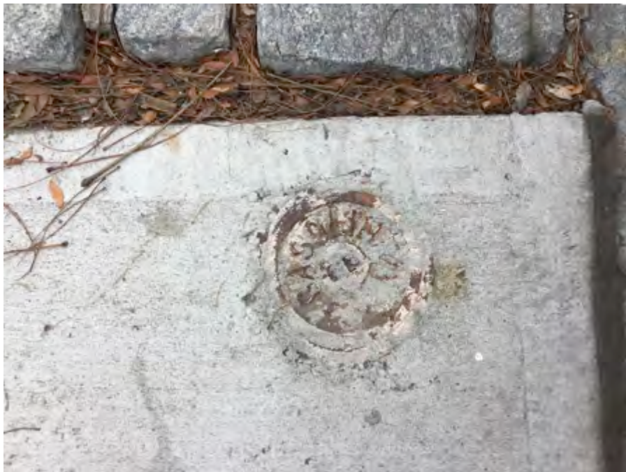
A gasoline fill cap on the southern property boundary along Clay Street.
