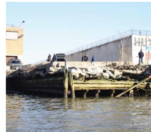
FIGURE 2-11: LOW-LEVEL PLATFORM, HURON STREET
