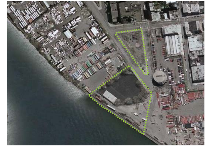
FIGURE 5-7: EXISTING SITE PHOTO OF NEWTOWN BARGE TERMINAL AND GREENPOINT PLAYGROUNDS
