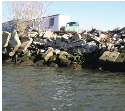
FIGURE 2-5: CONCRETE RUBBLE SLOPE, COMMERCIAL STREET & FRANKLIN STREET
