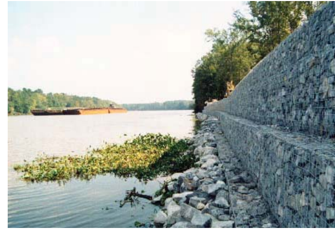
FIGURE 6-33: RIPRAP AND GABION WALLS, PHOTO COURTESY OF THE INTERNATIONAL EROSION CONTROL ASSOCIATION
