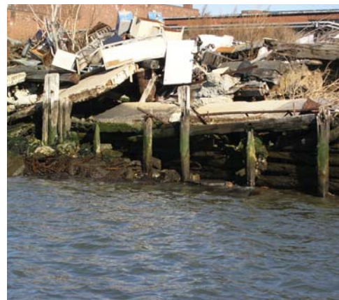
FIGURE 2-10: TIMBER CRIB WALL, BUSHWICK INLET
