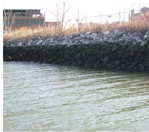
FIGURE 2-6: STONE RIPRAP SLOPE, KENT STREET
