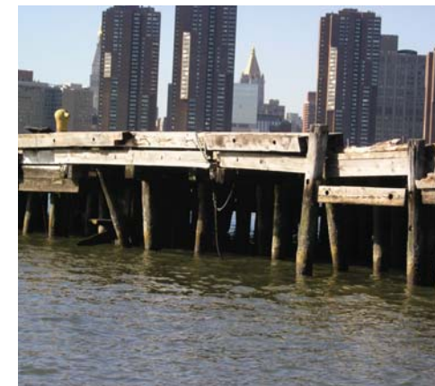
FIGURE 2-12: HIGH-LEVEL PLATFORM, GREEN STREET PIER
