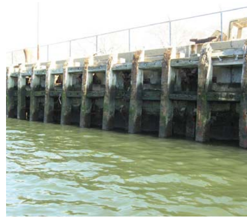
FIGURE 2-7: TIMBER BULKHEAD WALL, MANHATTAN AVE.
