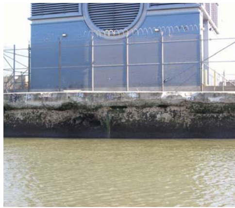
FIGURE 2-9: CONCRETE SEAWALL, N. 7TH STREET
