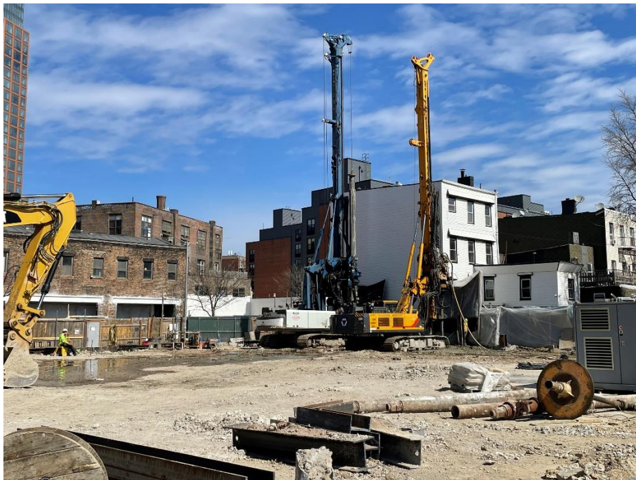
Photo 2: Alternate view of soil mix wall installation facing northeast.
