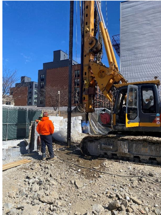
Photo 1: View of drill rig for installation of soil mix wall.
