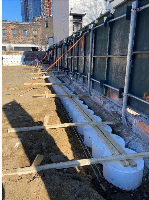
Photo 1: View of styrofoam formwork installation along northeastern perimeter of site.
