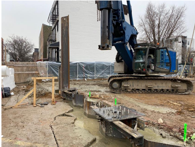
Photo 1: View of sheet pile installation along northeastern perimeter of the site.
