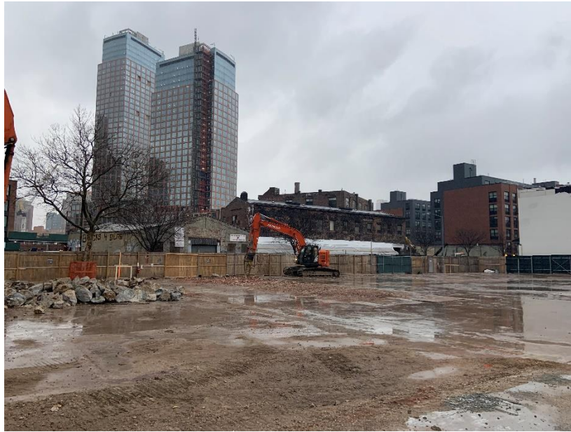
Photo 1: View of contractor preparing for sheet pile installation.
