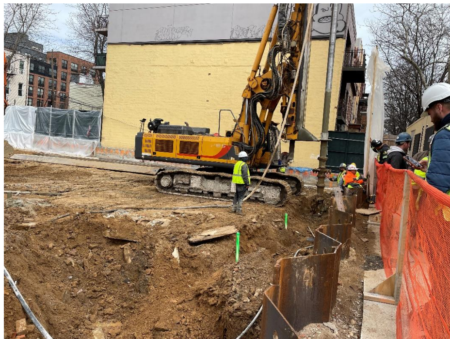
Photo 2: Alternate view of soil mix wall installation facing east.
