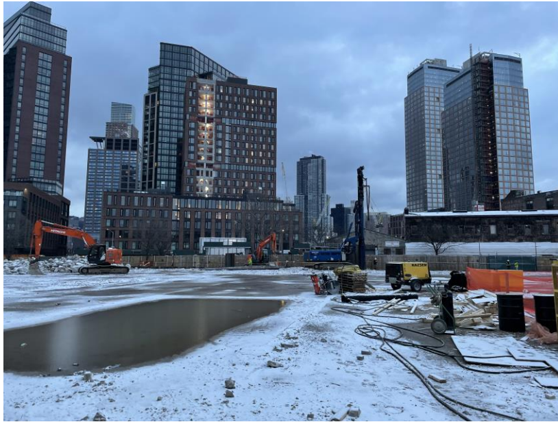
Photo 1: View of contractor installing sheet pile wall along Clay Street.
