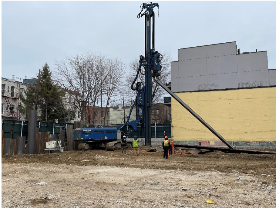
Photo 1: View of sheet pile wall installation in Lot 57.
