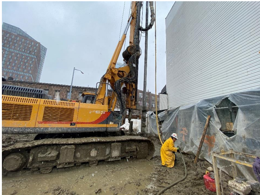
Photo 2: Alternate view of soil mix wall installation facing north.
