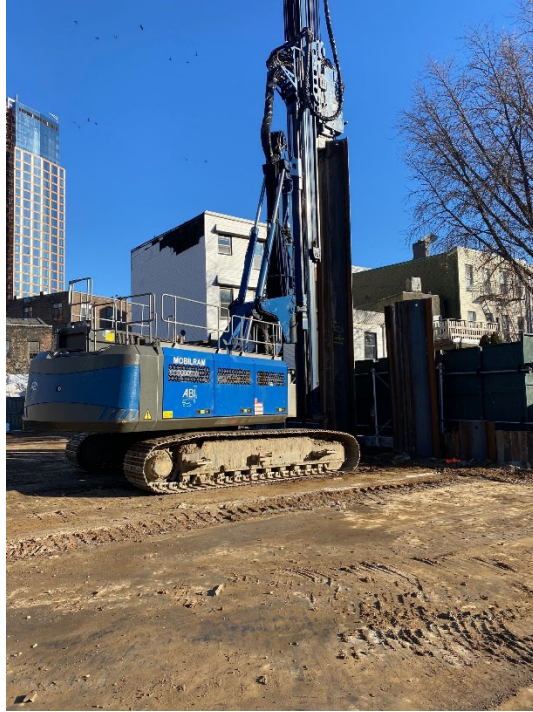
Photo 1: View of sheet pile wall installation along eastern perimeter of site.
