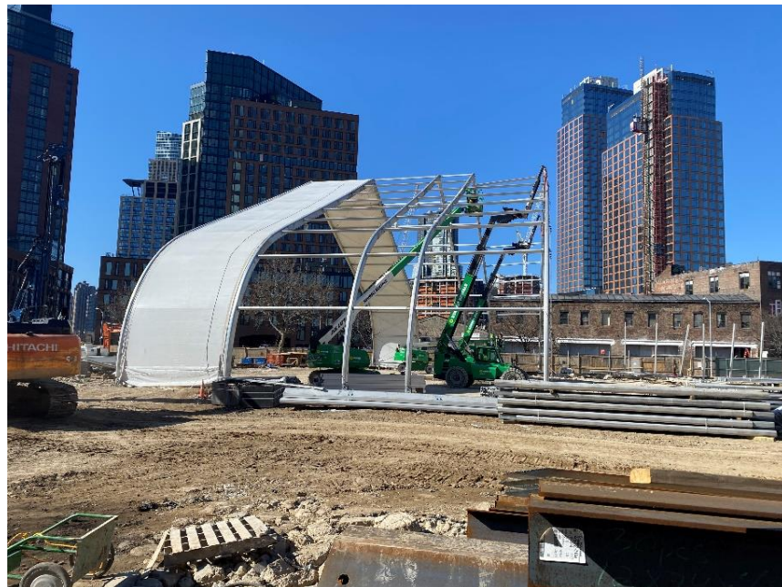
Photo 2: Alternative view of tent structural support steel installation facing northwest.
