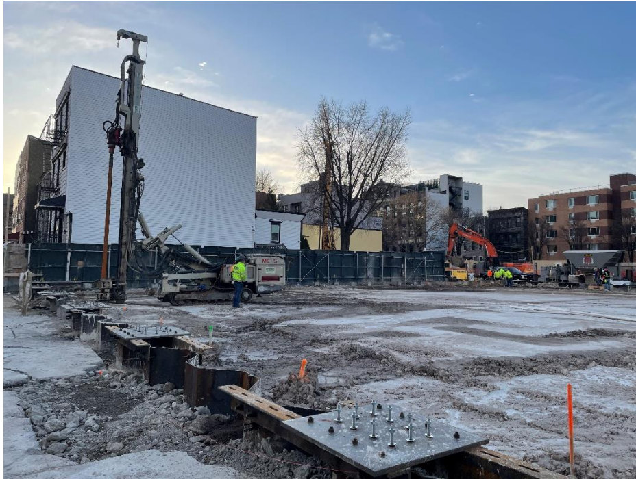
Photo 1: View of contractor installing dewatering point.
