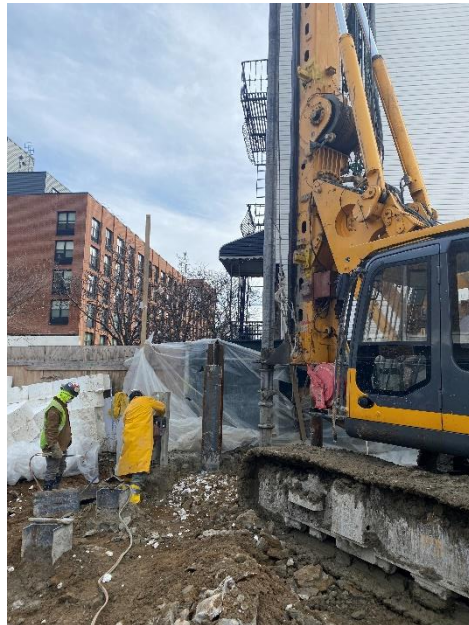
Photo 2: Alternate view of soil mix wall installation.
