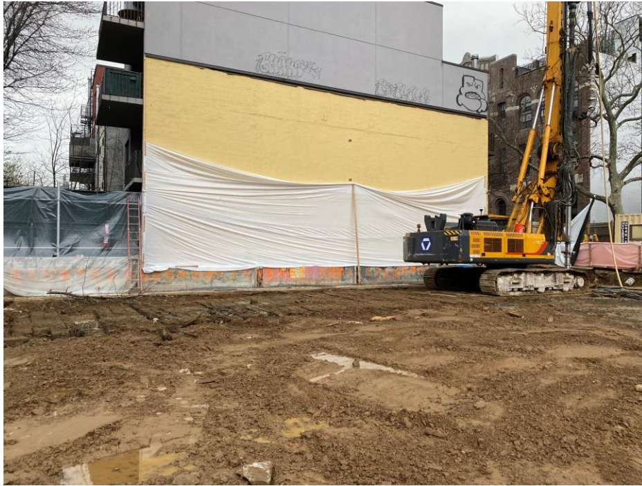
Photo 1: View of soil mix wall installation facing east.
