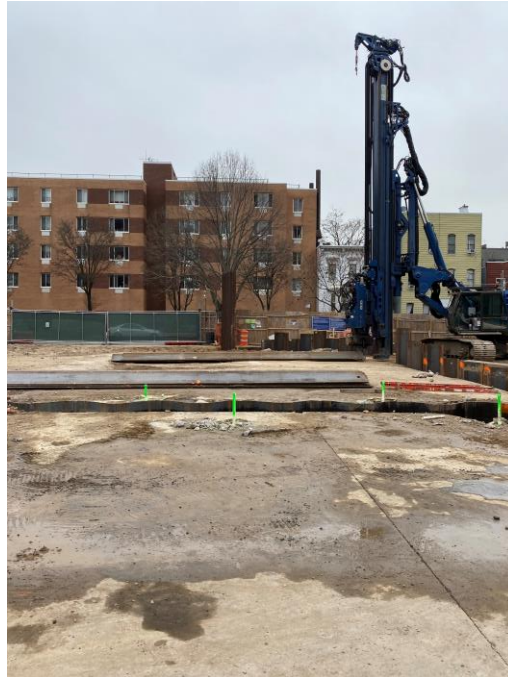
Photo 1: View of sheet pile wall installation.
