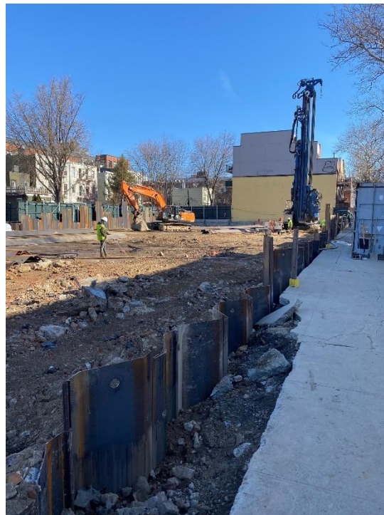
Photo 2: View of sheet pile wall facing east.
