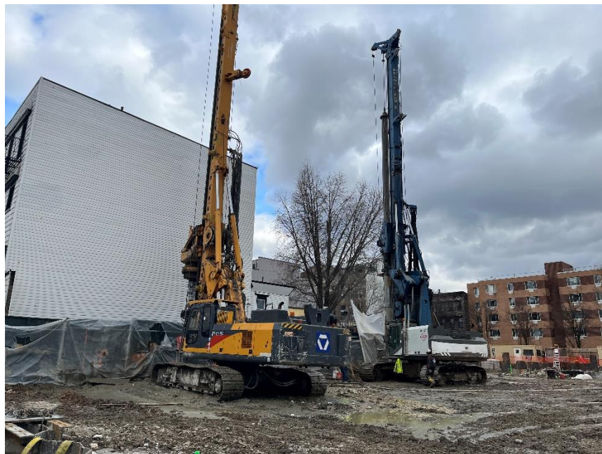
Photo 2: Alternate view of soil mix wall installation.
