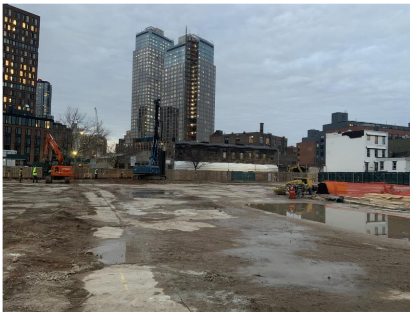
Photo 2: View of contractor installing sheet pile wall along Clay Street.
