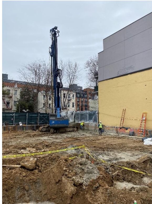
Photo 1: View of drilling for soil mix wall, facing northeast.
