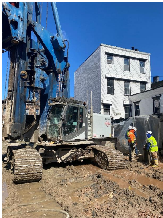
Photo 2: Alternate view of soil mix wall installation facing north.
