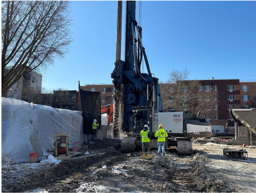
Photo 1: View of northeastern soil mix wall installation facing south.
