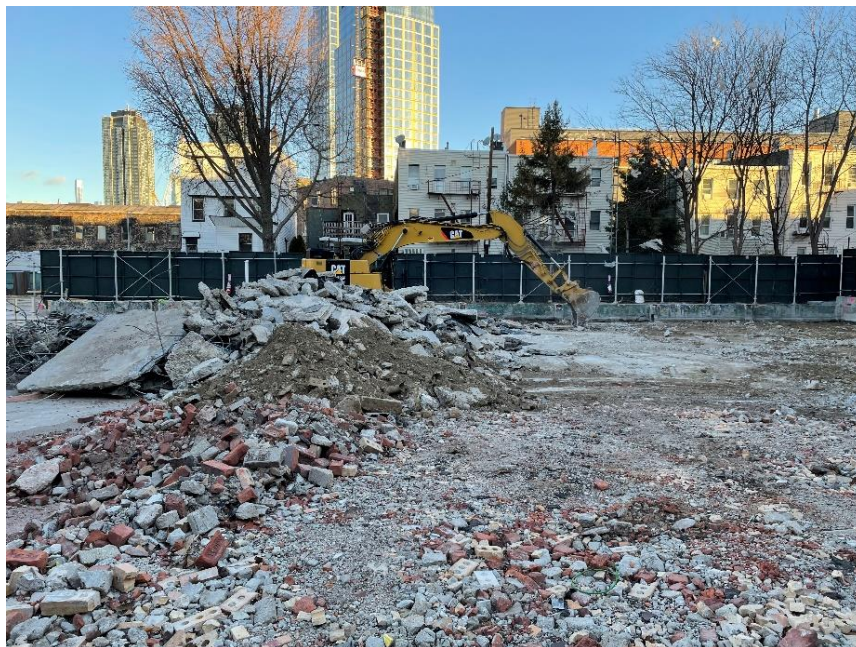
Photo 2: View of contractor preparing for installation of soil mix wall.
