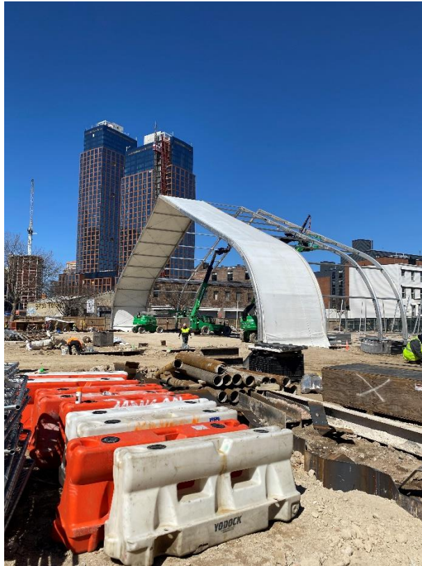
Photo 1: View of tent structural support steel installation, facing northeast.
