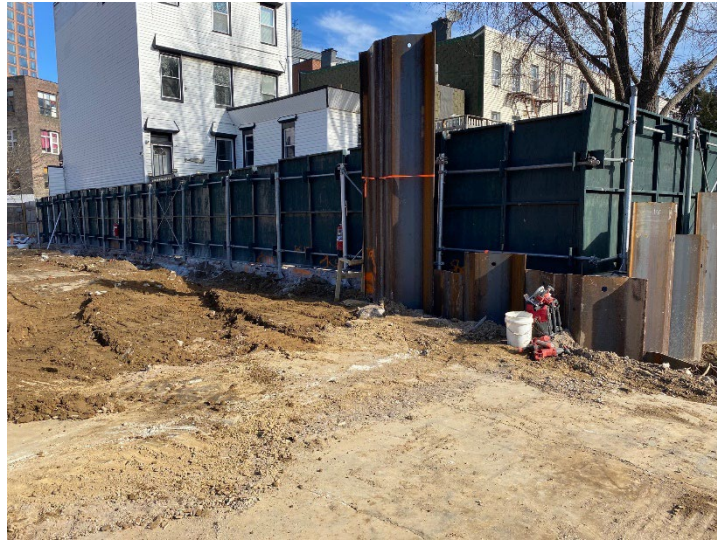
Photo 1: View of sheet pile wall installation along northeastern perimeter of site.
