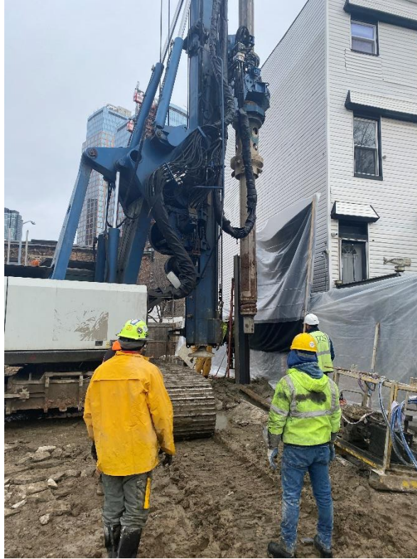
Photo 1: View of soil mix wall installation facing north.
