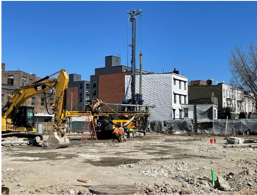
Photo 1: View of soil mix wall installation facing southeast.
