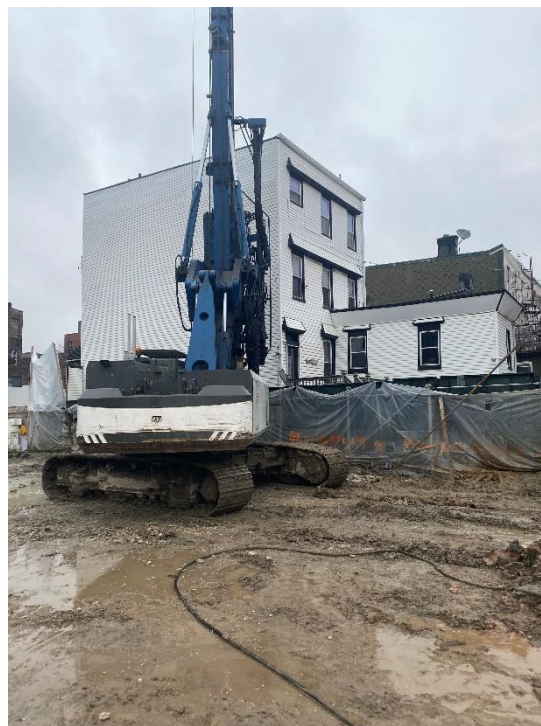
Photo 2: Alternate view of soil mix wall installation facing northeast.
