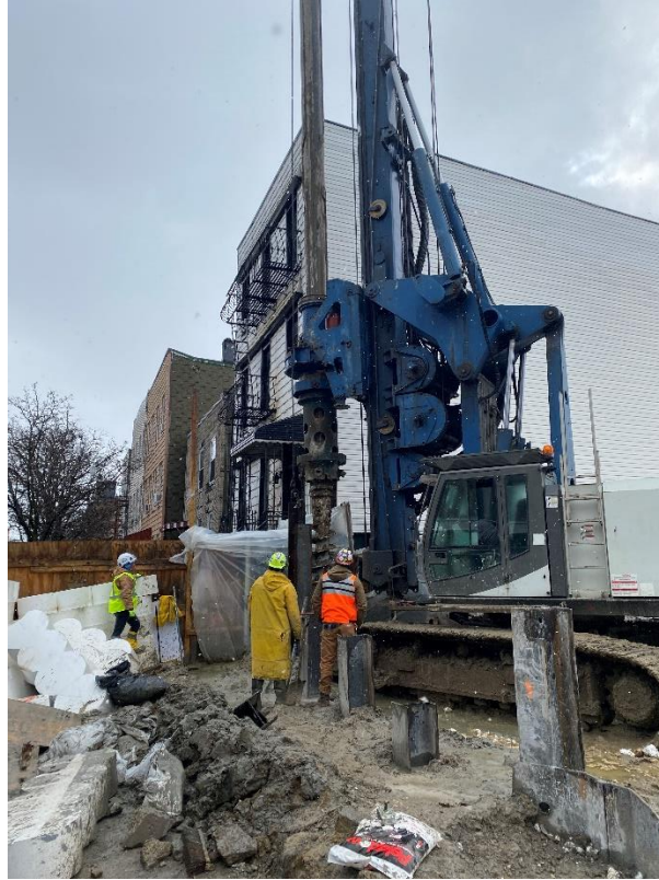
Photo 1: View of soil mix wall installation facing east.
