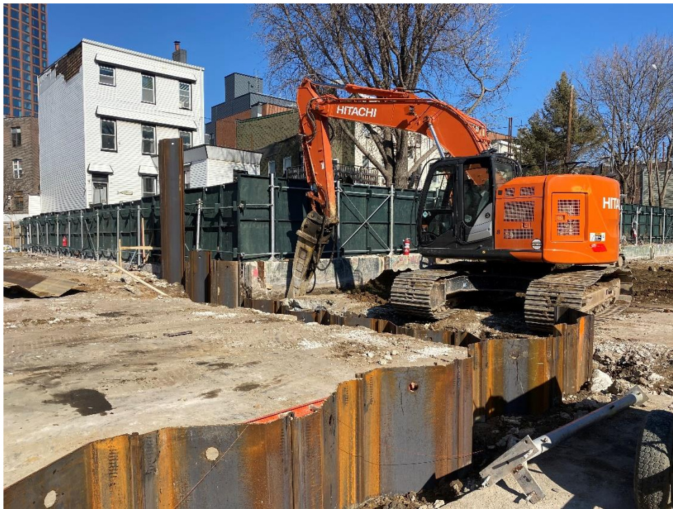
Photo 2: View of site preparation for installation of sheet piles.
