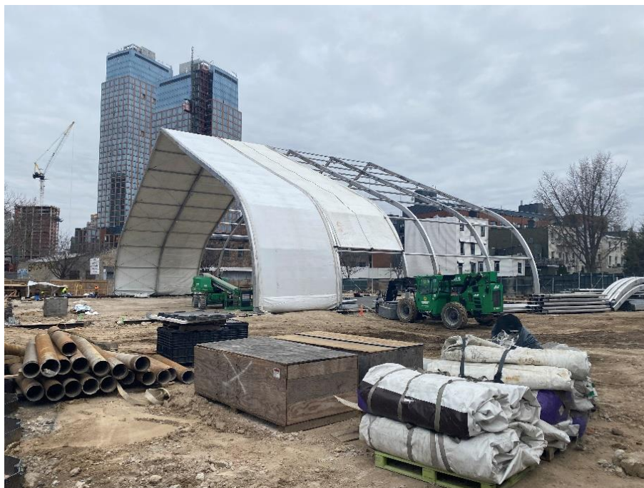
Photo 2: View of tent structural support steel installation facing northeast.
