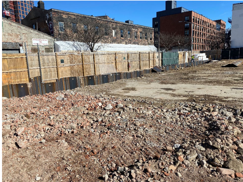
Photo 2: View of sheet pile wall installation facing northeast.
