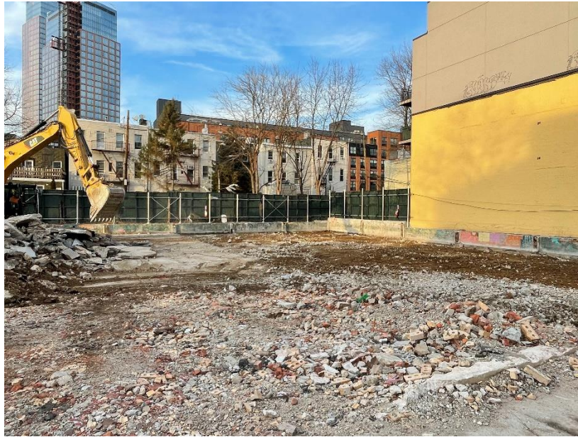
Photo 1: View of contractor preparing for installation of soil mix wall.
