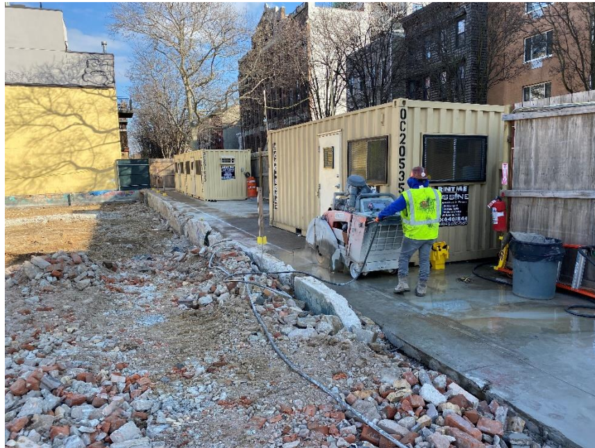
Photo 2: View of contractor saw cutting along Lot 57 Dupont Street sidewalk.
