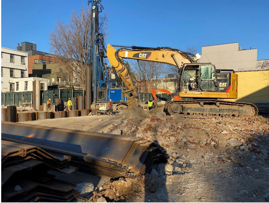
Photo 1: View of concrete slab demolition and excavation.
