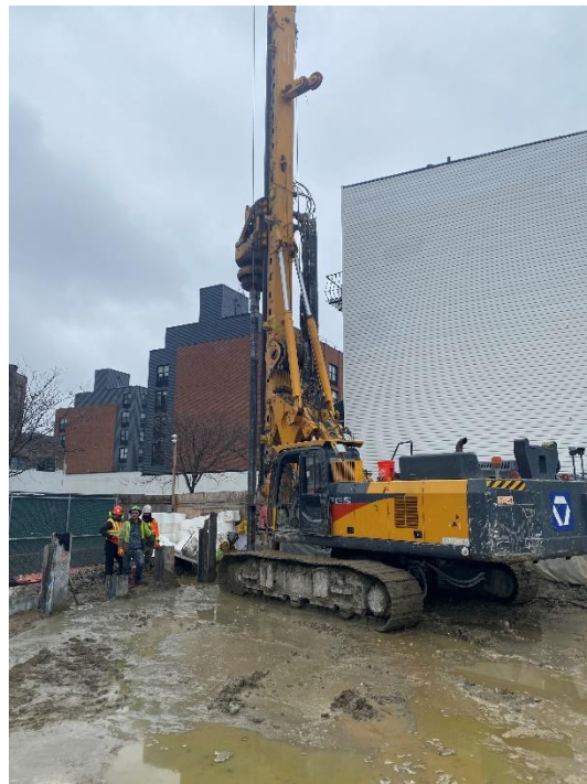
Photo 1: View of soil mix wall installation facing northeast.
