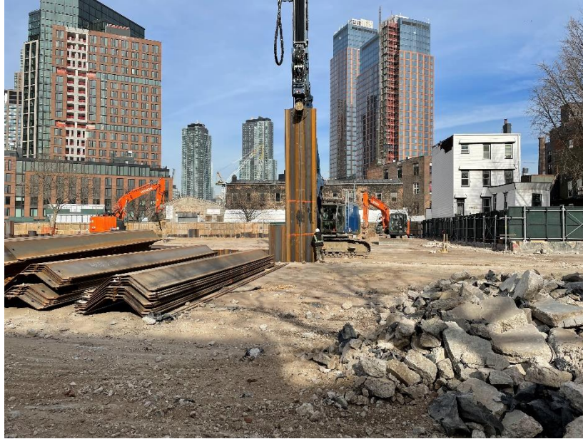
Photo 1: View of sheet pile installation along center of the Site.
