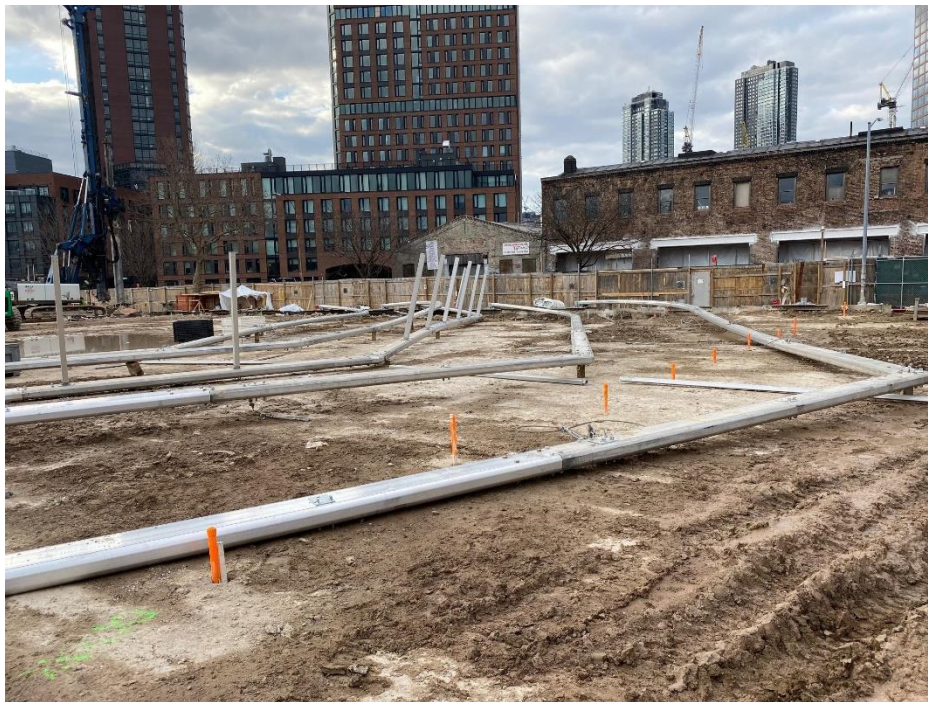
Photo 2: View of tent structural support steel installation facing north.
