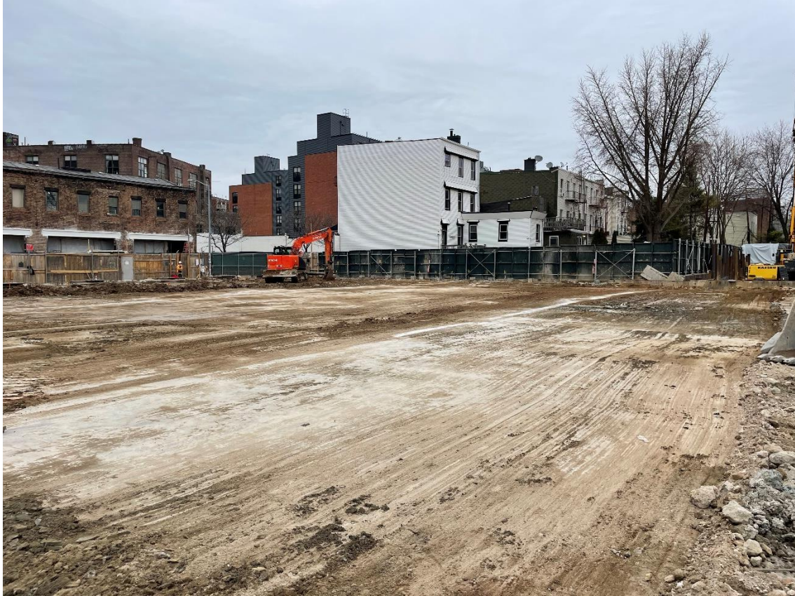
Photo 1: View of site conditions facing northeast.
