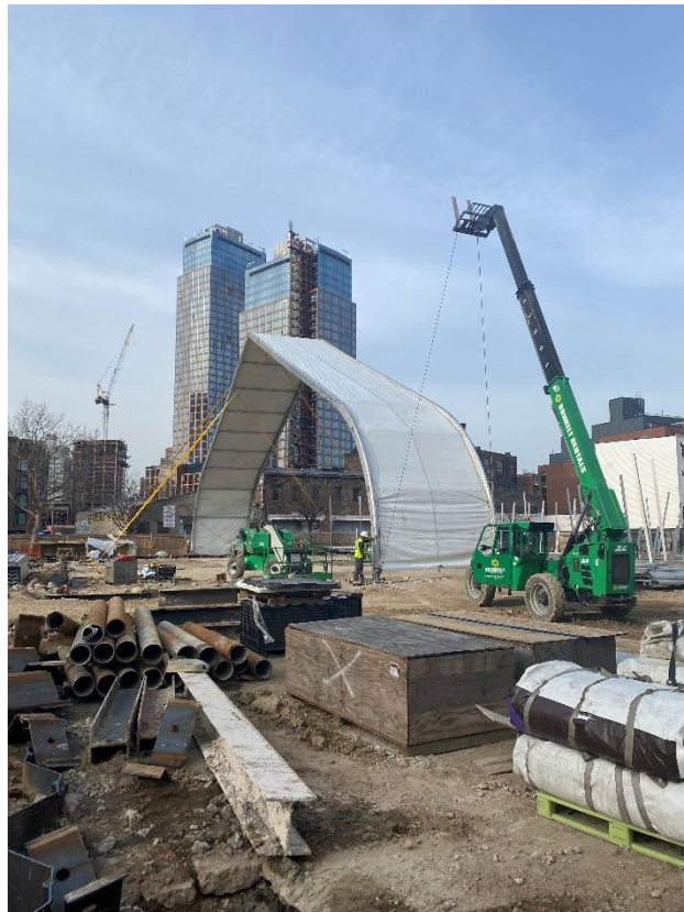
Photo 2: View of tent structural support steel installation facing north.
