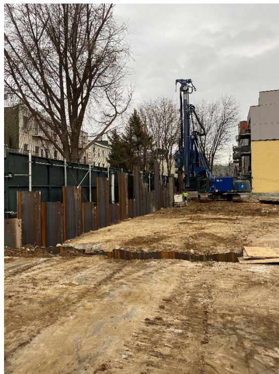
Photo 2: Alternate view of sheet pile installation in Lot 57.
