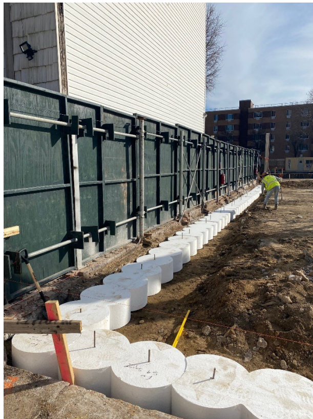
Photo 2: View of styrofoam formwork installation along northeastern perimeter of site.
