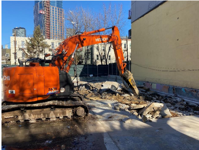
Photo 1: View of contractor preparing the area for the soil mix wall.
