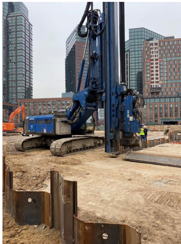
Photo 2: Alternate view of sheet pile wall installation.
