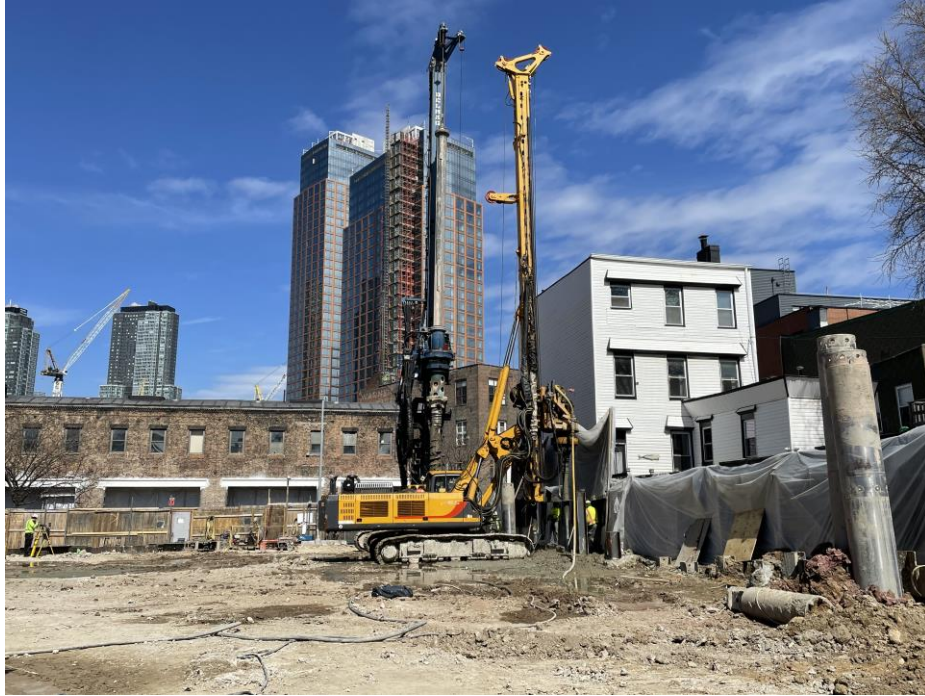
Photo 1: View of soil mix wall installation facing north.
