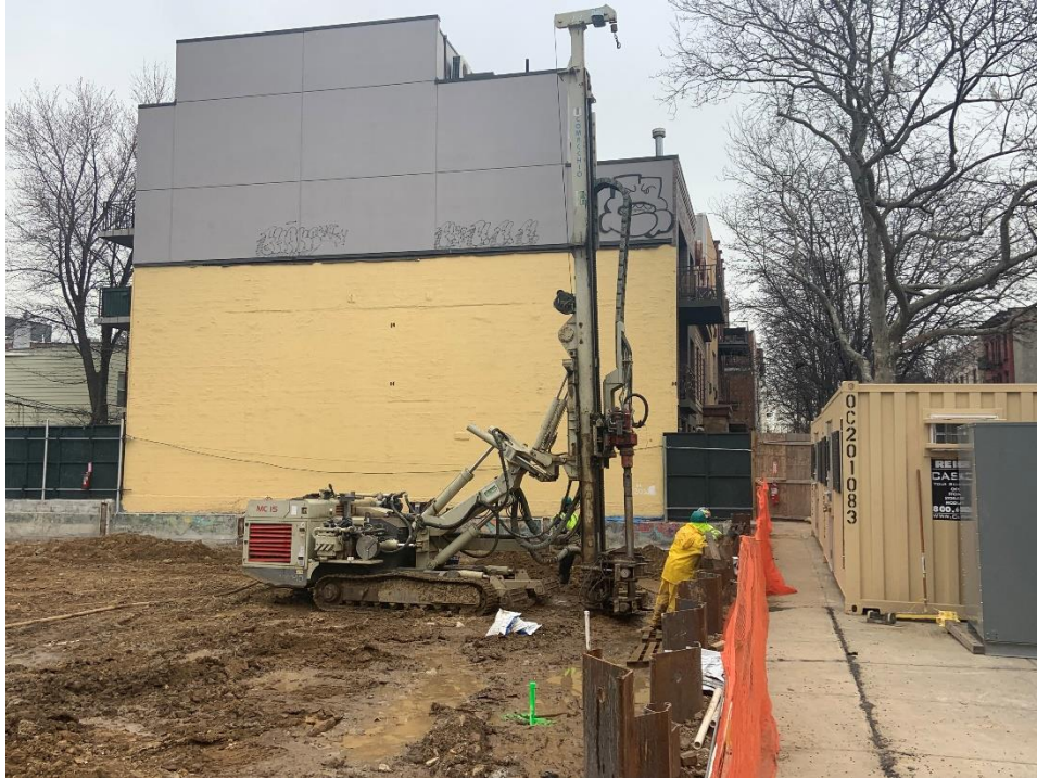
Photo 1: View of contractor installing dewatering points, facing East.
