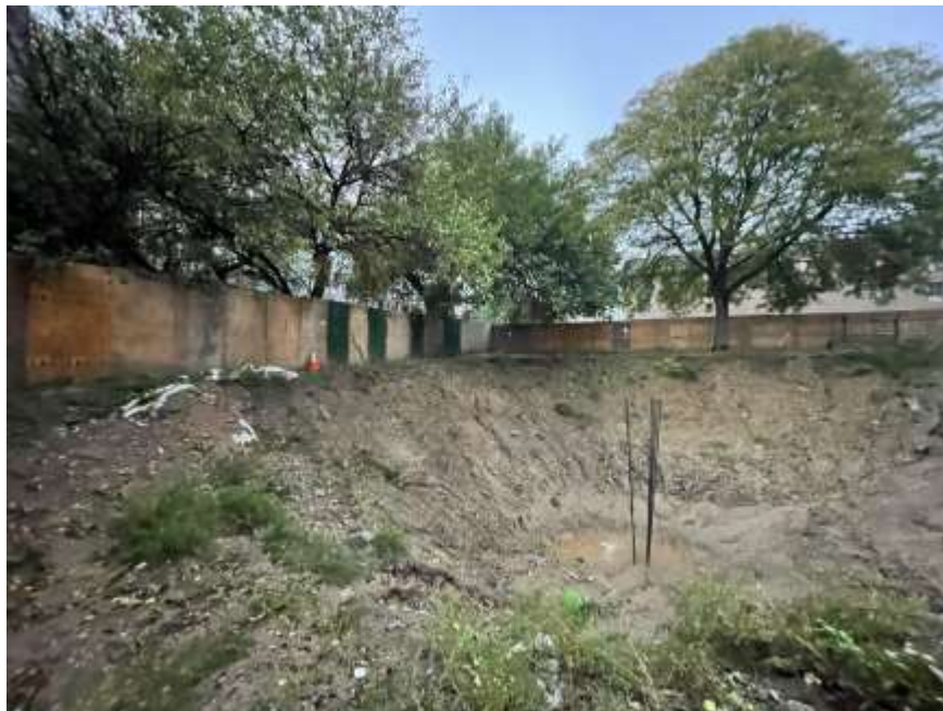
Photo 2: General view of the site (facing northwest).
