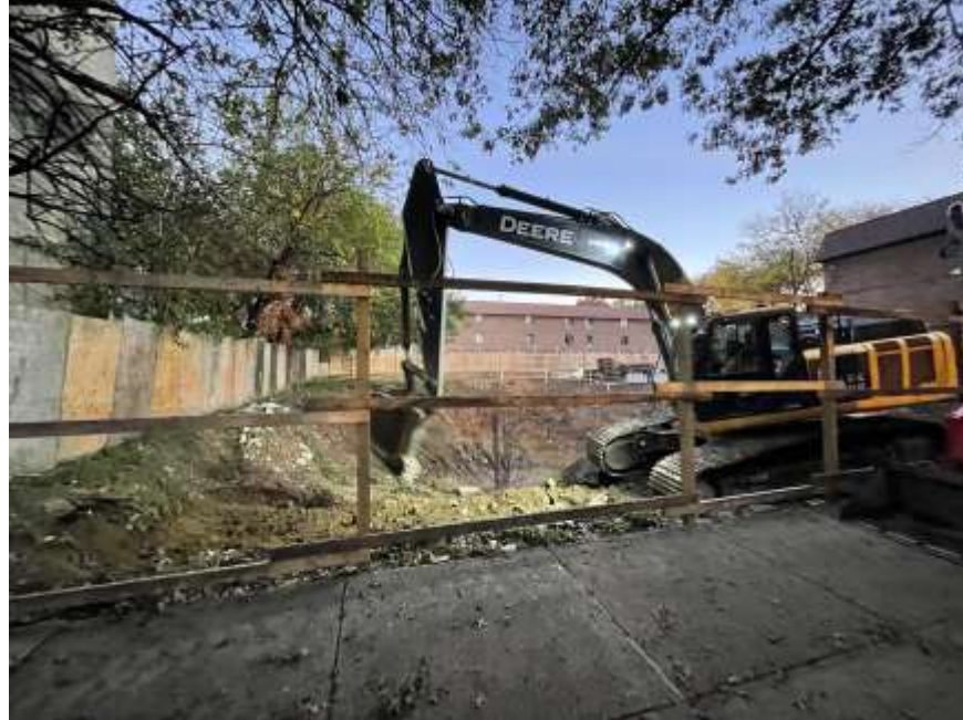
Photo 1: View of Rise grading non-hazardous historic fill in the southwestern part of the site (facing north).
