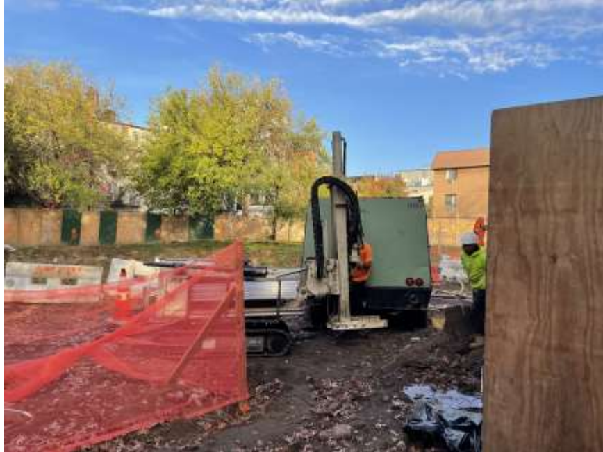
Photo 1: View of Lakewood advancing a soil boring in the southeastern part of the site (facing southwest).
