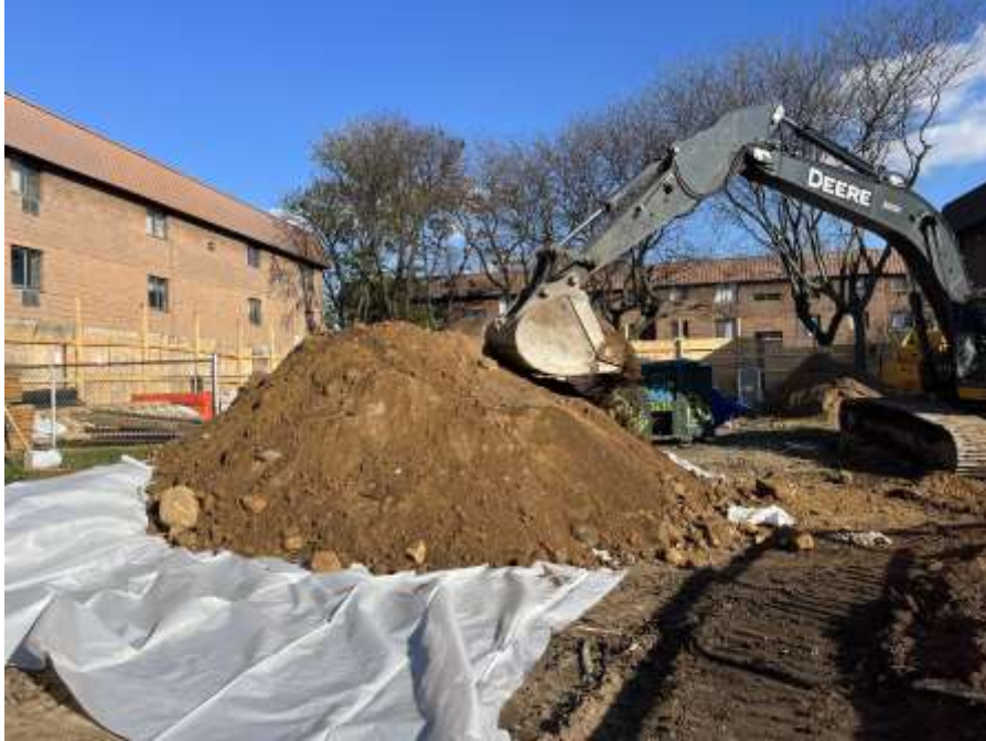
Photo 1: View of Rise stockpiling non-hazardous fill in the northeastern part of the site (facing east).
