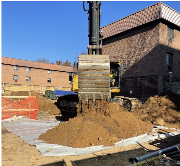
Photo 2: View of Rise stockpiling non-hazardous fill on polyethylene sheeting in the southeastern part of the site (facing northeast).
