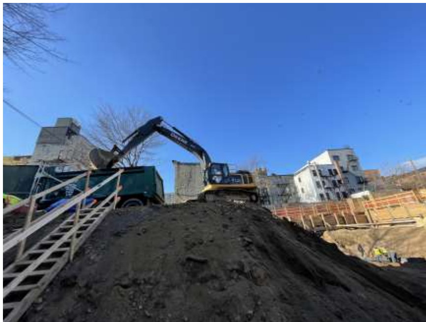
Photo 2: View of Rise live-loading non-hazardous fill/soil into permitted tri-axle trucks for off-site disposal (facing west).
