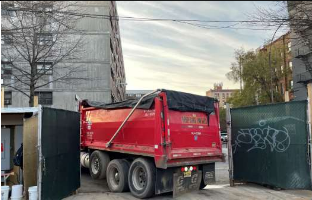
Photo 3: View of typical secured tarp for trucks transporting non-hazardous fill to disposal facility (facing east).
