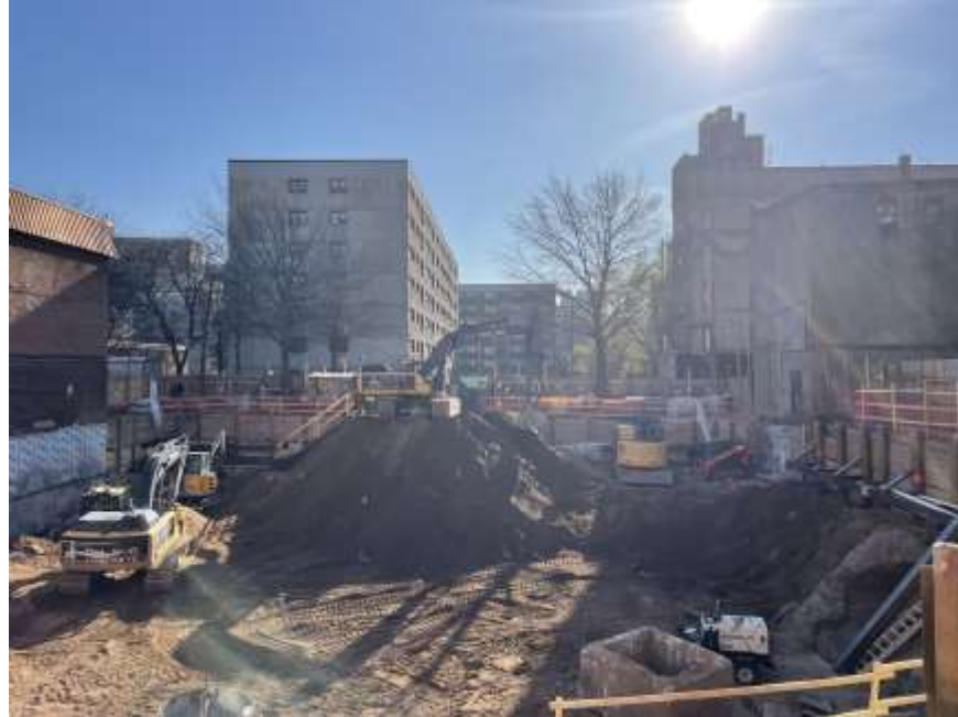
Photo 1: View of Rise live-loading non-hazardous fill into permitted tri-axle trucks for off-site disposal (facing south).
