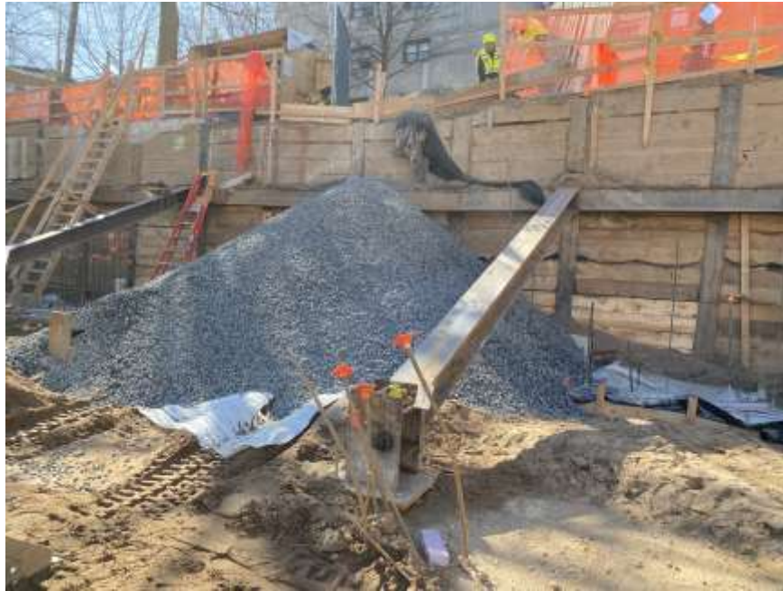
Photo 1: View of \frac{3}{4} -inch virgin stone stockpiled in the southern part of site (facing southeast).
