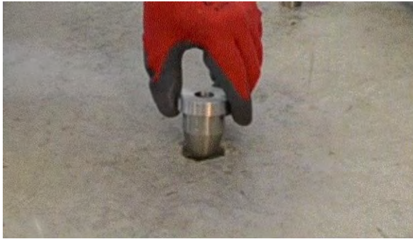
Figure 3. Testing Depth with the Drilling Guide
