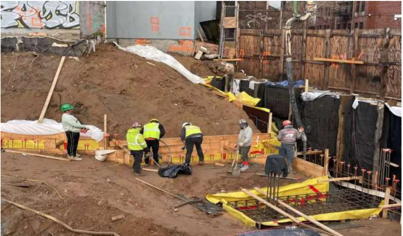
Photo 3: Concrete was distributed by pump truck and consolidated by vibrators
