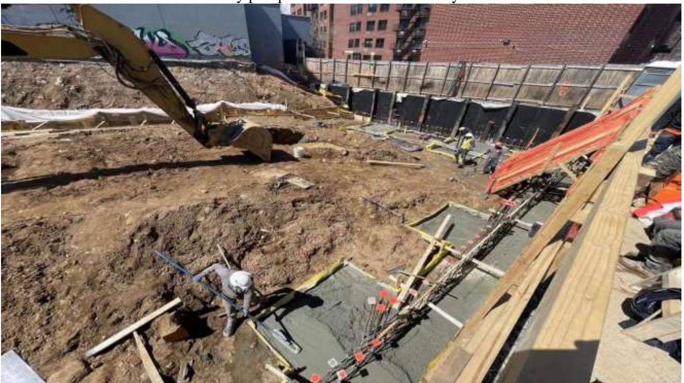
Photo 4: Strike-off by trowels and concreting was finished
