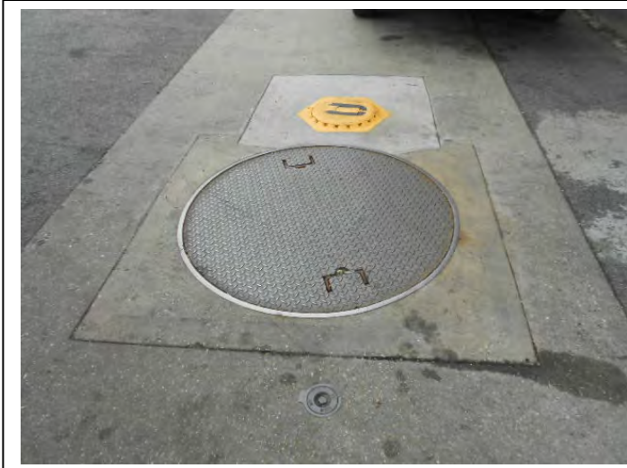
UNDERGROUND STORAGE TANK
