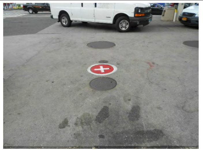
UNDERGROUND STORAGE TANK
