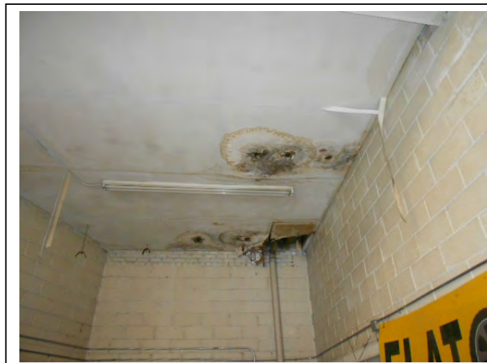
SUSPECT MOLD
