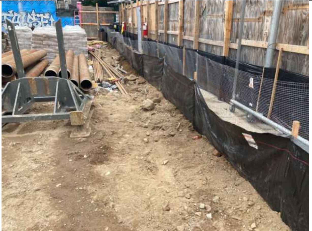
Photo 4 – Silt fence along Bayard Street.
