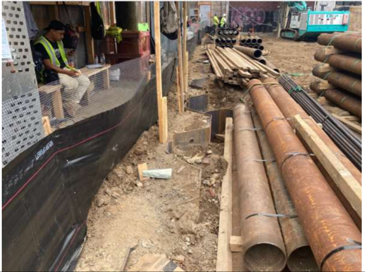
Photo 3 – Silt fence install along Graham Ave.
