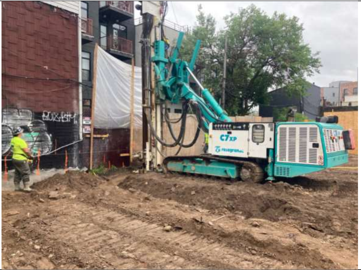
Photo 1 – Piling drilling in grid B3.
