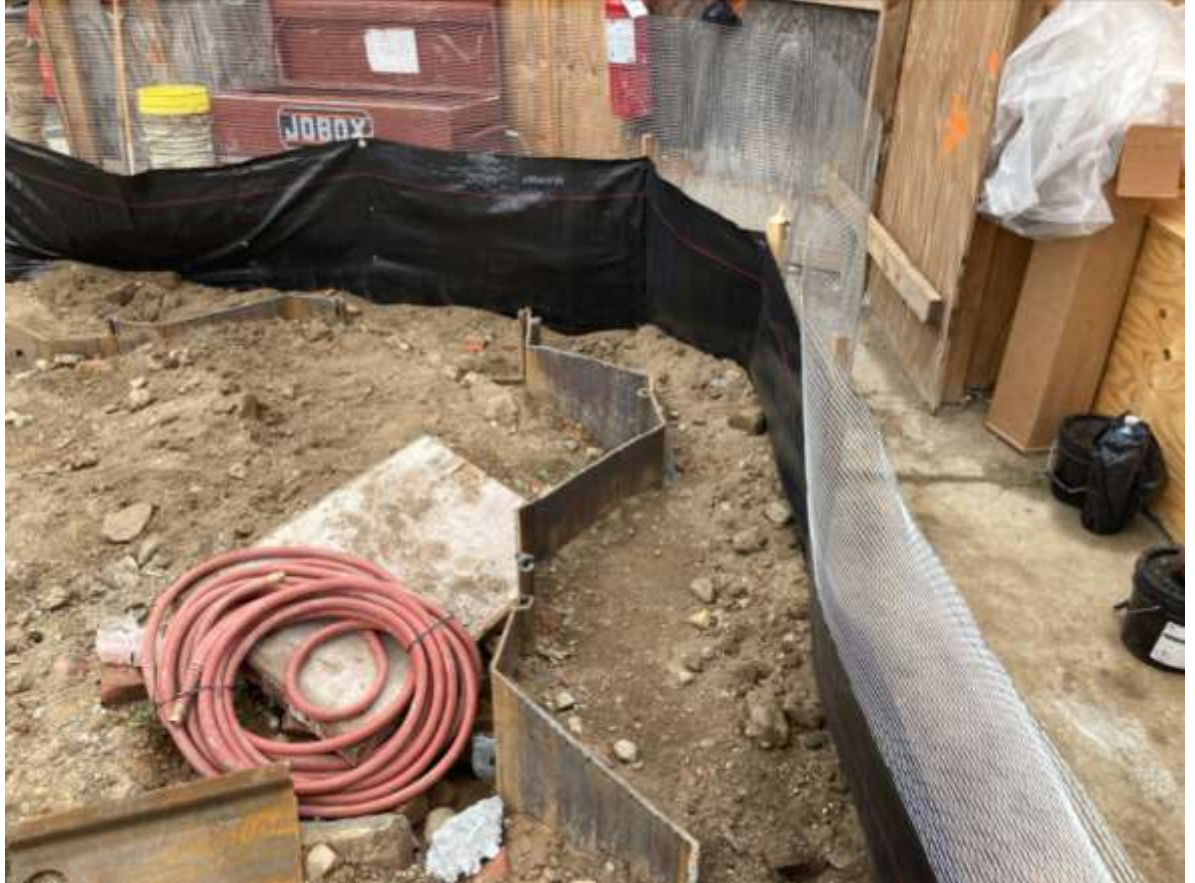
Photo 2 – View of silt fence installed at Bayard/Graham corner.
