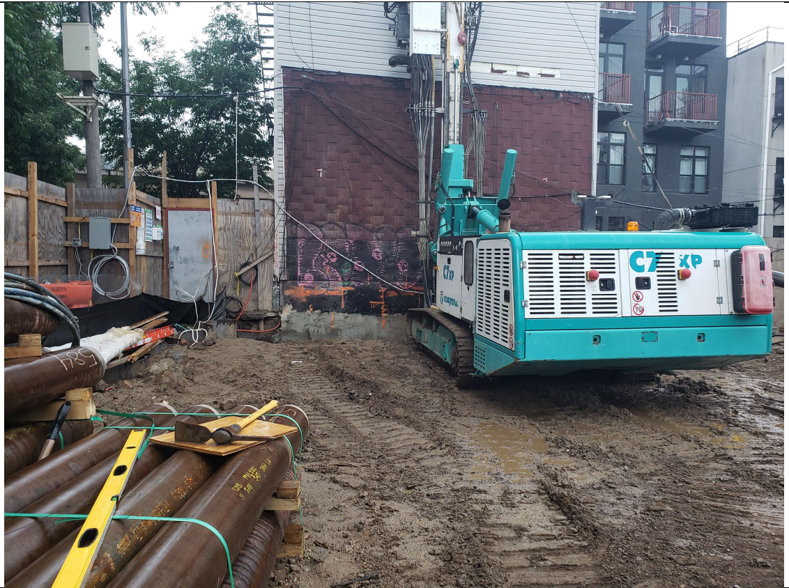
Photo 1 – View of pile driving along in Grid B3 along lot 24
