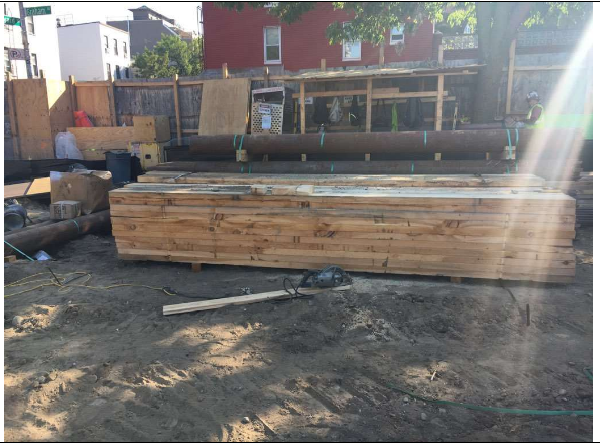
Photo 3 – View of silt fence along corner of Graham and Bayard.
