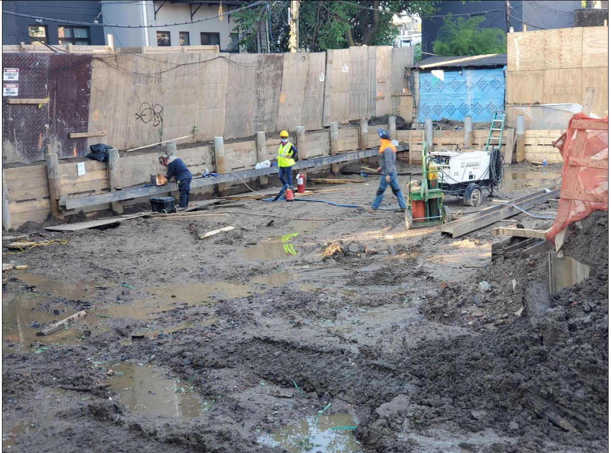
Photo 2 – Welding waler to piles for SOE at south side of Grid A3 and B3 along neighboring properties on Graham Ave. View is facing southwest from Graham Ave.
