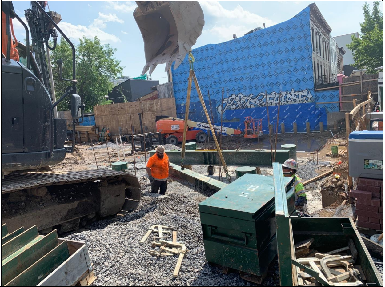
Photo 3 – View of concrete load beams being offloaded on site and being put together for the load test to occur.
