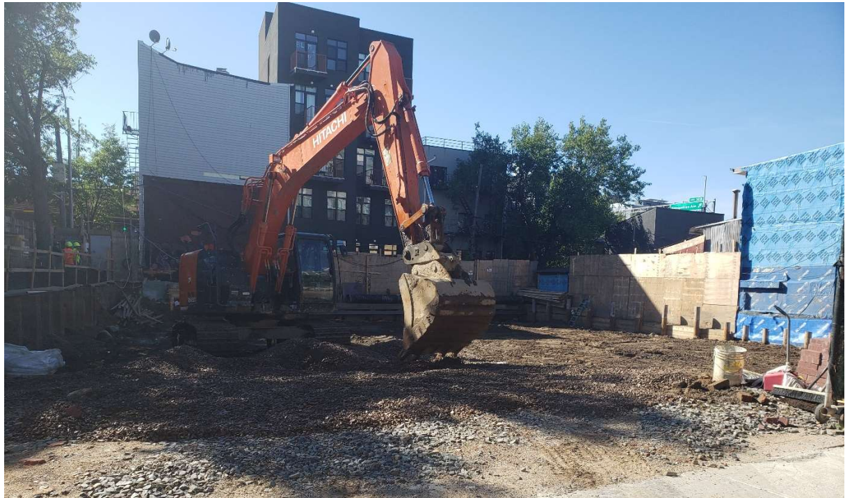
Photo 3 – View of gravel being spread for stabilized construction entrance in grid B1
