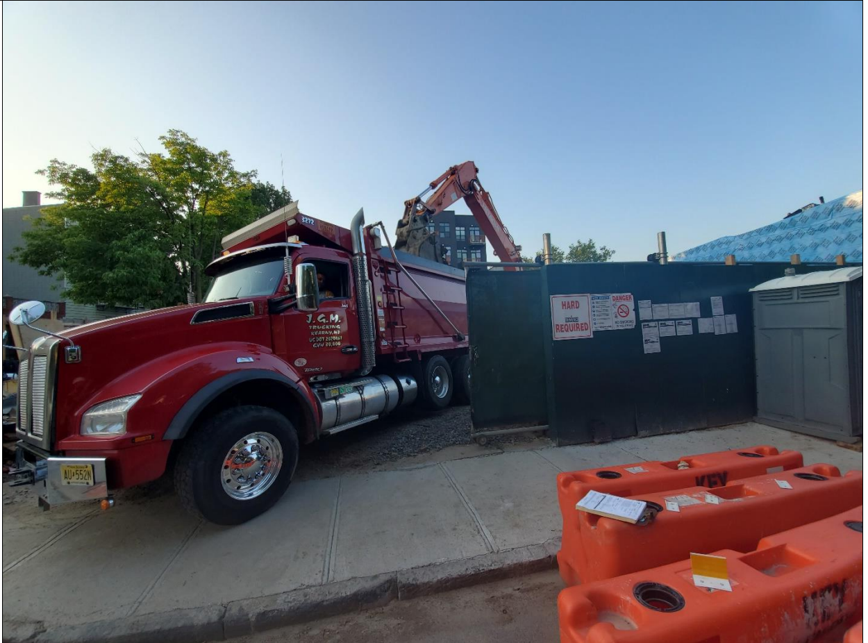
Photo 2 – Truck being loaded with soil (0-5') to be sent to Former New Jersey Zinc-West Plant, Palmerton PA. View is facing south towards site entrance on Bayard St.
