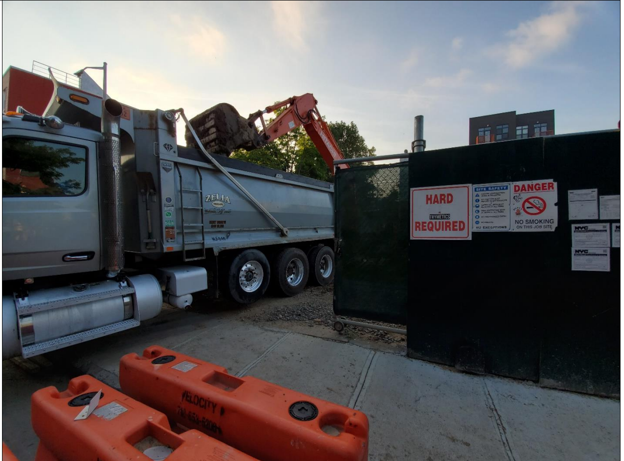
Photo 2 – Truck being loaded with soil (0-5') to be sent to Former New Jersey Zinc-West Plant, Palmerton PA. View is facing southeast towards site entrance on Bayard St.
