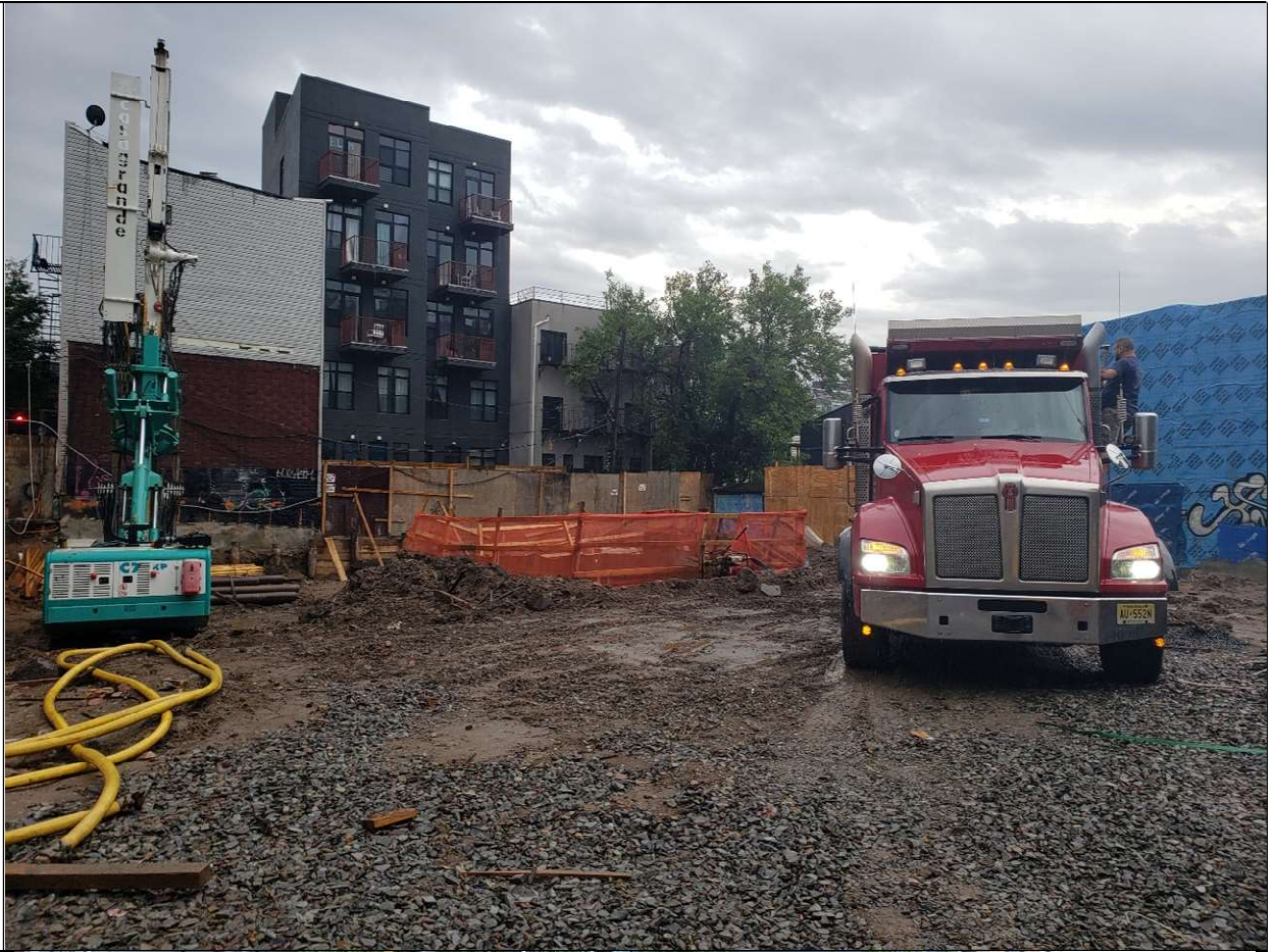
Photo 1 – Trucking 0-6’ from grids A2/A3, west and southwest of elevator pit in center of site.
