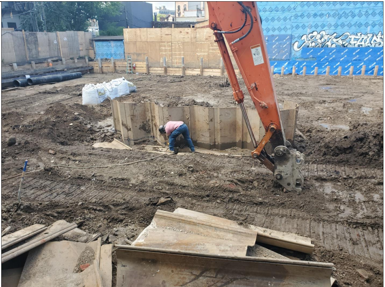
Photo 3 – Sheet piles at center of site being cut to 5'bsg, view is facing southwest from Graham Ave side of site.
