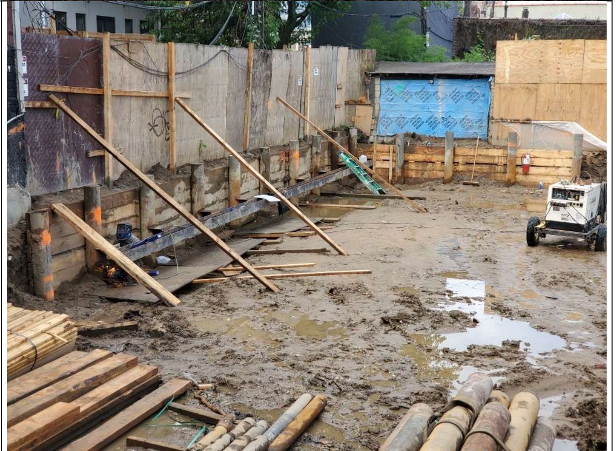
Photo 2 – View of whalers installed in A3 along South property boundary
