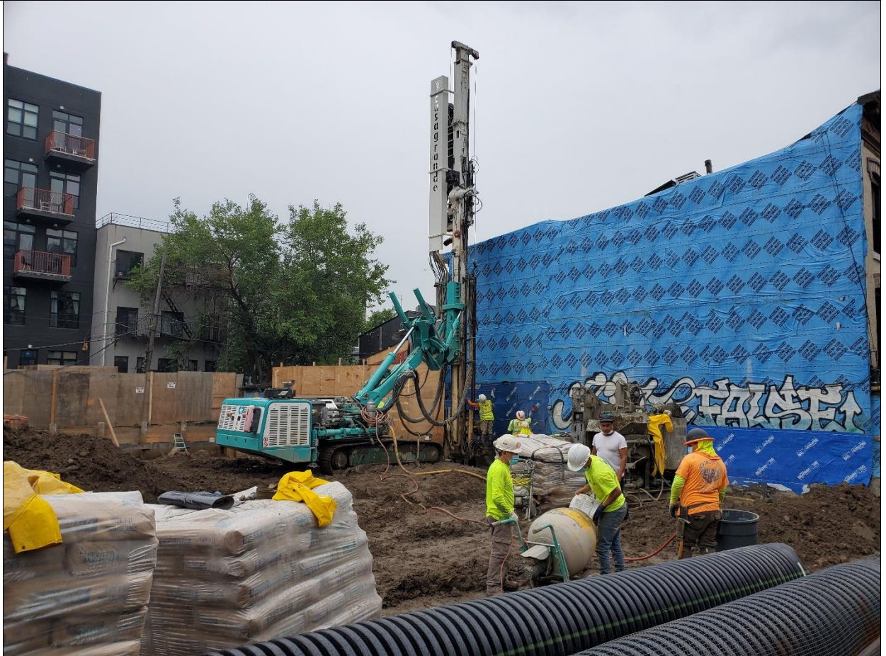
Photo 2 – Piles being driven with water and grouted at west side of Grid A1/A2 along neighboring property on Bayard St, view is facing southwest from Bayard St.
