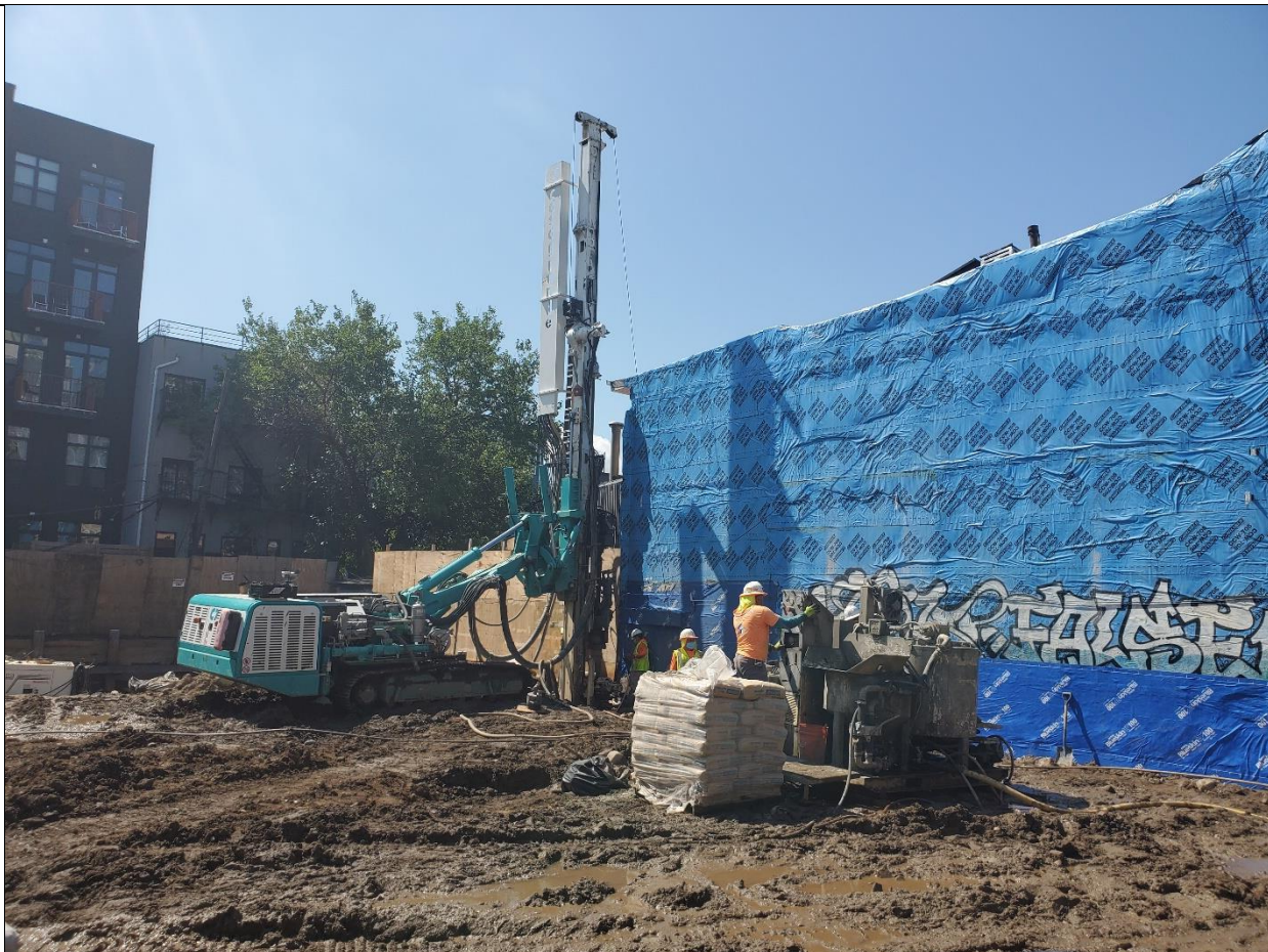
Photo 3 – Piles being grouted at west side of site along neighboring properties on Bayard St. View is facing southeast from Bayard St.
