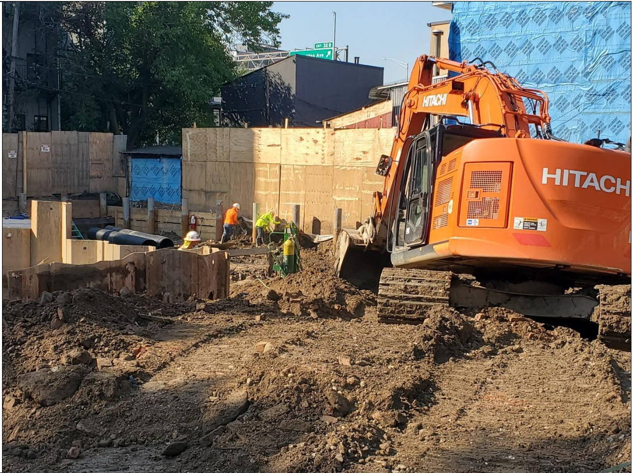
Photo 3 – Sheet piles at center of site being cut to 5' bsg and lagging being installed to 5' bsg at southwest side of site in Grid A3 along neighboring property on Bayard St. View is facing southwest from site entrance on Bayard St.
