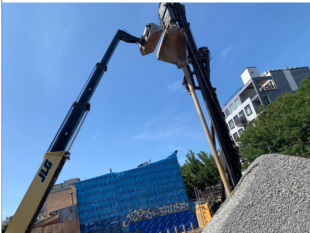
Photo 3 – View of piledriver being filled with gravel for soil improvement grouting.
