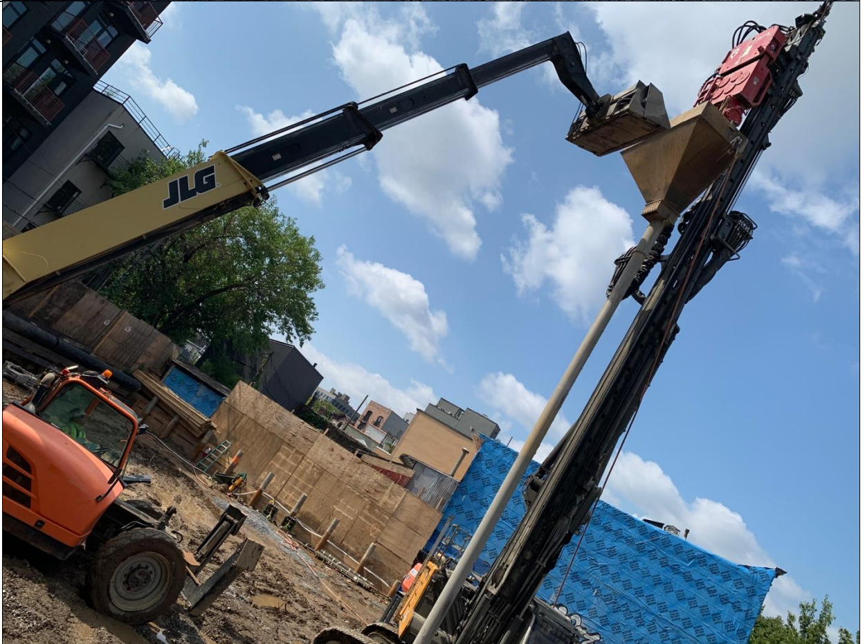
Photo 2 – View of hopper attached to piledriver to be used for soil improvement grouting. View is N towards grid B2.
