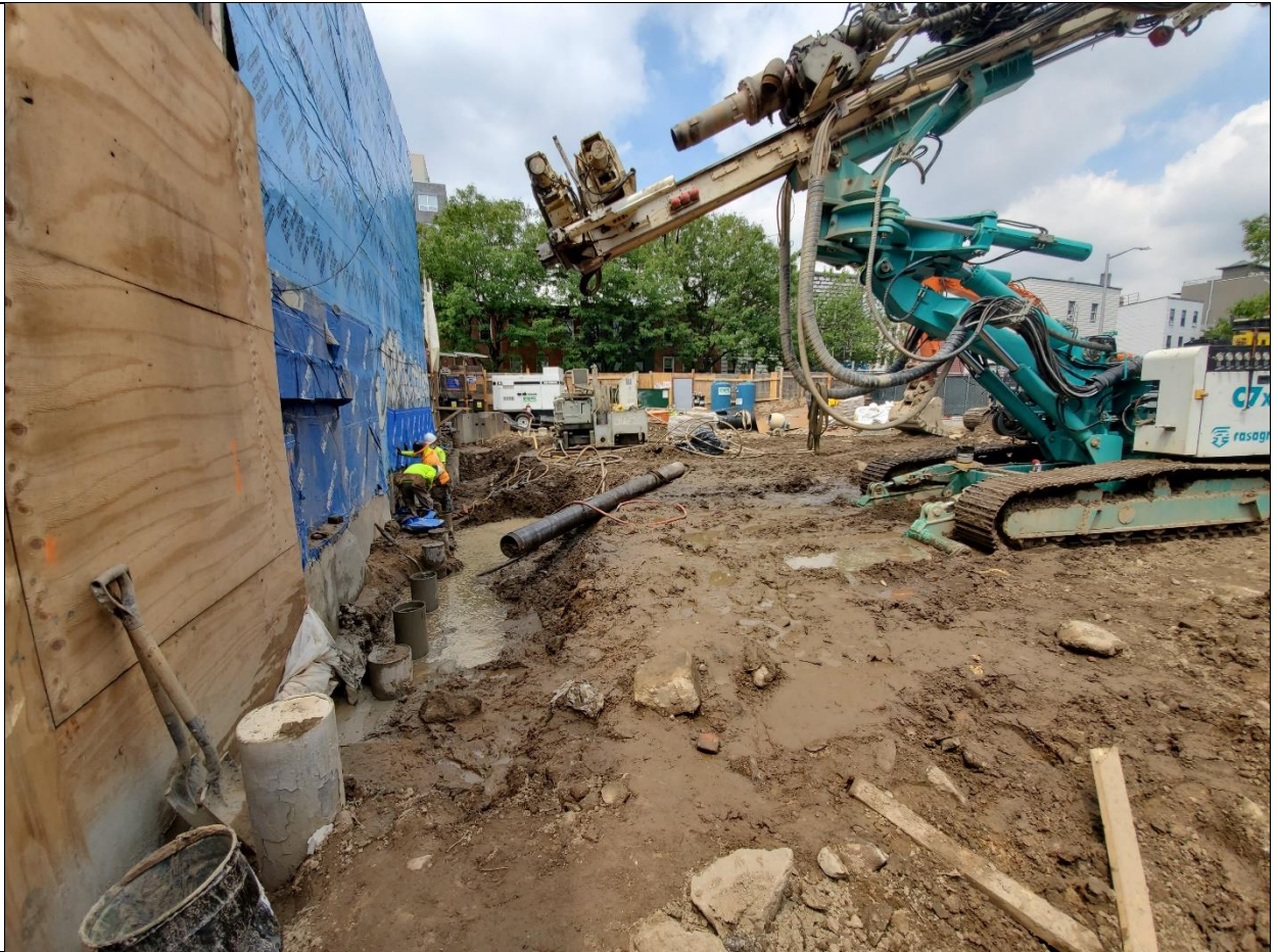
Photo 3 – Close up of piles driven with water and grouted at west side of Grid A1/A2 along neighboring property on Bayard St.
