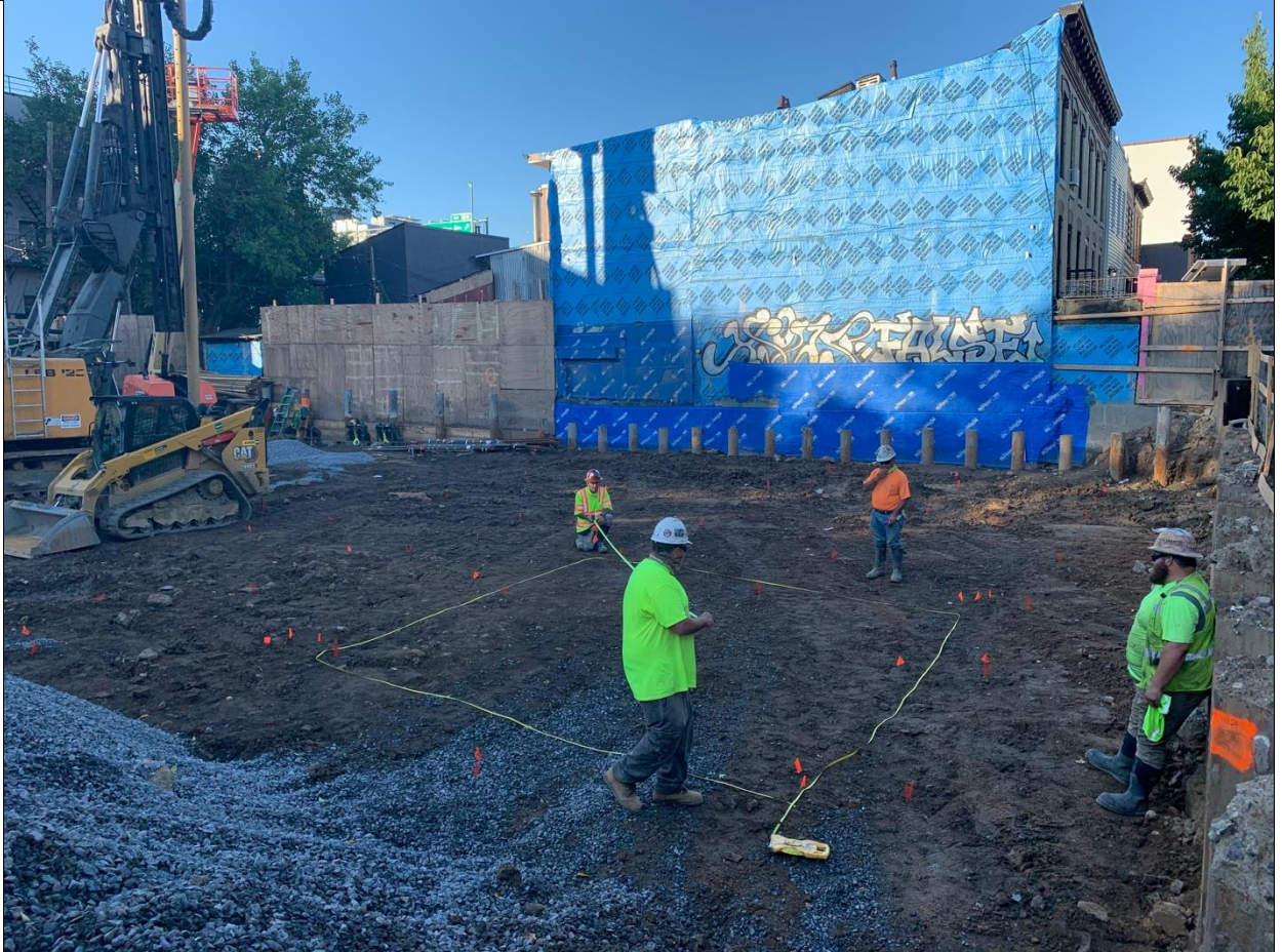
Photo 2 – Mapping out where exactly drilling will occur on site. This is within boundary A1.
