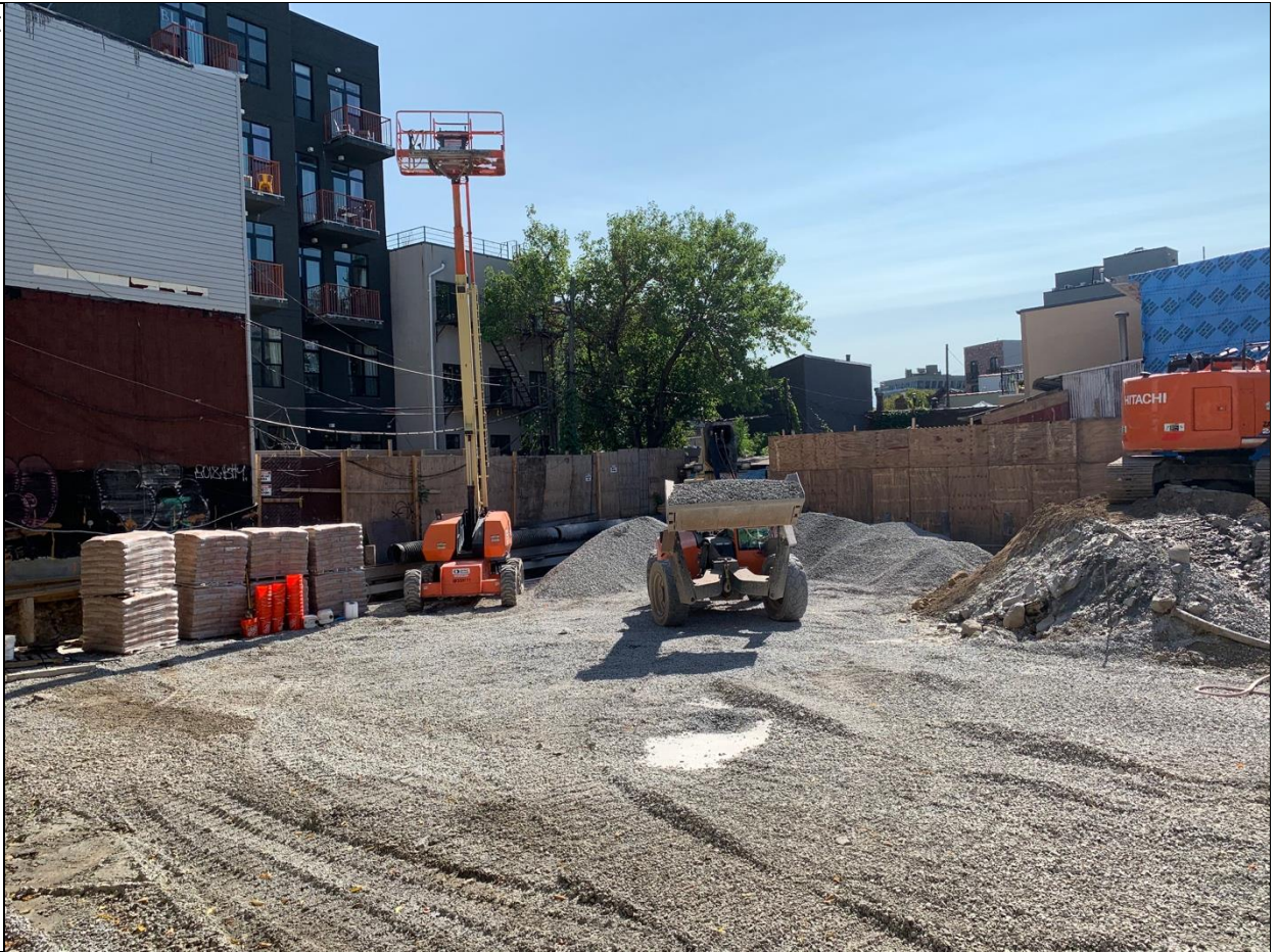
Photo 5- A look at the site towards the end of the day, where gravel is being brought to the pile driving machine for soil grouting improvement.
