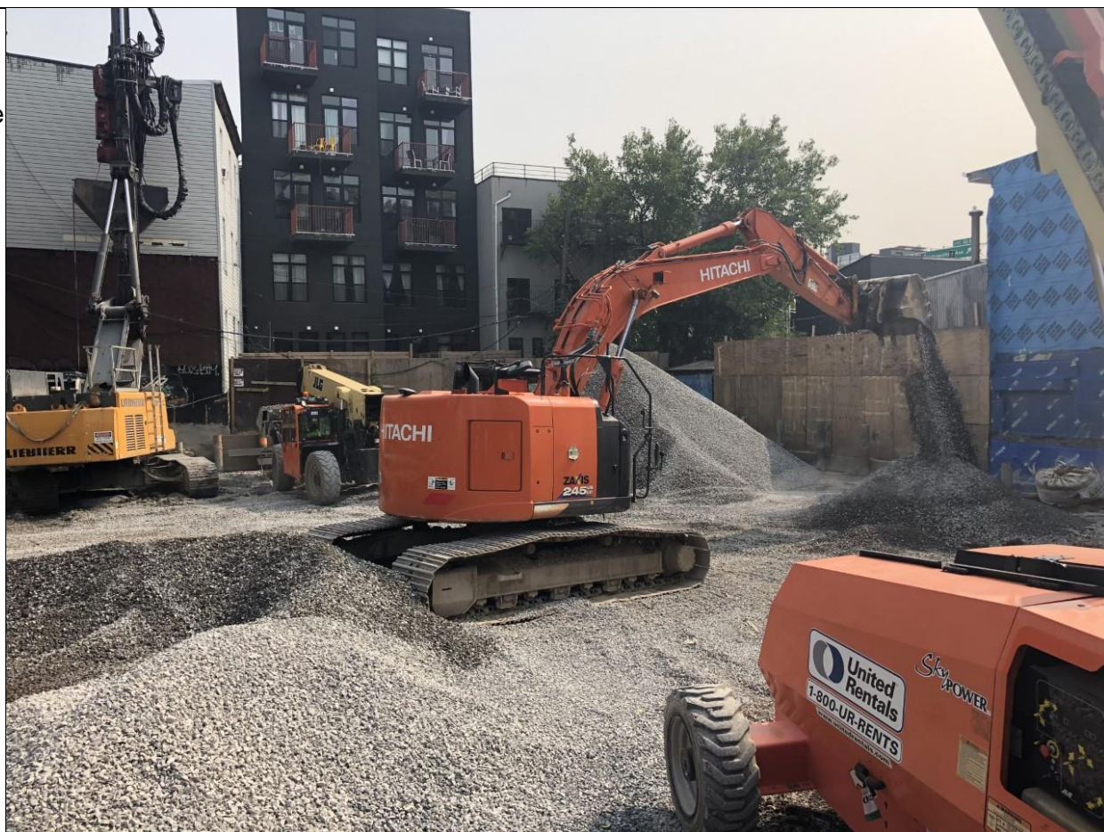
Photo 7 – View of Moncon relocating gravel from site entrance ramp to Grid A2 for continued stabilization piling.
