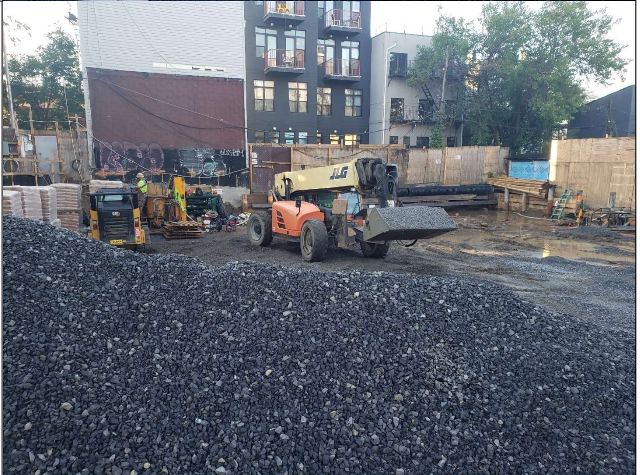
Photo 2 – Telescopic Handler en route to pile driver with bucket of \frac{3}{4} " stone
