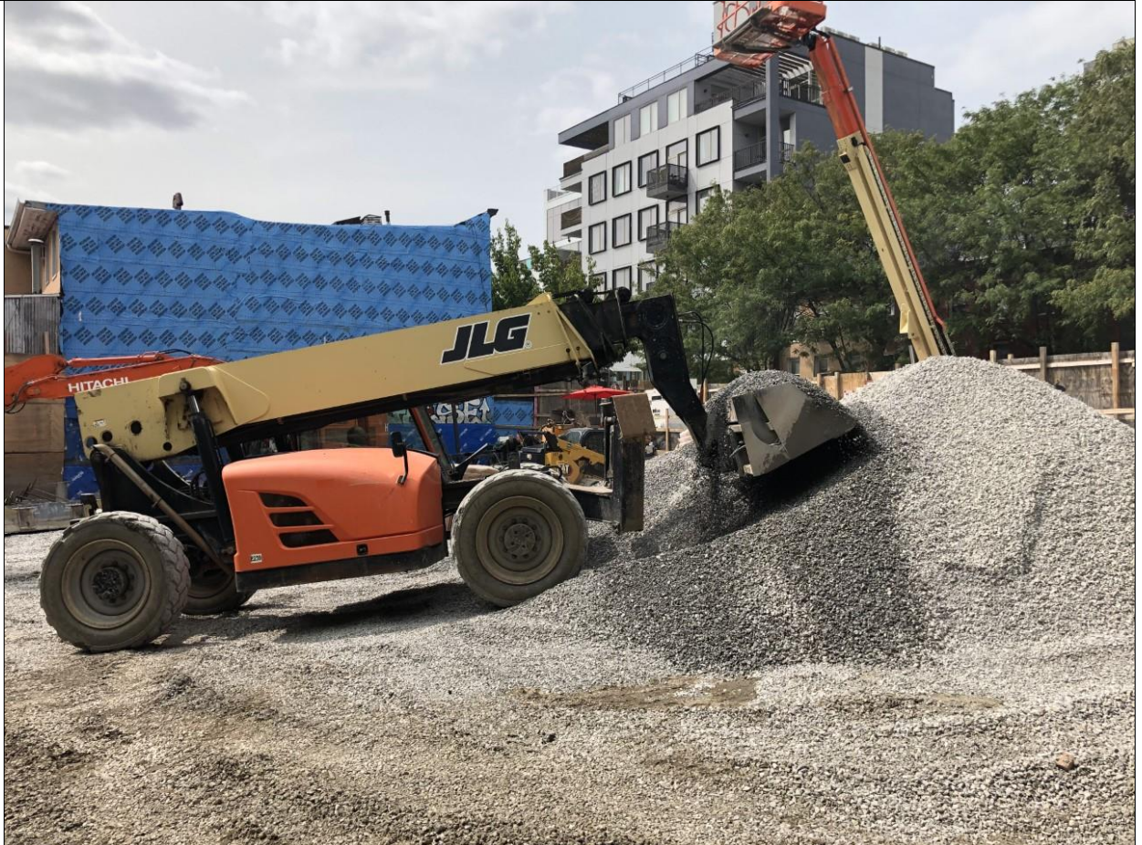
Photo 2 – Moncon spreading and stockpiling gravel with a JLG Telehandler for construction mixing. Grid B1 corner of site.
