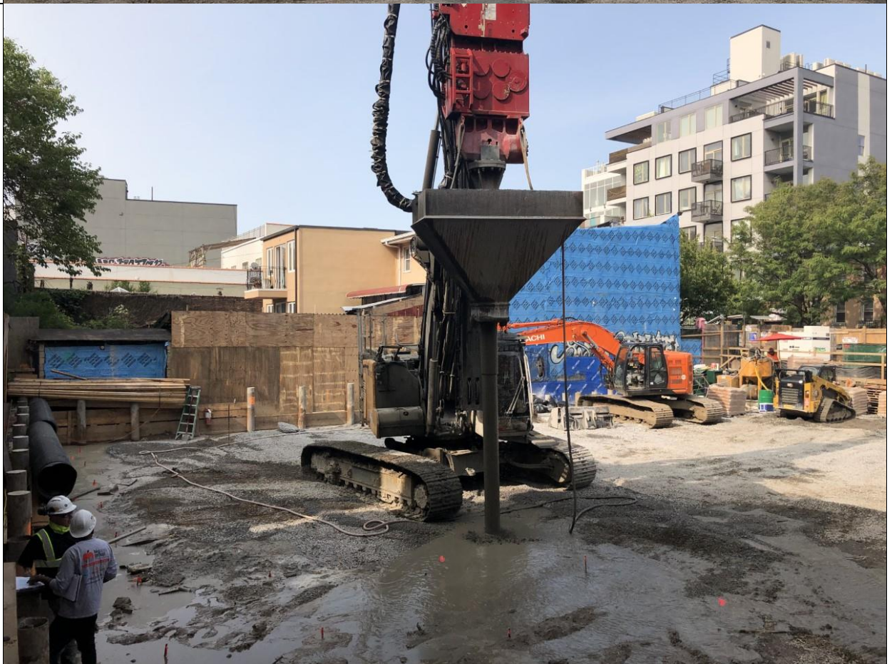
Photo 4 – Alternate view of stabilization piles being made with gravel and grout. View is facing northwest towards Bayard Street.
