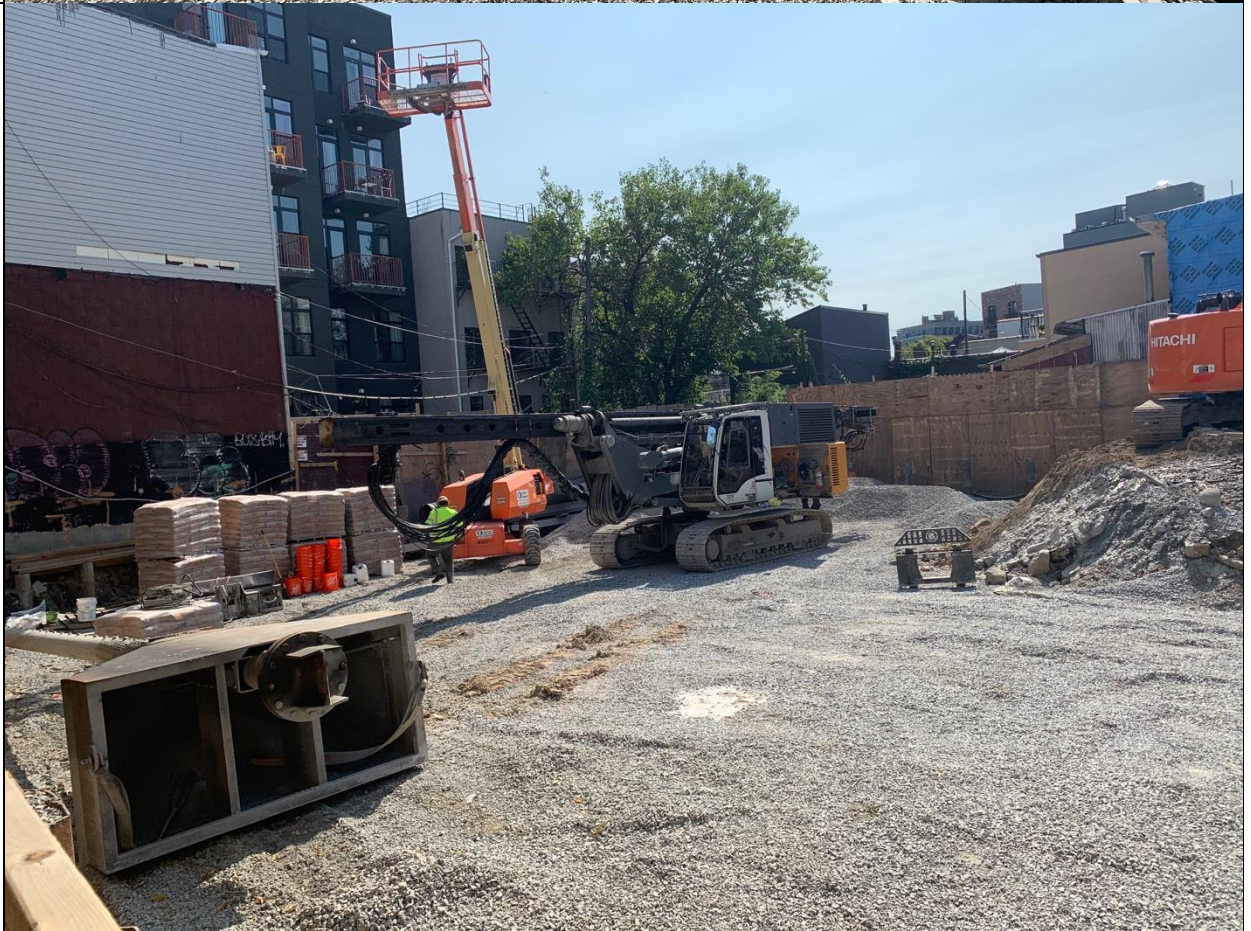
Photo 6- A photo towards the end of the day, which faces towards grid A3/B3. The drill piler is being dismantled.
