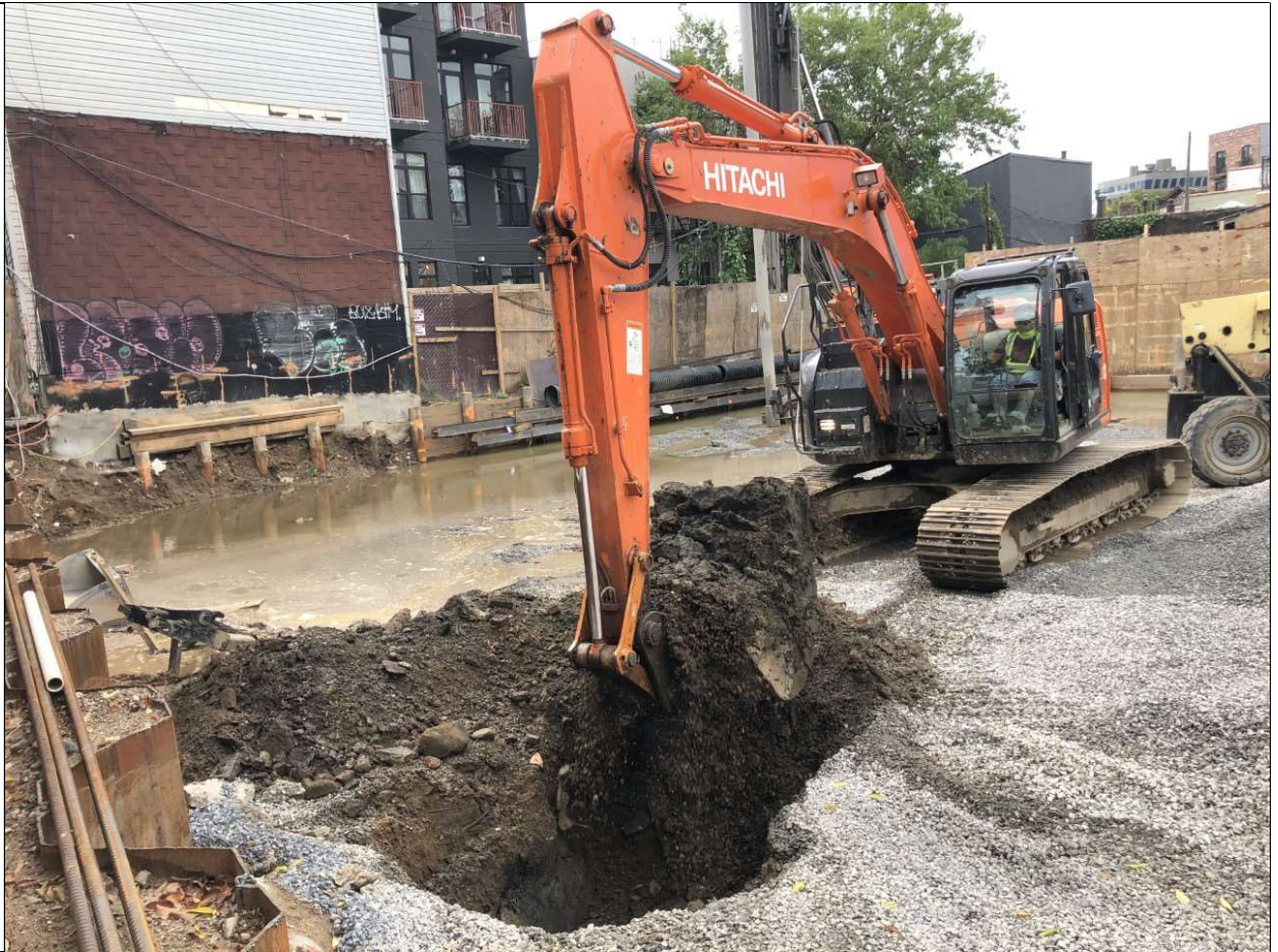
Photo 5 – Excavation of a 5-foot-deep pit on Grid B2 to drain excess water from Grids A3 and B3.
