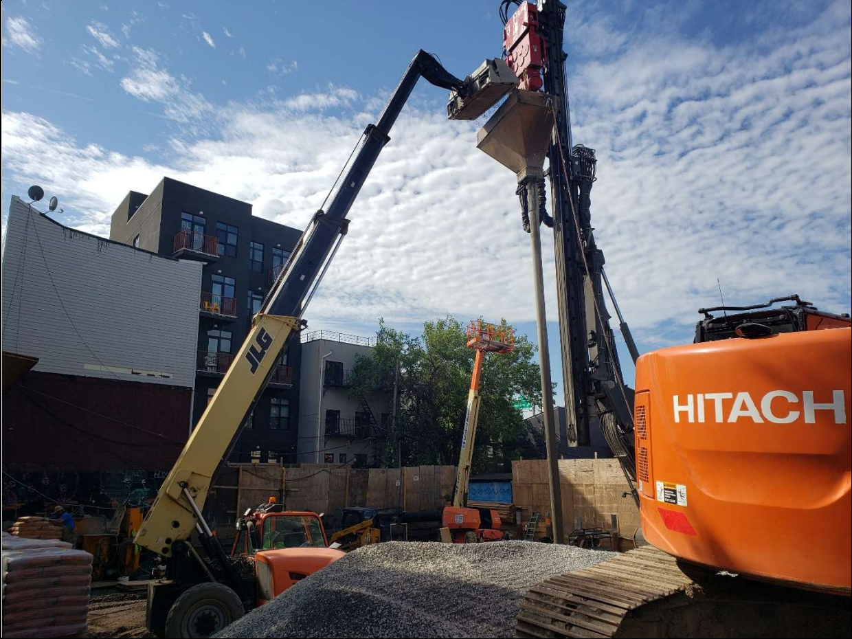
Photo 2 – Loading gravel into hopper for grout mixture for soil improvement micropiles
