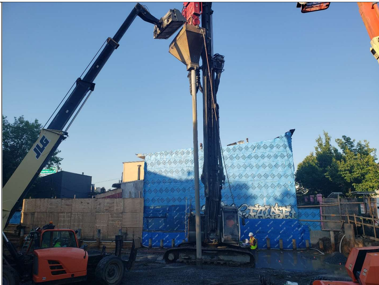
Photo 3 – Telescopic Handler loading \frac{3}{4} " gravel into hopper for grout mixture for micropiles
