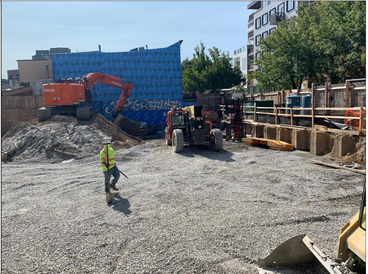
Photo 5- A look at the site towards the end of the day, where there is preparation occurring to create a ramp for the drill piler to be removed from the site.
