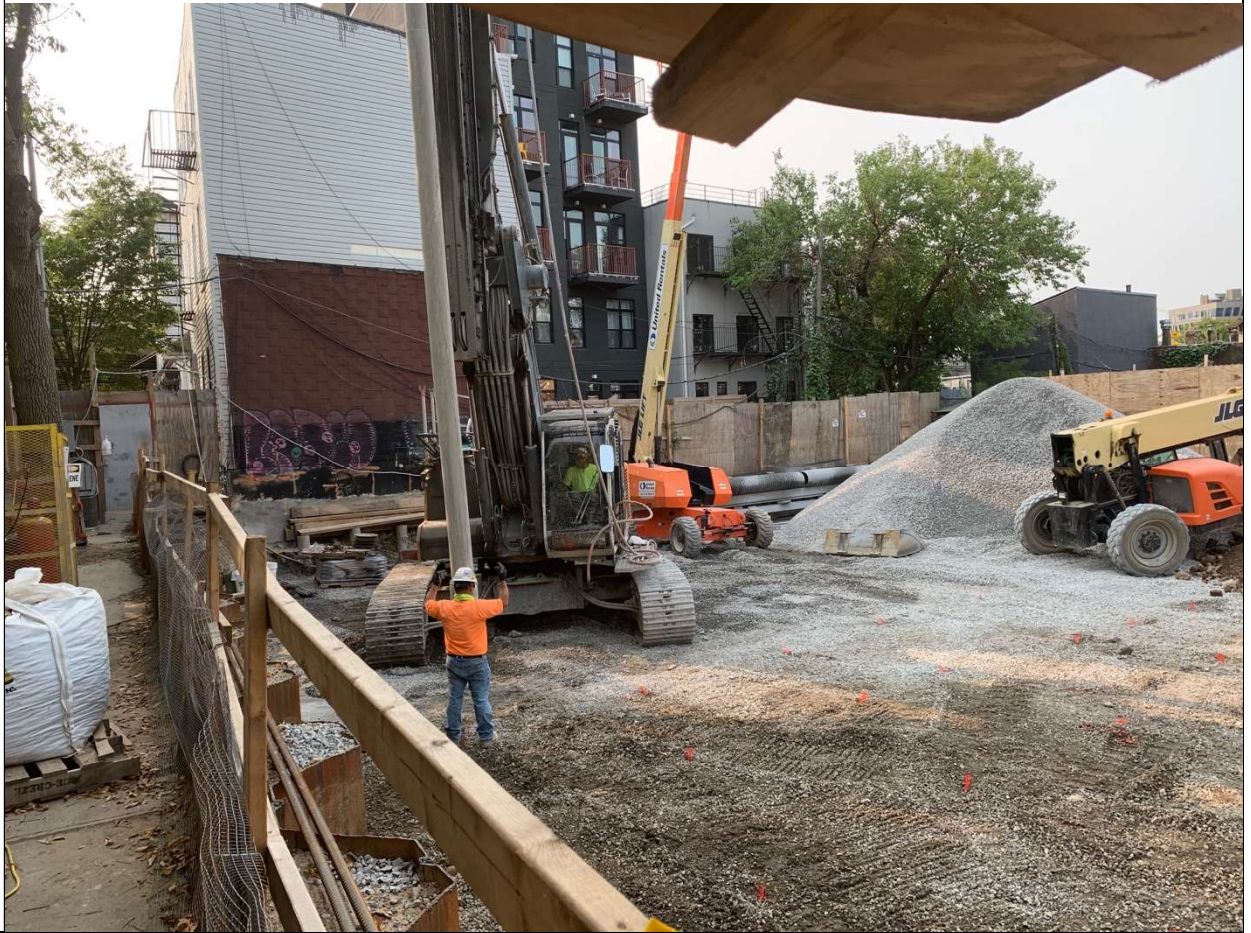
Photo 3 – A look at the driller being directed to the proper point for execution of drilling.
