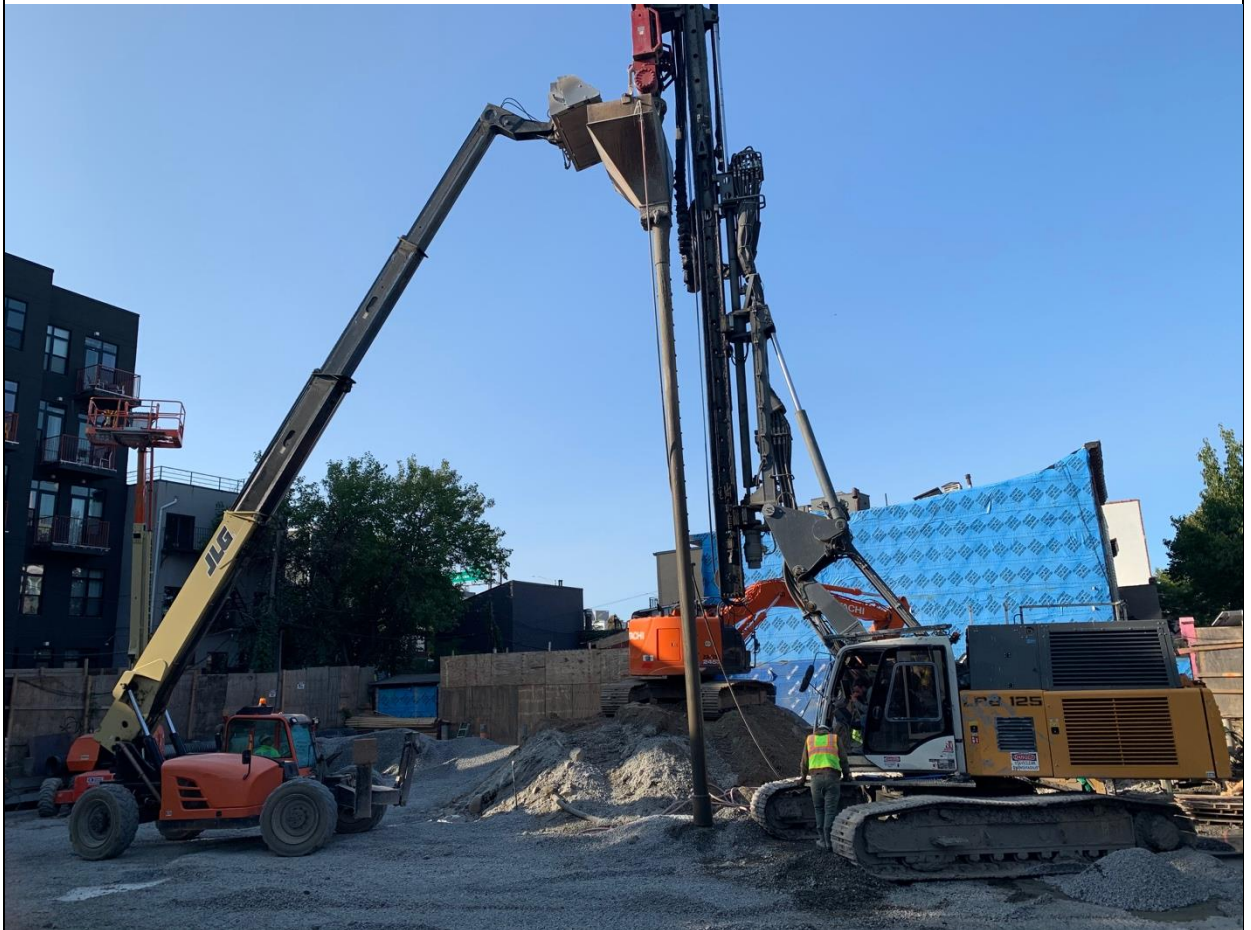
Photo 4 – A look at drilling that was occurring in grid B2, at around 9:30 a.m. Gravel is being put into the driller.
