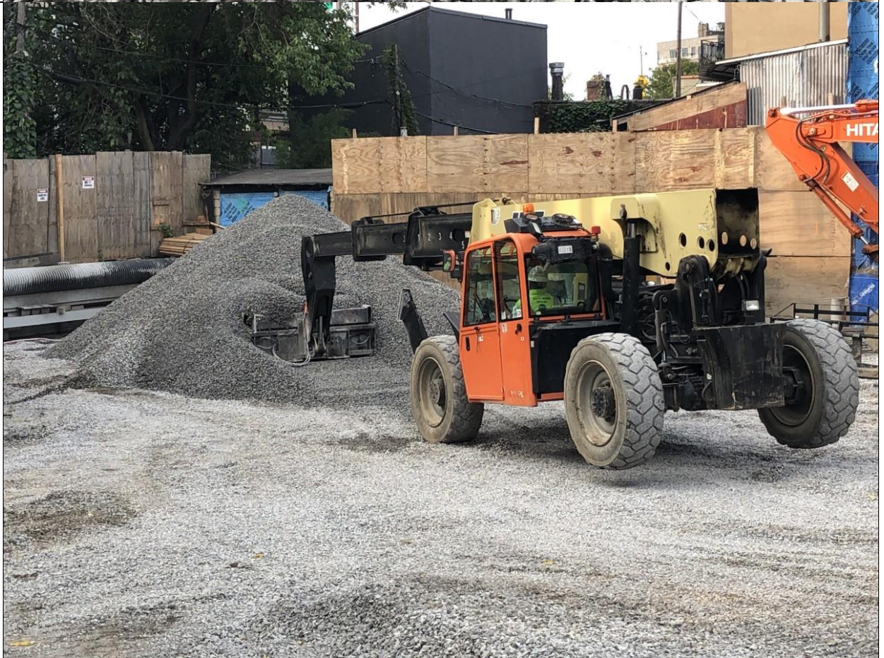
Photo 4 – Moncon spreading and stockpiling gravel with a JLG Telehandler for construction mixing. Grid A3 corner of site.
