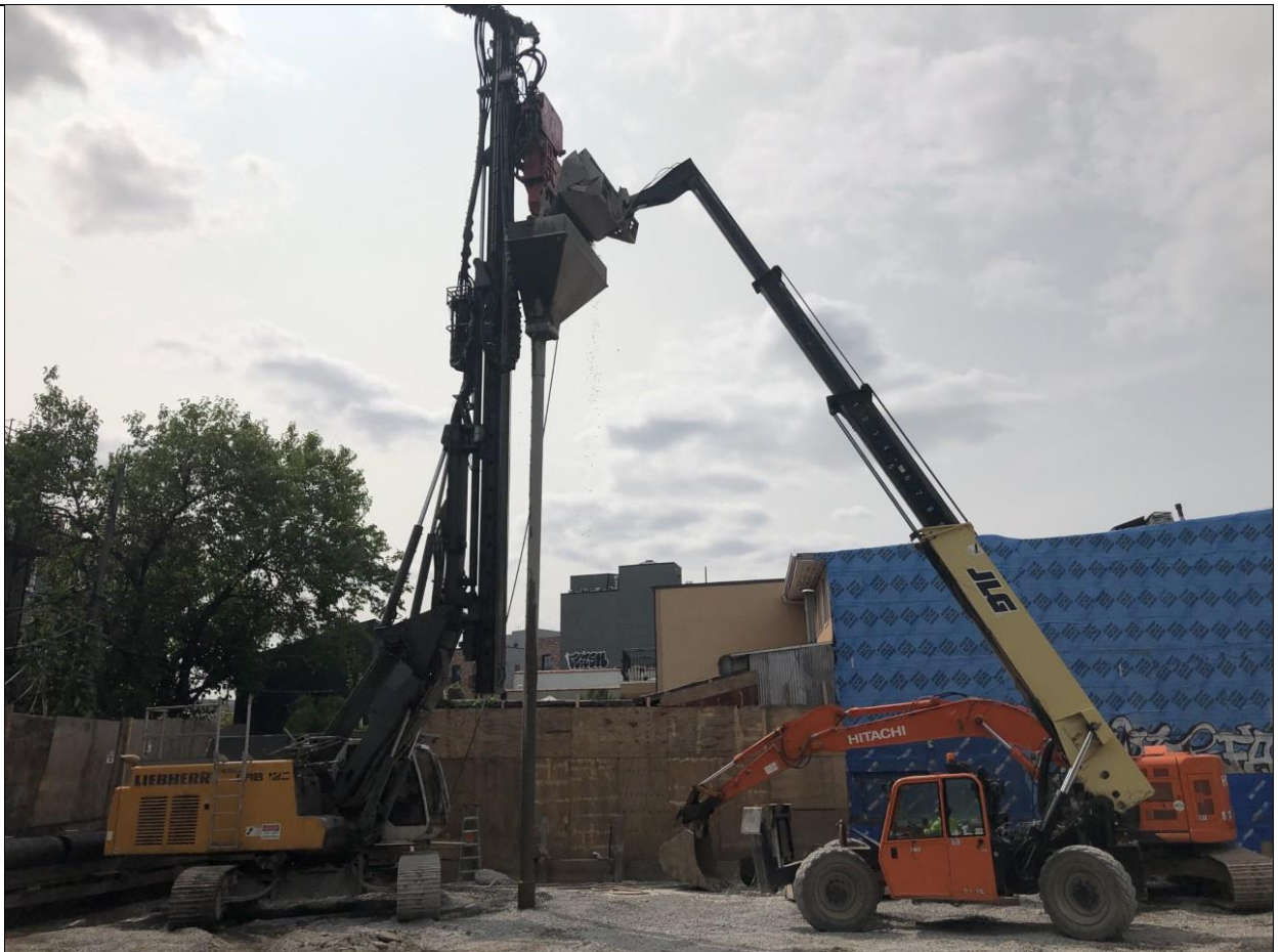
Photo 3 – View of hopper being loaded with gravel for stabilization pile construction on Grid A3. View is facing south west from Graham Avenue.
