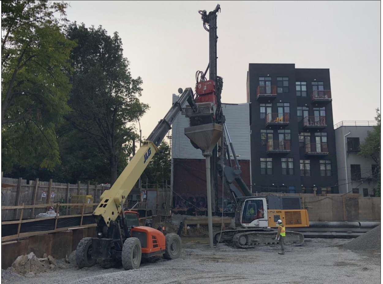
Photo 5 – View of hopper being loaded with gravel for stabilization pile construction on Grid A3. View is facing south east from Graham Avenue.
