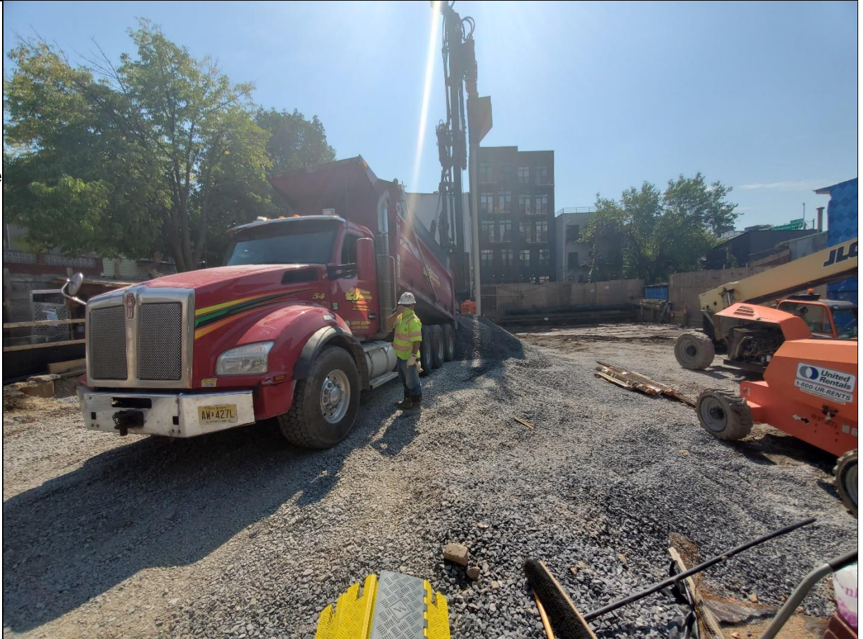
Photo 2 – Truck unloading 3/4" gravel for soil improvement micropile installation, view is facing south from site entrance on Bayard St.
