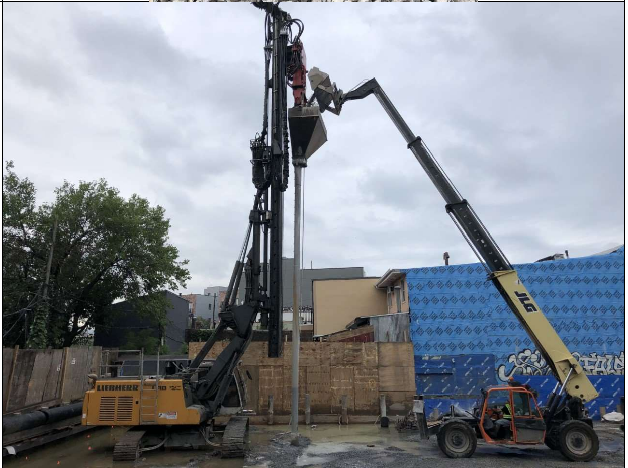
Photo 4 – View of hopper being loaded with gravel for stabilization pile construction on Grid A3. View is facing south west from Graham Avenue.
