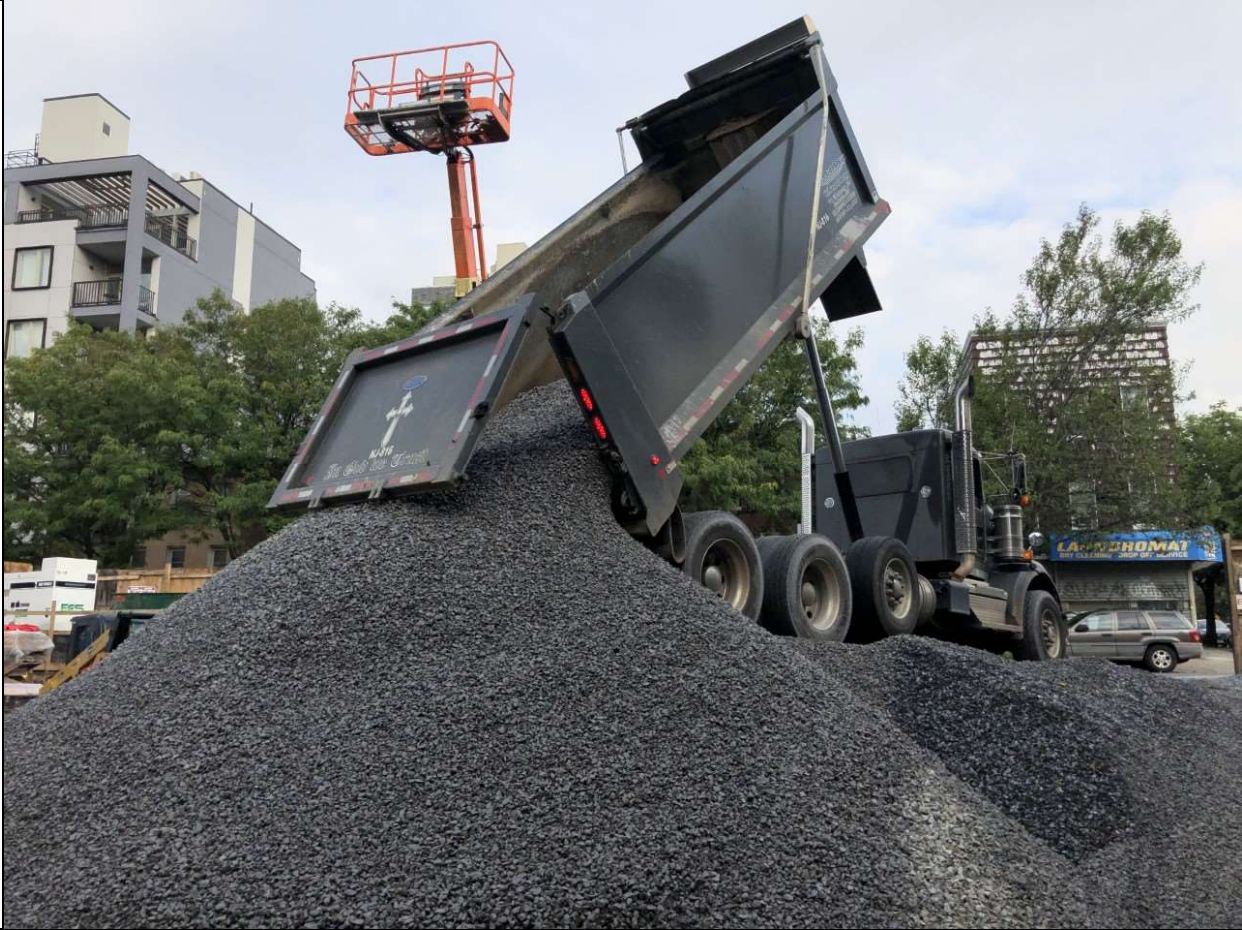
Photo 2 – Truckload of gravel being imported for construction mixing with grout. Grid B1 corner of site.
