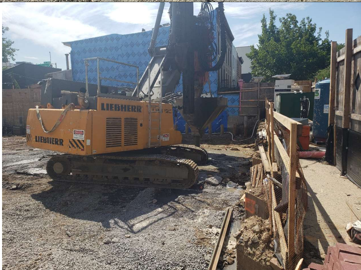
Photo 3 – View of drilling and grouting of micropiles in grid A1
