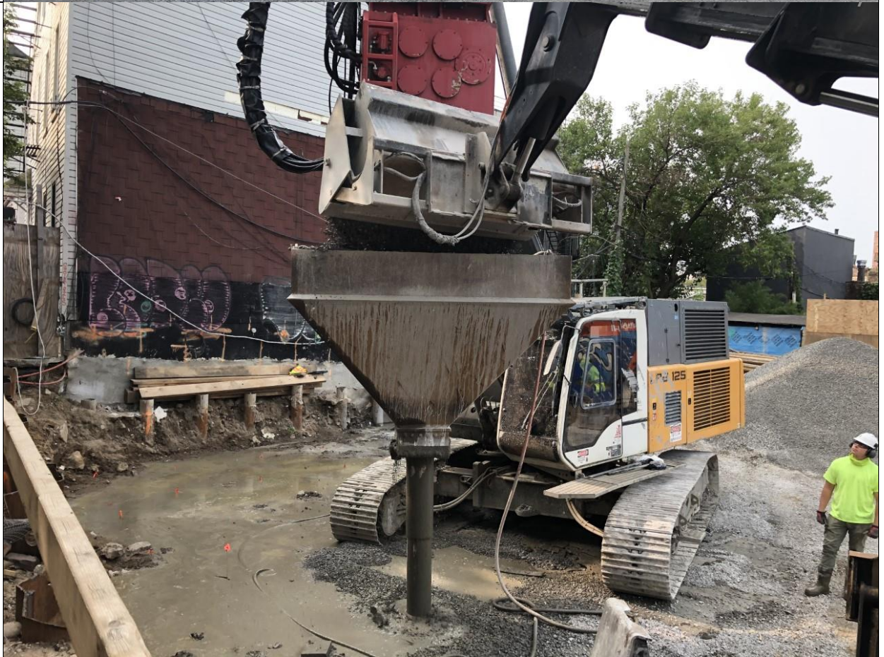
Photo 6 – Alternate view of stabilization piles being made with gravel and grout. View is facing south from Graham Avenue.
