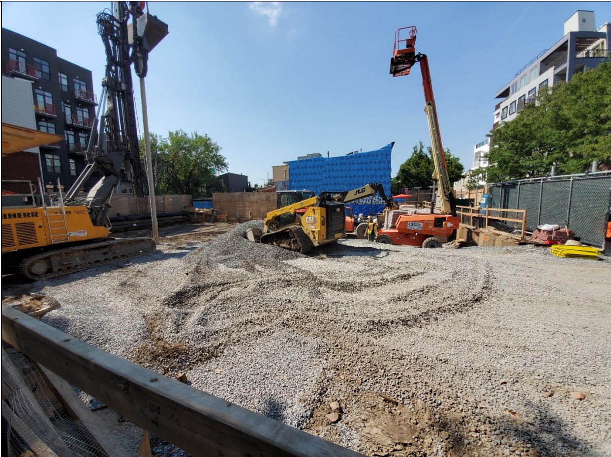
Photo 3 – ¾" gravel import being spread in Grids A1 and B1, view is facing west towards neighboring property on Bayard St.
