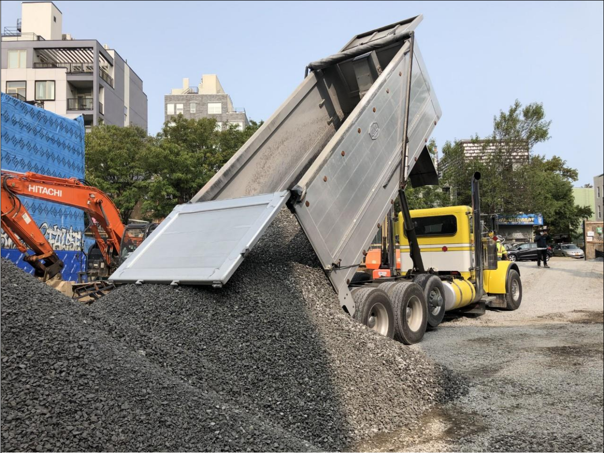
Photo 2 – Truckload of gravel being imported for construction mixing with grout. Grid A3 corner of site.
