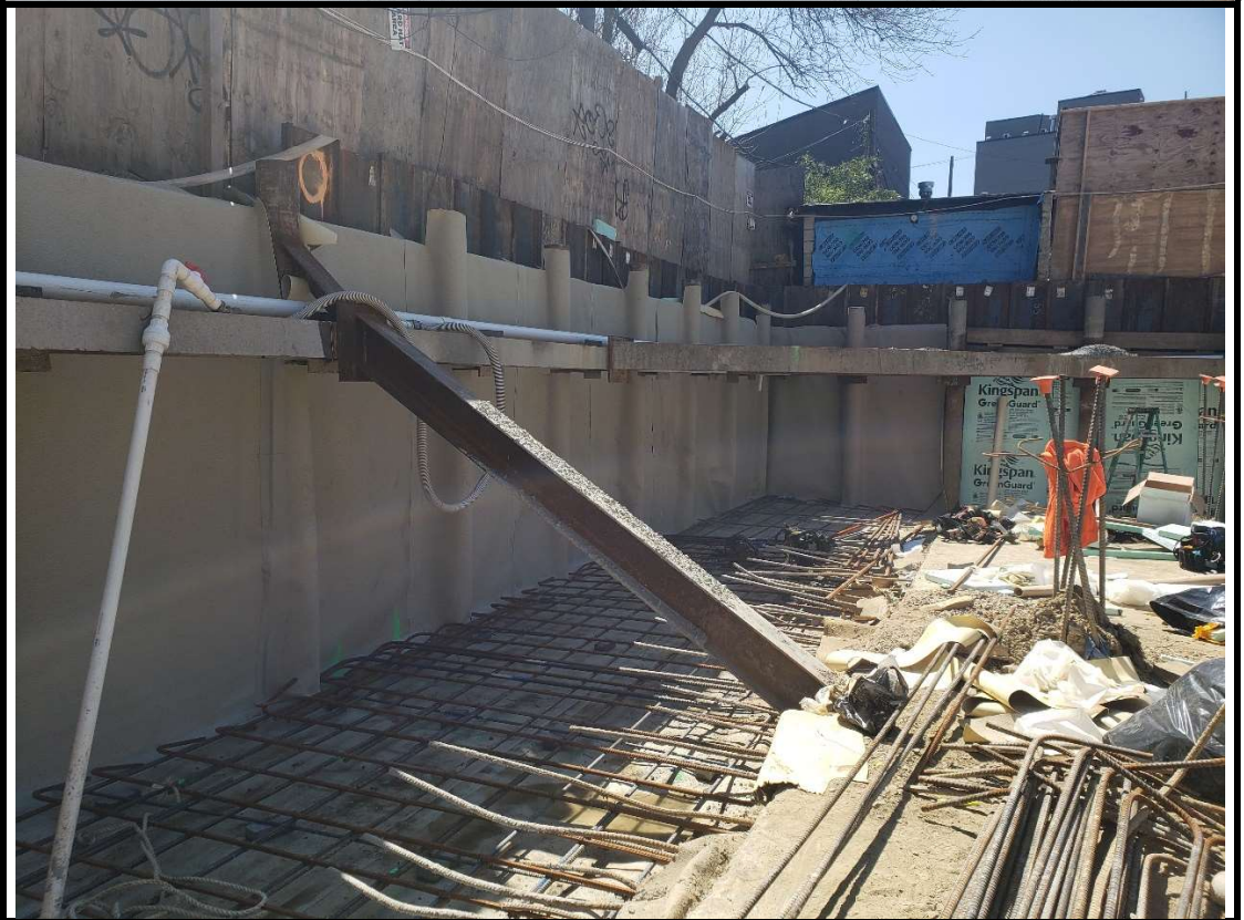
Photo 4: Rear wall in grid A3, installation still in progress
