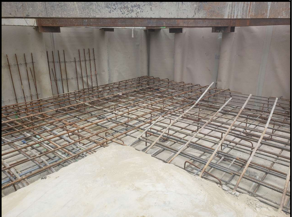
Photo 2: Sikaproof A+12 installation, southwest corner
