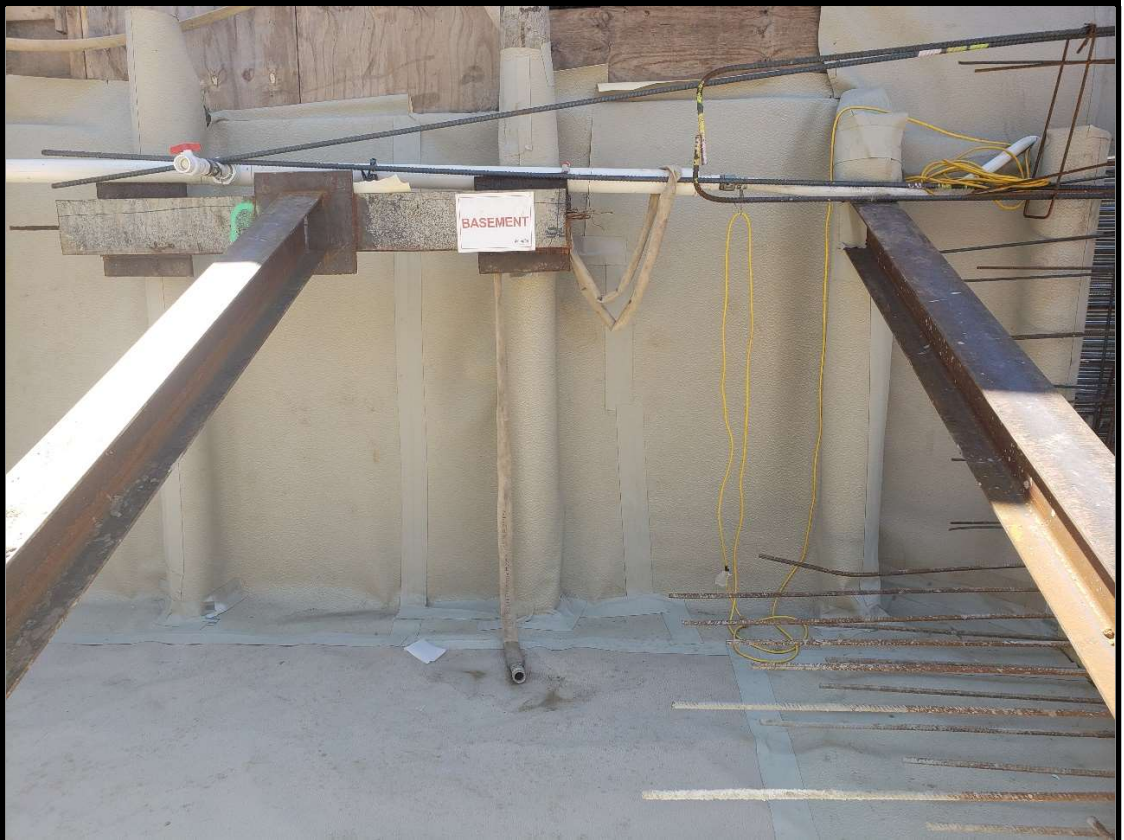
Photo 3: Installation of SikaProof A+12 for west footing and west wall in grid A3
