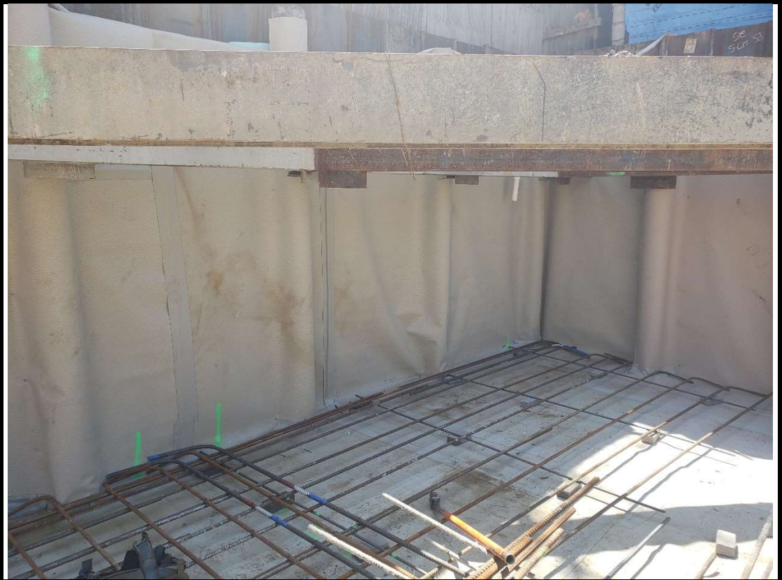
Photo 2: Sikaproof A+12 installation, southwest corner
