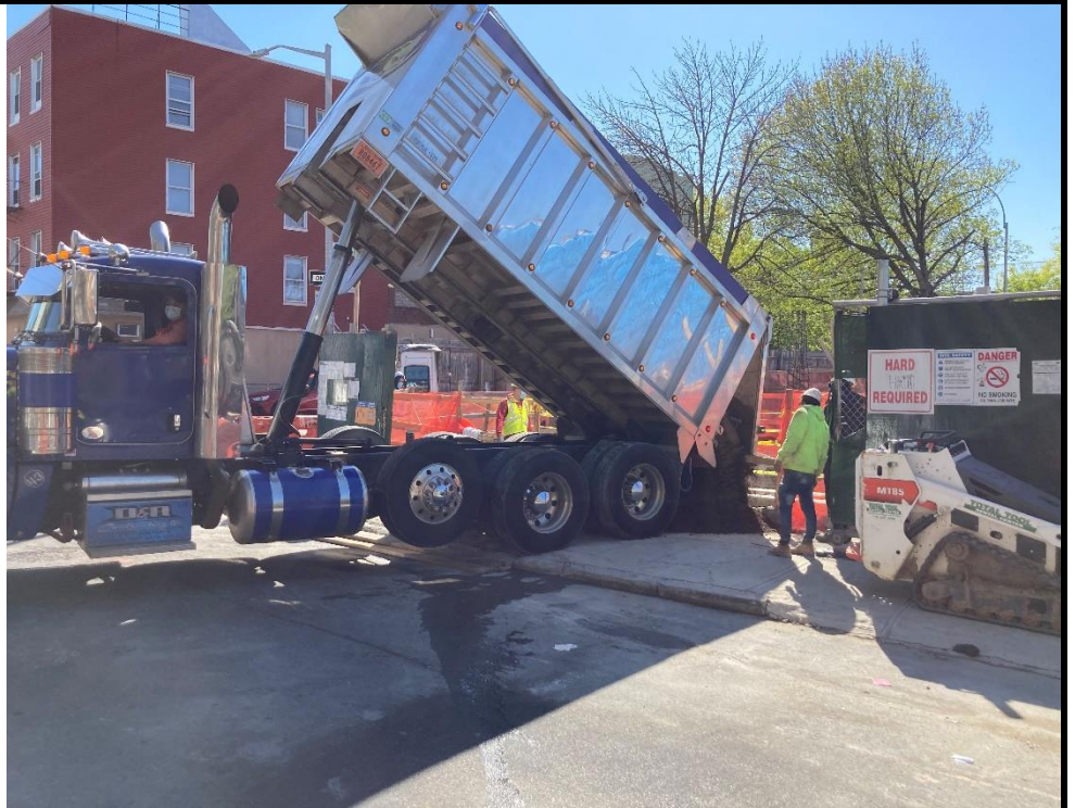
Photo 3: Offloading clean fill for backfill
