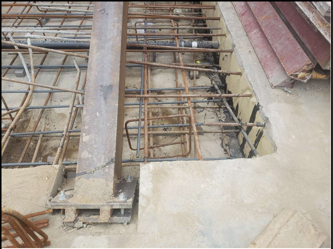
Photo 1: View of SikaProof A+12 connected to waterproofing below Mat slab, west area of grid A3
