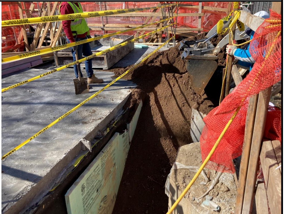
Photo 4: Spreading backfill onsite.
