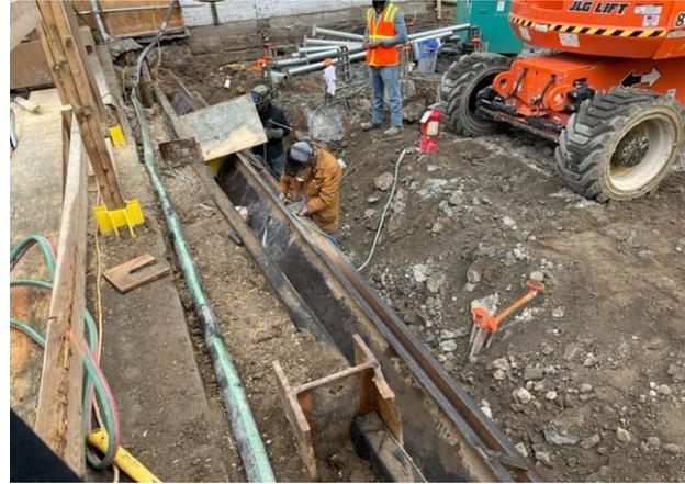
View of welding brackets and clamps to the south welders.
