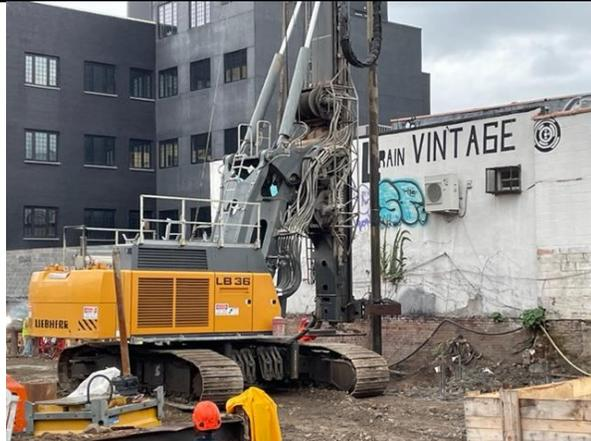
View of New Leaf drilling for pile production on the western side of the site.
