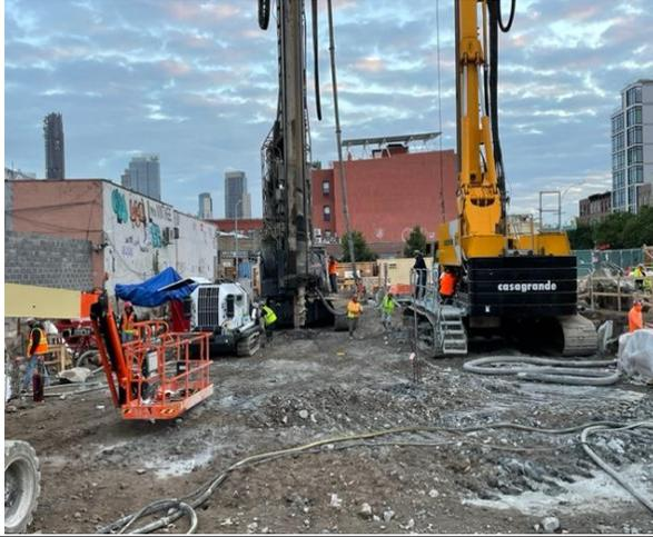
View of tie back installation on the south boundary wall.
