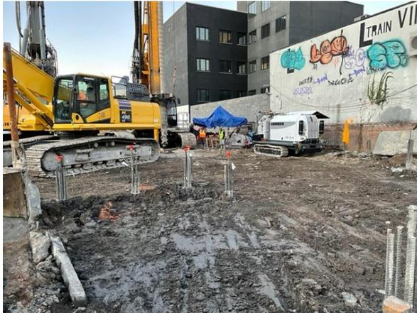
View of installed tie backs on the south boundary wall.
