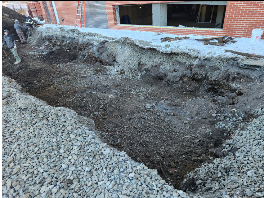
Photo 3: View of excavation to accommodate dry well installation.
