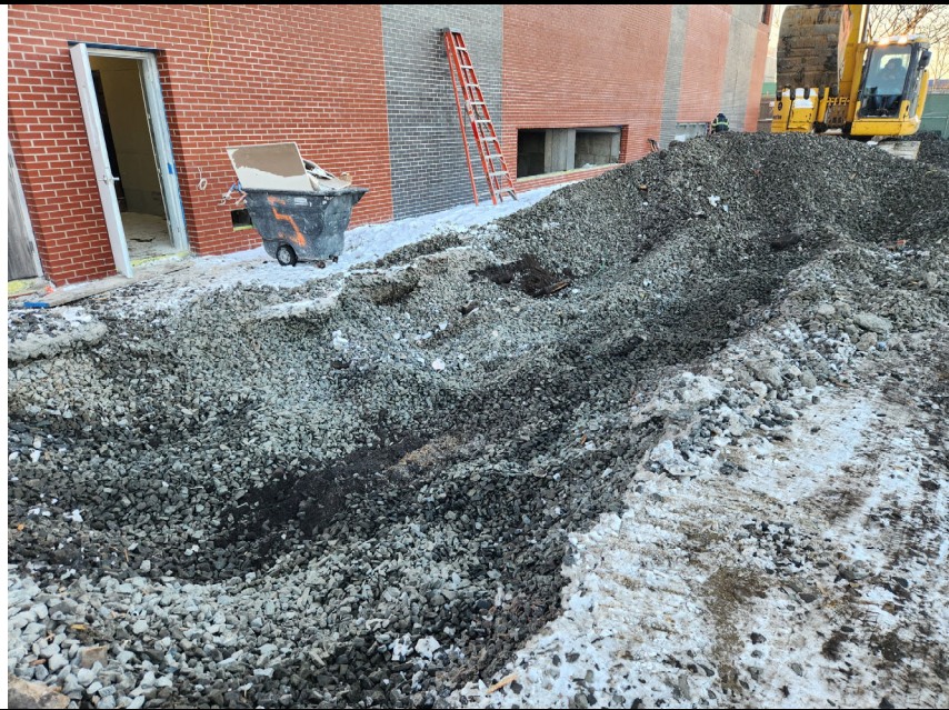
Photo 1: View of excavation to accommodate dry well installation.
