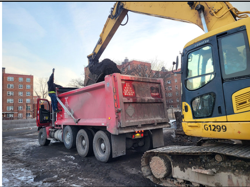
Photo 1: View of soil being loaded into a truck for offsite disposal.
