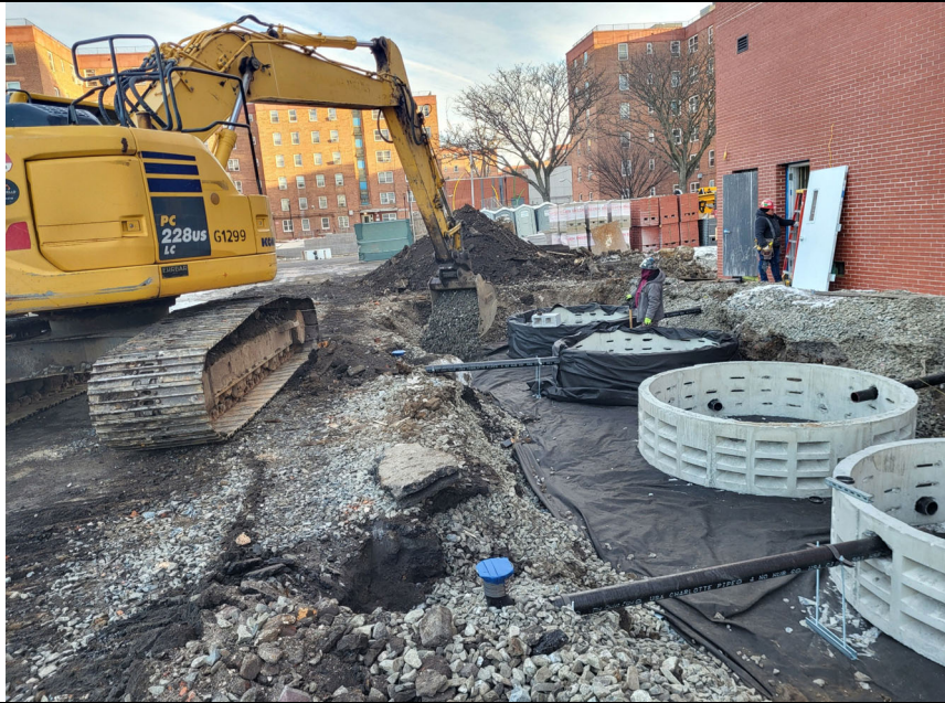
Photo 3: View of backfill with clean stone.
