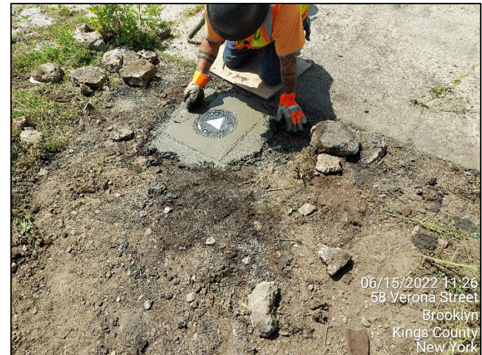
Photograph 4: Installation of flush-mounted well cover at a newly installed monitoring well in the western portion of the Site. (June 2022)
