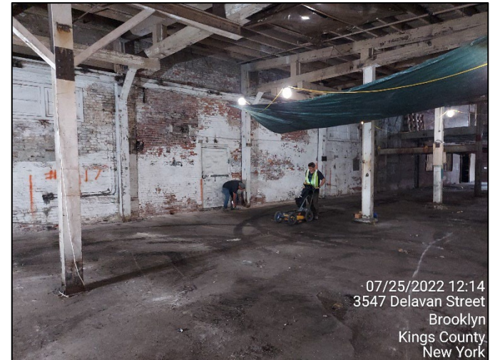
Photograph 14: Completion of a geophysical survey across accessible portions of the Site. (July 2022)
