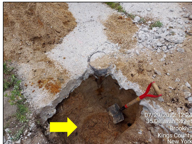
Photograph 22: Confirmation of an UST at the magnetic anomaly that was identified in the concrete lot in the western portion of the Site. (July 2022)
