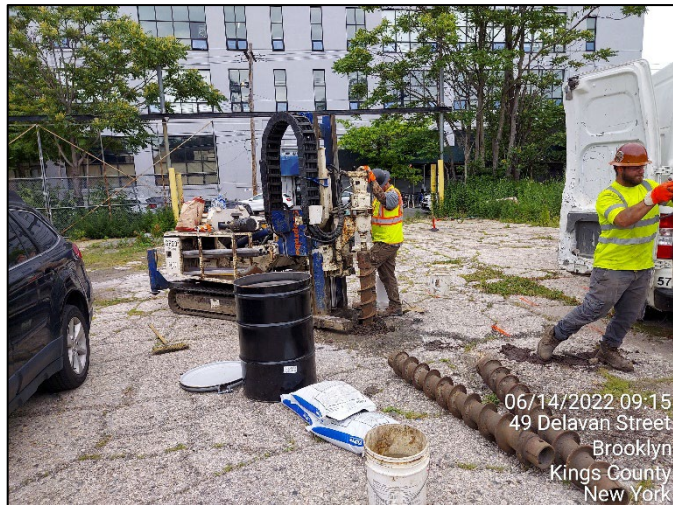
Photograph 3: Installation of a groundwater monitoring well in the western portion of the Site. (June 2022)
