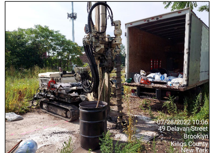
Photograph 16: Installation of groundwater monitoring well in the northwestern portion of the Site. (July 2022)
