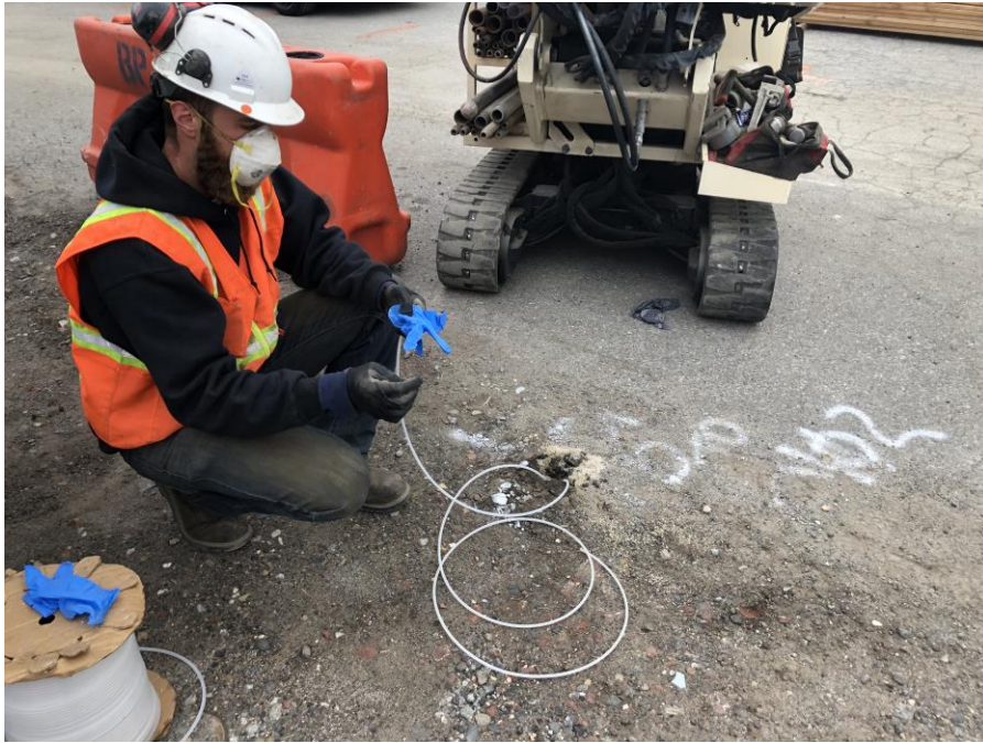
Photo 5, 5/08/2020: View of Eastern installing soil vapor point SV02, facing east.
