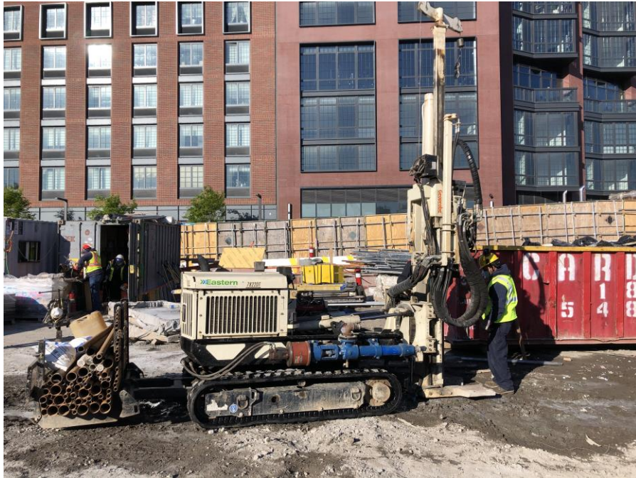
Photo 11, 5/13/2020: View of Eastern drilling soil boring LB16, facing west.
