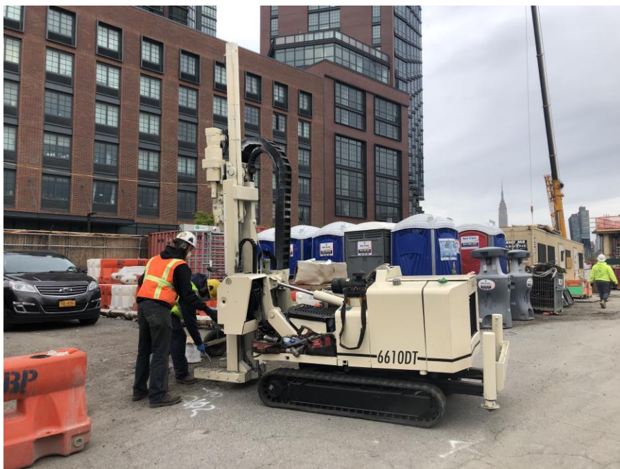
Photo 4, 5/08/2020: View of Eastern installing soil vapor point SV02, facing northwest.
