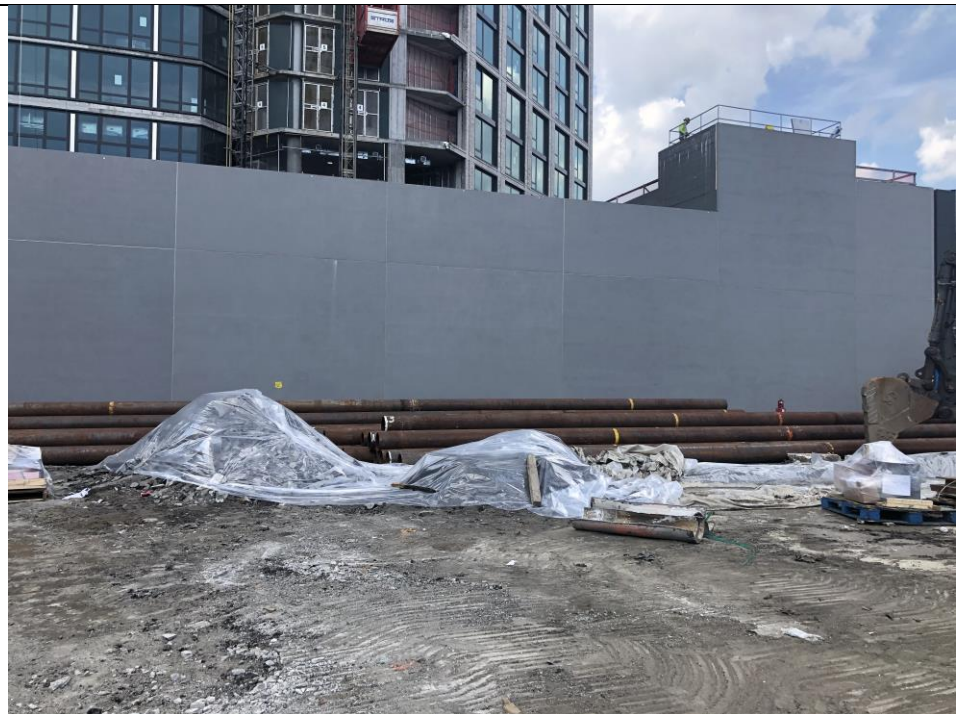
Photo 4: View of segregated soil and asphalt stockpiles covered with polyethylene sheeting located in COMP J North (facing north).
