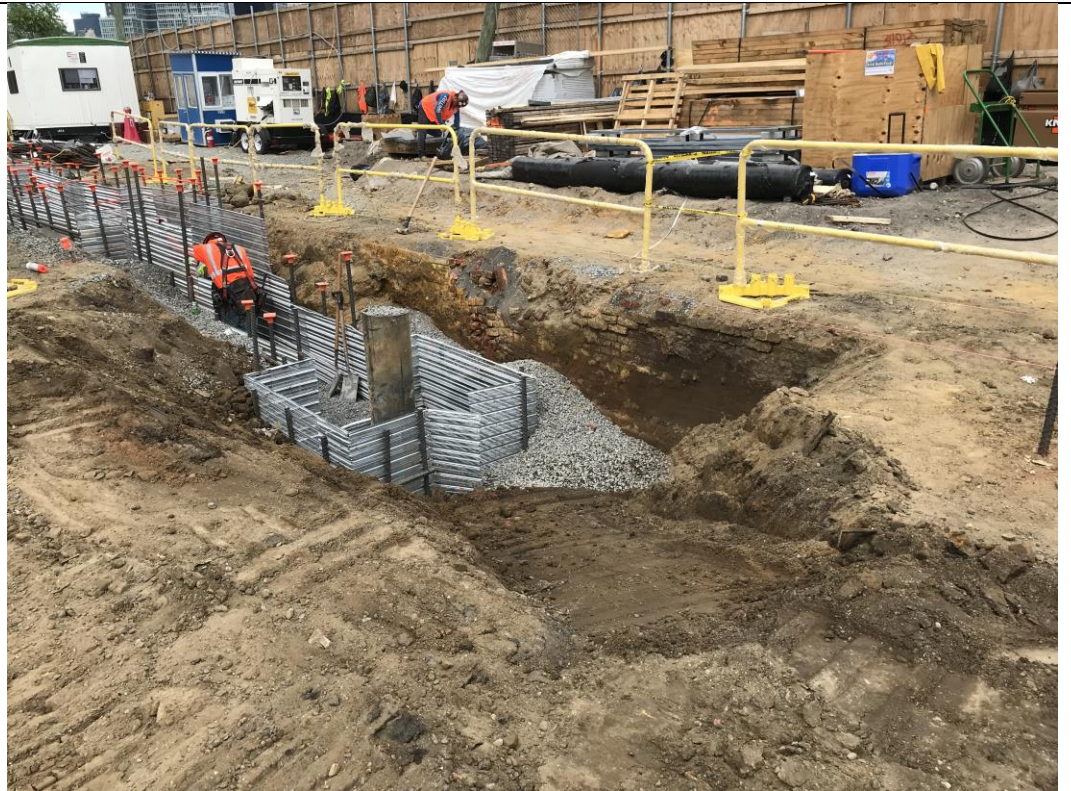
Photo 2: View of STNY backfilling with of 0.75-inch virgin stone in waste characterization grid COMP A (facing east).
