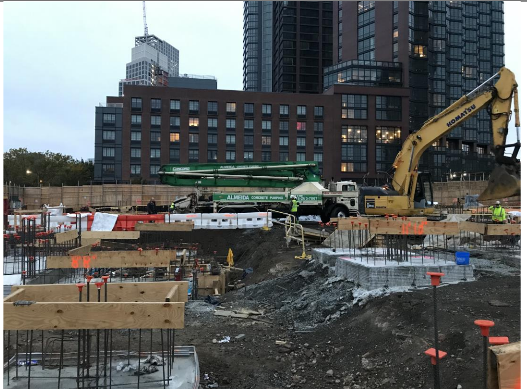
Photo 1: General view of the site (facing west)
