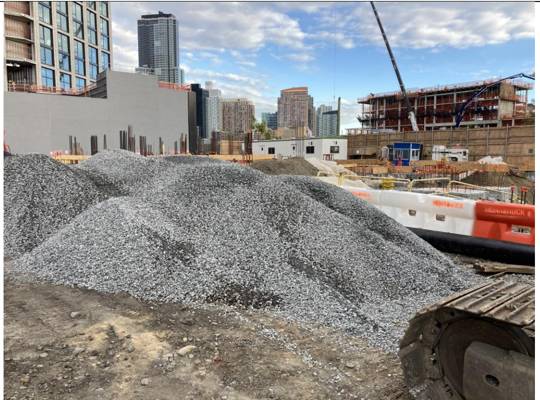
Photo 2: View of imported 0.75-inch stone stockpile located in waste characterization grid COMP J North (facing northeast).
