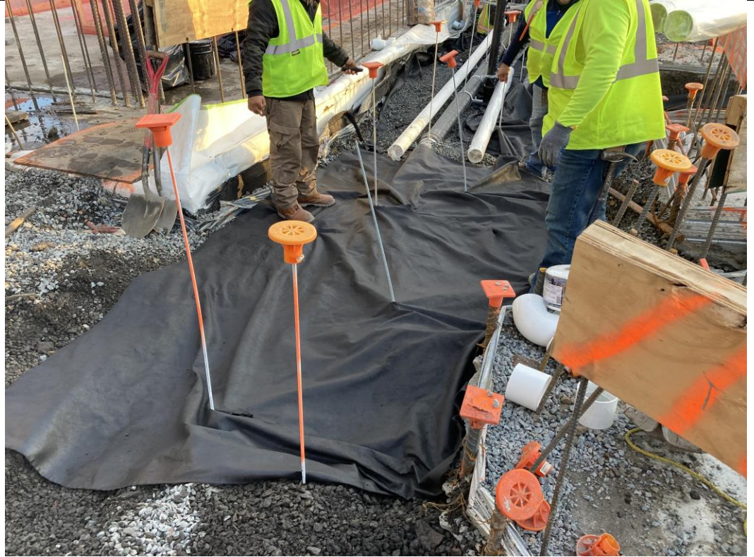
Photo 3: View of STNY placing geotextile fabric in waste characterization grid COMP D (facing east).
